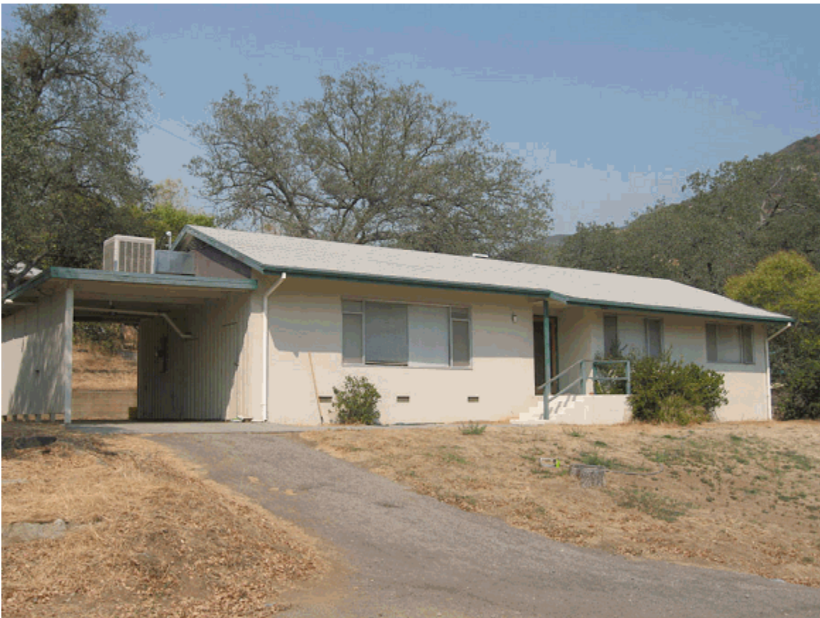
Buildings and Structures #4: Mission 66 era structure (bldg. #1405) at Buckeye, constructed in 1959. This building is representative of all Mission 66 residences at Buckeye since they were all constructed using the same design. (SEKI, 2008)
