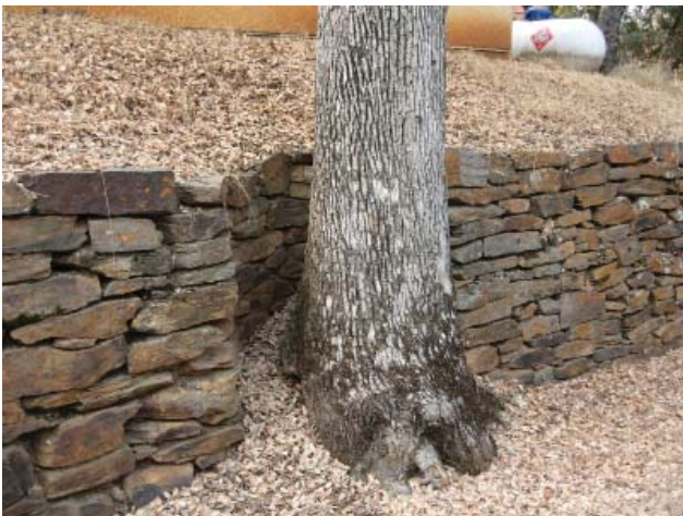
Ash Mountain Schist Retaining Wall (Contributing)
