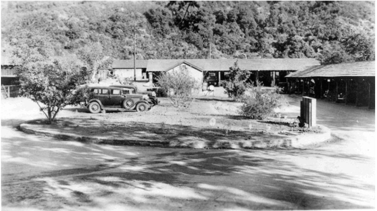
Physical History #7: Maintenance yard after landscaping improvements by CCC workers, 1937. The service station (#168) visible in the center of the photo and the most distant building, (#159), are extant (SEKI Archives, negative 3054).
