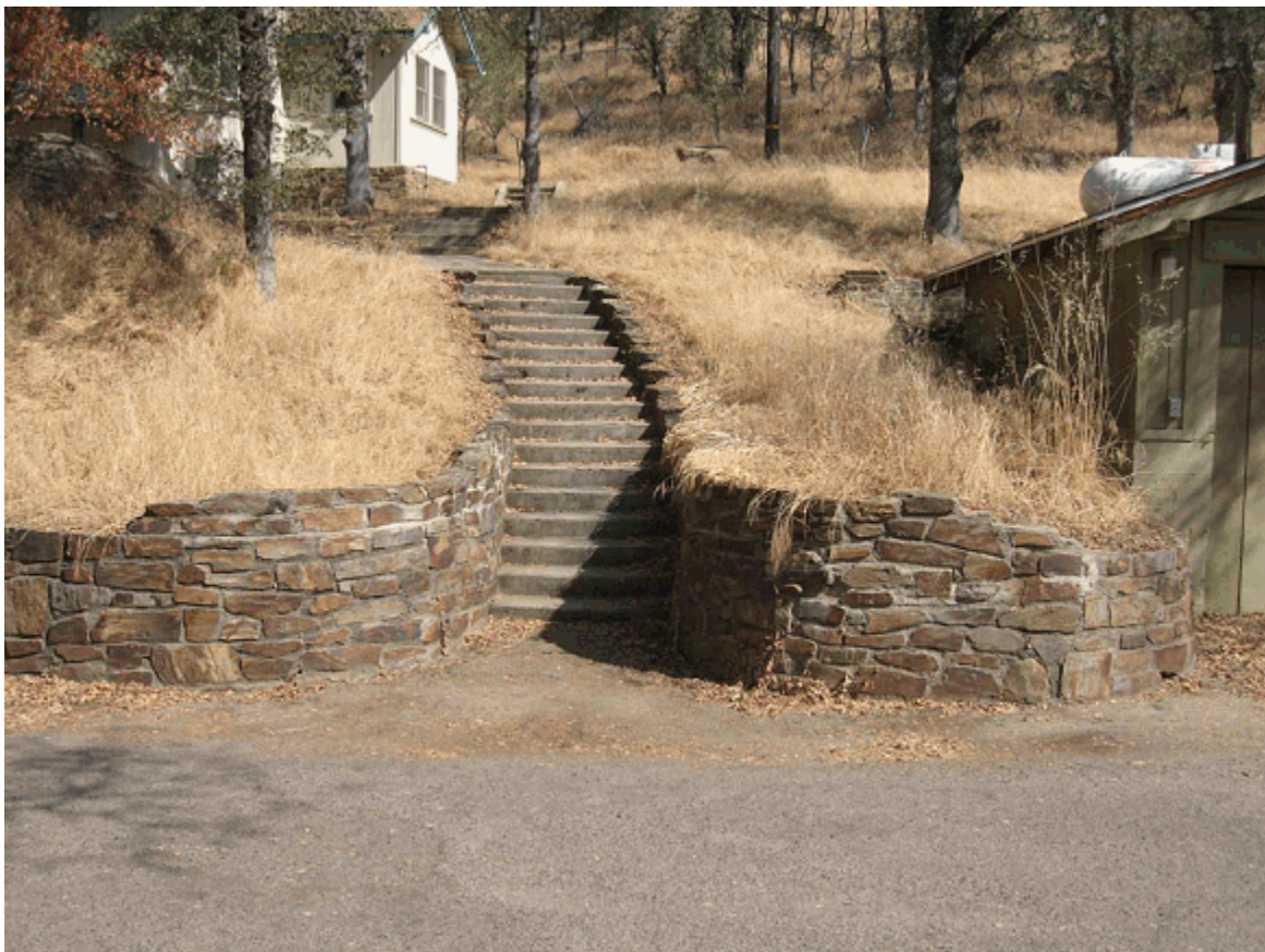
Small Scale Features #1: Schist retaining wall and stairway leading up to bldg. # 93. Notice how the retaining wall creates a level platform for the garage and seamlessly ties into the stairway. (SEKI, 2008)
