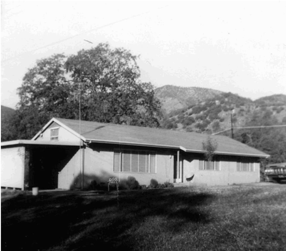
Physical History #10: Photo from 1961 of residence #1409 at Buckeye Residential Area. This building was constructed in 1959 as part of Mission 66 and remains largely unchanged (SEKI Archives, building files).
