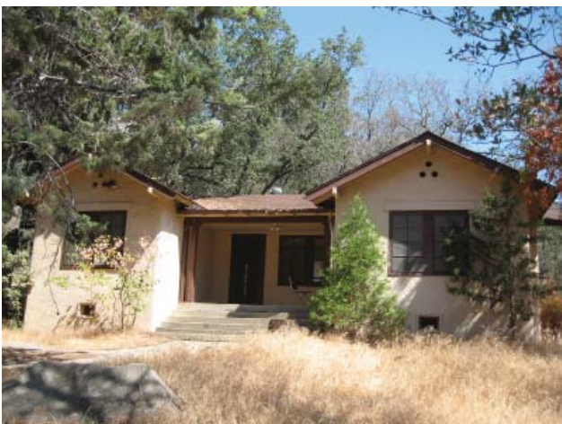
Ash Mountain Exercise and Laundry House/ Residence #15 (Contributing)
