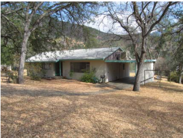
Buckeye Residence #1414 (Contributing)
