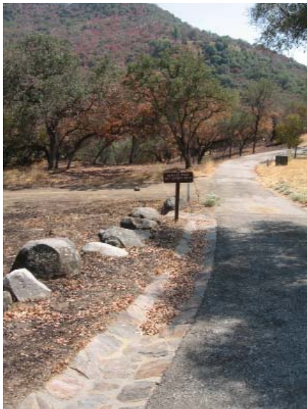
Research Loop Road with Schist Gutter (Contributing)
