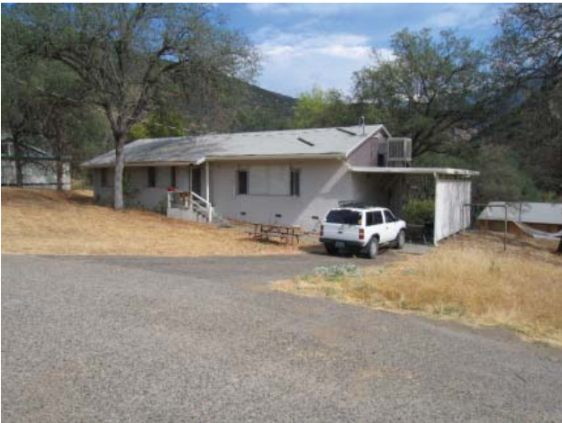
Buckeye Residence #1412 (Contributing)
