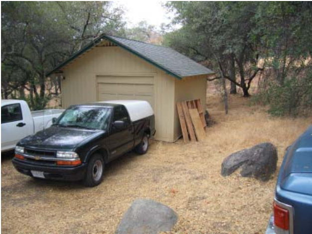
Ash Mountain Garage for Residence #18A (Noncontributing)
