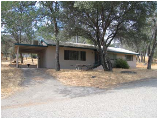
Buckeye Residence #1401 (Contributing)
