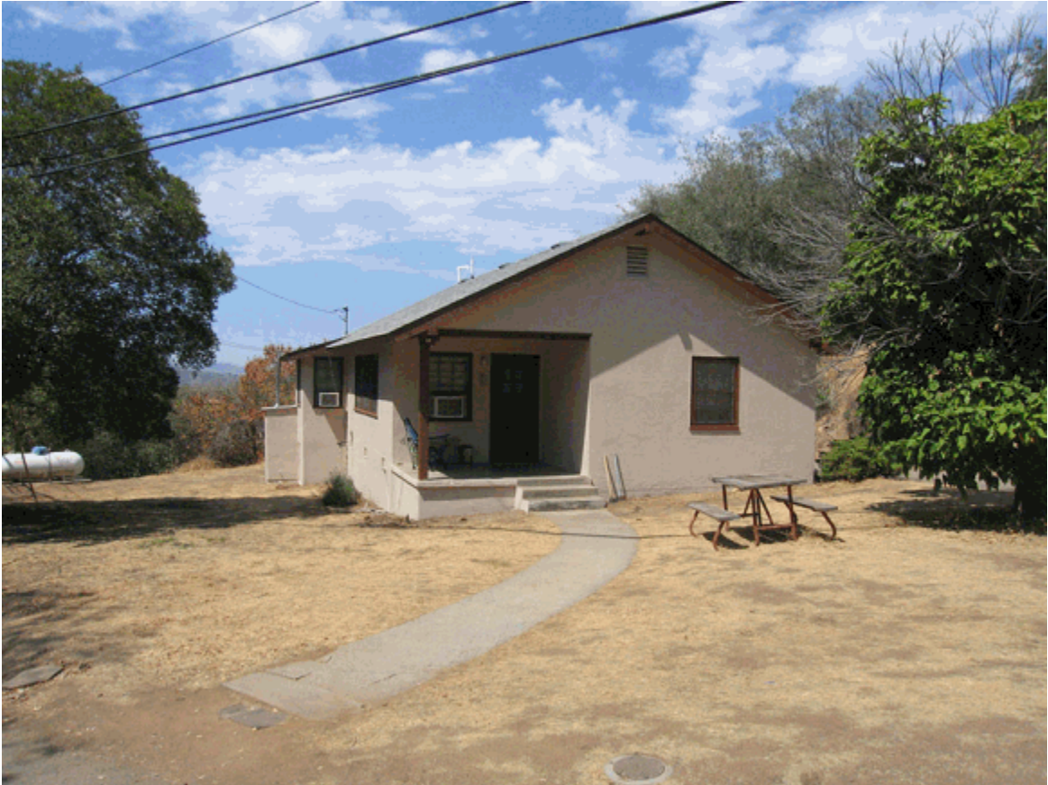
Buildings and Structures #2: CCC-constructed residence (bldg. #95) within Ash Mountain, built in 1941. This structure retains its original stucco exterior. (SEKI, 2008)
