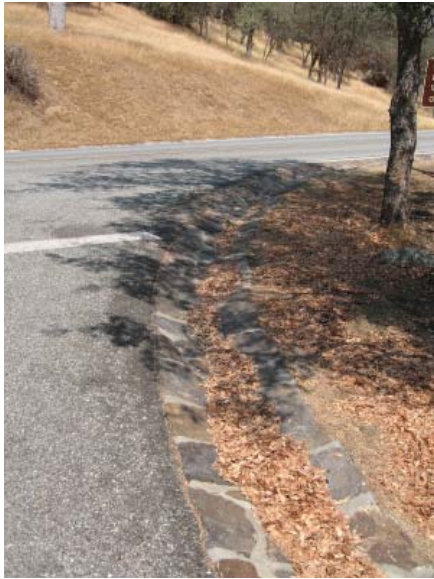
Ash Mountain Schist Gutter ( Contributing )
