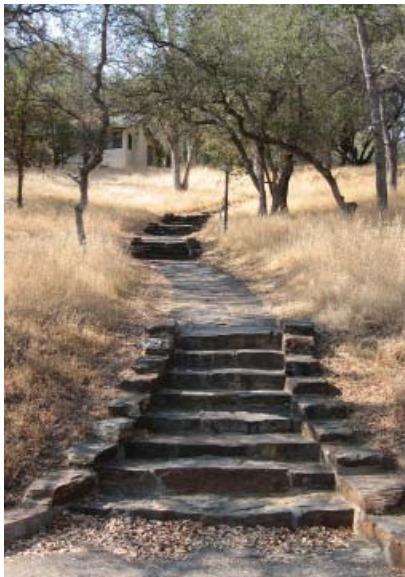
Ash Mountain Schist Stairway ( Contributing )
