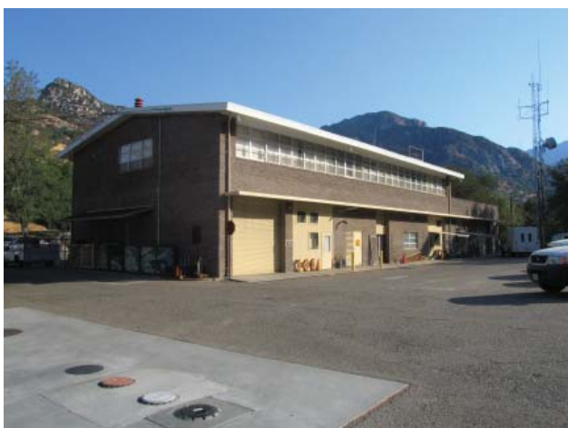
Ash Mountain Fire Control Building/ Fire Dormitory (Contributing)
