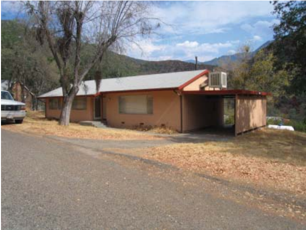
Buckeye Residence #1404 (Contributing)
