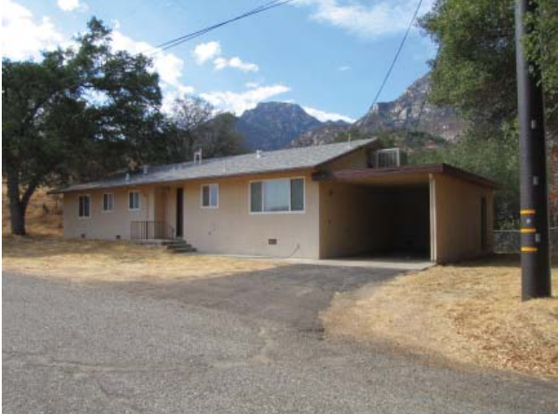
Buckeye Residence #1420 (Contributing)
