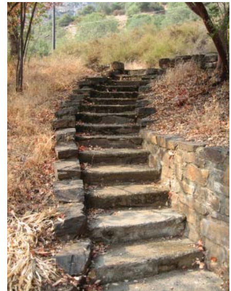
Ash Mountain Schist Stairway ( Contributing )
