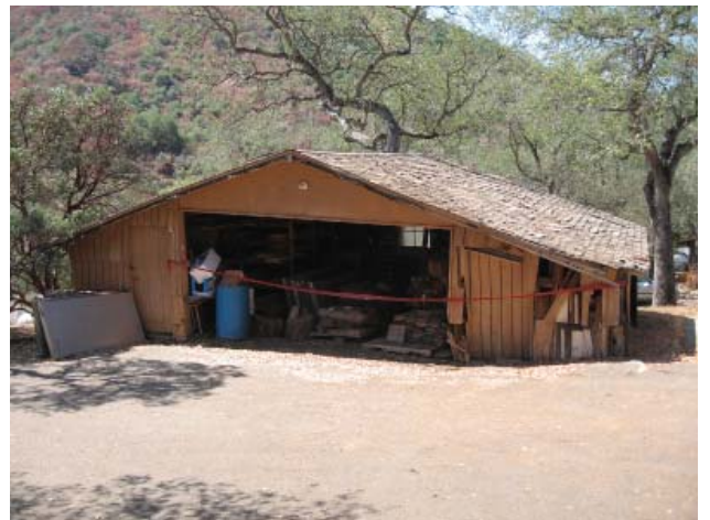
Ash Mountain Garage for Residence #5 and #7 (Contributing)
