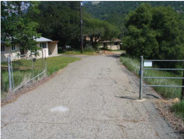
Sierra View Lane (Contributing)
