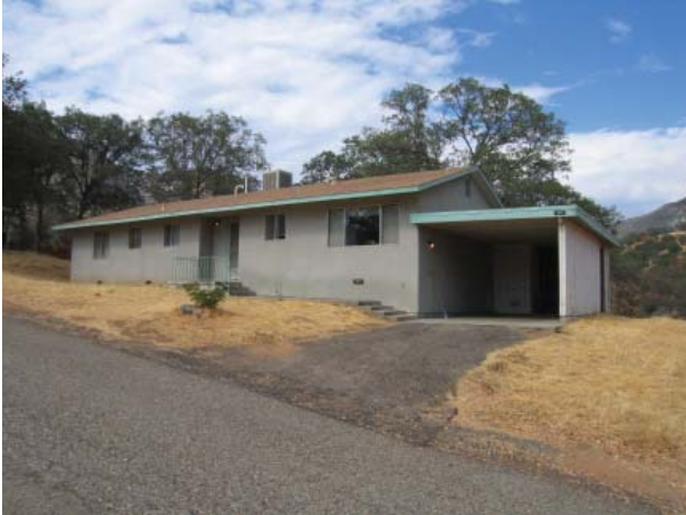
Buckeye Residence #1417 (Contributing)
