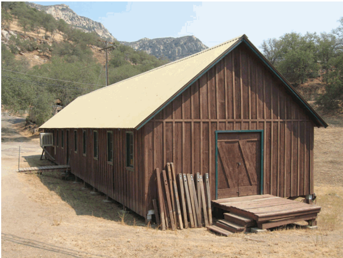
Buildings and Structures #3: This structure (bldg. 140) was the original messhall of the CCC camp at Sycamore. It was built in 1934 and is currently used as a storage building. (SEKI 2008)
