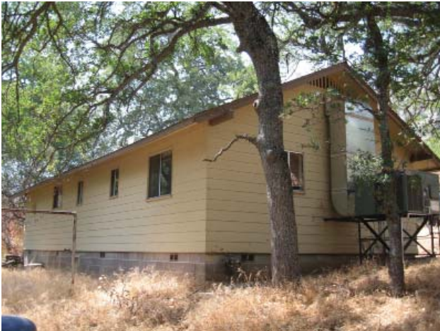
Ash Mountain Residence #6A (Noncontributing)
