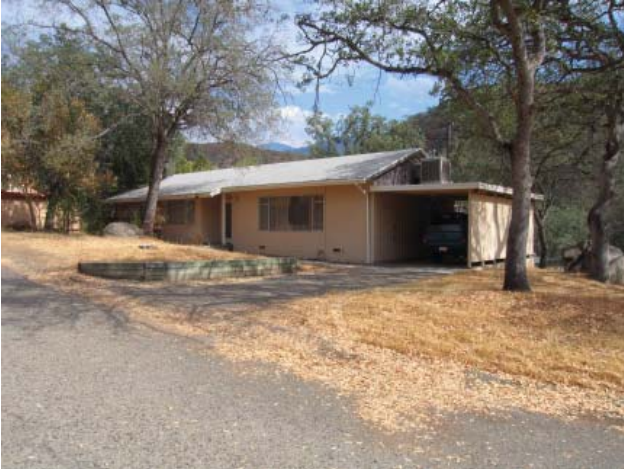
Buckeye Residence #1406 (Contributing)
