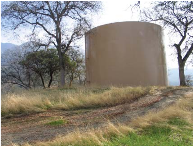
Buckeye Water Tank (Contributing)
