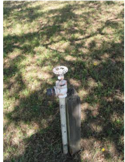
Sycamore Standpipe (Undetermined)
