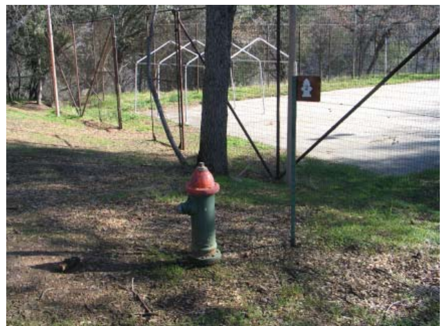
Ash Mountain Fire Hydrant (typical) (Undetermined)
