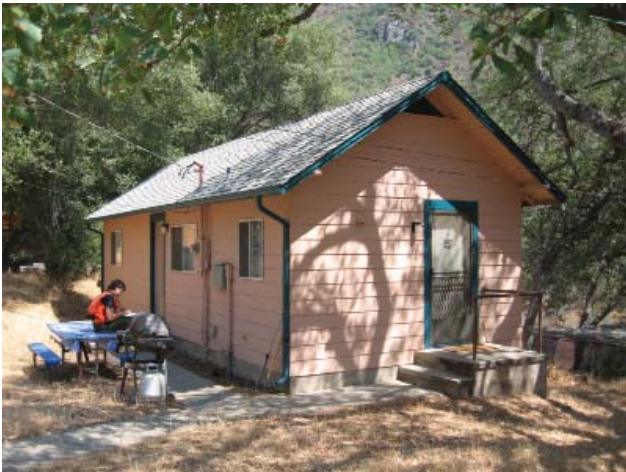
Ash Mountain Residence #17A (Noncontributing)
