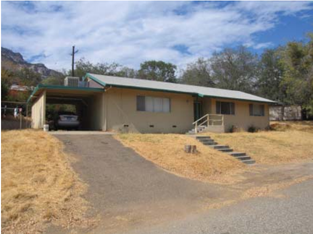
Buckeye Residence #1403 (Contributing)
