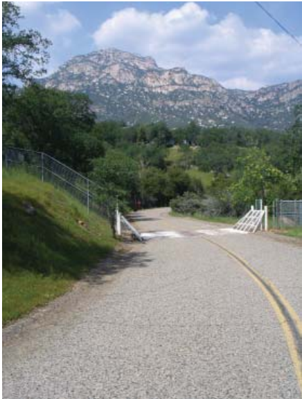
Canyon View Drive (Contributing)
