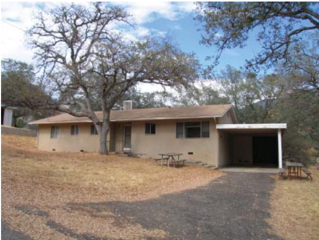
Buckeye Residence #1415 (Contributing)
