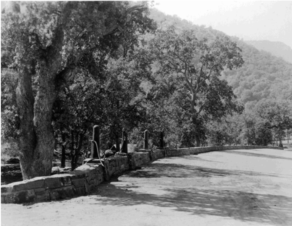
Physical History #5: Generals Highway through Ash Mountain, 1934, near the current visitor center. This rock wall was constructed by CWA workers, which included water pumps and hoses allowing motorists to fill their radiators (SEKI Archives, Box 104).
