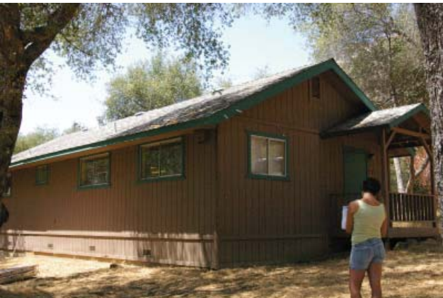
Ash Mountain Residence #10/ Water Laboratory (Noncontributing)
