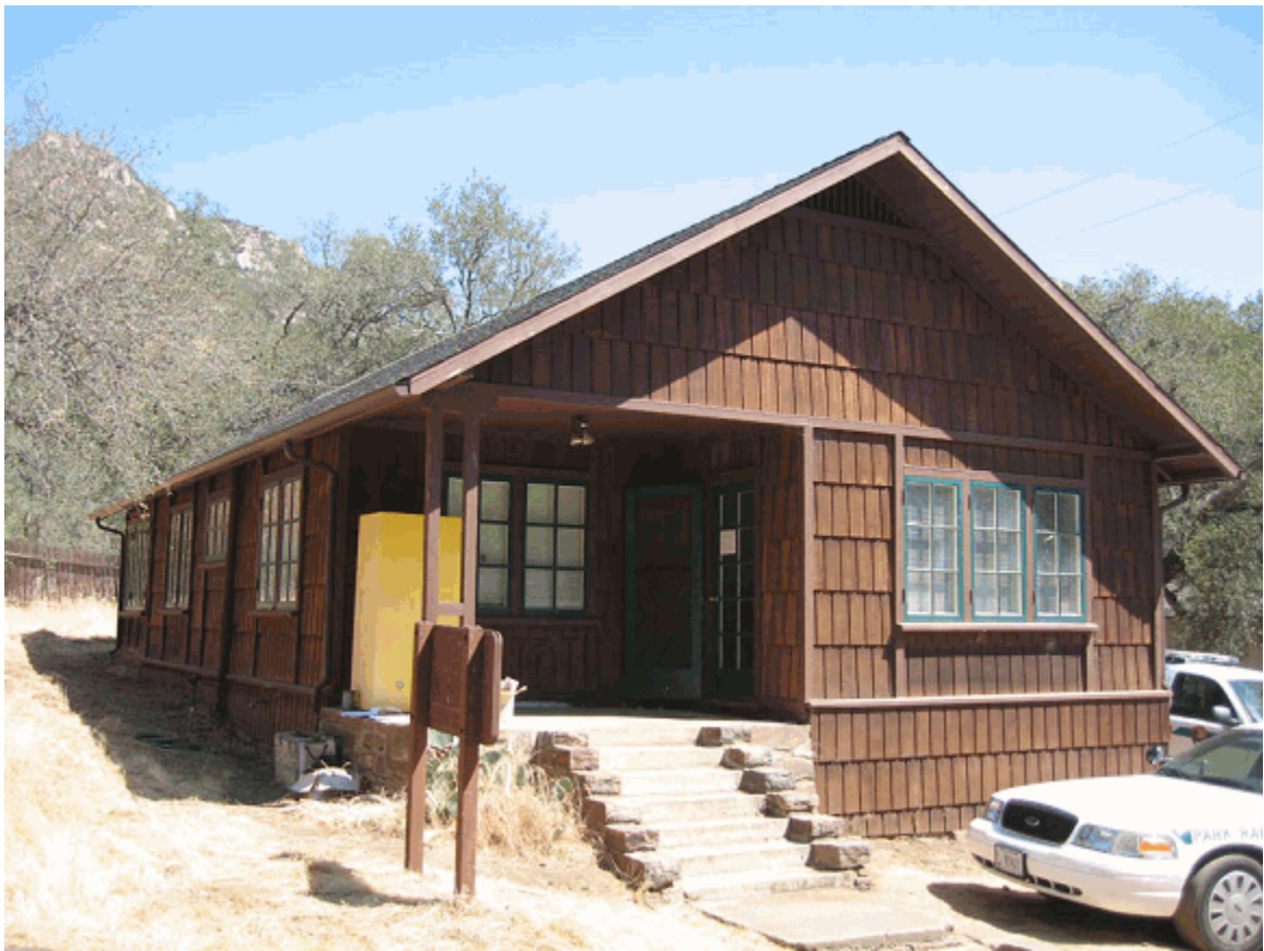
Buildings and Structures #1: Recently rehabilitated residence within Ash Mountain (bldg. #5). Due to recurrent damage from woodpeckers, it was rehabilitated using a cement fiber shingle that replicates the appearance of redwood shake siding. (SEKI 2008)
