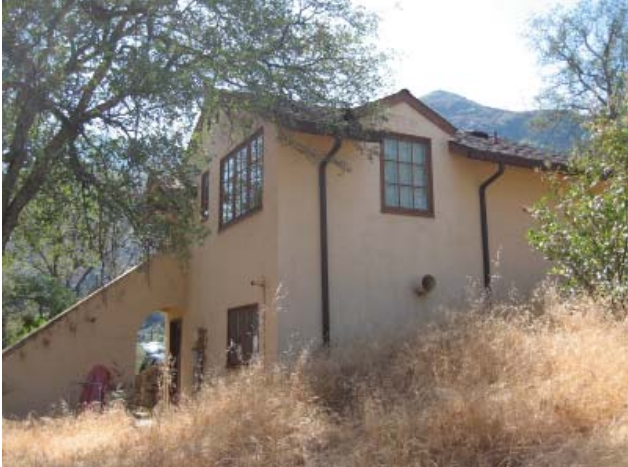
Ash Mountain Garage for Residence #12 Water Lab (Contributing)
