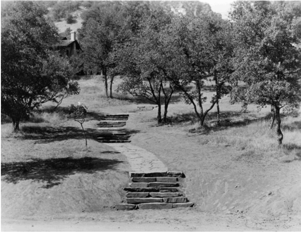
Physical History #6: Photo showing rockwork pathways installed by CWA workers on Mather Drive near residences #14 and #15, 1934 (SEKI Archives, Box 104).
