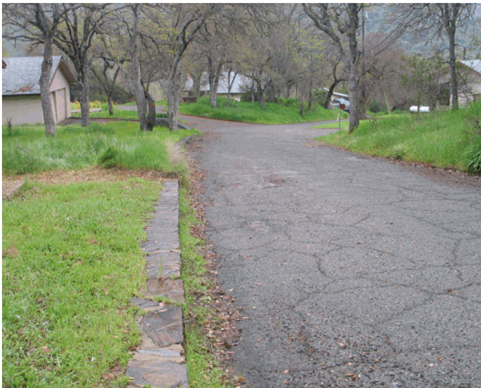
Drury Lane was constructed in the 1920 and 1930s. This road is typical of contributing residential roads in Ash Mountain proper, with a narrow cross-section, curvilinear alignment and schist curbing. (SEKI 2010).
