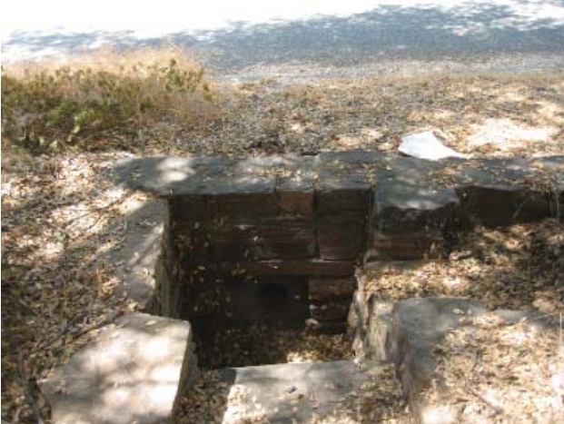
Ash Mountain Schist Drop Culvert (Contributing)
