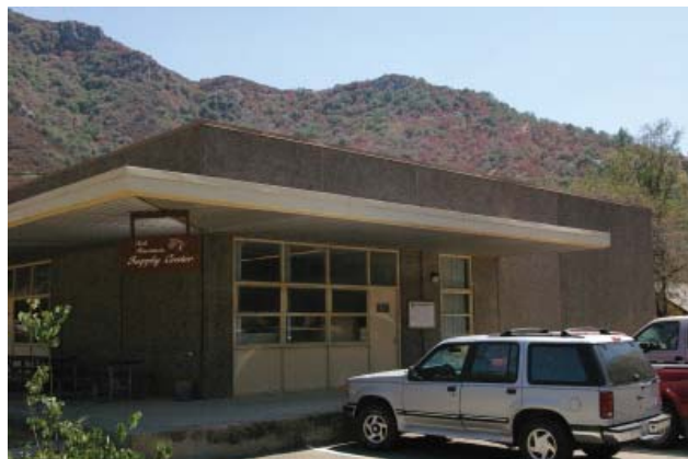
Ash Mountain Warehouse (Contributing)
