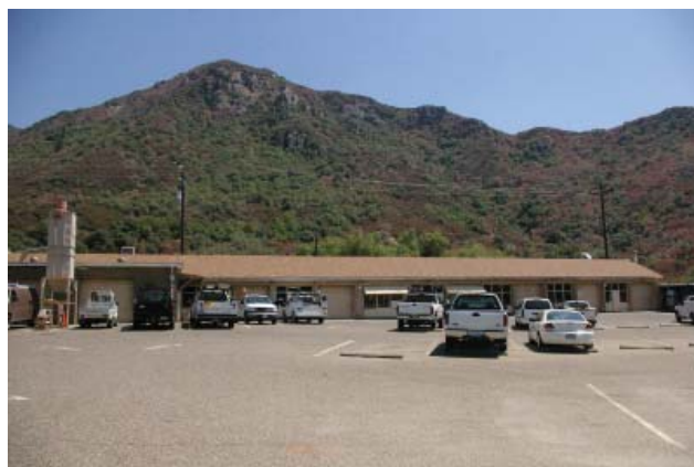
Ash Mountain Equipment Shed/ Maintenance Building (Contributing)
