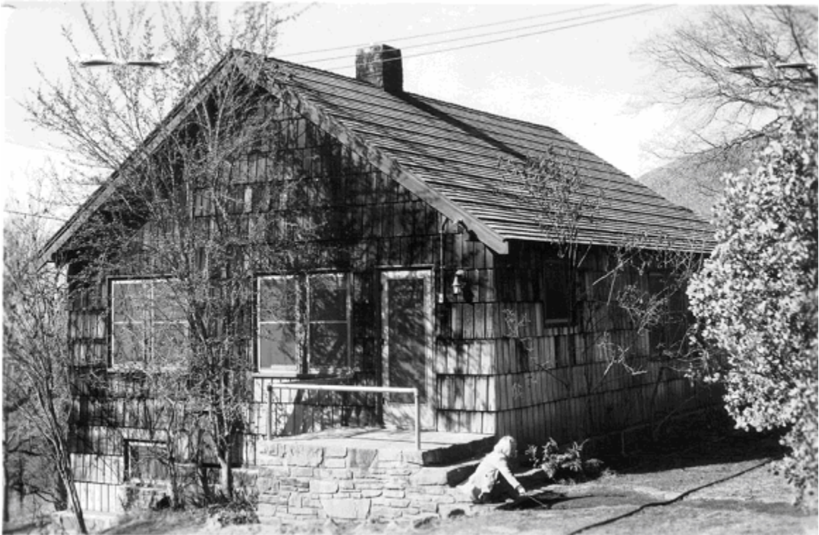
History Photo #8: Residence #87. This 1938 building was built by the CCC and is typical of the residences from this time. It had a cedar shingle roof with a double coursing of shingles every fourth row for enhanced texture and protection (SEKI Archives).
