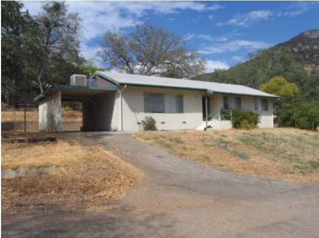
Buckeye Residence #1405 (Contributing)
