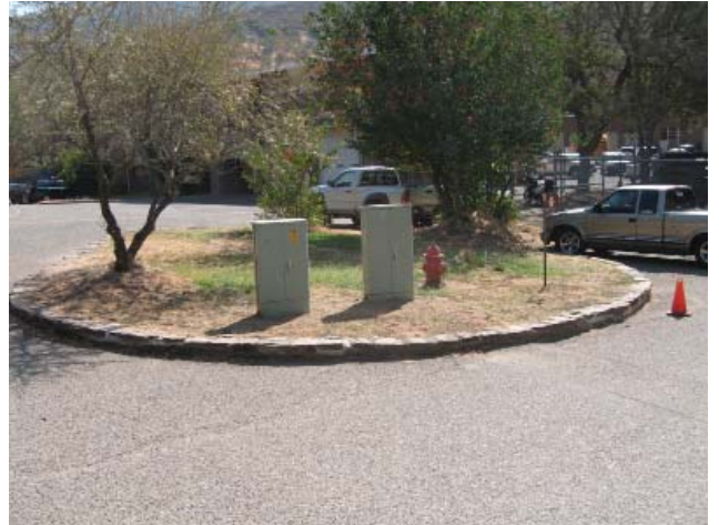
Maintenance Yard Road (Contributing)
