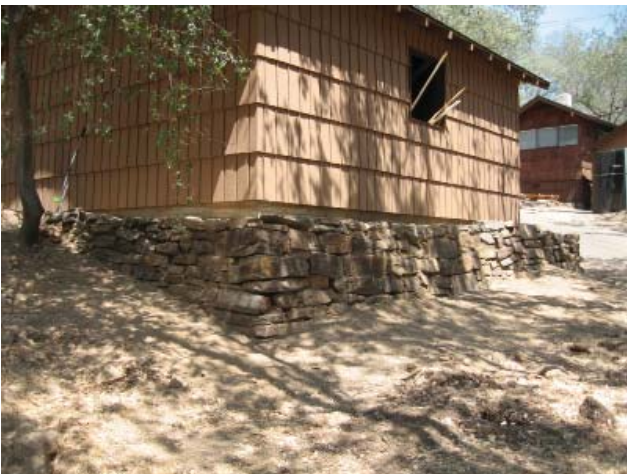
Ash Mountain Schist Retaining Wall (Contributing)
