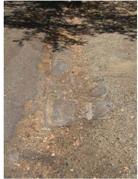
Ash Mountain Schist Gutter ( Contributing )
