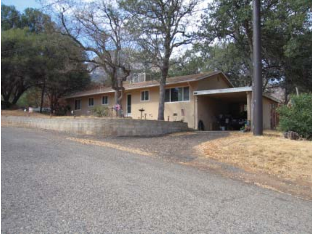
Buckeye Residence #1419 (Contributing)
