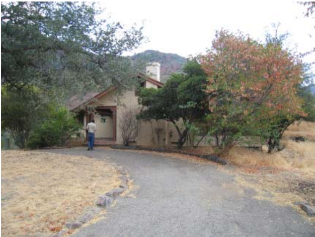
Ash Mountain Research Office/Residence #12 (Contributing)
