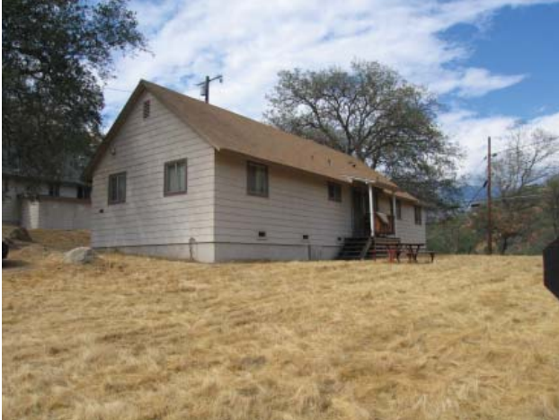
Buckeye Residence # 127/ Foreman's Dormitory (Noncontributing)
