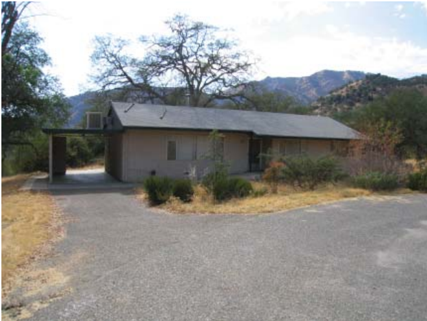
Buckeye Residence #1409 (Contributing)
