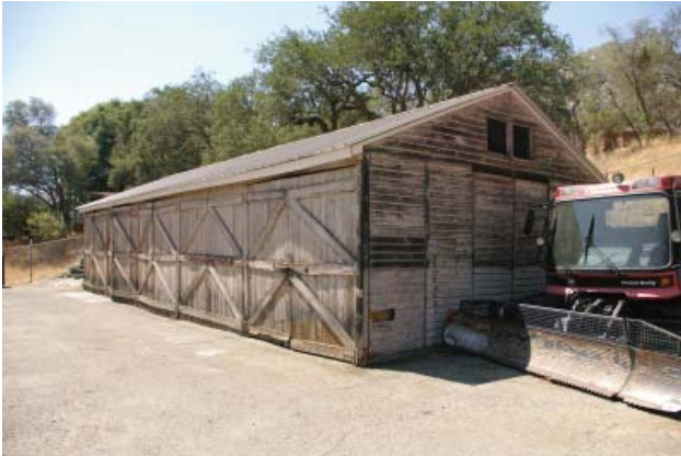
Ash Mountain Storage Building/ Lower Maintenance Shed (Contributing)
