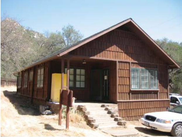
Ash Mountain Sub District Ranger Office/ Residence #5 (Contributing)
