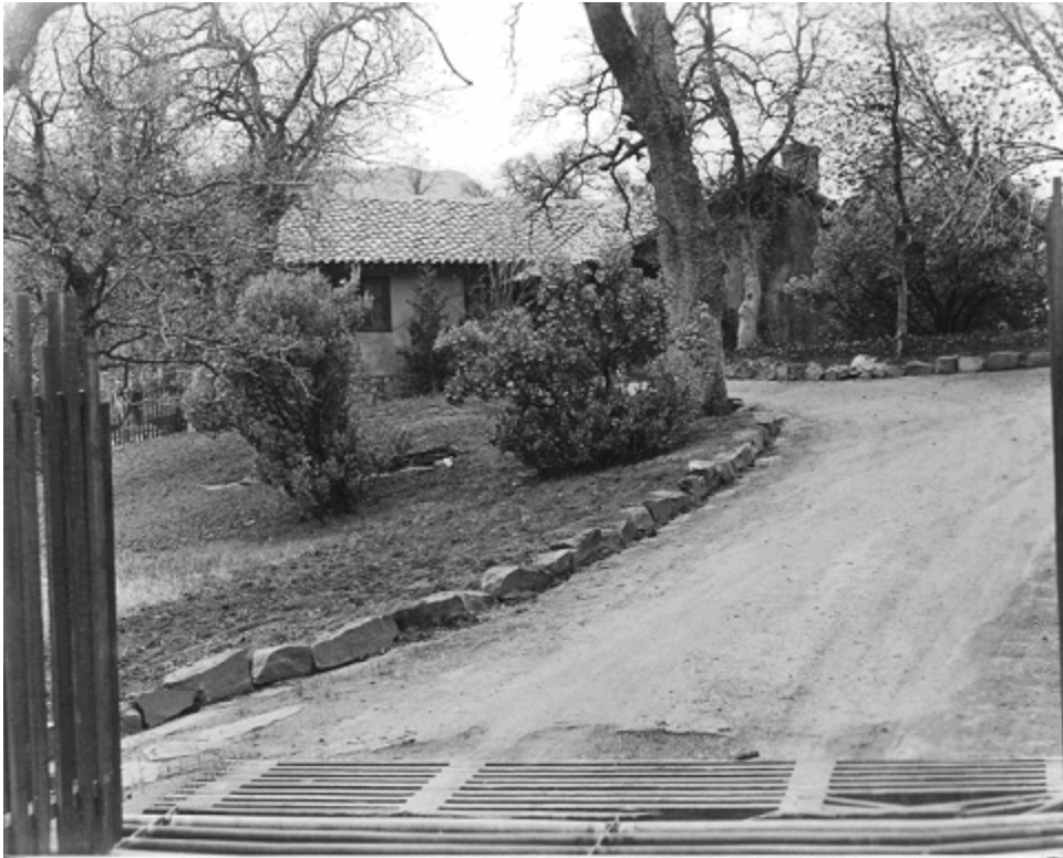
Physical History #4: Superintendent's residence (#12) and grounds, 1934. The residential areas had a mix of stucco structures in the Spanish Eclectic style (such as this one), and rustic structures with shake siding (SEKI Archives).
