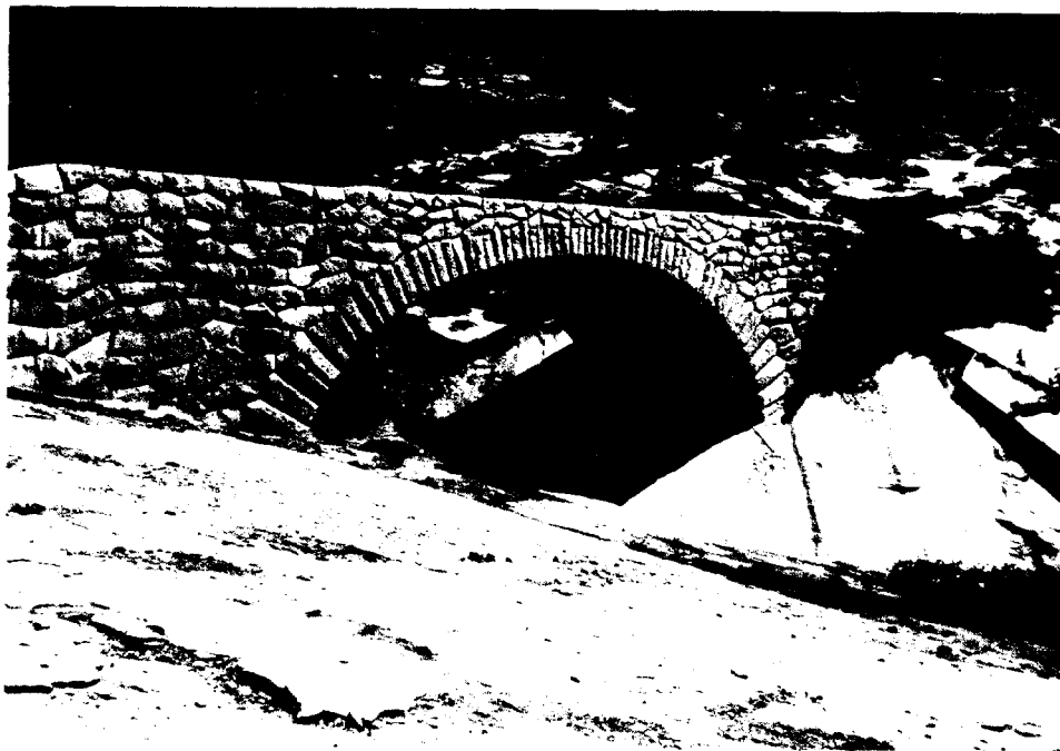
Photograph No. 79 -- Clover Creek Bridge; downstream side
