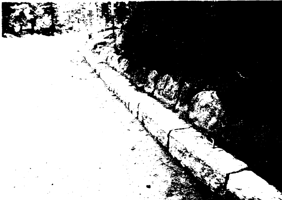
Photograph No. 3 -- Cut stone curbing and rock bench along highway across from Giant Forest Market Plaza
