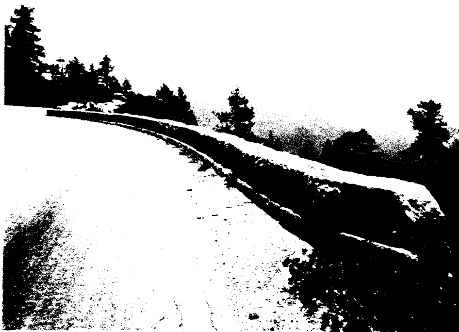
Photograph No. 93 -- Masonry parapet wall along downslope side of highway just above Redwood Mountain Grove turnout
