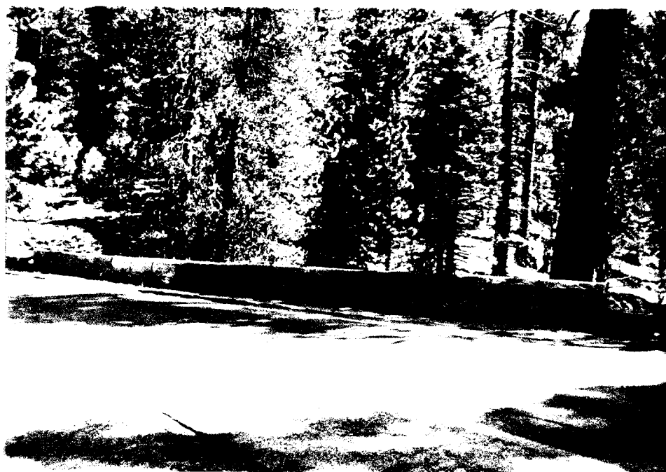
Photograph No. 73 -- Masonry rock parapet wall on bridge over Marble Fork of Kaweah River on downslope side of highway
