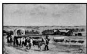
• SCBL 21 - "ROCK CREEK STATION". Watercolor depicting covered ox-drawn wagons near some log buildings.
