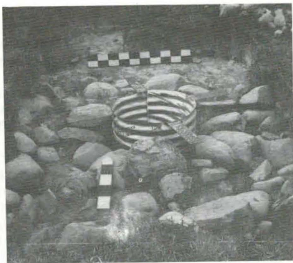
Figure 7. The Woodworth well, after a culvert was inserted in 1985 to prevent collapse.
