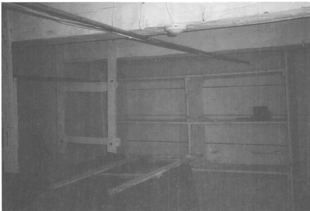
Figure 153. Food storage room (Room 003), looking southeast.
