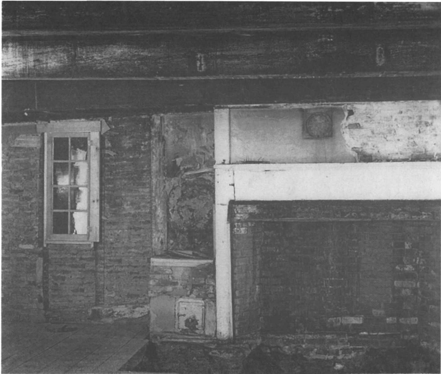
Figure 59. Schuyler House: First story of kitchen wing after ca.-1815 lath and plaster removed; view of east wall showing post-1780 window, fireplace, mantel, and boiler station (1958).
