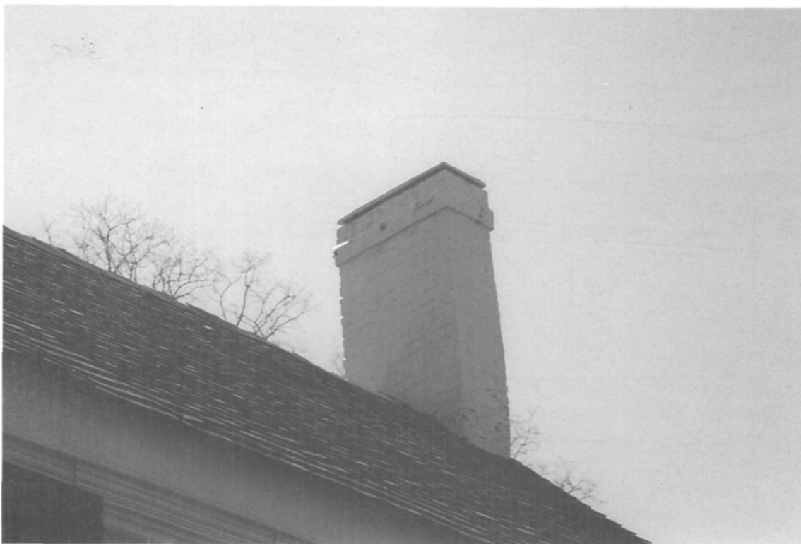
Figure 135. Main house, south chimney.
