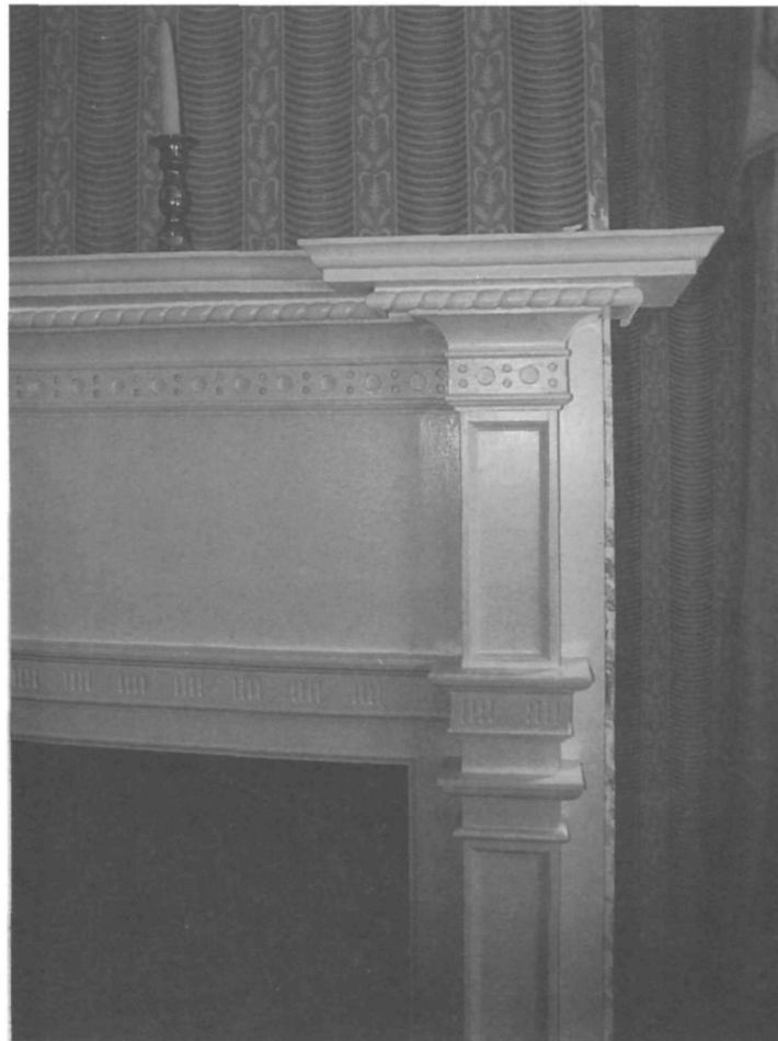
Figure 172. Parlor (Room 102), south-wall mantelpiece detail.
