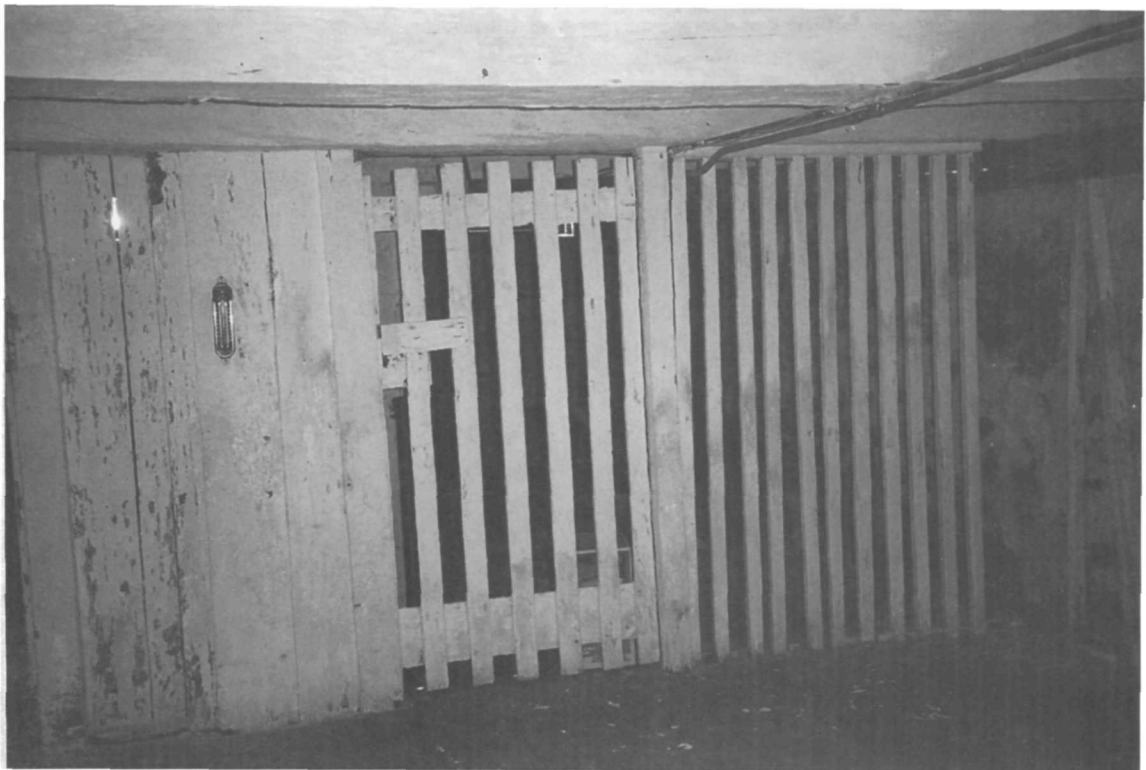
Figure 149. Cellar storage room (Room 002), south wall.
