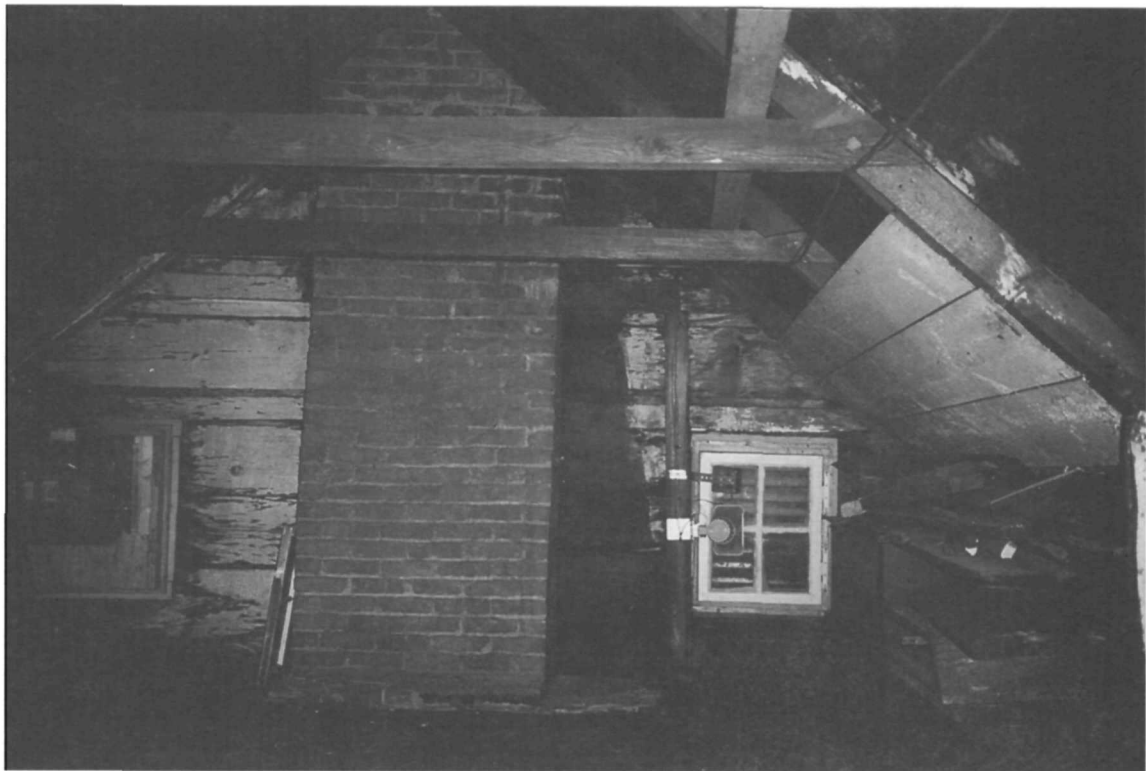
Figure 248. South attic room (Room 301), south wall.
