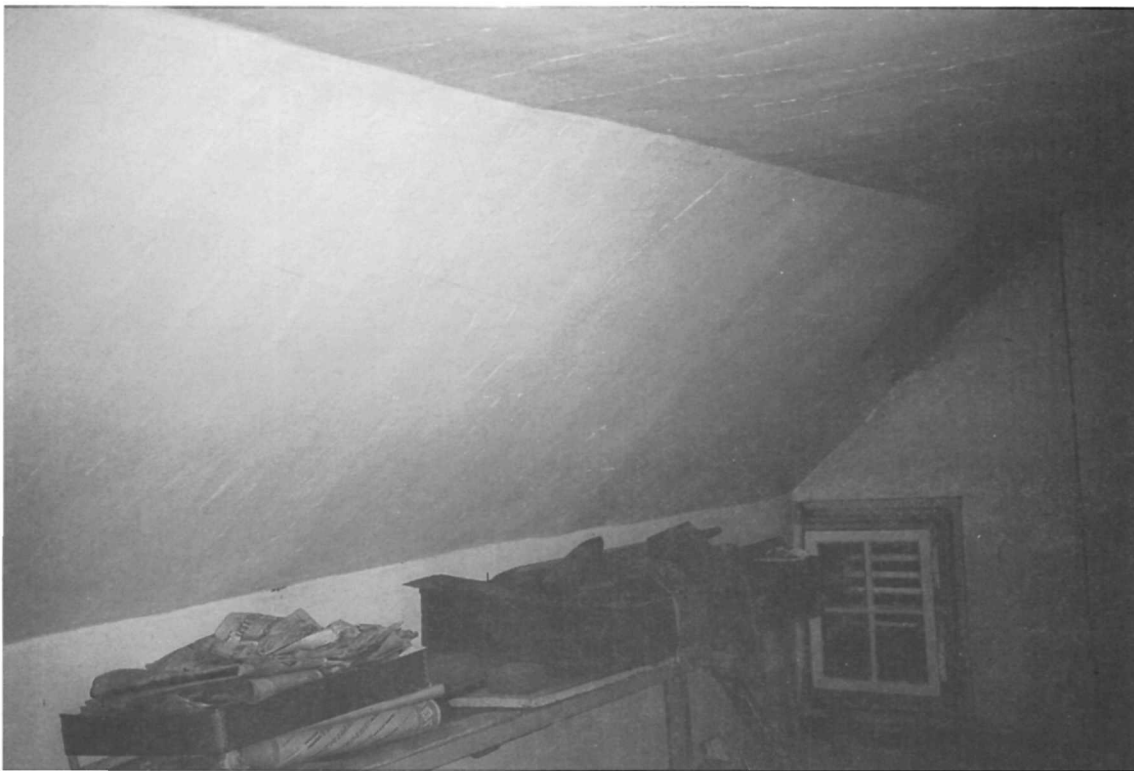
Figure 253. North attic room (Room 302), looking northwest.
