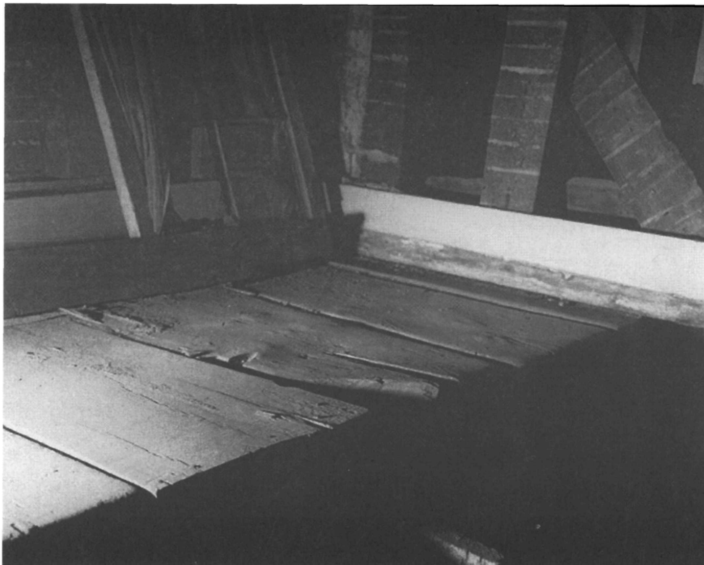
Figure 61. Schuyler House: Second story of kitchen wing after ca.-1815 lath and plaster removed; worn flooring in hall (Room 206) at location of ca.-1780 staircase landing (1958).
