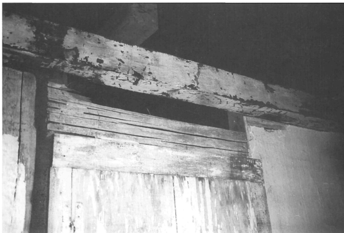
Figure 246. East servants' room (Room 209), west wall, stud-pocket evidence of former doorway.
