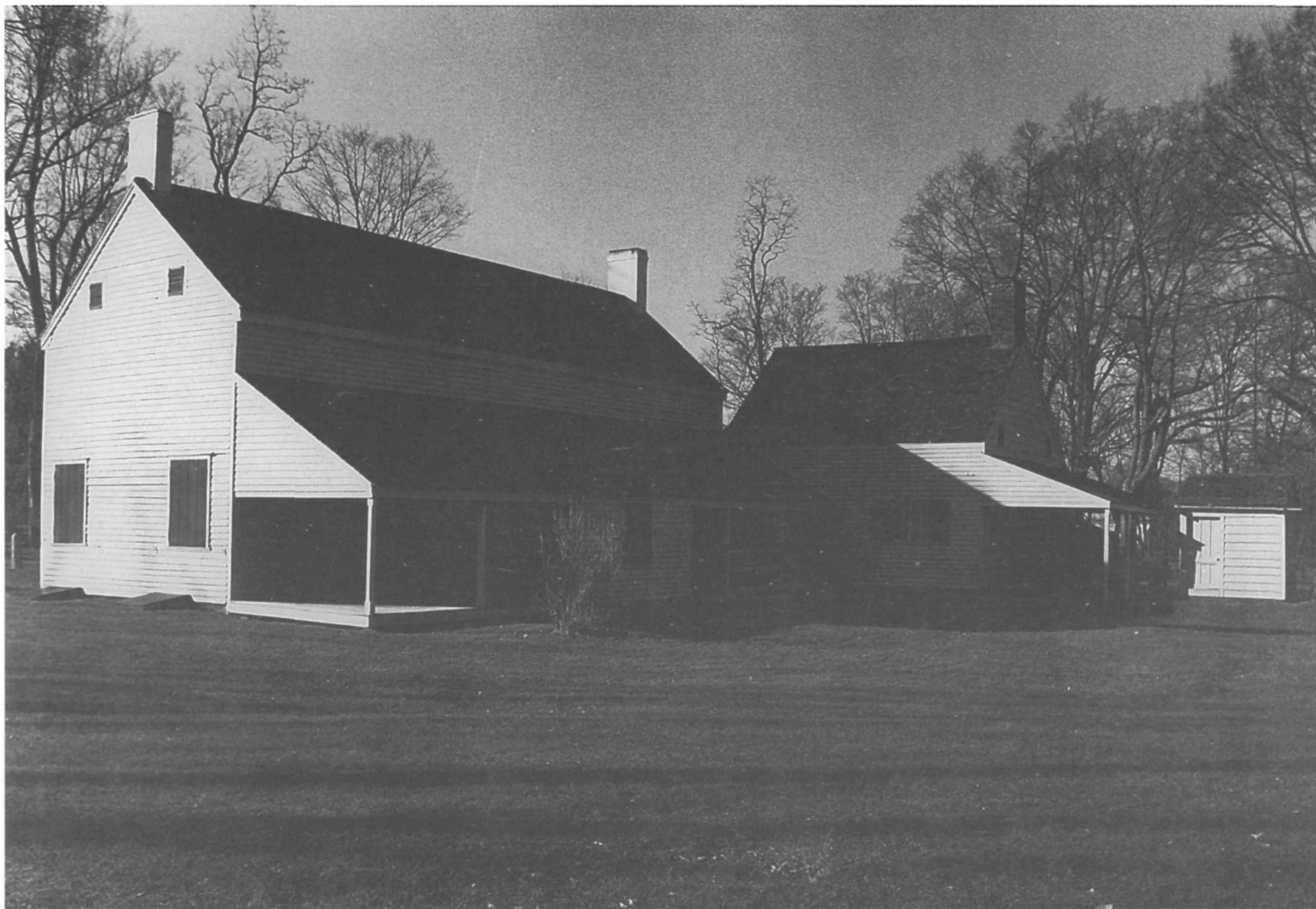
Figure 87. Schuyler House: View from the southeast (ca. 1990).
