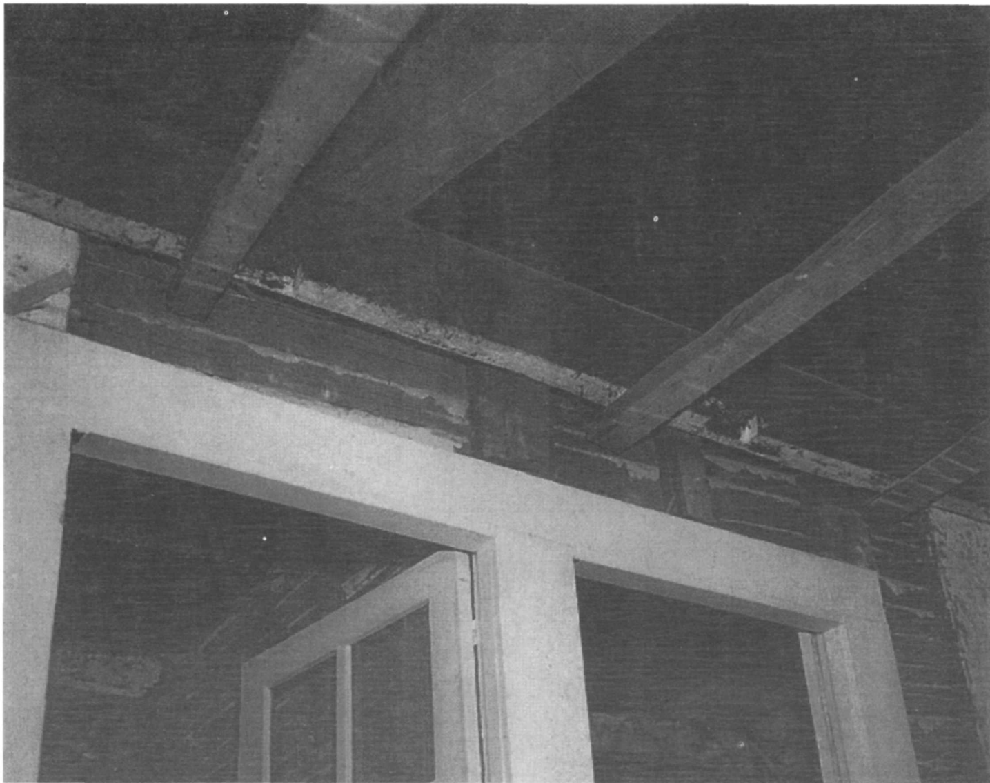
Figure 63. Schuyler House: Second story of kitchen wing after ca.-1815 lath and plaster removed; east wall of hall (Room 206), where mortises in collar beam over ca.-1815 doorways mark location of ca.-1780 doorway (1958).
