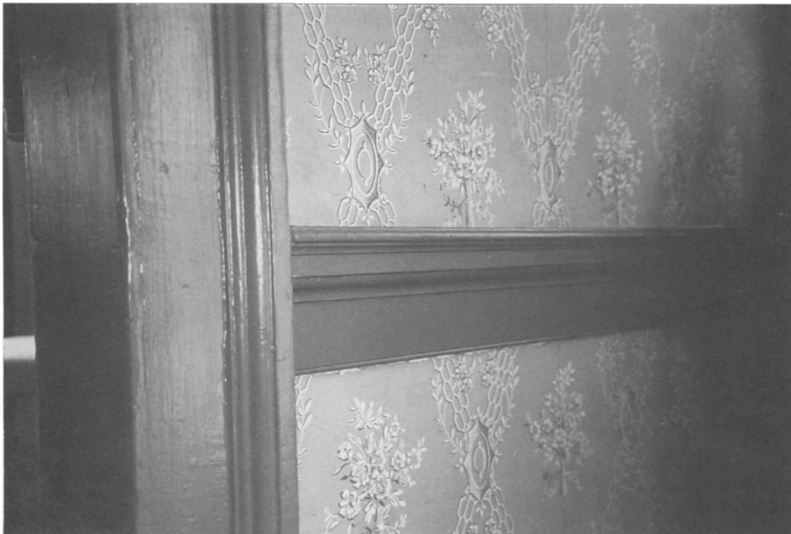
Figure 164. Reception hall (Room 101), west end of south wall, chair-rail detail.
