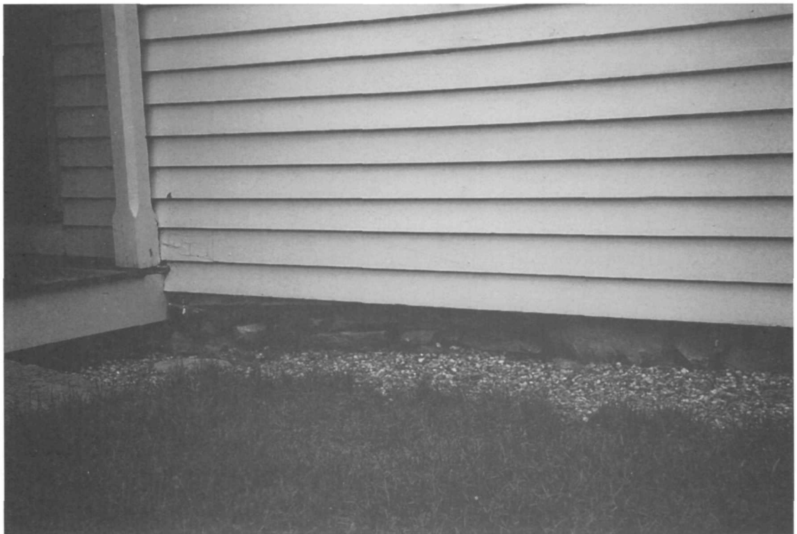
Figure 131. Kitchen wing, south elevation, fieldstone foundation.
