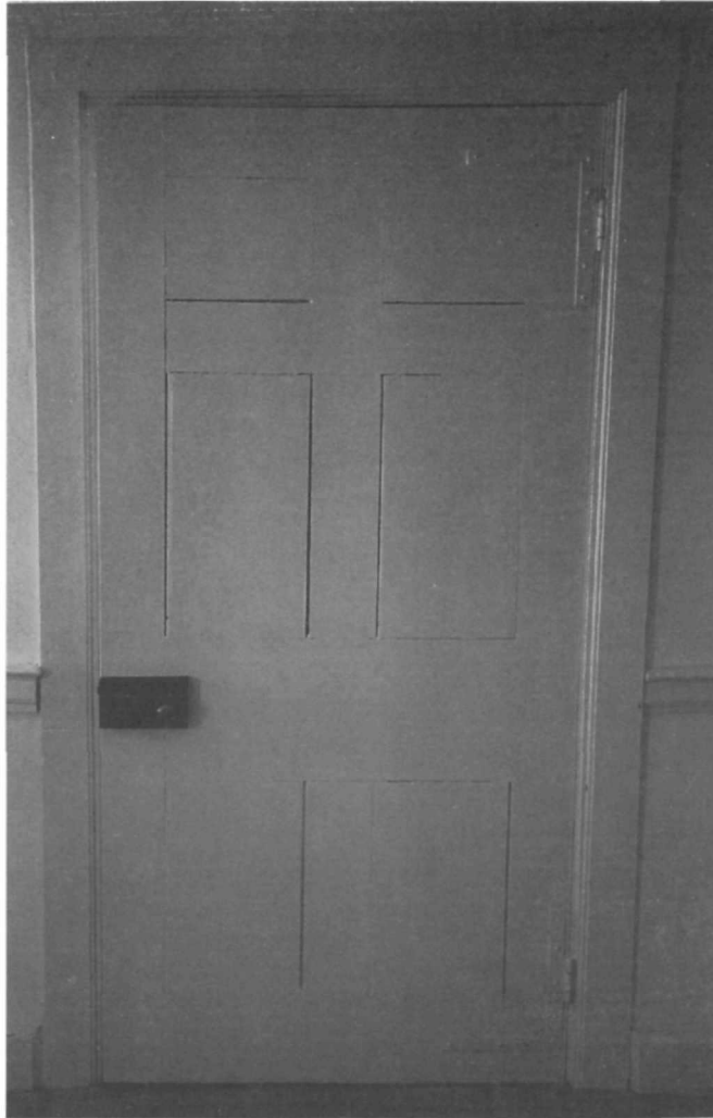
Figure 205. South chamber (Room 202), north wall, doorway D201.
