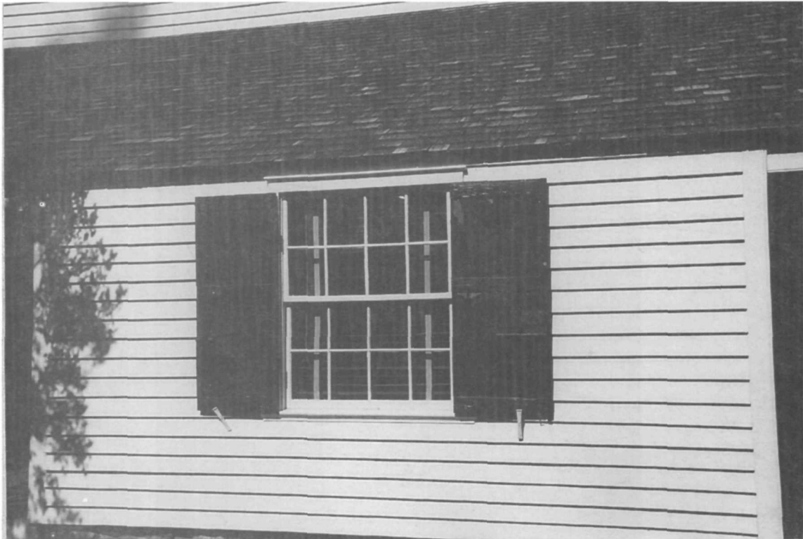
Figure 121. Rear addition, east elevation, window W109.
