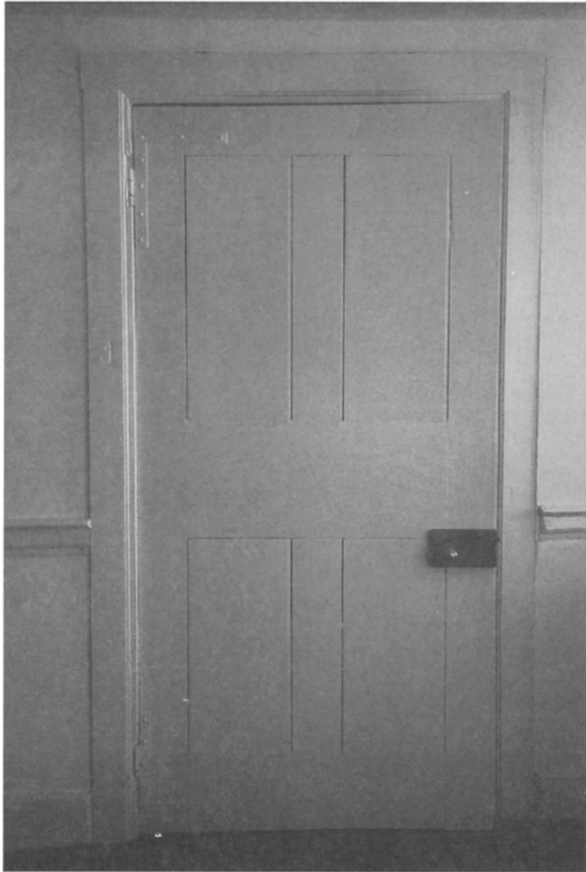
Figure 215. North chamber (Room 205), south wall, doorway D203.
