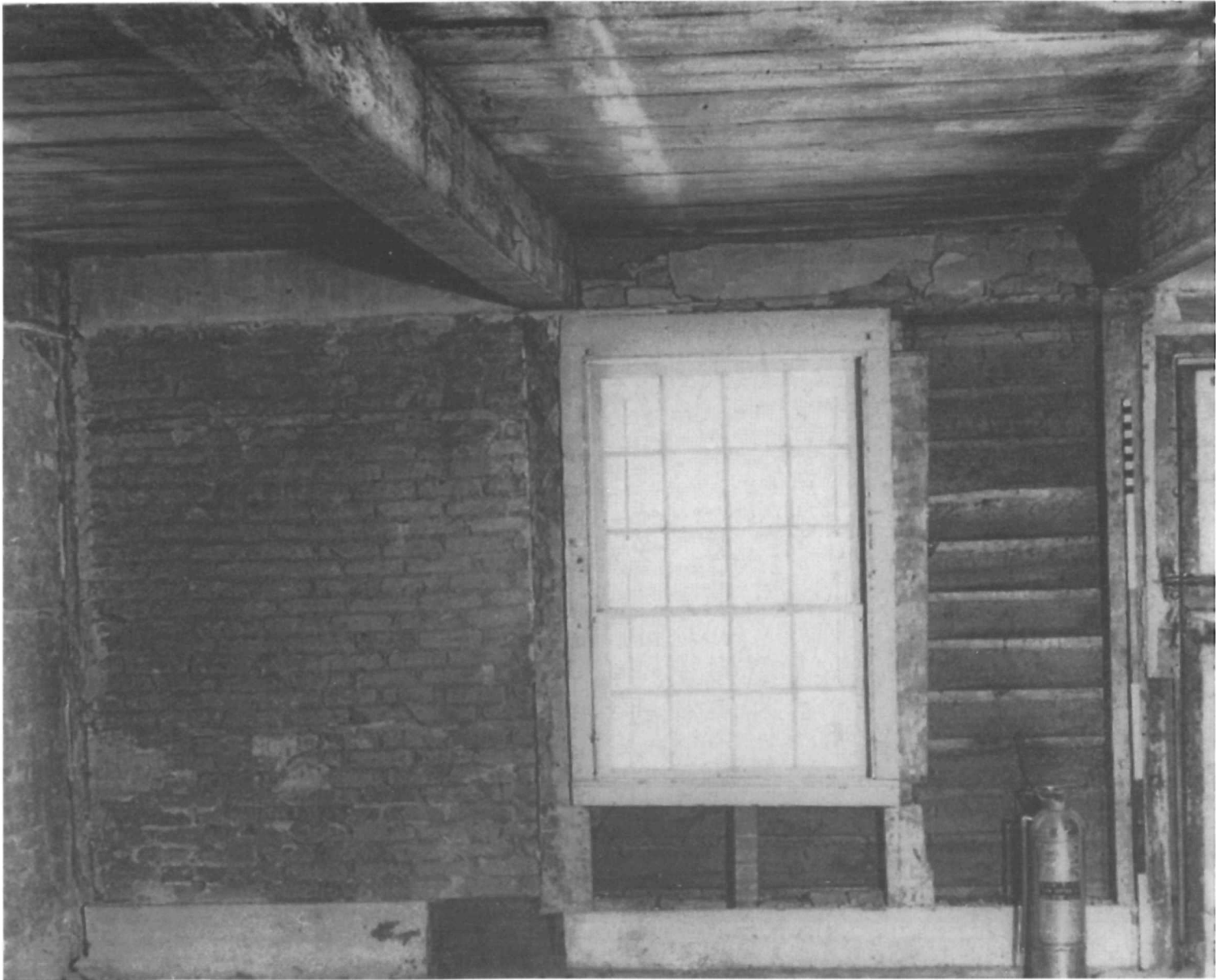
Figure 55. Schuyler House: First story of kitchen wing after ca.-1815 lath and plaster removed; view toward west end of north wall, showing mark of ca.-1780 partition in line with later window (1958). Original nogging for storage room at left.
