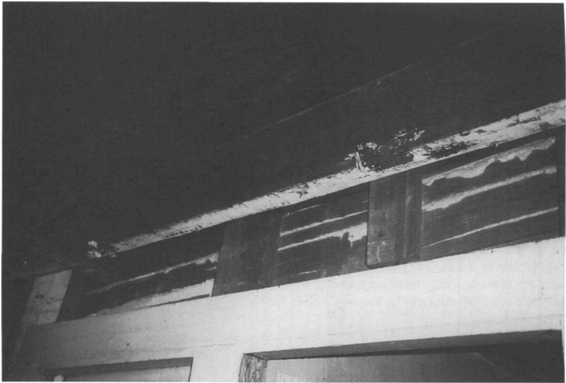
Figure 228. Second-story kitchen hall (Room 206), east wall, stud-pocket evidence of former doorway.
