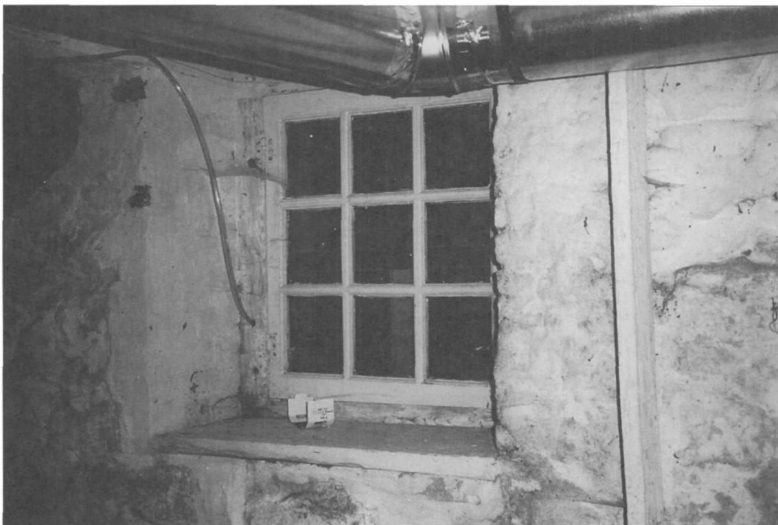
Figure 158. Cellar kitchen (Room 004), west wall, window W002.
