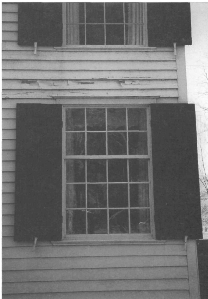
Figure 125. Main house, north elevation, window W112.
