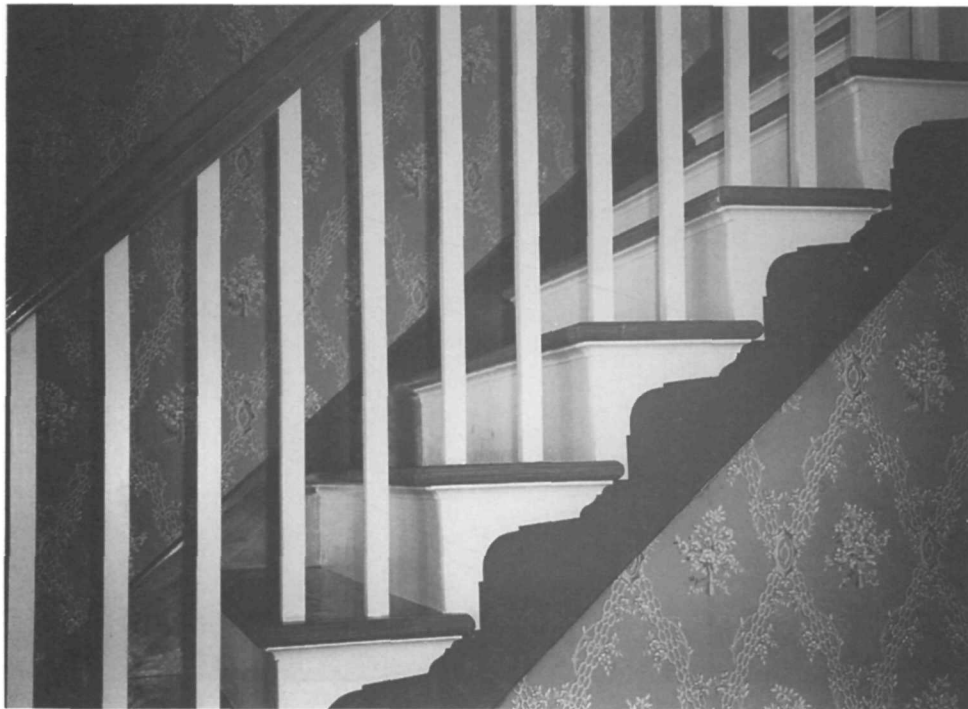
Figure 166. Reception hall (Room 101), north-wall staircase detail.
