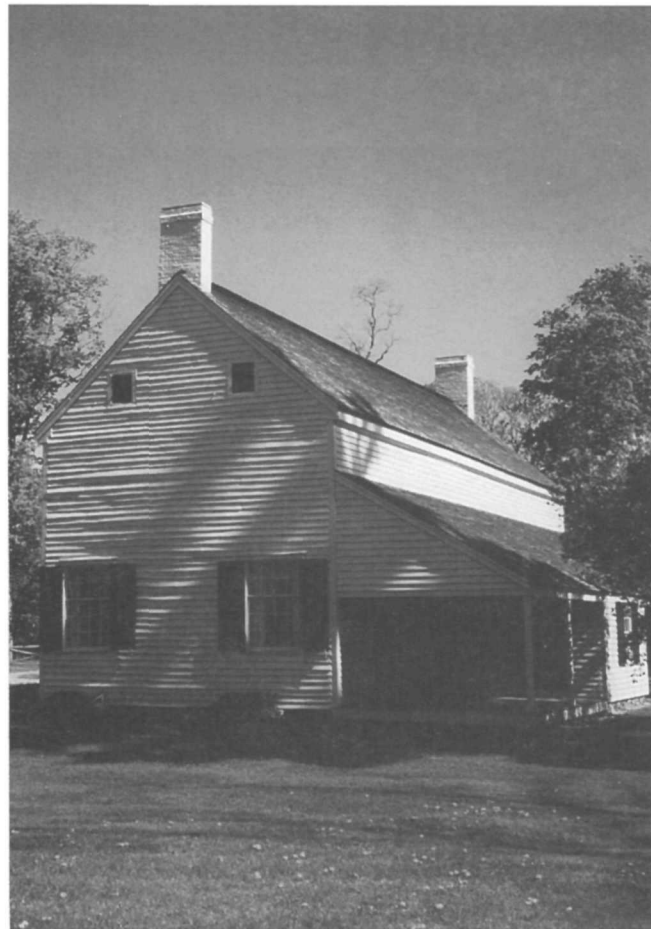
Figure 103. Main house, south elevation.
