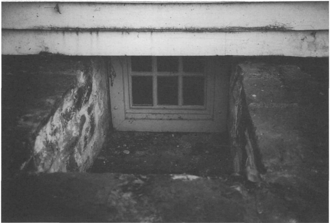
Figure 116. Main house, north elevation, window W106.
