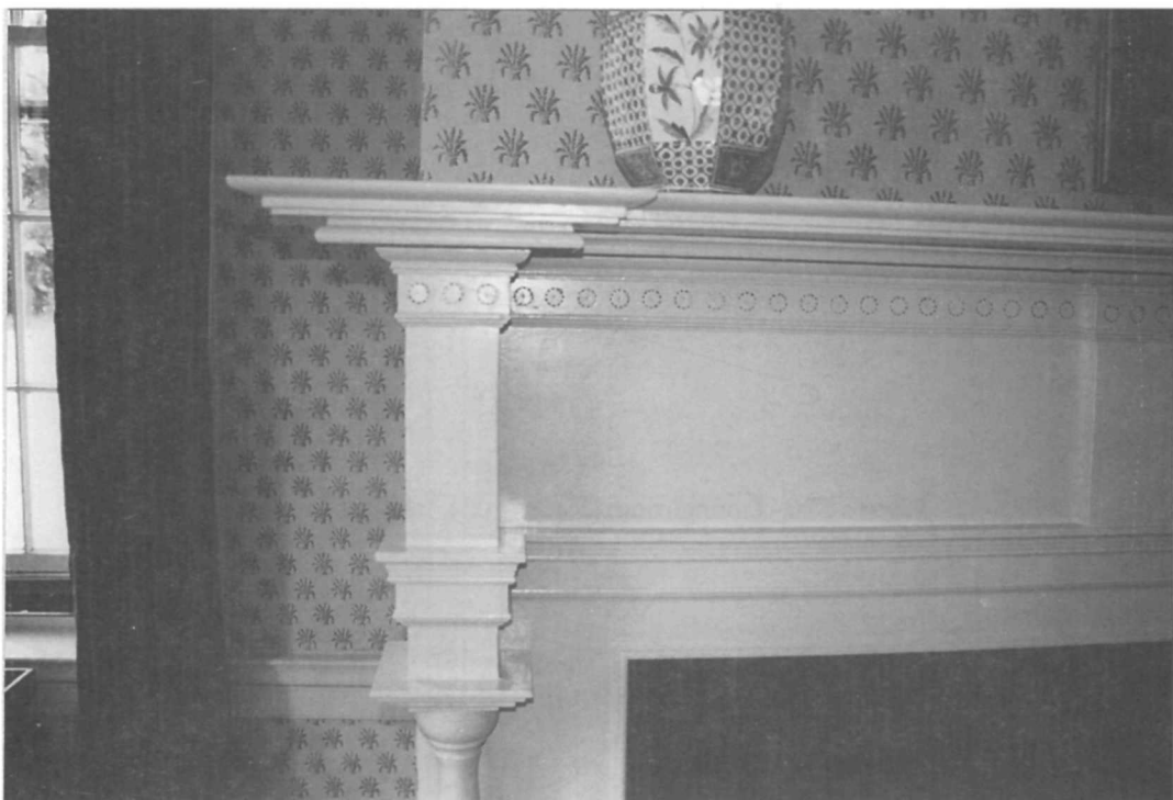
Figure 178. Dining room (Room 103), north-wall mantelpiece detail.
