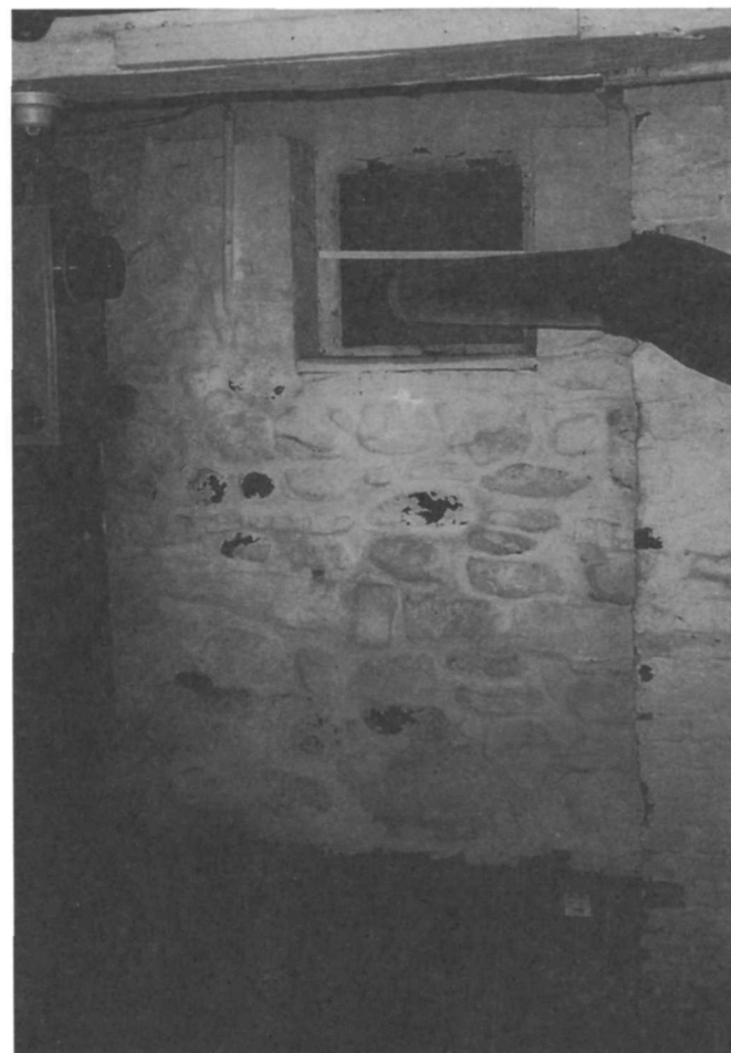
Figure 160. Cellar kitchen (Room 004), south wall, window W004.
