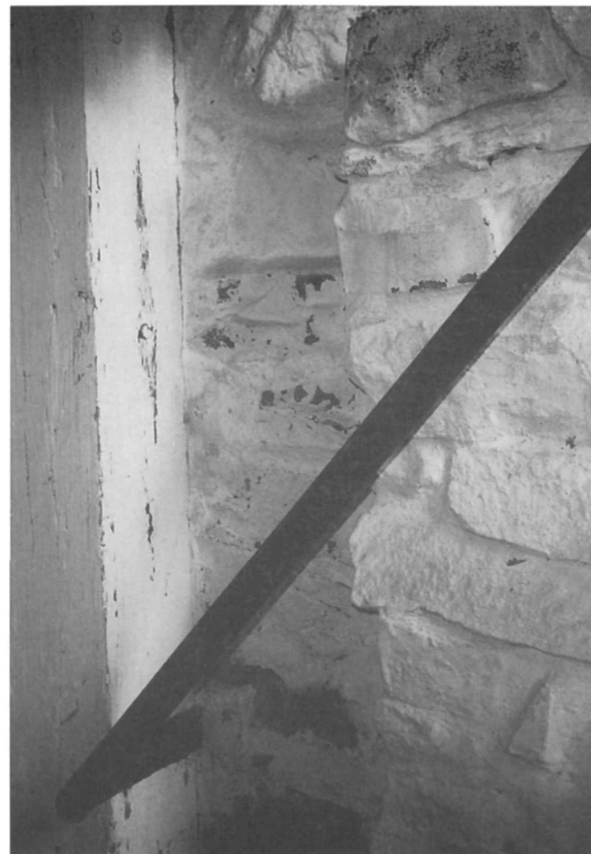
Figure 147. Cellar hall (Room 001), north wall of bulkhead, showing former location of doorway jamb.
