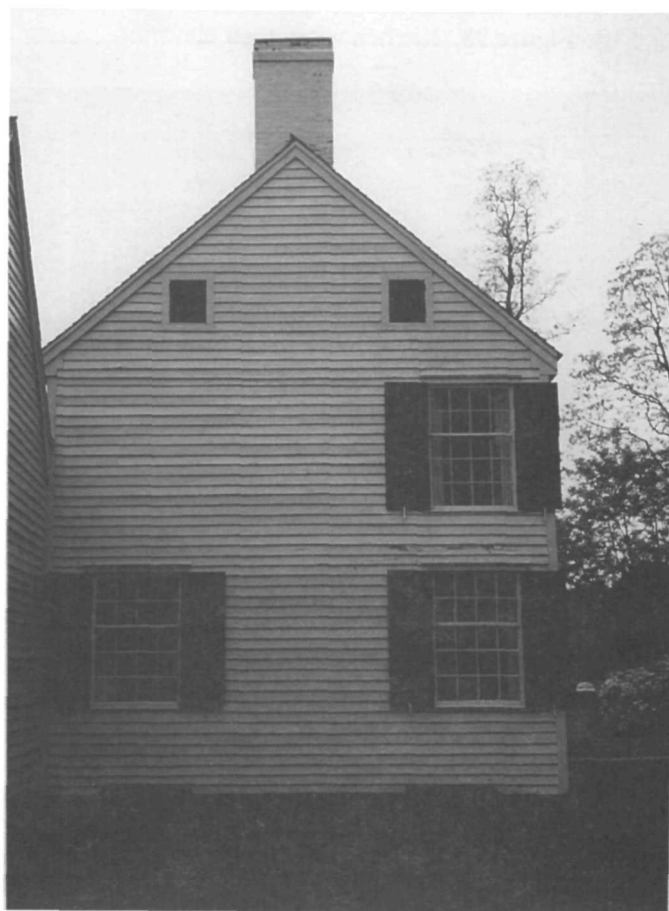
Figure 97. Main house, north elevation.
