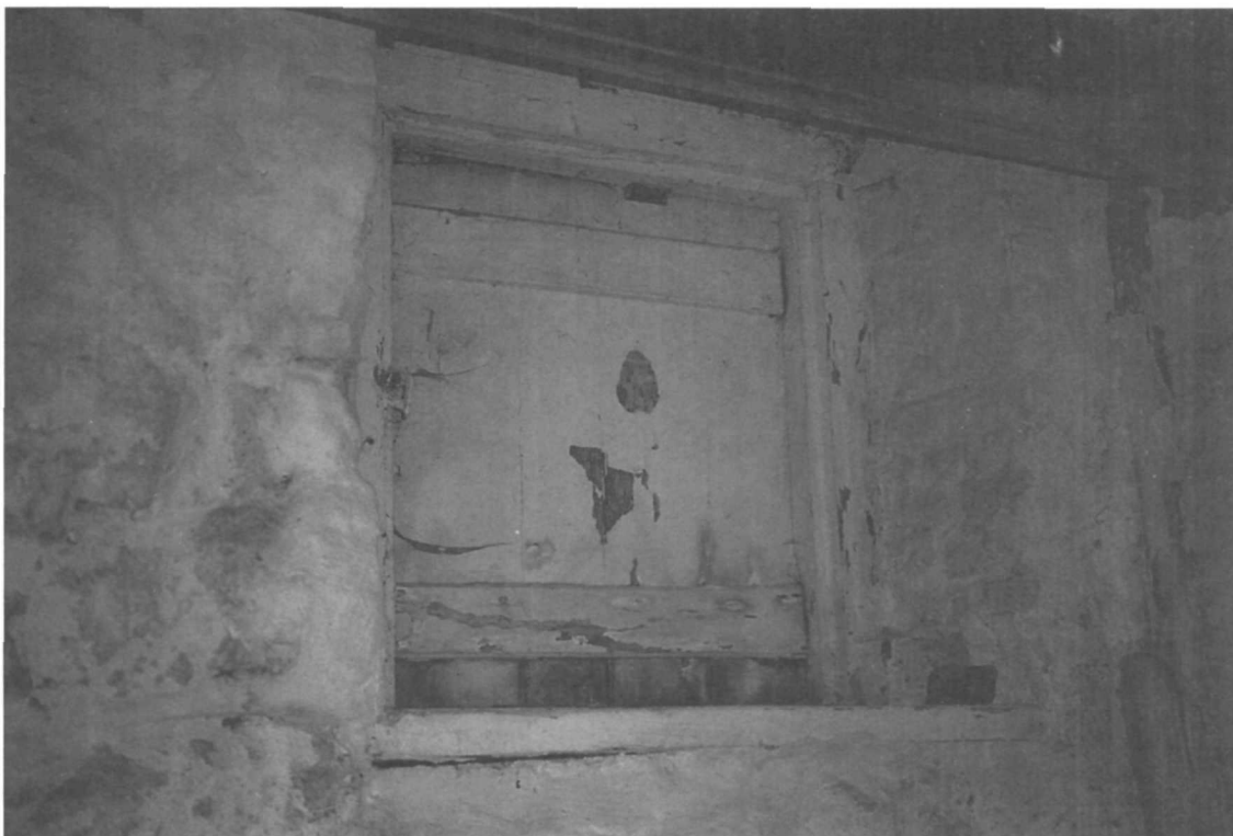
Figure 157. Cellar kitchen (Room 004), west wall, opening O001.
