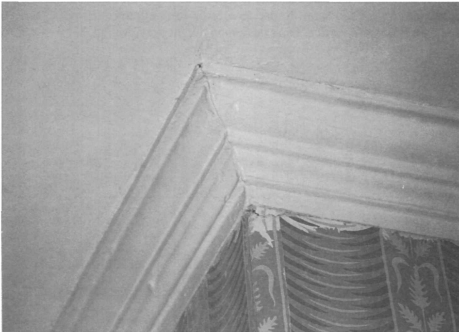
Figure 175. Parlor (Room 102), south-wall cornice detail.
