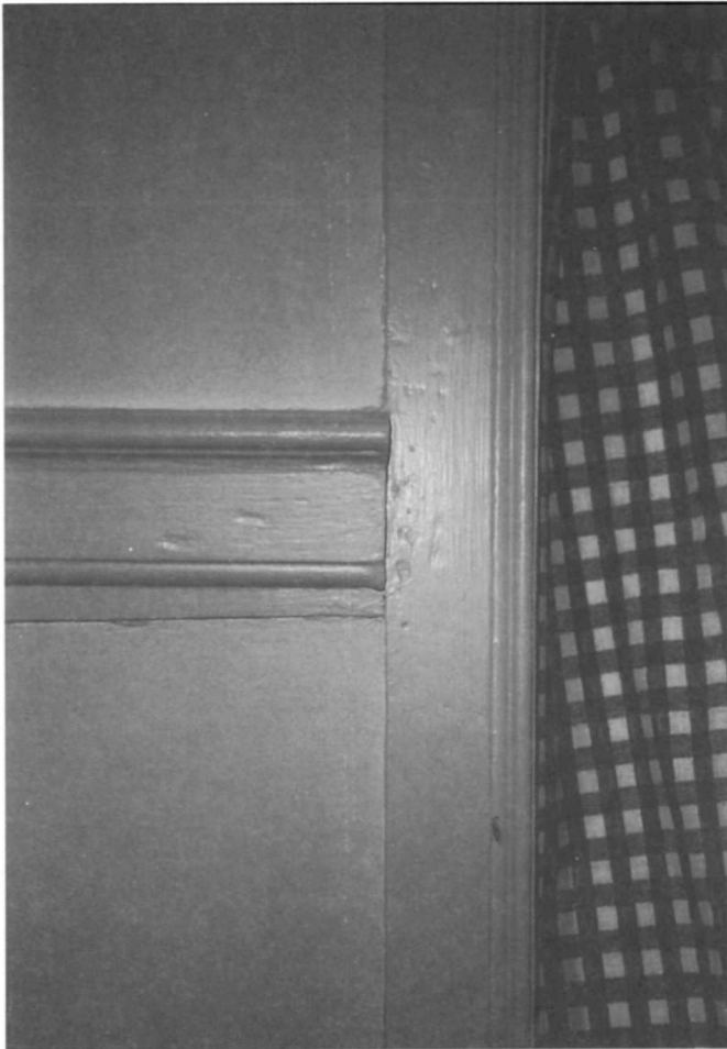
Figure 221. North chamber (Room 205), detail of window casing and chair rail.
