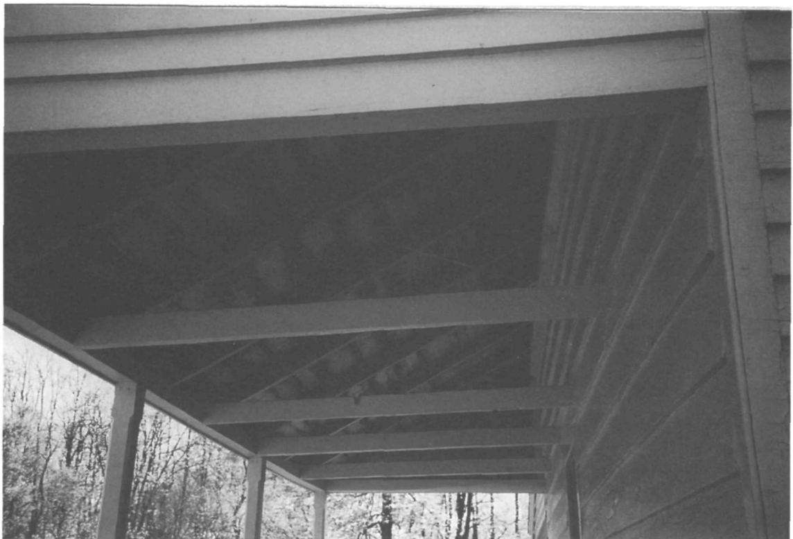
Figure 138. Kitchen wing, porch on north elevation.
