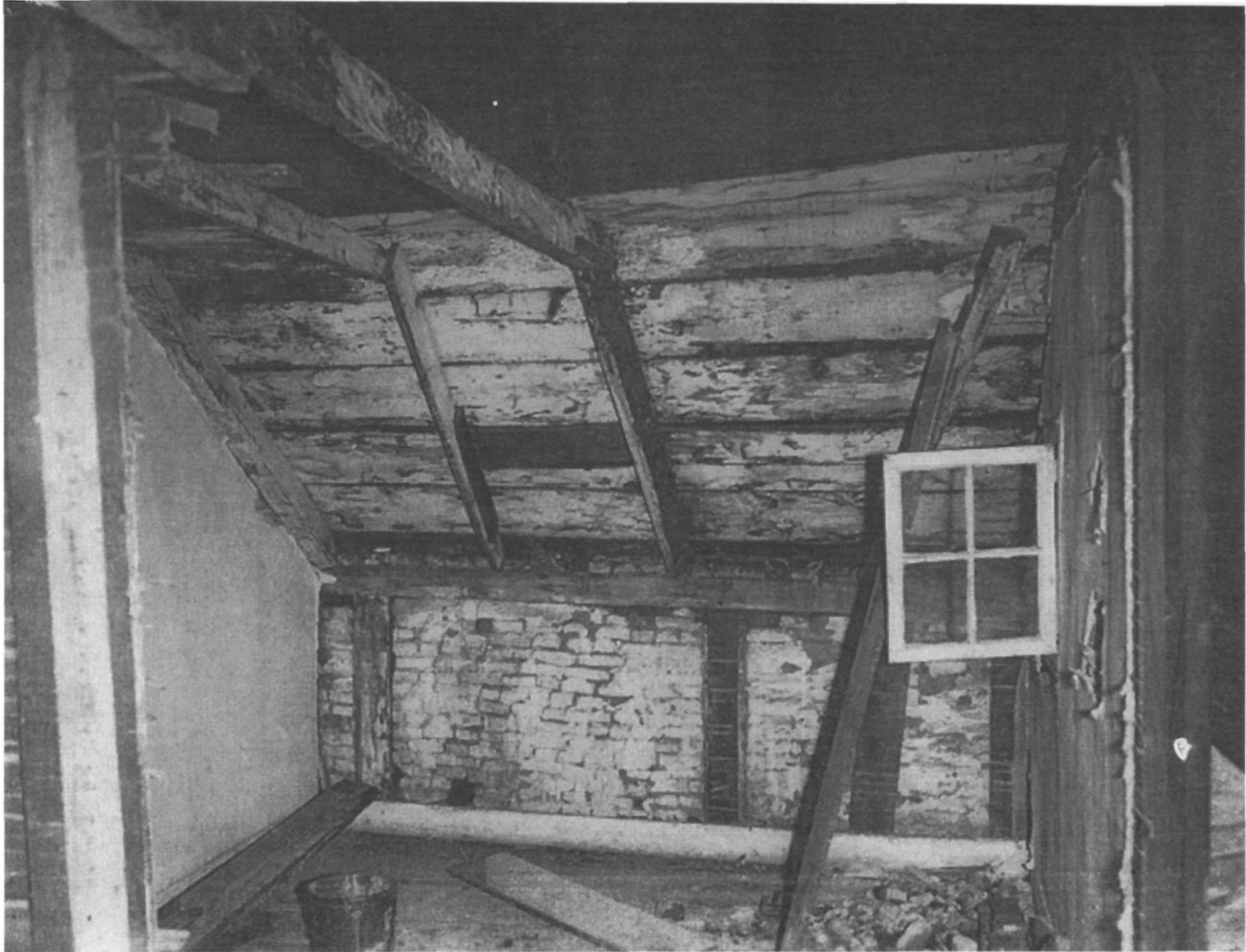
Figure 64. Schuyler House: Second story of kitchen wing after chimney removed; view looking north in east servants' room (Room 209), showing pre-1815 whitewash on nogging and ceiling boards, ca.-1815 plaster walls, and mid-19 th century window sash to right (1958).
