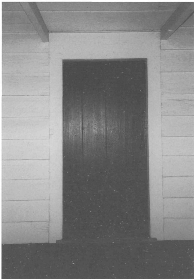
Figure 113. Kitchen wing, north elevation, doorway D105.
