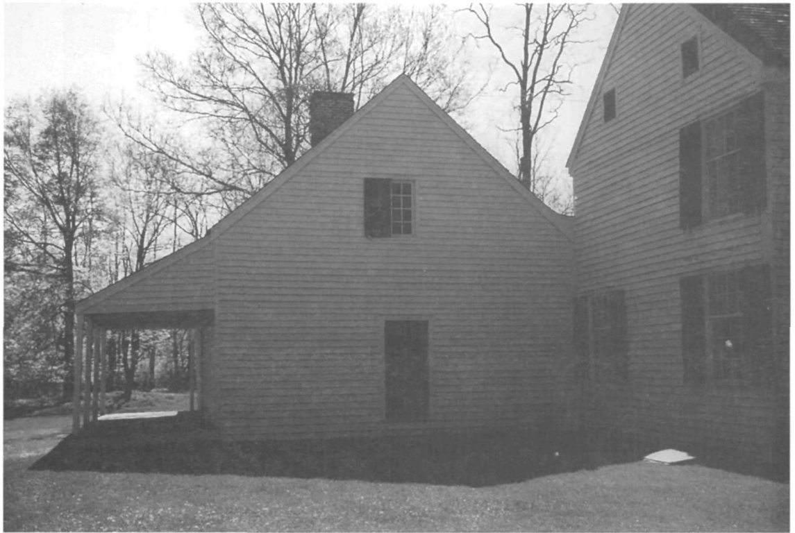
Figure 98. Kitchen wing, west elevation.
