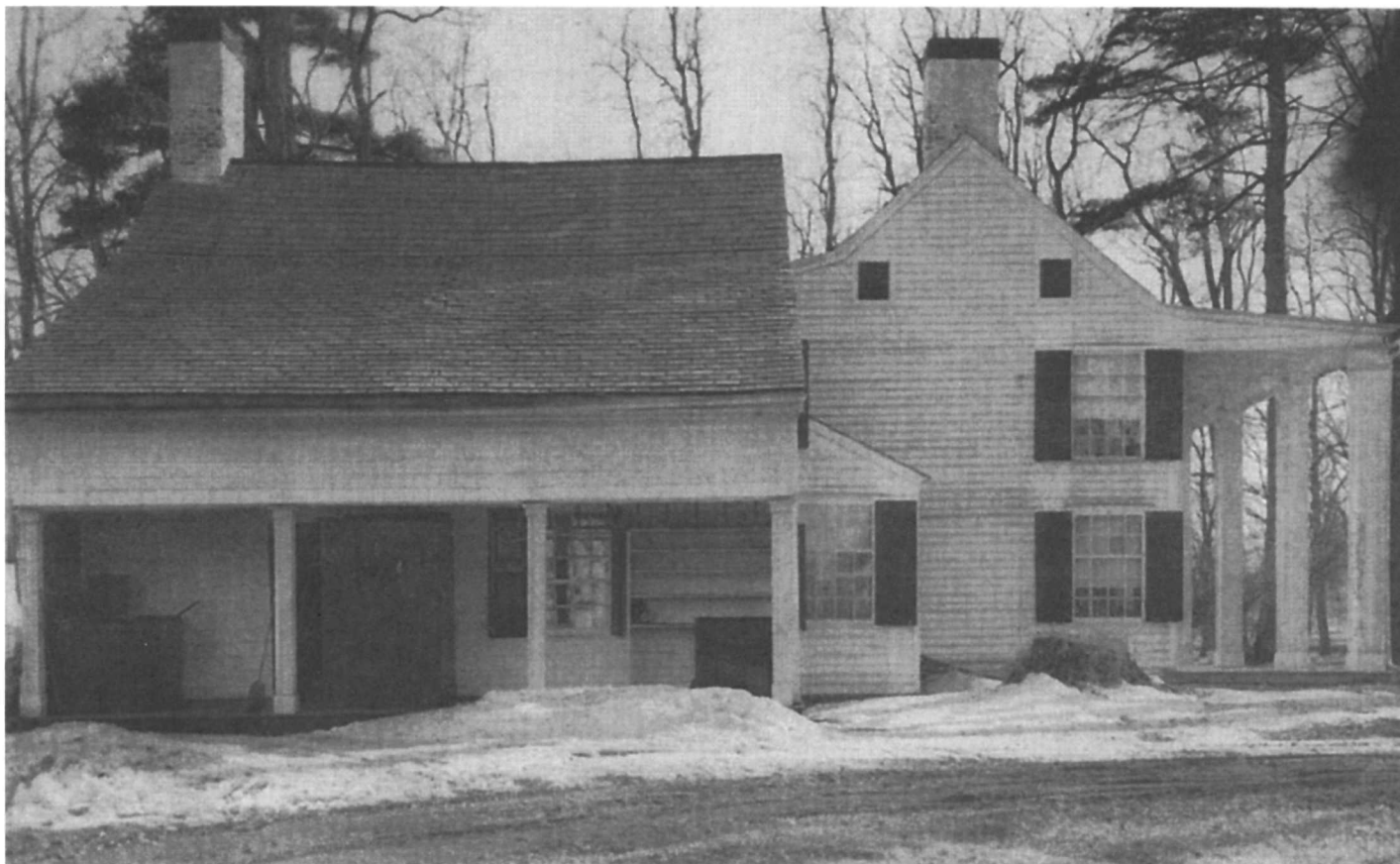
Figure 11. Schuyler House: North elevation (1947).
