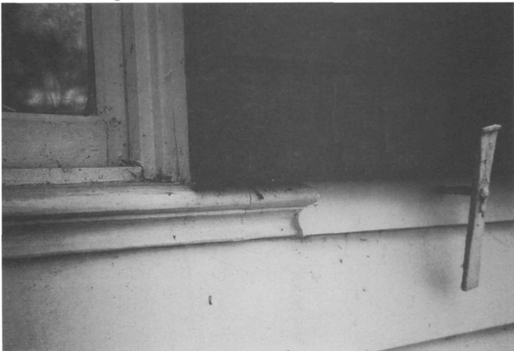
Figure 124. Main house, north elevation, sill detail of window W111.
