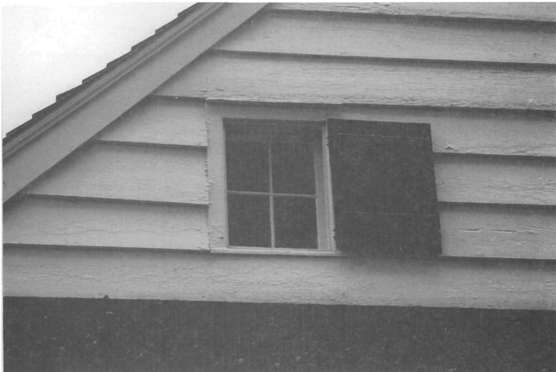
Figure 129. Kitchen wing, east elevation, window W208.
