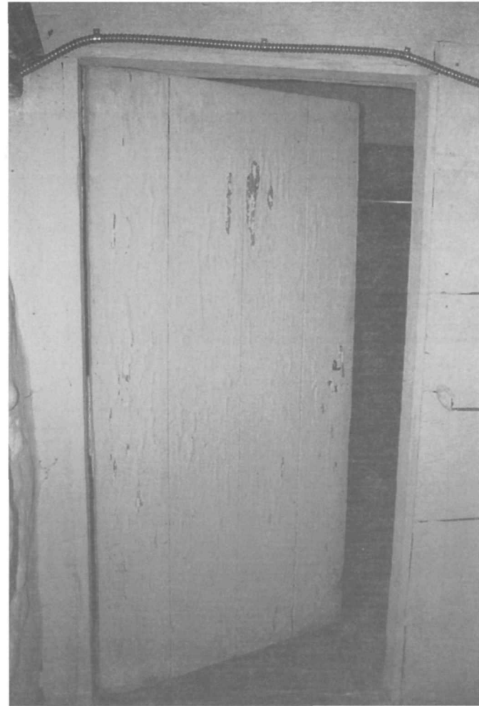
Figure 143. Cellar hall (Room 001), south wall, doorway D005.
