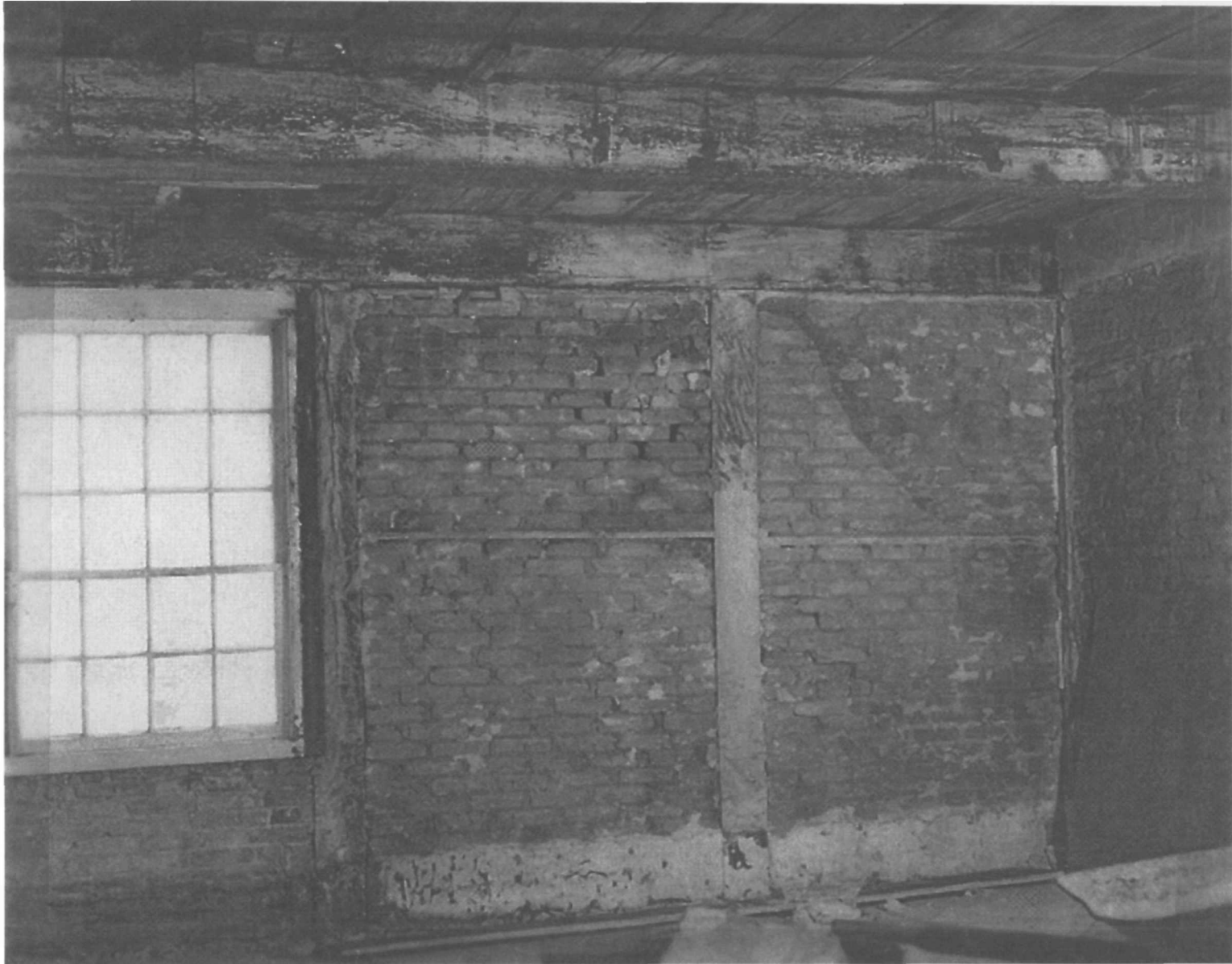
Figure 56. Schuyler House: First story of kitchen wing after ca.-1815 lath and plaster removed; north end of west wall in location of ca.-1780 storage room (1958). Window at left was originally a ca.-1780 exterior doorway.
