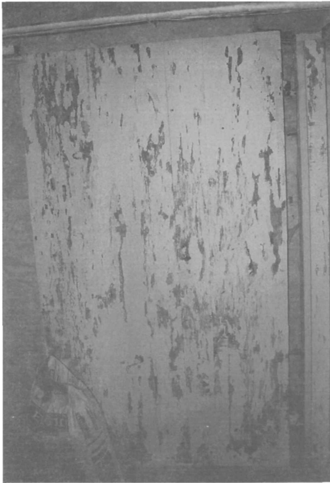
Figure 142. Storage-room side of door in doorway D003.
