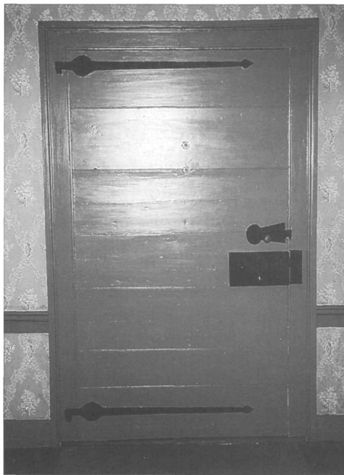
Figure 167. Reception hall (Room 101), west wall, doorway D101.
