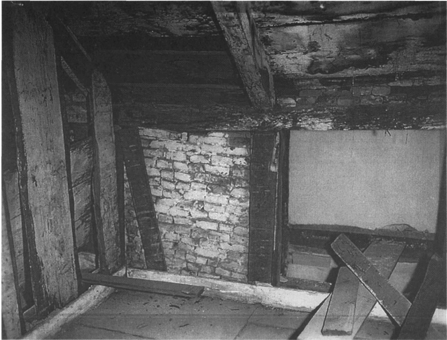
Figure 65. Schuyler House: Second story of kitchen wing after ca.-1815 lath and plaster removed; southeast corner of south servant's room (Room 207), showing whitewash lines on edges of planks where other planks had originally overlapped (1958).
