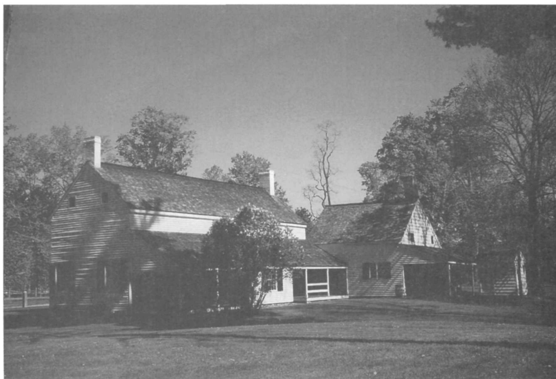
Figure 101. View from the southeast.
