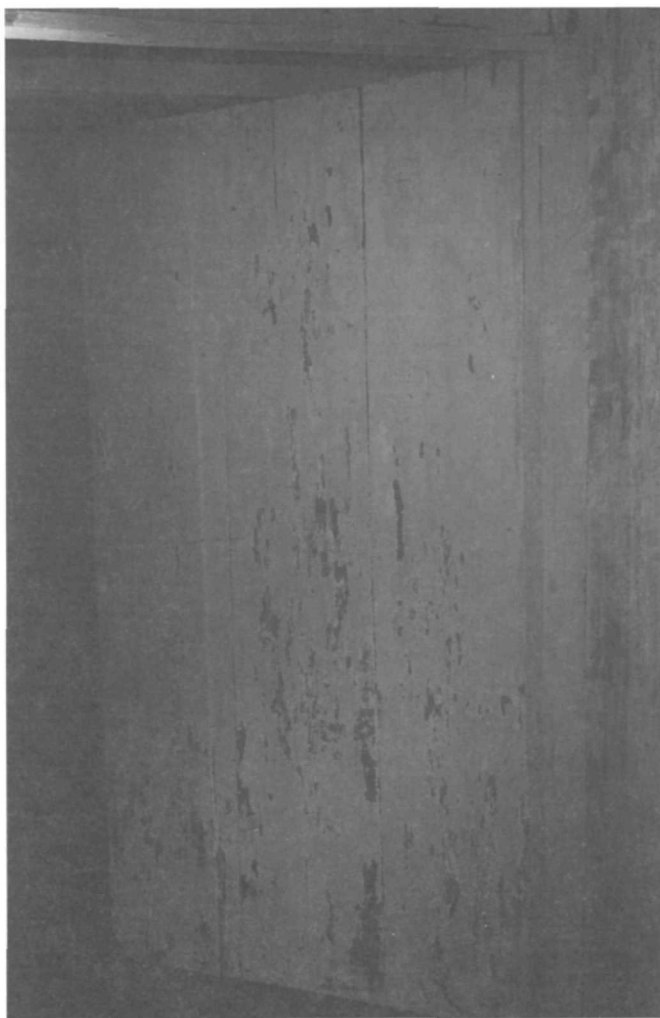
Figure 144. Cellar hall (Room 001), west wall, doorway D004.
