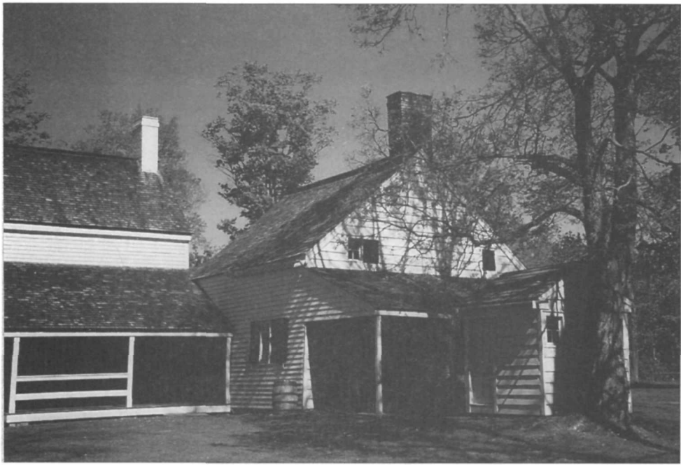
Figure 102. Kitchen wing, view from the east/southeast.
