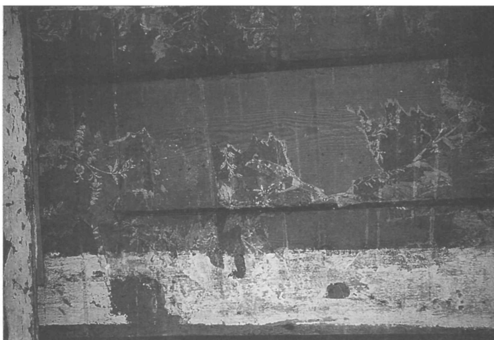
Figure 231. South servant's room (Room 207), east wall, pre-1815 wallpaper and whitewash.
