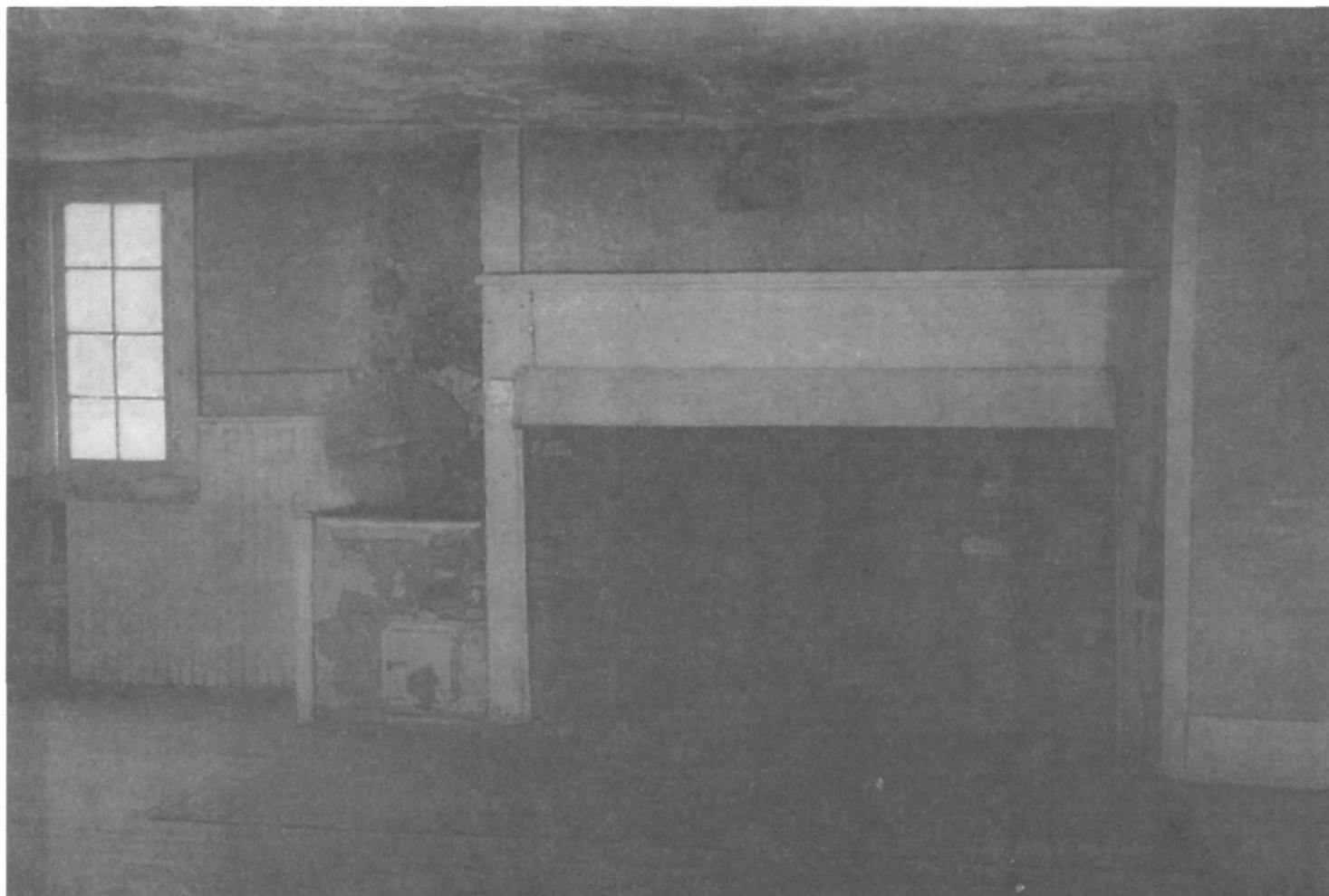
Figure 31. Schuyler House: Kitchen wing, east wall of kitchen (Room 105) before restoration (ca. 1955).
