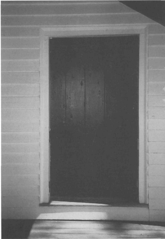
Figure 111. Kitchen wing, south elevation, doorway D104.
