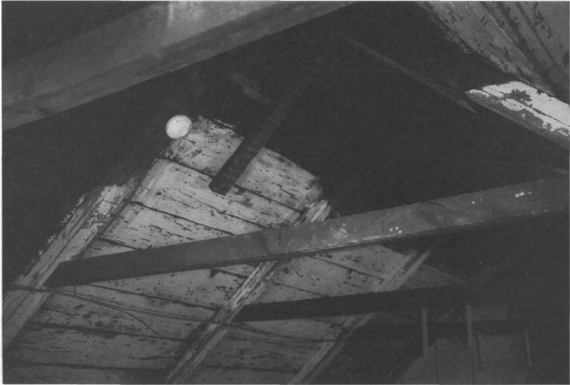
Figure 249. South attic room (Room 301), ceiling apex.
