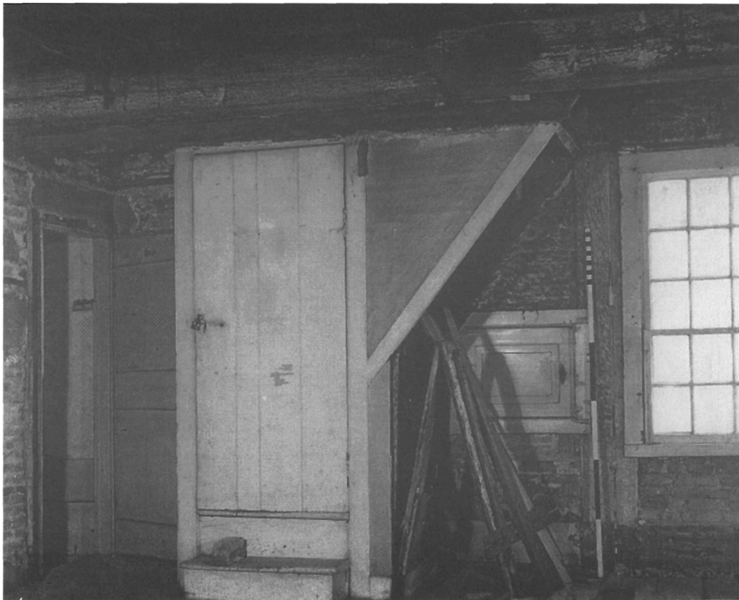
Figure 57. Schuyler House: First story of kitchen wing after ca.-1815 lath and plaster removed; ca.-1815 features at south end of west wall (1958). From left: doorway to east tier, doorway and staircase to second story, pass-through to dining-room pantry, and window in former ca.-1780 exterior doorway.
