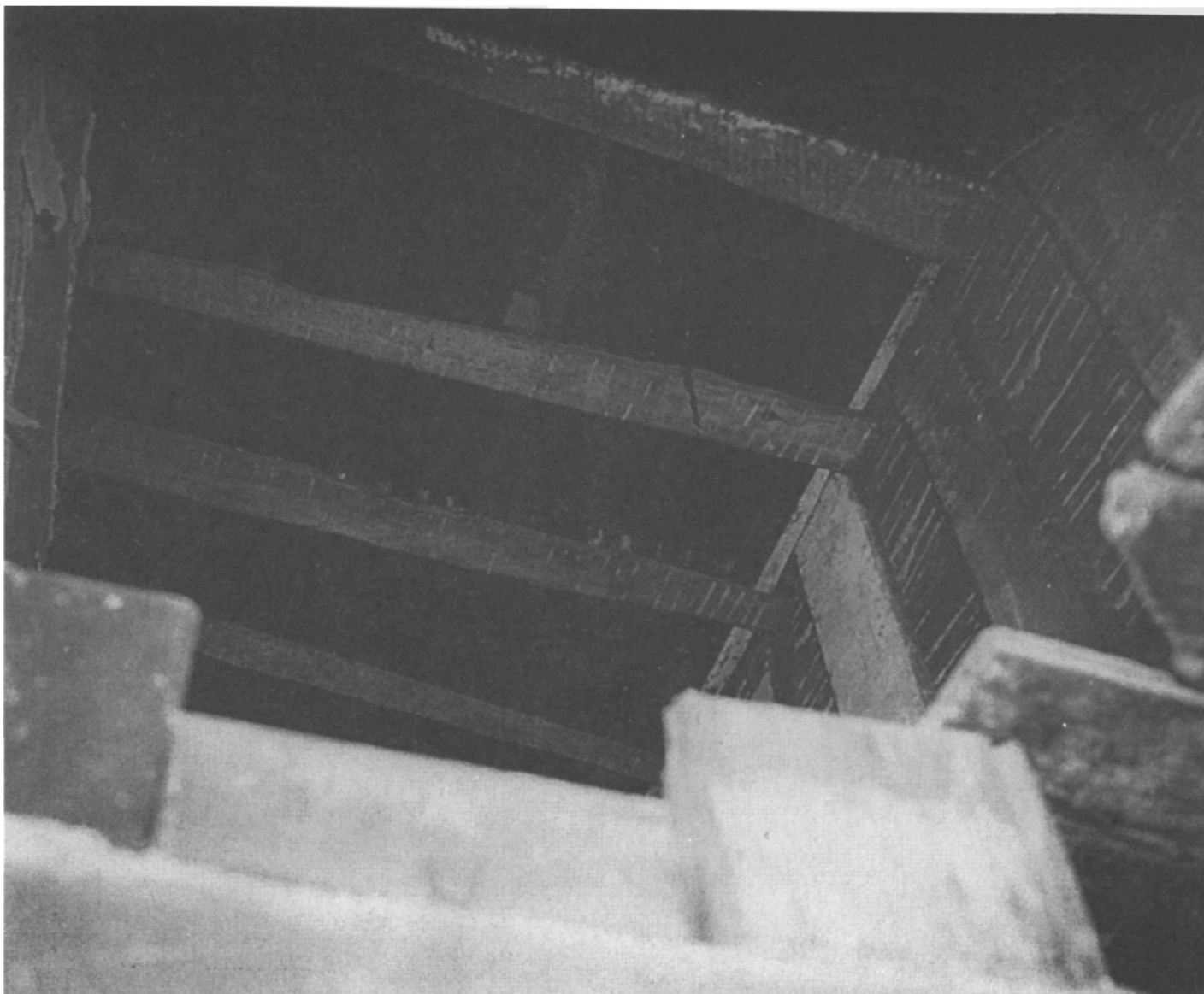
Figure 62. Schuyler House: Second story of kitchen wing after ca.-1815 lath and plaster removed; remnants of original newel post in hall (Room 206) at location of ca.-1780 staircase (1958).
