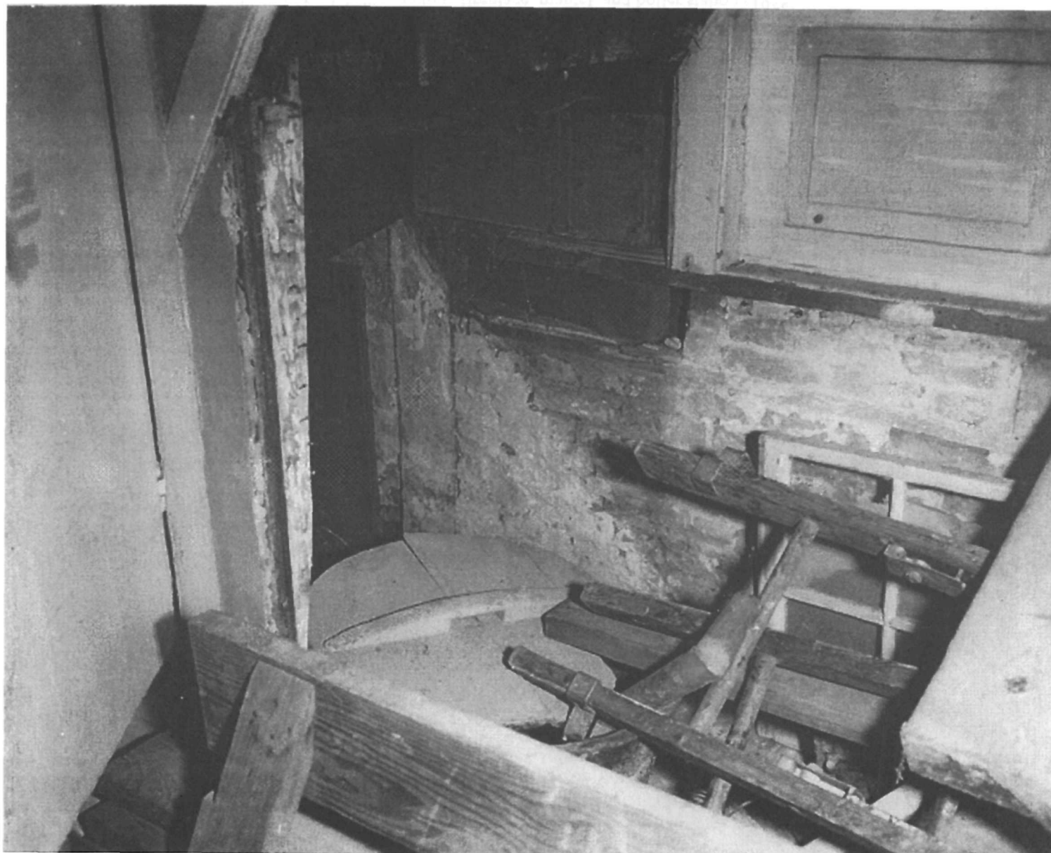
Figure 58. Schuyler House: First story of kitchen wing after ca.-1815 lath and plaster removed; west wall, area under ca.-1815 pass-through to dining-room pantry and paint line of original staircase to second story (1958).
