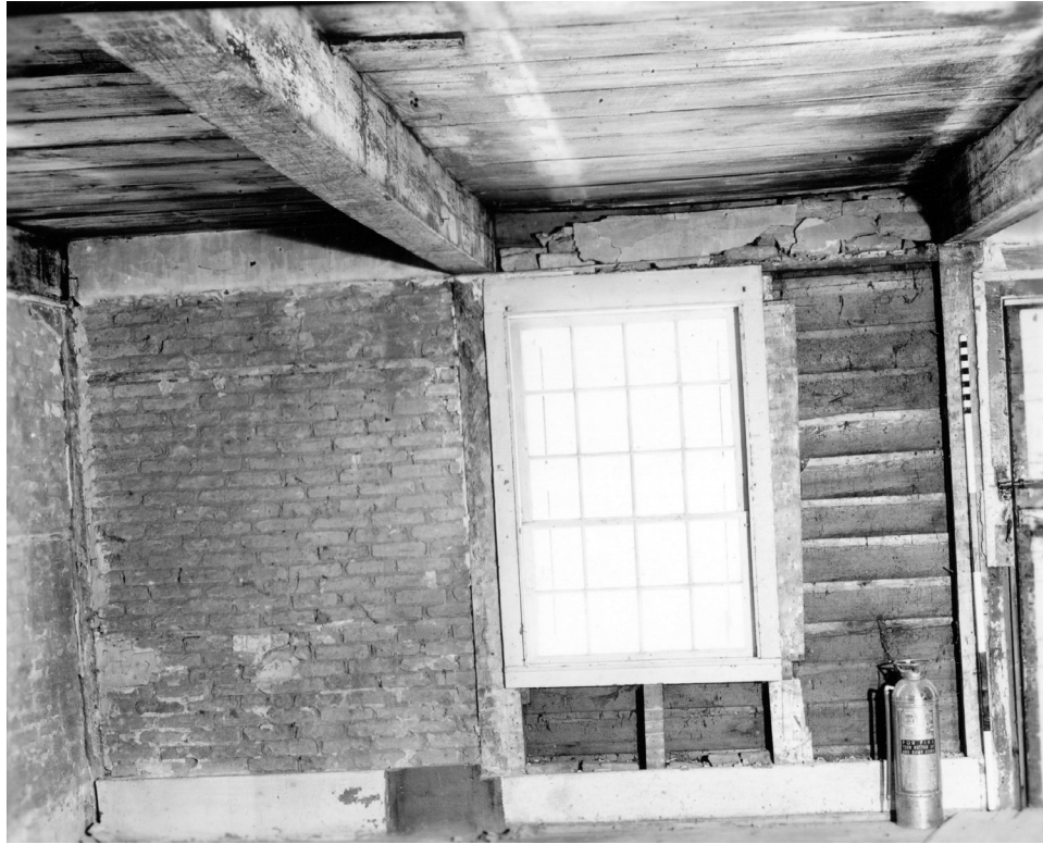
Figure 36. The north wall of the kitchen with original unfired brick nogging. Photograph by Henry Judd, 1958. SARA.
