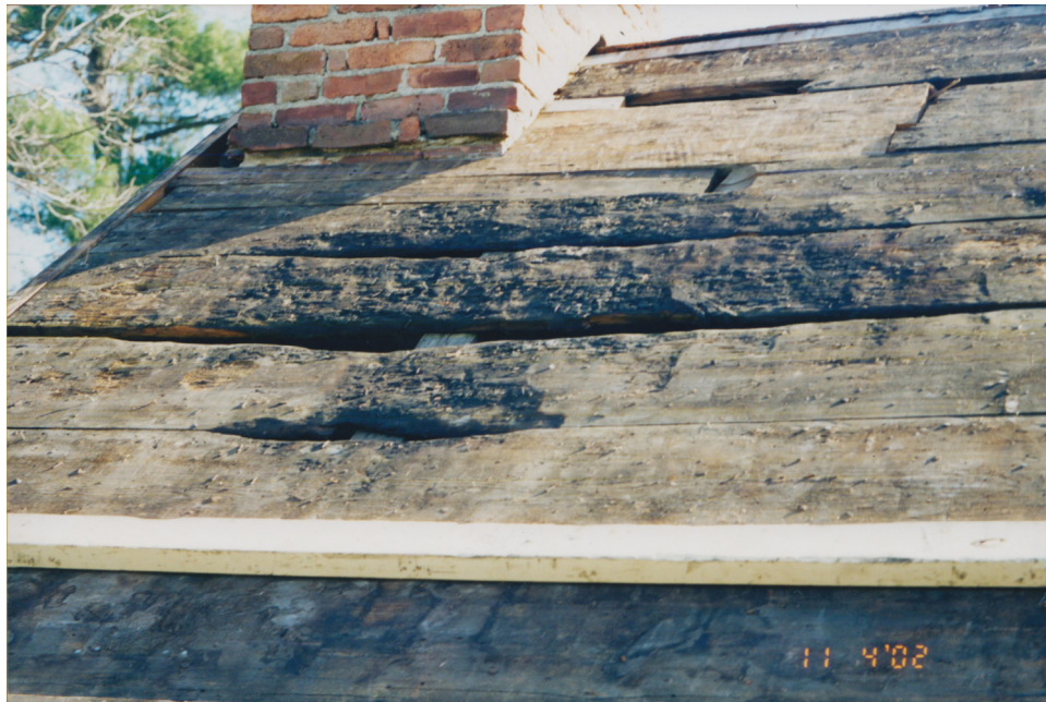
Figure 71. New cedar shingles were installed on the kitchen roof in 2002. Note the section of burned roof boards possibly relating to a chimney fire, revealed when the old shingles were removed. SARA, Box 41, Folder 7.
