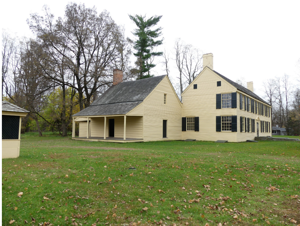
Figure 96. The Philip Schuyler House from the northwest. JGWA, 2020.
