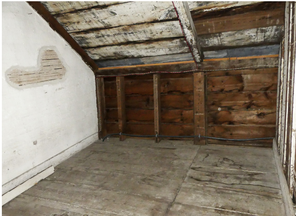
Figure 115. North room (208), looking north. Note that the brick nogging has been removed. JGWA, 2020.
