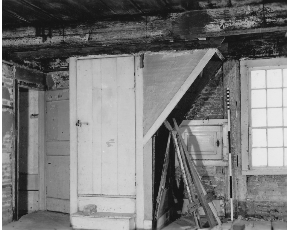
Figure 42. The nineteenth-century stair to the garret. Photograph by Henry Judd, 1958. SARA.
