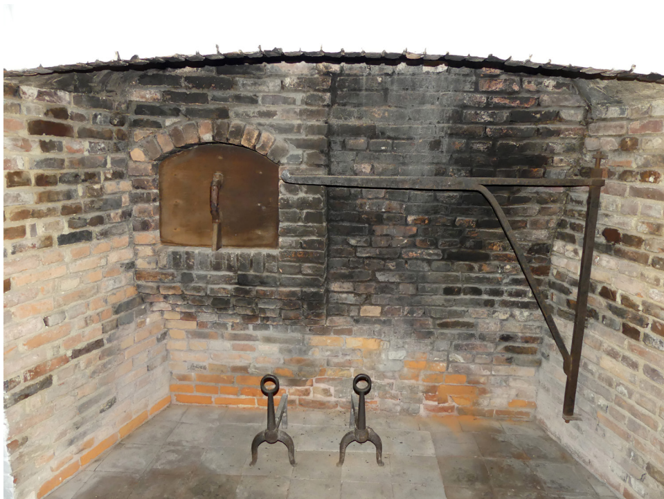
Figure 107. Kitchen firebox and oven. JGWA, 2020.
