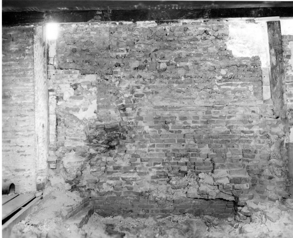
Figure 35. The fireplace after removals. An arched opening to a bake oven was found at the back of the firebox. Photographs by Gordon Whittington, 1958. SARA.
