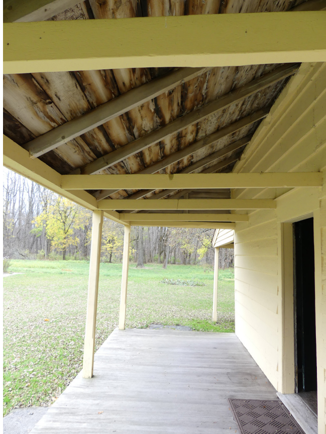
Figure 98. The north porch, looking east.
