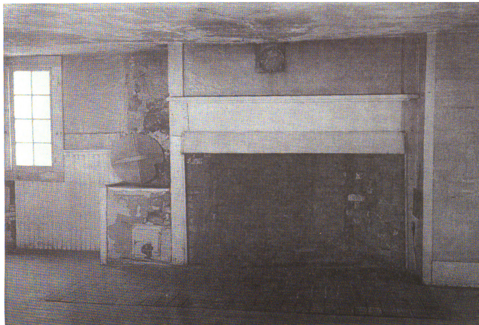
Figure 15. The kitchen circa 1955, looking east. Note the boiling pot and casement window north of the fireplace. A covered opening for the kitchen range flue pipe is visible above the mantle. 2003 HSR, p. 124.
