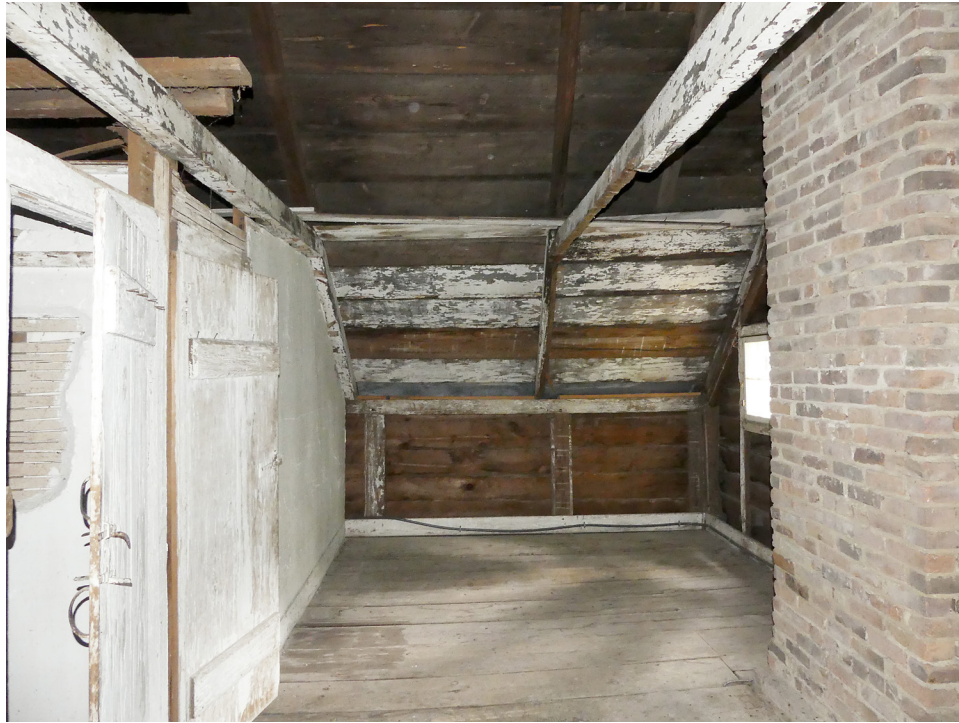
Figure 118. The East room, looking north. JGWA, 2020.
