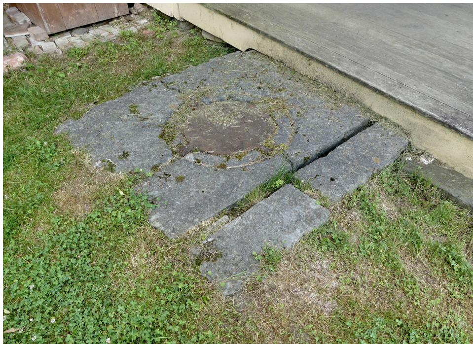
Figure 99. The drywell/cistern at the east end of the north porch.
