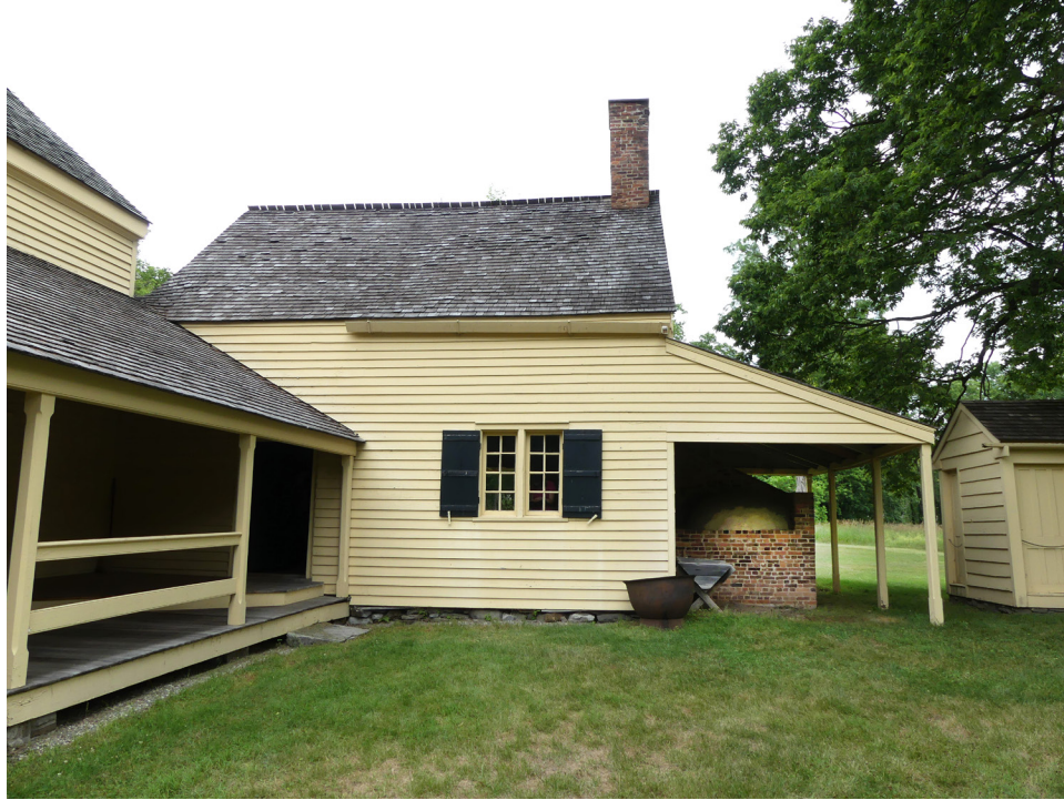
Figure 102. The kitchen wing from the south. JGWA, 2020.
