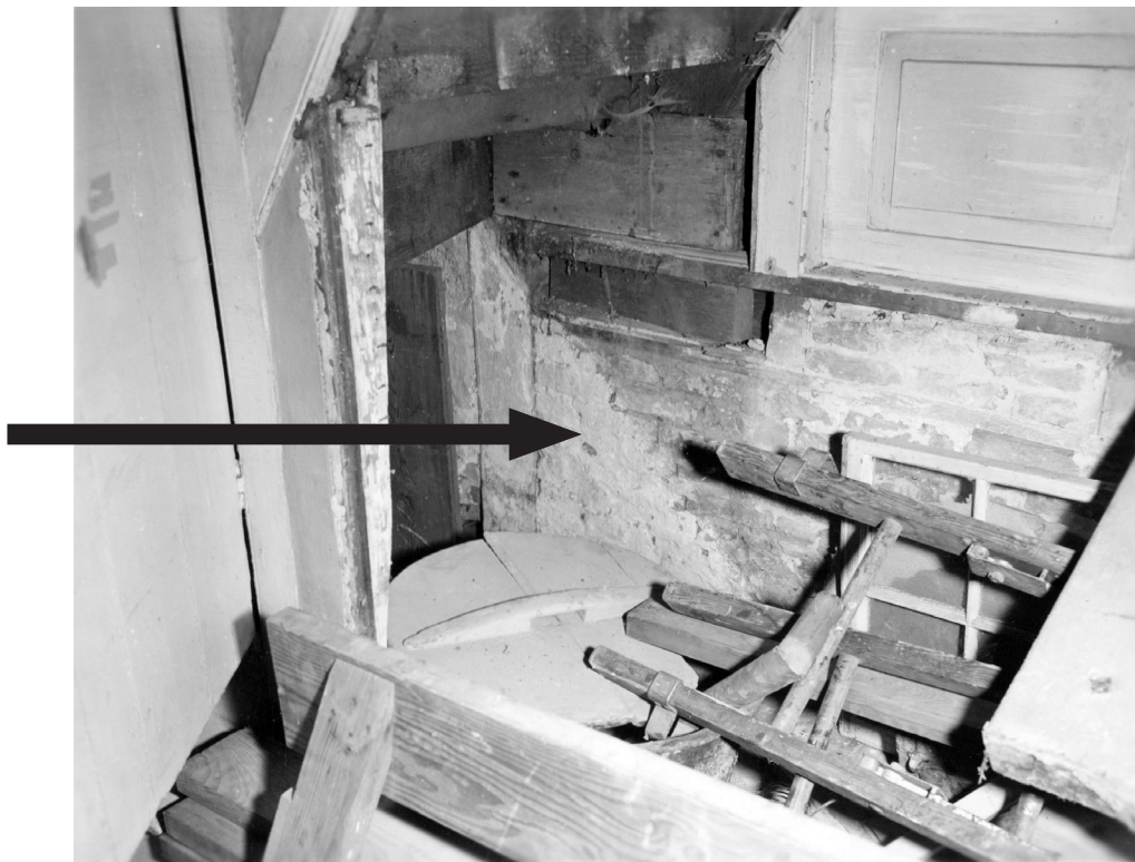
Figure 43. Ghost of the original stair to the garret. Photograph by Charles Hutchins, 1958. SARA.
