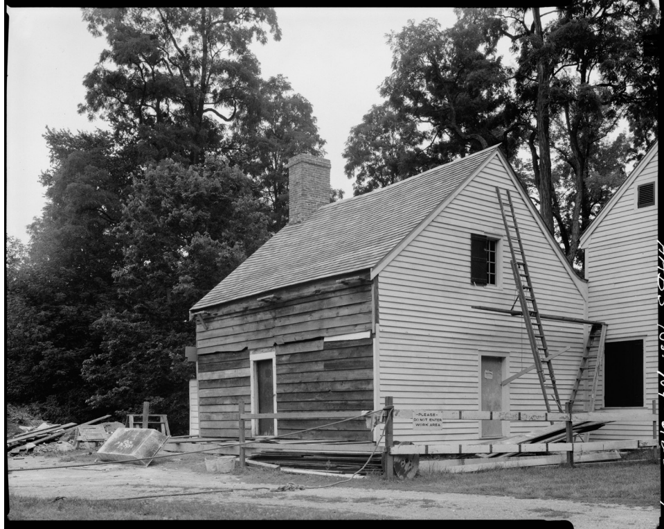
Figure 66. The kitchen wing under construction in 1963. Photograph by Jack Boucher. Library of Congress, HABS No. NY-6122-4.
