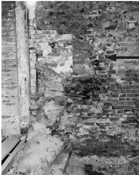
Figure 35. The fireplace after removals. An arched opening to a bake oven was found at the back of the firebox. Photographs by Gordon Whittington, 1958. SARA.
