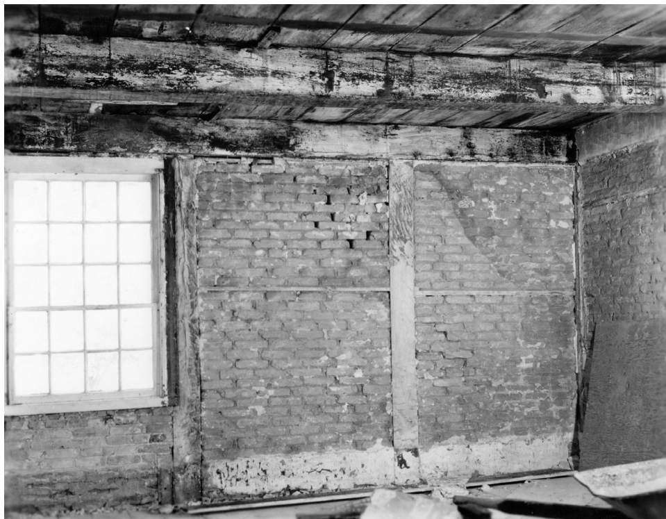
Figure 37. The west wall of the kitchen with original unfired brick nogging. The window opening replaced an original doorway. Photograph by Henry Judd, 1958. SARA.
