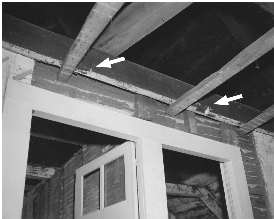
Figure 45. The evidence for the original doorway into the center garret room—marks for the door framing in the joist—was found in 1958 when the plaster and lath were removed from the east partition in the stair hall. Photograph by Charles Hutchins, 1958. SARA.
