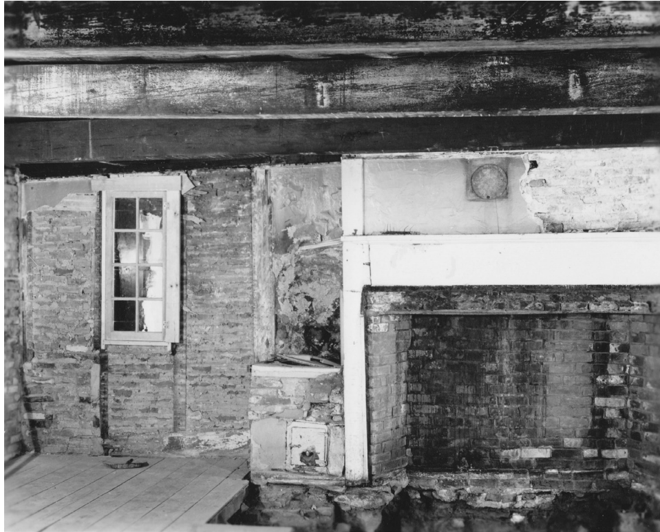
Figure 34. The east wall of the kitchen in 1958, before removal of the later fireplace and boiling pot. Photograph by Henry Judd, 1958. SARA.
