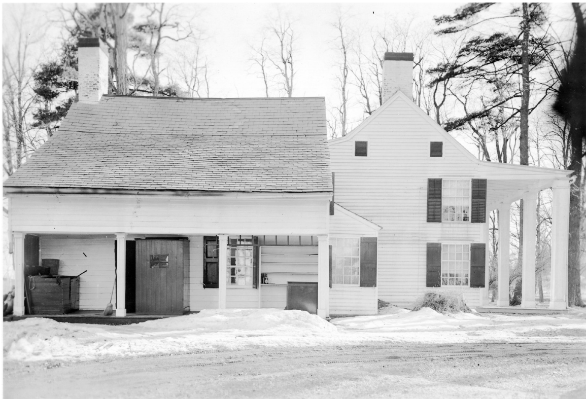
Figure 13. The Schuyler House and kitchen in 1947. The upper part of the kitchen porch is enclosed, and a small enclosed addition to the west connects the kitchen to the dining room. Note the weather vestibule that protects the door into the kitchen. SARA, 22345.
