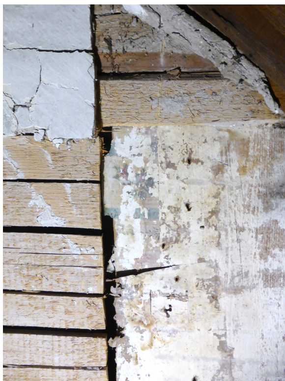
Figure 116. North room (208) wallpaper probe. A section of plaster was removed from one of the board “studs” to reveal early nineteenth-century wallpaper remnants on the vertical wood plank partition. JGWA, 2021.
