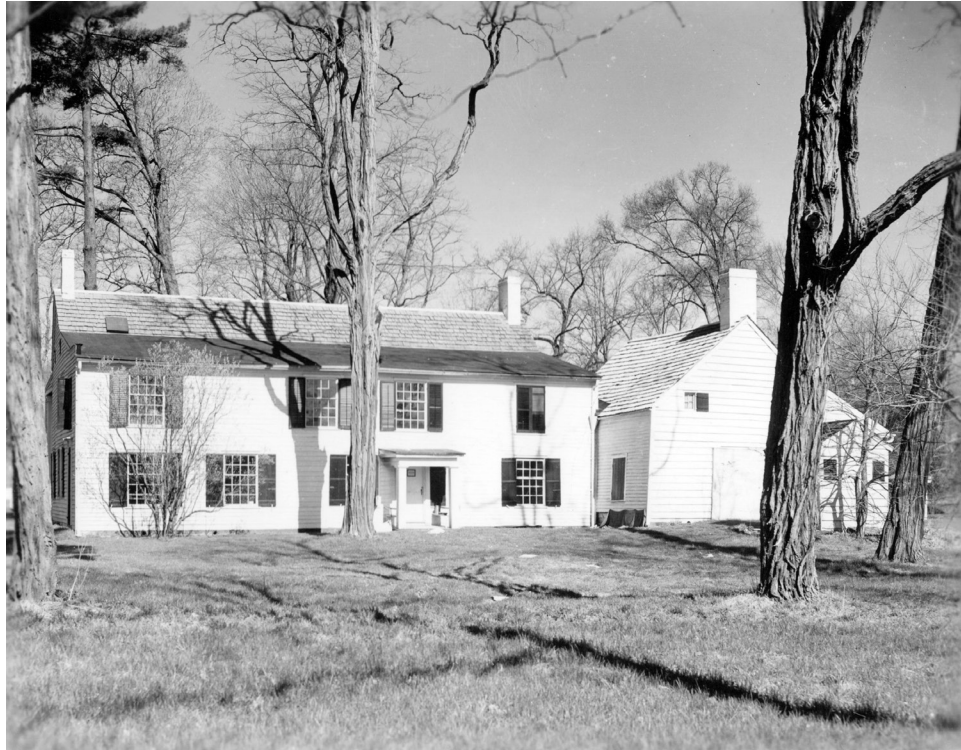
Figure 18. A rare view of Schuyler House from the east, showing the two-story addition along the east facade. The small structure east of the kitchen wing is the privy. Photograph by Henry Judd, July, 1956. SARA.
