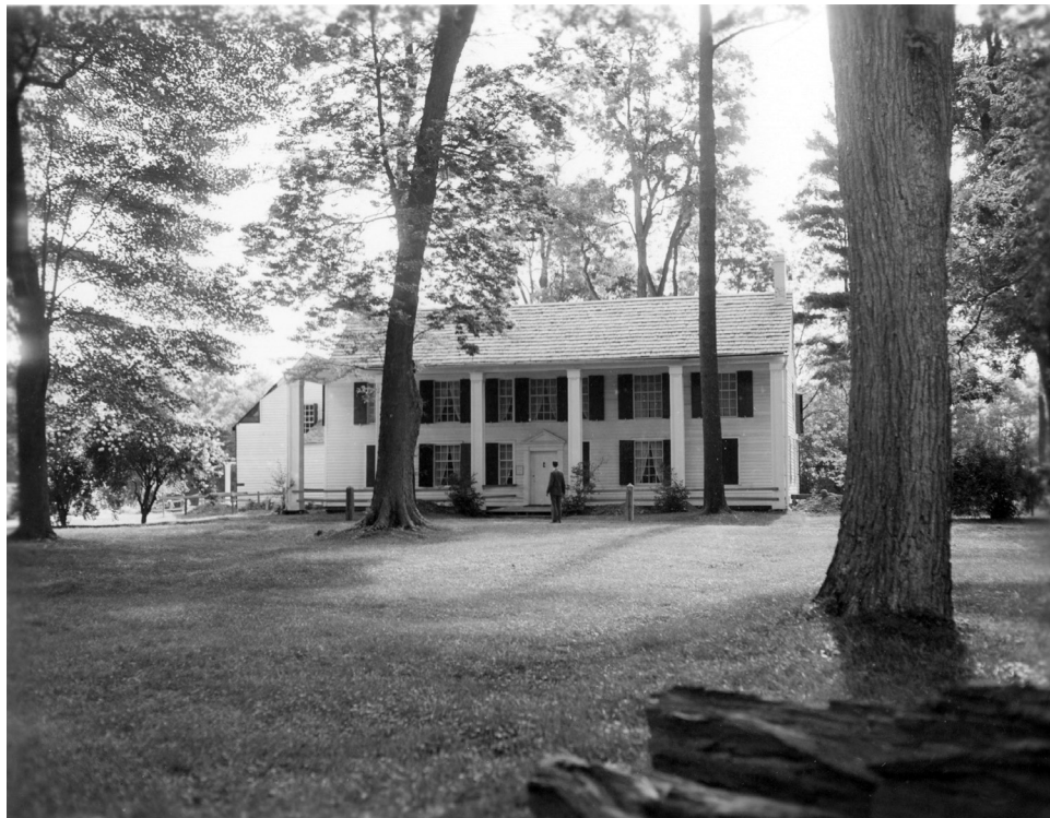
Figure 19. Schuyler House in August, 1958; photograph by Henry Judd. SARA.
