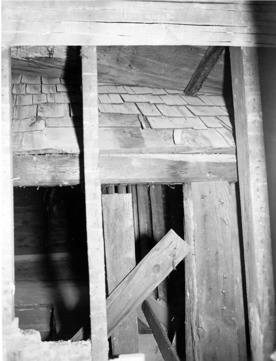
Figure 33. A section of original wood shingles on the south slope of the kitchen roof "where covered by the cricket." Photograph by Henry Judd, 1958. SARA.
