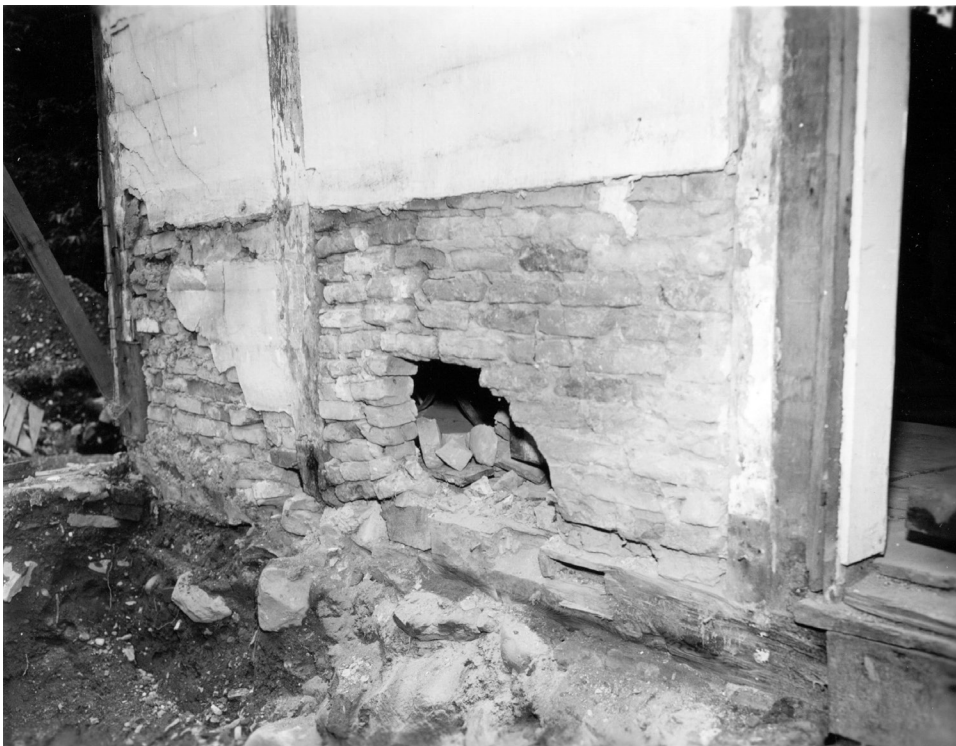
Figure 41. The nogging in the north wall, from the exterior. Note the plaster finish. Photograph by Charles Hutchins, 1958. SARA.
