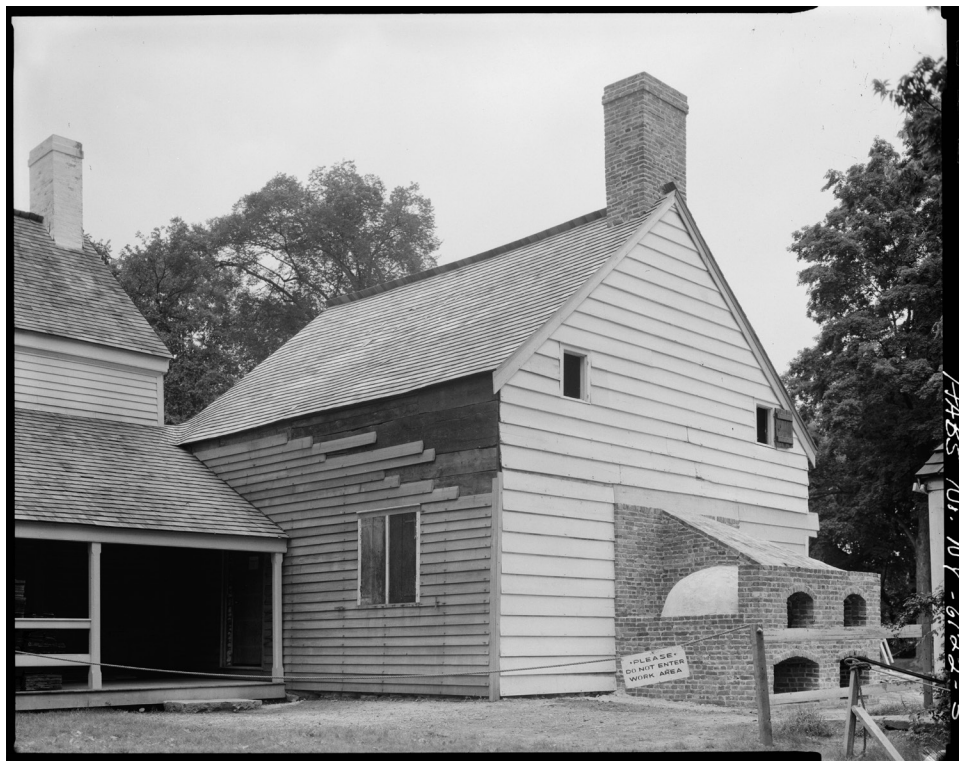
Figure 67. The kitchen wing under construction in 1963. Photograph by Jack Boucher. Library of Congress, HABS No. NY-6122-5.
