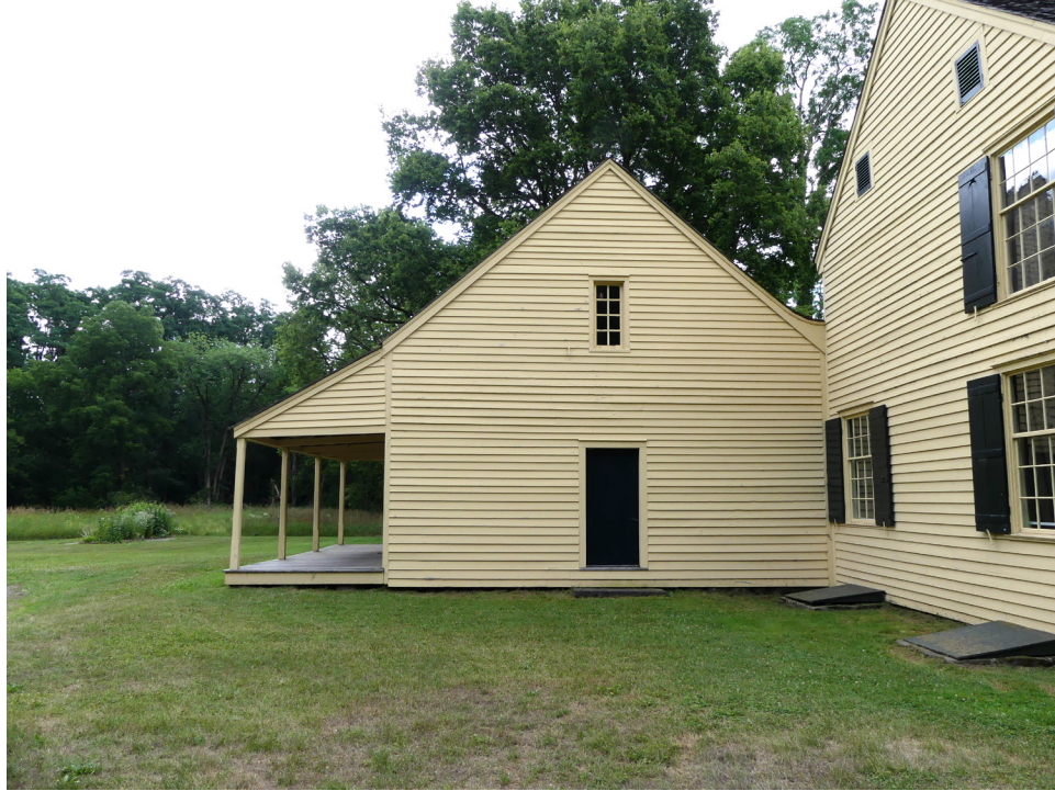
Figure 105. The kitchen wing from the west. JGWA, 2020.
