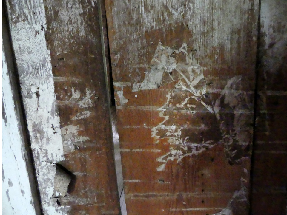
Figure 113. Fragments of eighteenth-century wallpaper on the boards forming the east partition of the south room (207). JGWA, 2020.
