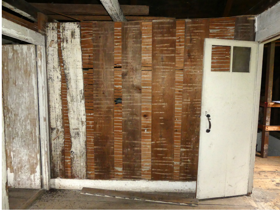
Figure 114. North room (208), looking south. JGWA, 2020.
