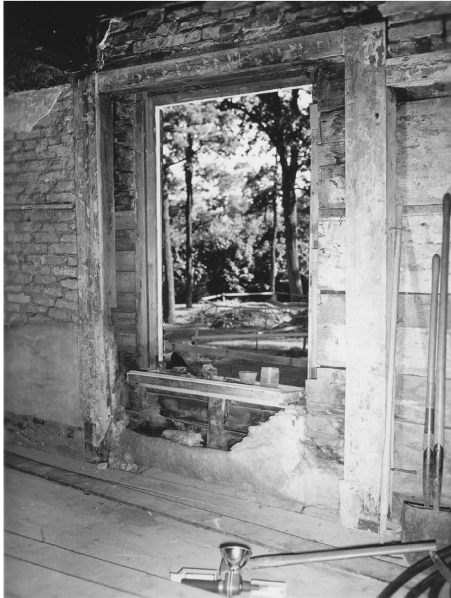
Figure 40. The original window opening found in the south wall of the kitchen. Photograph by Charles Hutchins, 1958. SARA.
