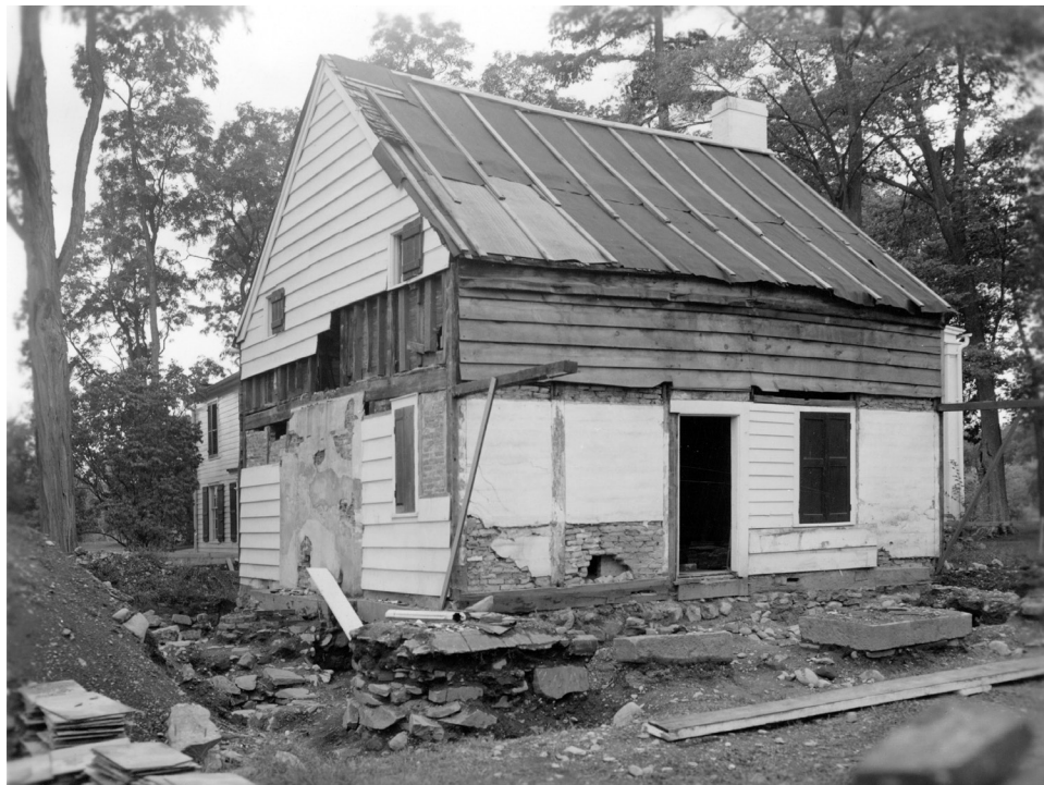
Figure 31. The kitchen after excavations and removals, July, 1958. The unfinished boards along the top of the north facade were thought to be original and never painted. Note the plaster applied directly to the nogging on the north facade in the two bays east of the door and the bay west of the window. Photograph by Charles Hutchins. SARA.
