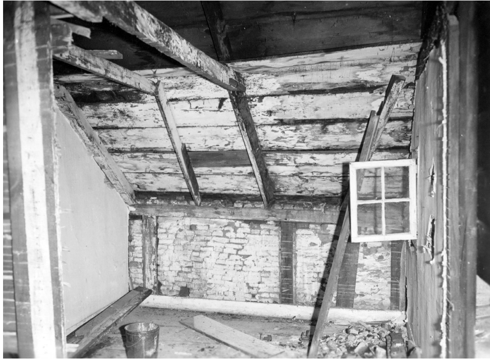
Figure 46. The south garret room in 1958. Note the later partition to the left that divided the east space into two rooms, and the brick nogging that was removed in the 1963 restoration. Photograph by Charles Hutchins. SARA.
