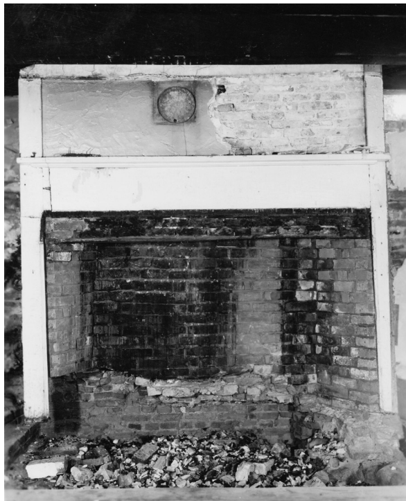
Figure 34. The east wall of the kitchen in 1958, before removal of the later fireplace and boiling pot. Photograph by Henry Judd, 1958. SARA.
