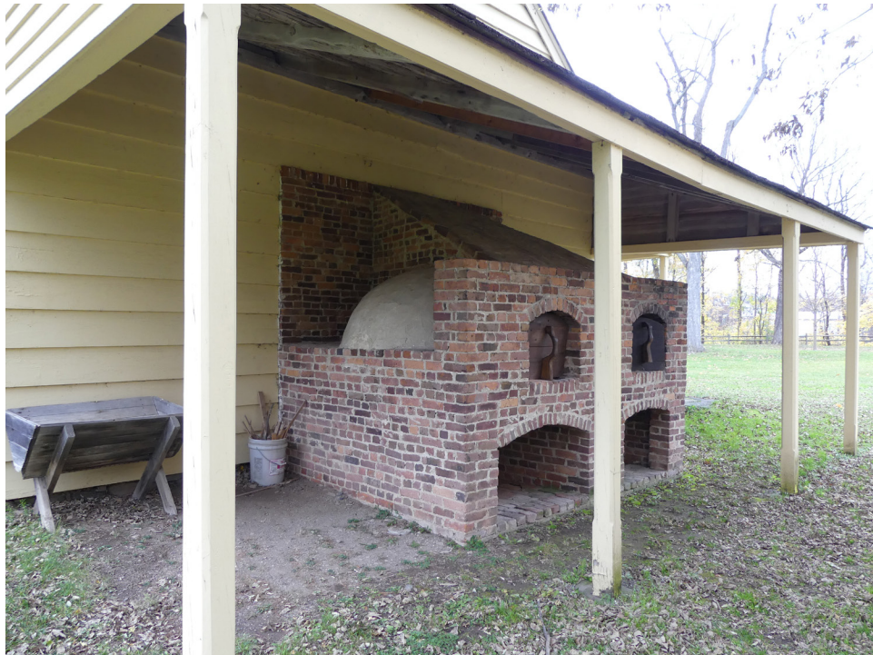
Figure 101. The 1950s ovens on the east side of the wing. JGWA, 2020.
