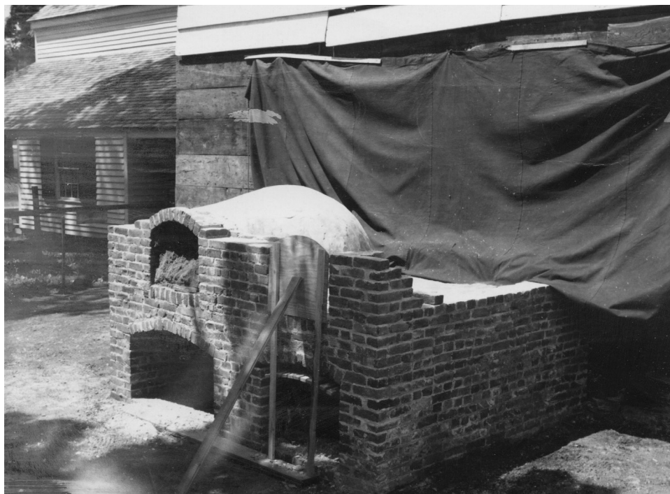
Figure 68. The oven under construction, 1963. SARA, Box 91, Folder 7.
