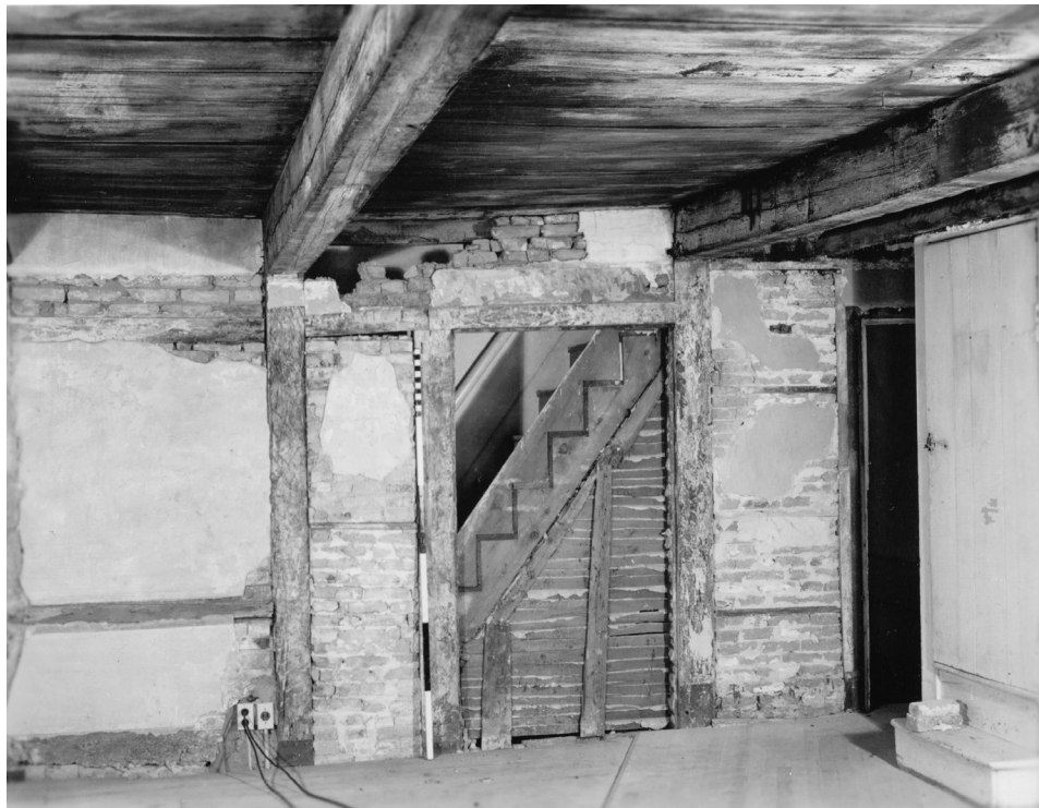
Figure 39. The south wall of the kitchen. The enclosed winding stair to the garret is to the right. The stair within the nineteenth-century two-story addition can be seen beyond the doorway. Photograph by Henry Judd, 1958. SARA.
