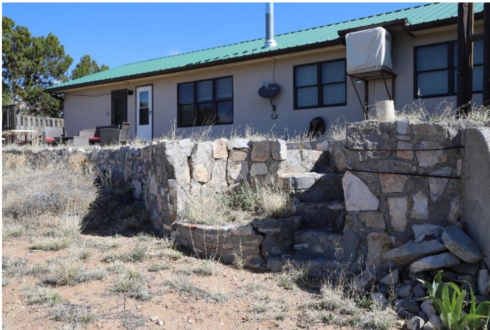
Figure 17 Residence 13 Stone Retaining Wall / Facing Northwest, April 2024
