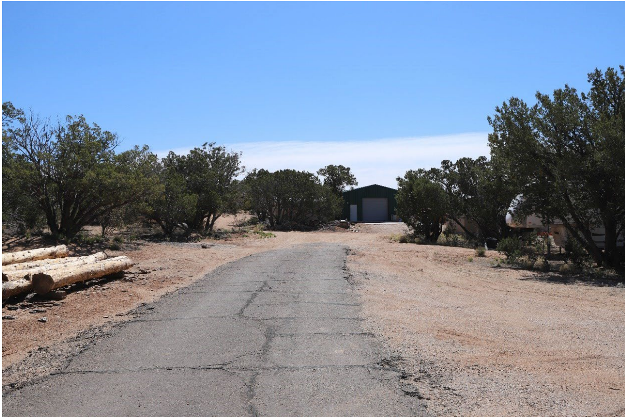
Figure 14 Maintenance Road toward Utility Building / Looking North-East, April 2024
