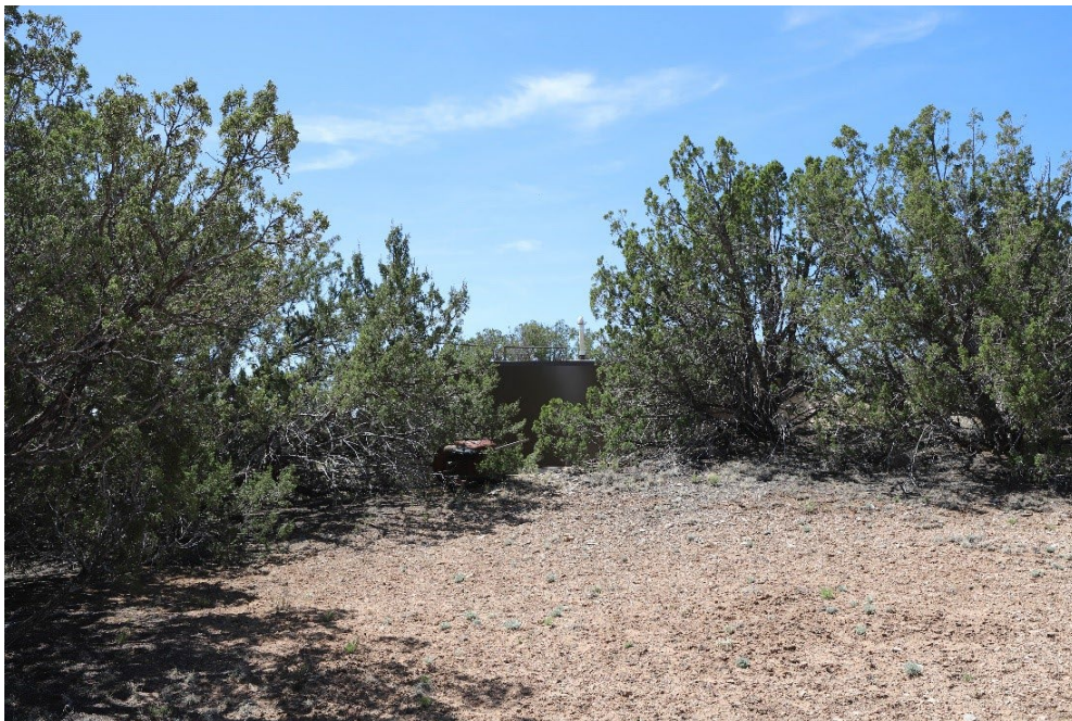
Figure 24 Water Storage Tank / Looking North, April 2024
