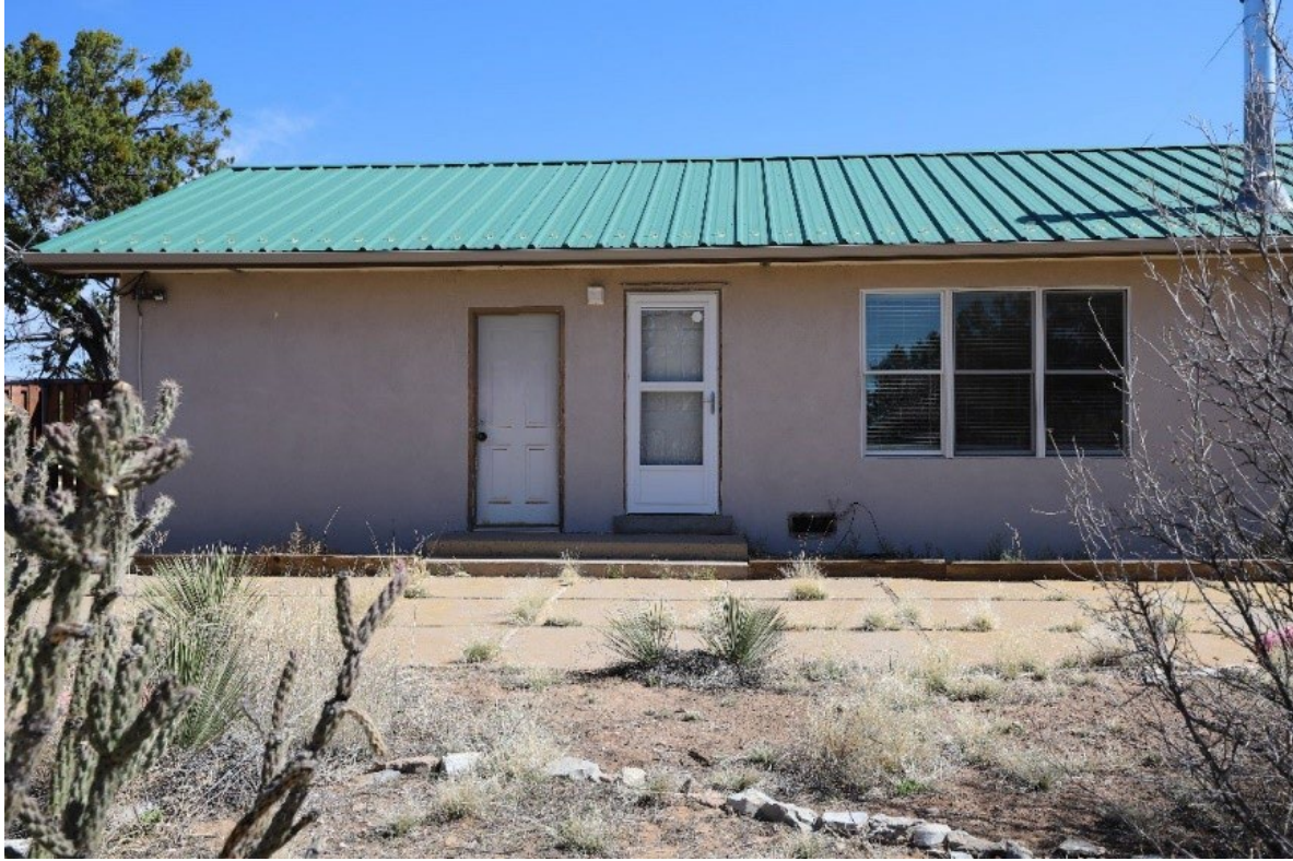
Figure 20 Residence 12 Rear Elevation, April 2024
