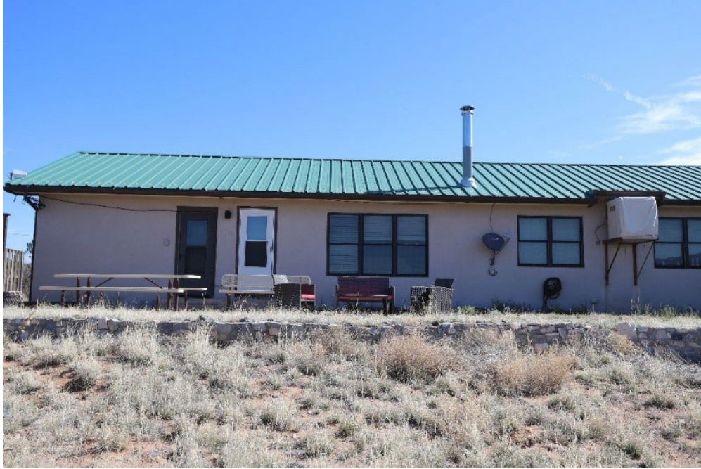
Figure 16 Residence 13 Rear Elevation and Retaining Wall/ Facing North, April 2024
