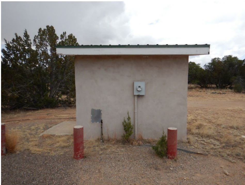
Figure 35 North Wall of Well House straight ahead, May 2025.
