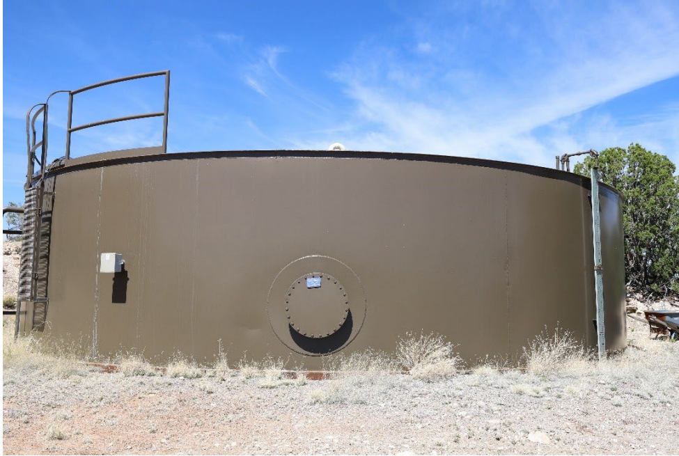
Figure 25 Water Storage Tank / Looking South, April 2024
