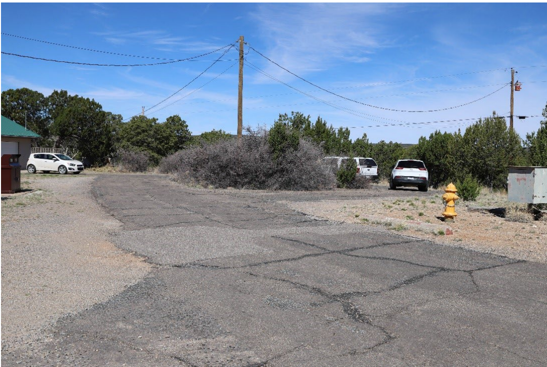
Figure 13 Residential Loop / Facing East, April 2024
