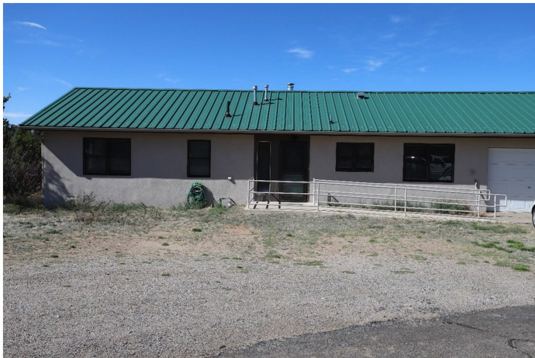
Figure 42 Residence 13, note how change in roofline alters overall design, feeling, and association of the property. Source: NPS, April 2024.
