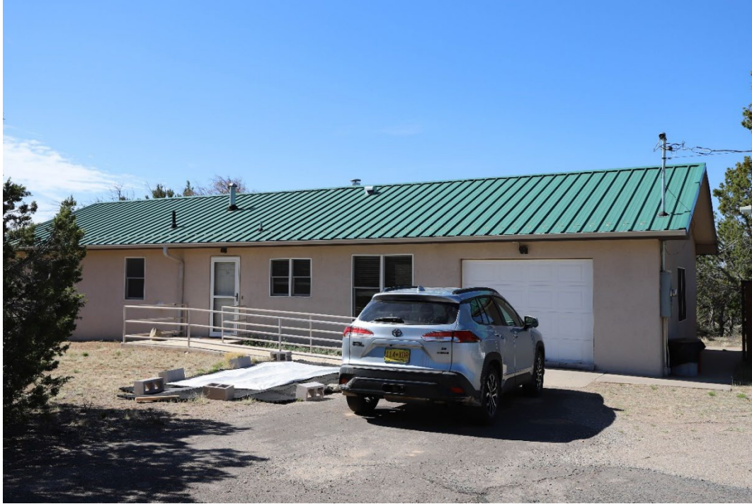
Figure 43 Residence 12- Note material changes and roofline alteration. Source: NPS April 2024.
