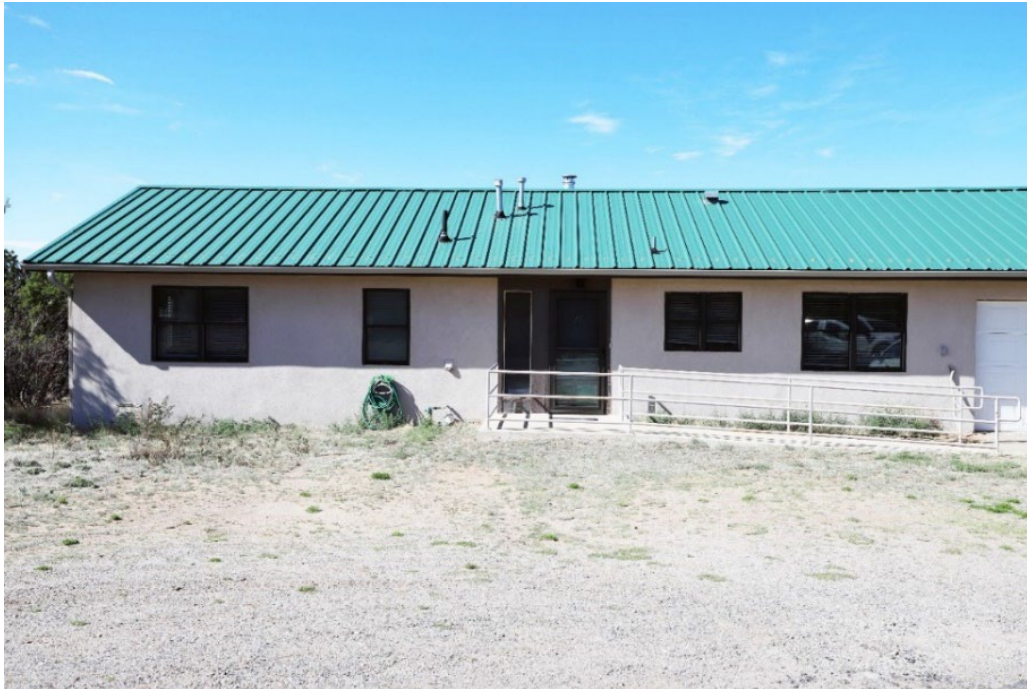
Figure 15 Residence 13 Front Facade / Facing Southwest, April 2024
