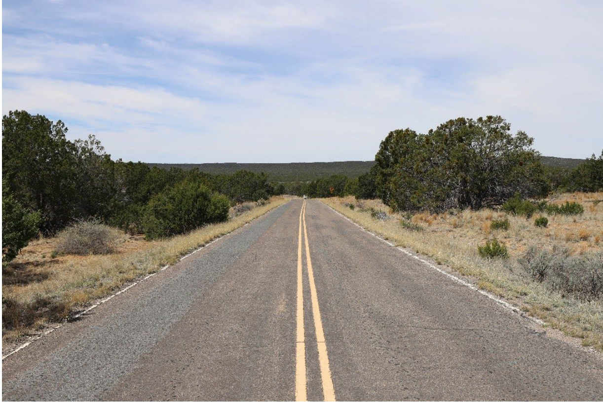
Figure 6 Entrance Road Framed by Native Vegetation / Looking West, April 2024
