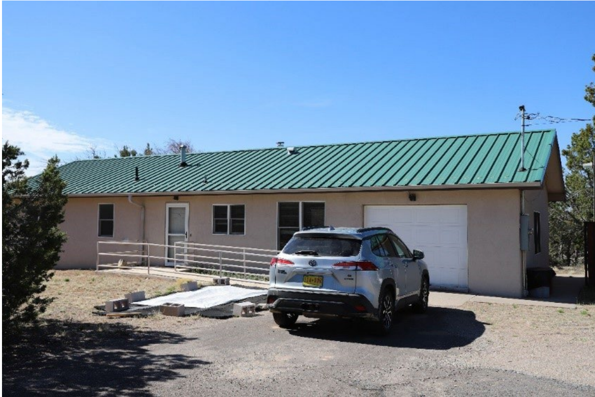
Figure 18 Residence 12 Front Facade / Oblique View, April 2024
