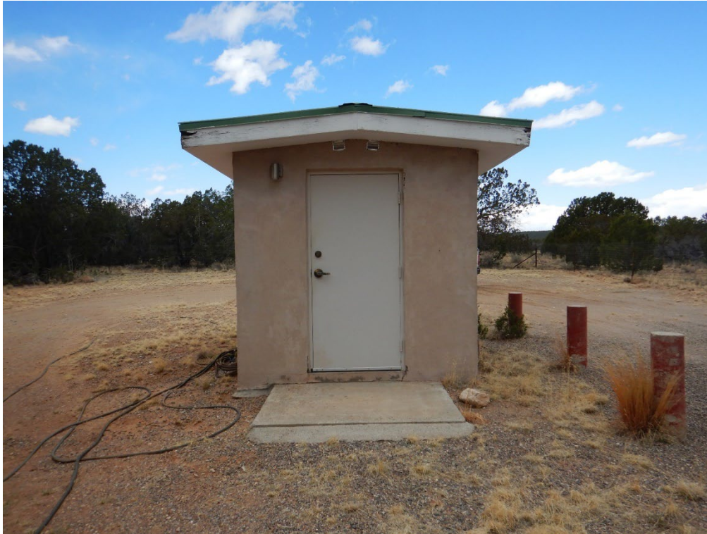
Figure 34 Well house entrance straight ahead, May 2025
