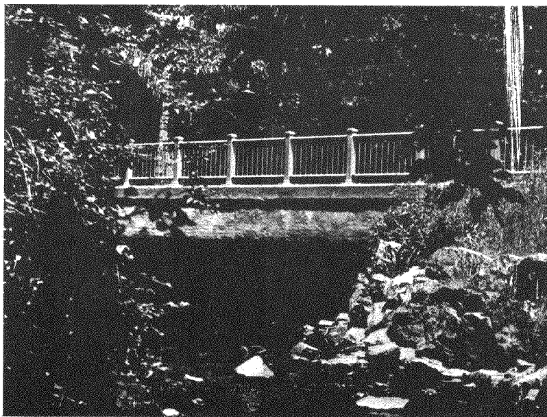
As the Bridge Over the Hutchinson Looks Today
