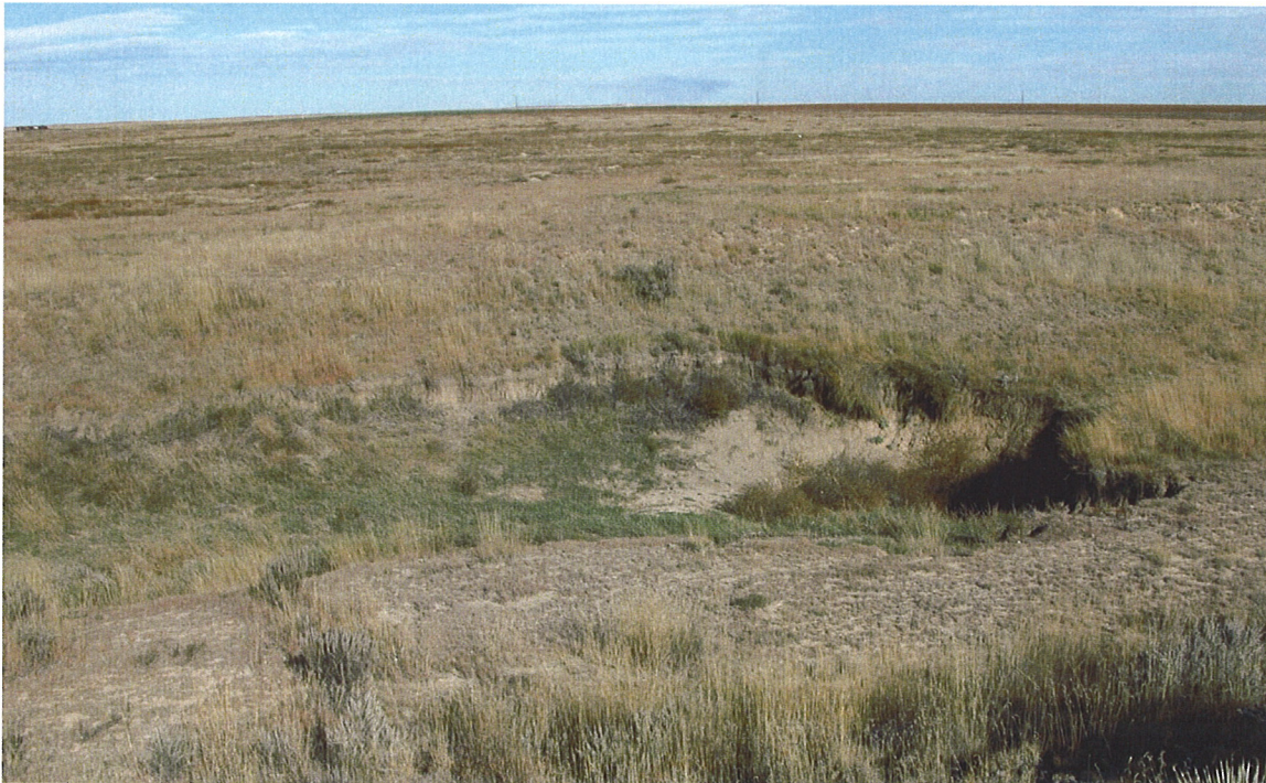
Figure 4: Head Cut Erosion within Canal Channel
