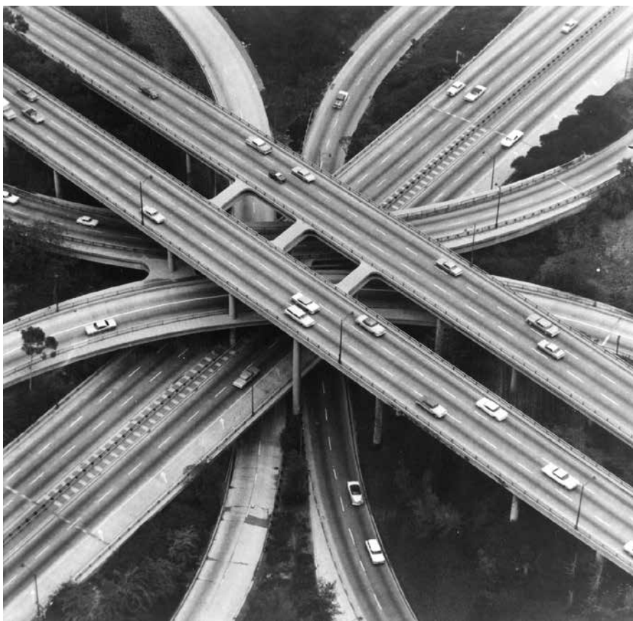
The four-level interchange that is part of the Arroyo Seco Parkway was an innovation in highway engineering as the “world’s first freeway-to-freeway connector.” Photo: Modernage Photo Service, Inc., Security Pacific National Bank Collection/Los Angeles Public Library.
