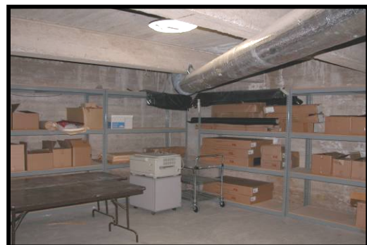
Central Hall Basement room.
