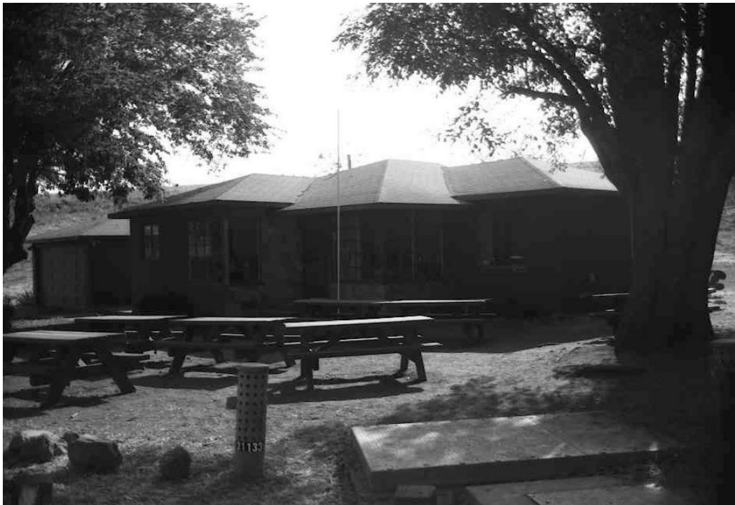
Buildings and Structures #9: A view of the noncontributing residence (old Danielson/Satwiwa Cultural Center building, NPS #402). (PGSO, CLI, SAMO-N-0006-5, 2002)
