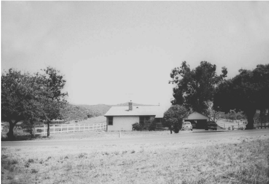
Vegetation #4: A view of the caretaker's residence and surrounding contributing vegetation. (PGSO, CLI, SAMO-N-0005-5, 2002)
