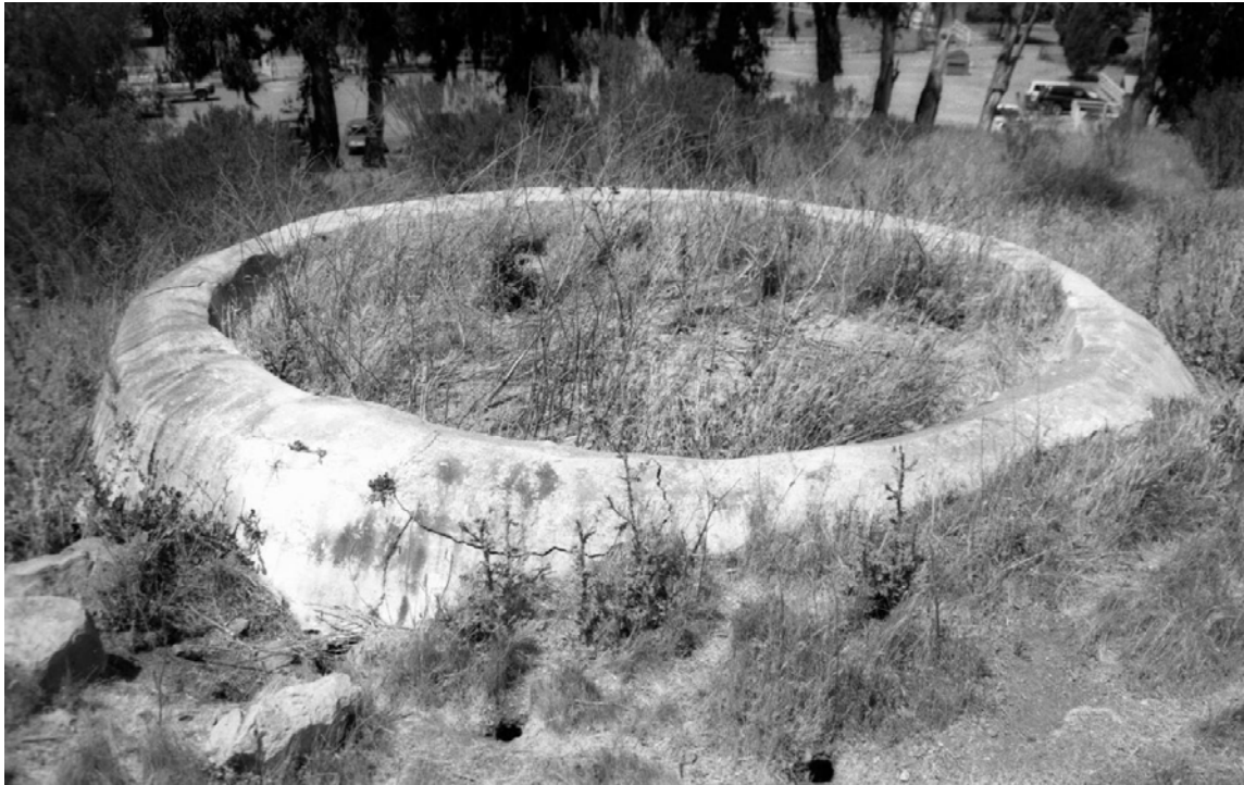
Small Scale Features #5: A view of the contributing concrete cistern. (PGSO, CLI, SAMO-N-0004-6, 2002)
