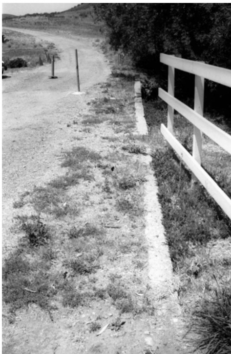
Circulation #3: A view down the contributing main entry road. (PGSO, CLI, SAMO-N-0004-4, 2002)
