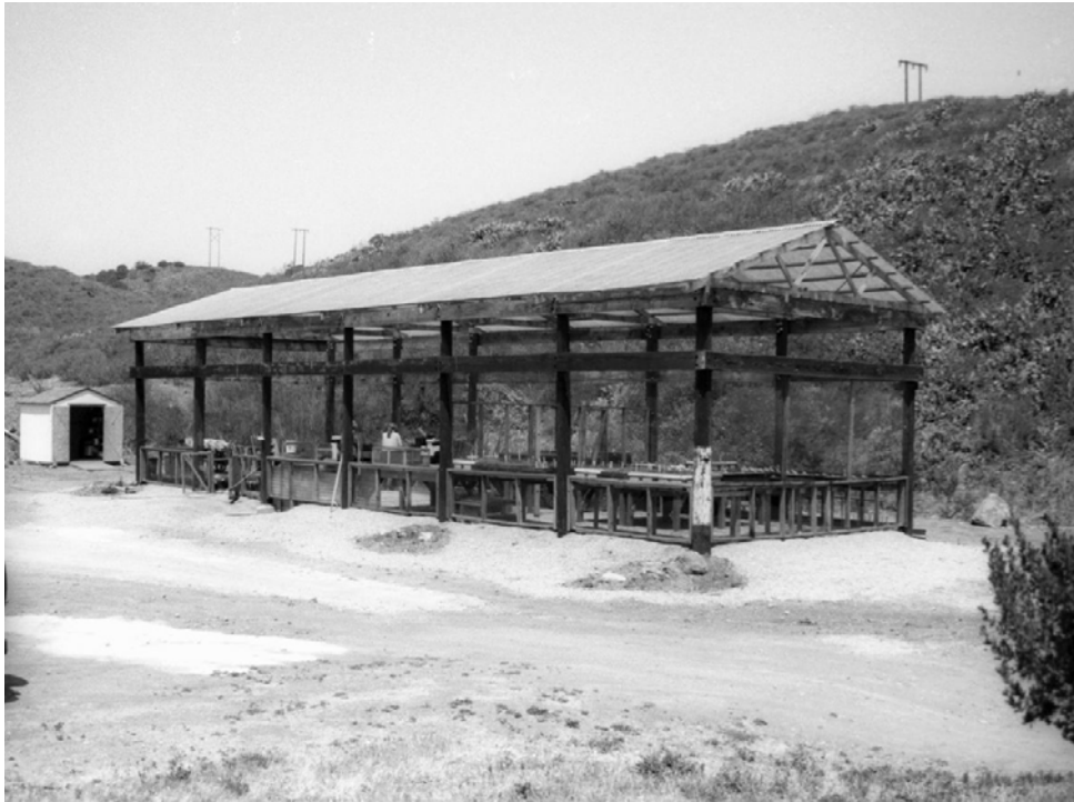
Buildings and Structures #8: A view of the noncontributing planting barn (no NPS #), note the shed in the background to the left. (PGSO, CLI, SAMO-N-0003-24, 2002)
