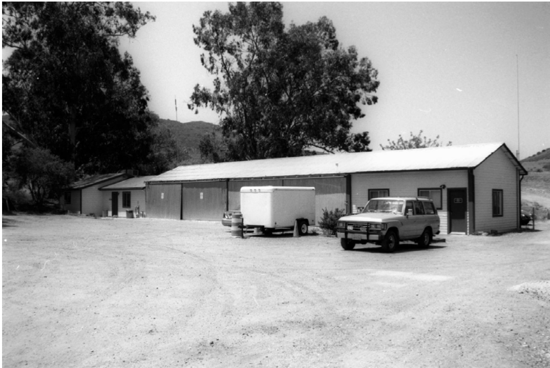
Buildings and Structures #3: A view of the contributing equipment shed (NPS# 108-408). (PGSO, CLI, SAMO-N-0004-0, 2002)
