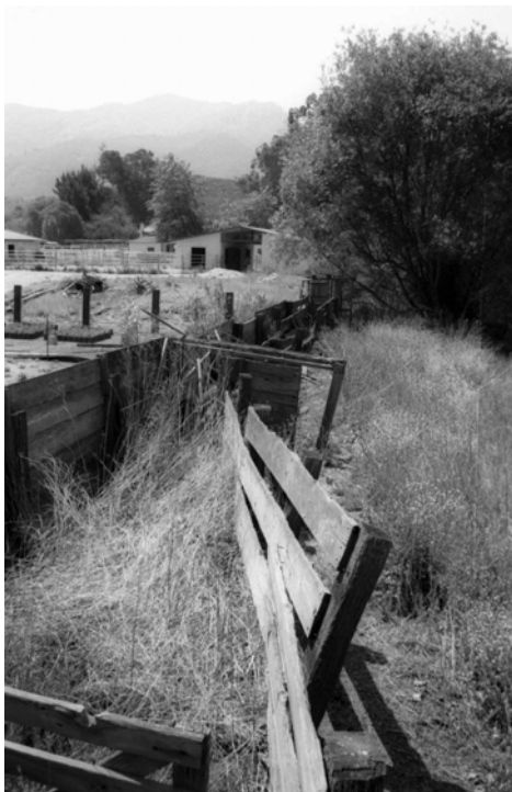
Small Scale Features #2: A detail view of the contributing chute along the eastern fence of the corral remains. (PGSO, CLI, SAMO-N-0003-19, 2002)
