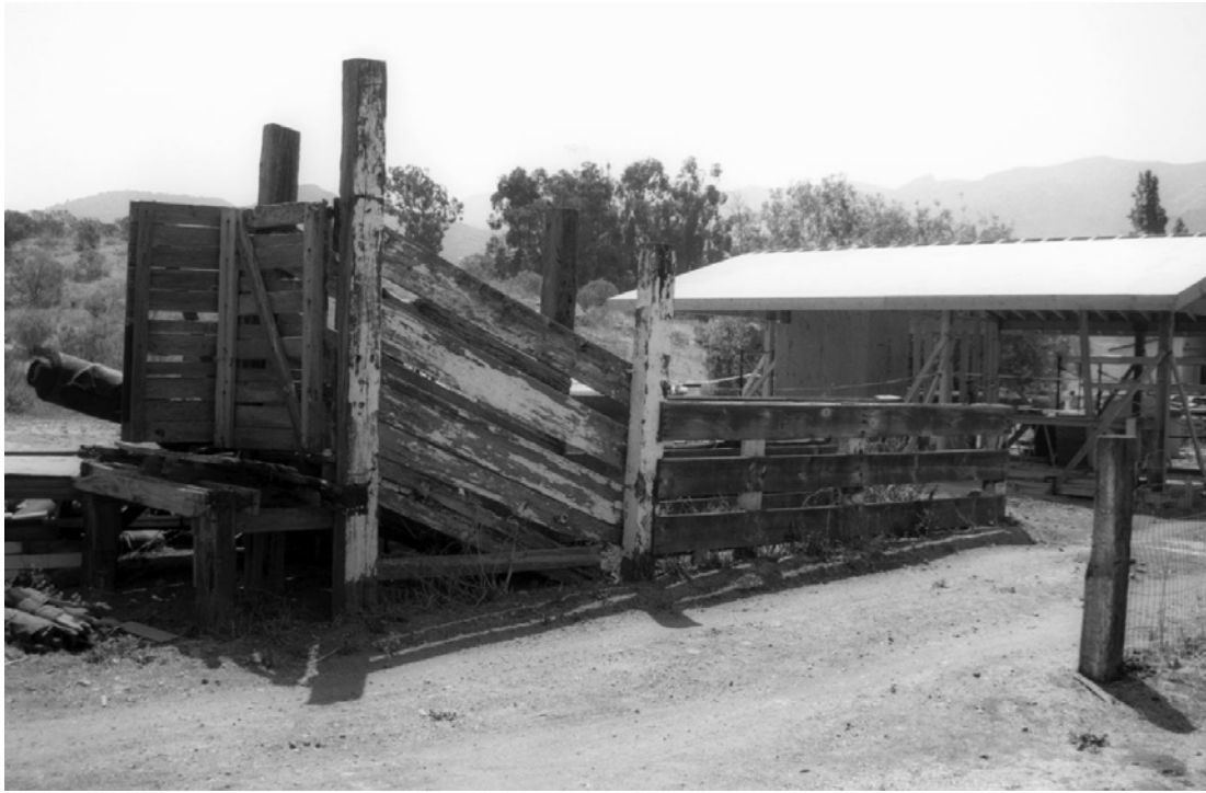
Small Scale Features #3: A view of the remains of a contributing chute, note the new shed in the background. (PGSO, CLI, SAMO-N-0003-16, 2002)
