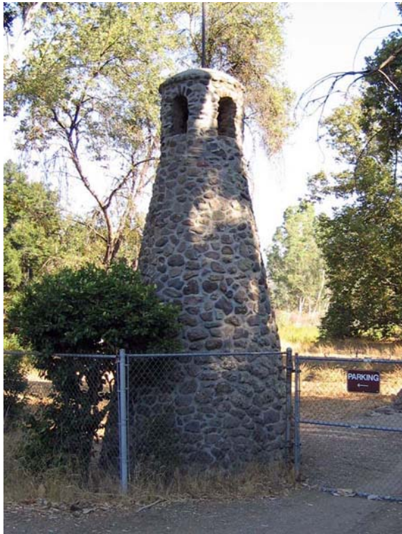
Buildings and Structures Photo #3. The gate tower was constructed by Harry Miller served as an entry to the property. (PWRO 2005)
