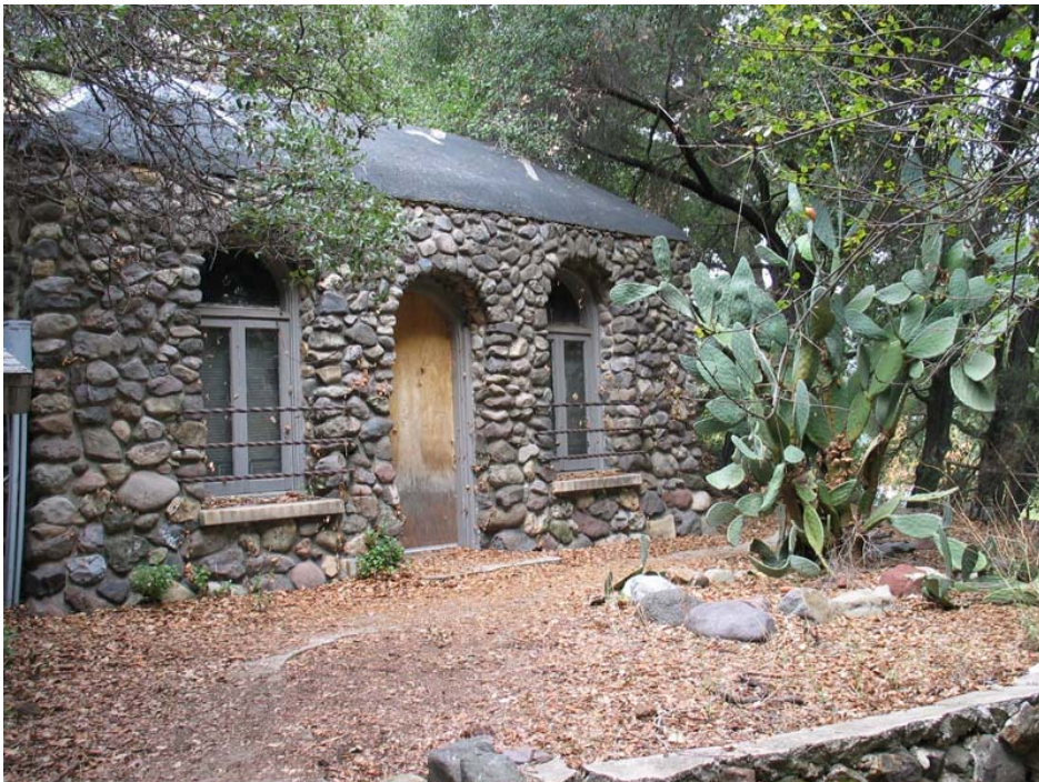
Buildings and Structures Photo #2. The radio house is constructed of mortared river stone with arched door and window openings and a hipped concrete roof. (PWRO 2005)
