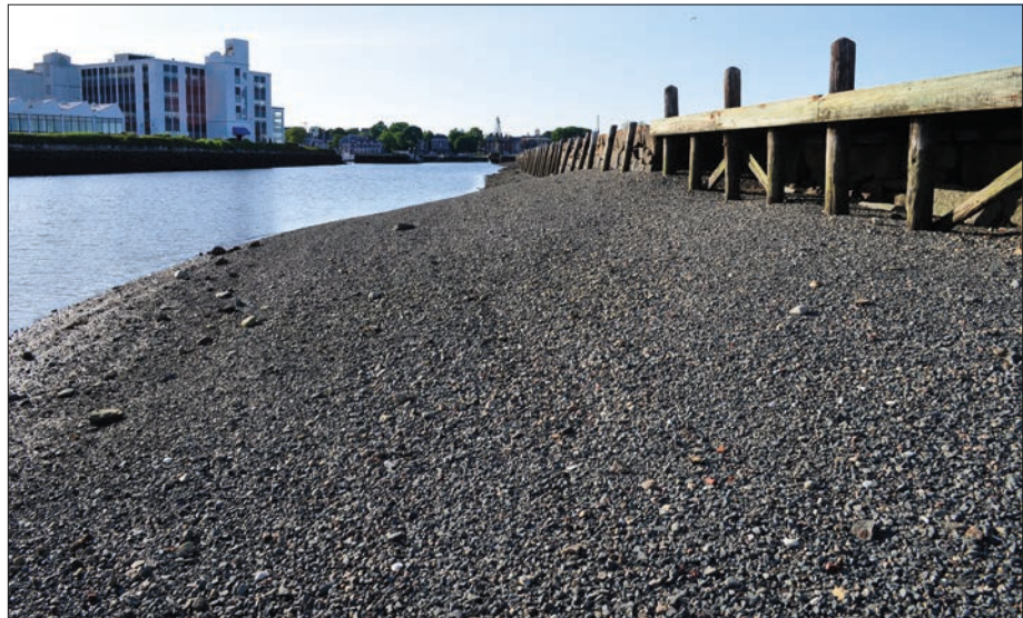
Figure A.17. View looking north on the west side of Derby Wharf about 1,800 feet from Derby Street. Gravel washes from the access road during storms and collects below the wharf, June 3, 2015 (OCLP).
