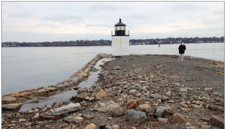
Figure A.24. View of Derby Wharf Lighthouse during high tide, February 2013 (OCLP).
