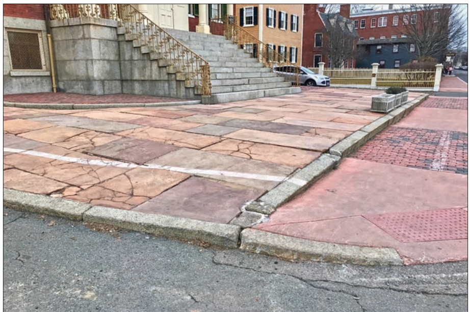
Figure 146. Improve accessibility of the Custom House terrace by resetting the flagstones in the southwest corner of the terrace, bringing the grade down to the level of the sidewalk and creating an accessible ramp (OCLP).
