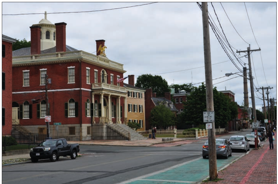
Figure 92. View looking east along Derby Street of the Custom House and other historic buildings along Derby Street, June 2015 (OCLP).
