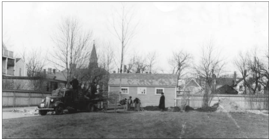
Figure 53. View looking north of a crew planting the area around the Comfort Station behind the Hawkes House, 1941 (National Park Service Collections, SAMA 08B-004).
