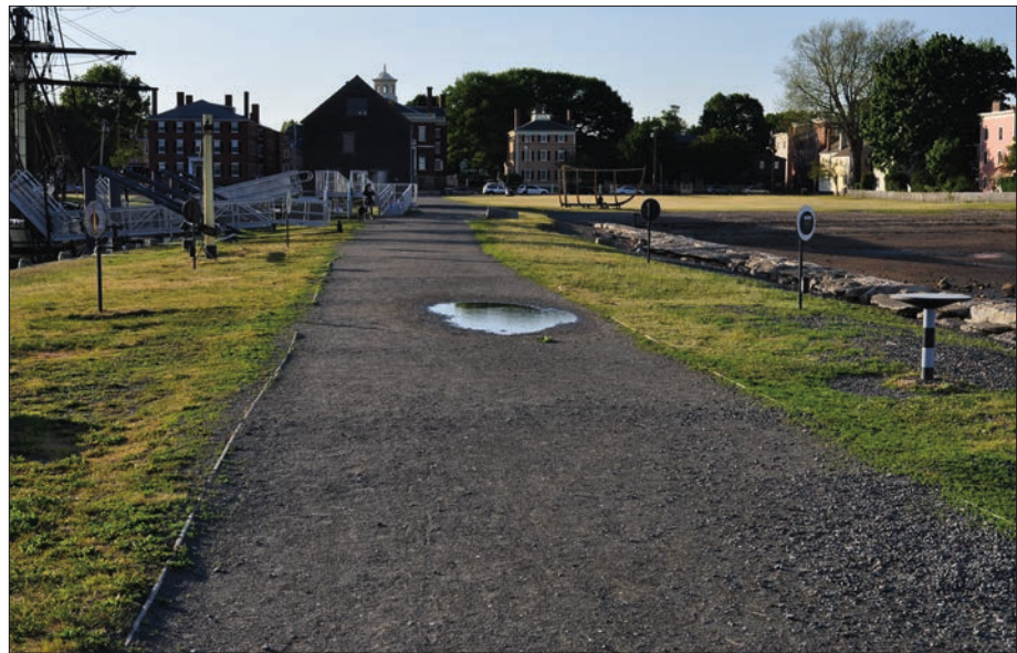
Figure A.15. View looking north on Derby Wharf about 600 feet from Derby Street. Wooden edging aids in holding the gravel surface material, but the material is still washed away during heavy storm surges as illustrated in the next two figures, June 3, 2015 (OCLP).
