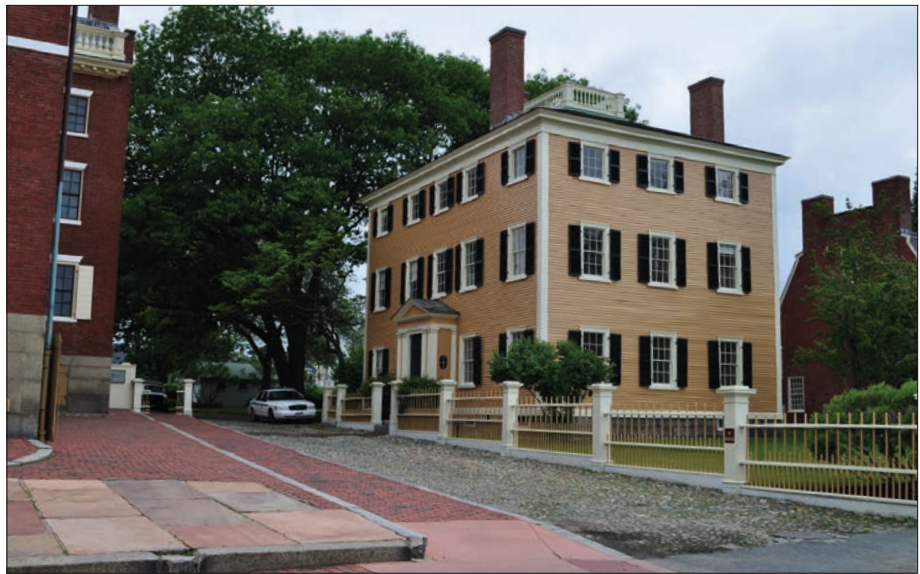
Figure 160. Existing condition of front of Hawkes house with elm tree removed and most of the shrub plantings extant. The red oak behind the Hawkes House with heavy limb over the Custom House Court, June 2015 (OCLP).
