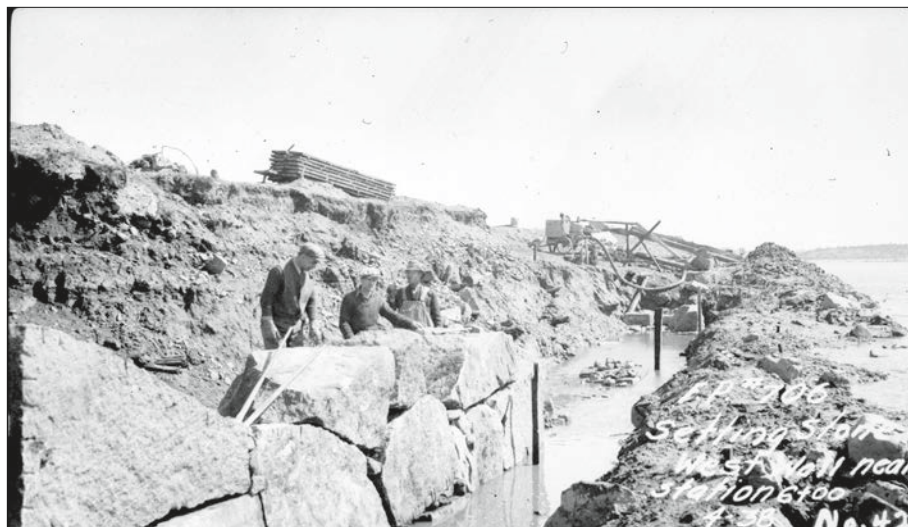
Figure 43. A crew repairs stonework on the west wall of Derby Wharf, April 1938 (National Park Service Collections, SAMA 14B-25).
