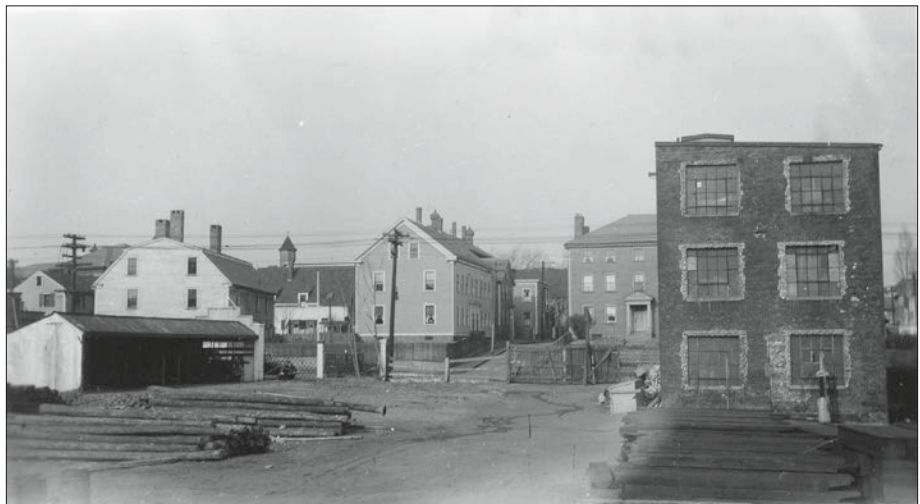
Figure 52. View north of preserved 1825 brick warehouse at the head of Central Wharf (Forrester's Warehouse), January 1939 (National Park Service Collections, SAMA 16B-001).
