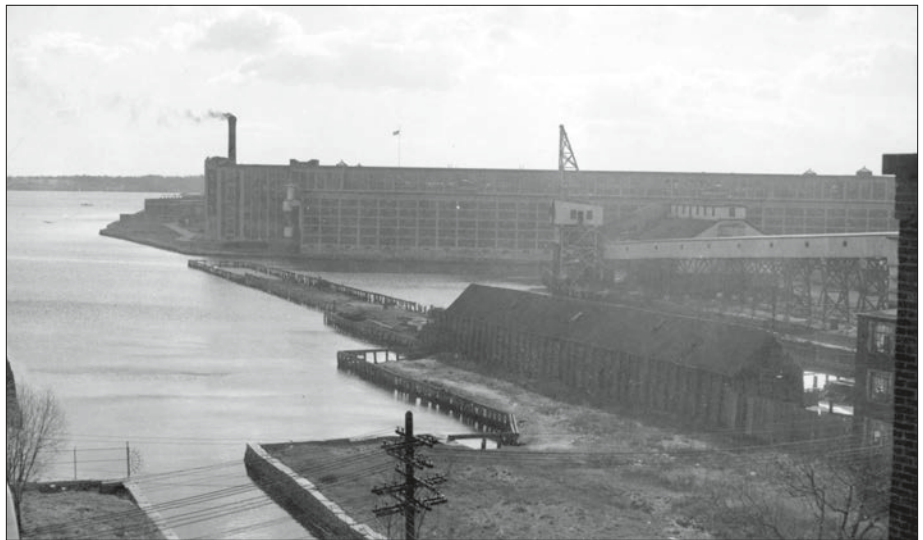
Figure 107. Central Wharf north end, July 18, 1977 (Salem Maritime National Historic Site 15B-140).
