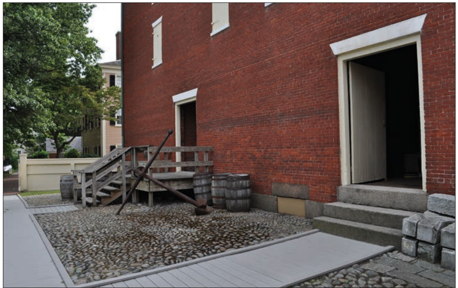
Figure 149. Existing conditions of inaccessible circulation behind the Public Stores, looking east, August 2013 (OCLP).
