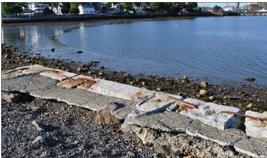
Figure A.05. Photograph of steel rods that act as staples to hold together the top course of the granite seawall, also referred to as “hairpins,” June 2015 (OCLP).
