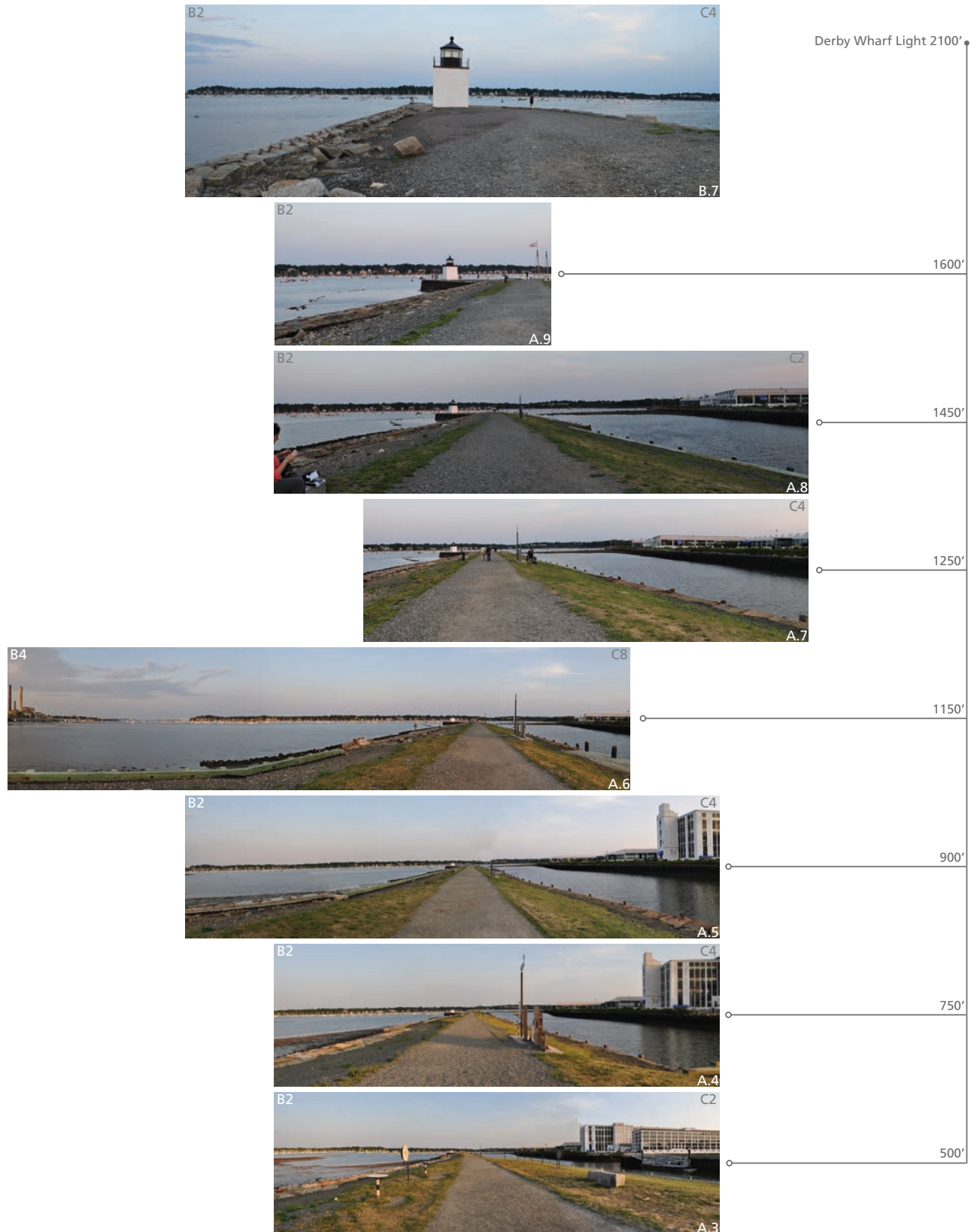
Figure A.10. Photographic sections illustrate the slight variations in construction methods along Derby Wharf. Markers along the right edge of the diagram correspond with interval markers in Figure 110 (OCLP).
