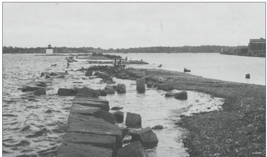
Figure A.29. View looking south toward the Derby Wharf Lighthouse showing deterioration of Derby Wharf due to lack of maintenance, April 1937 (Allan Rinehart, National Park Service Collections, SAMA 14B-003).
