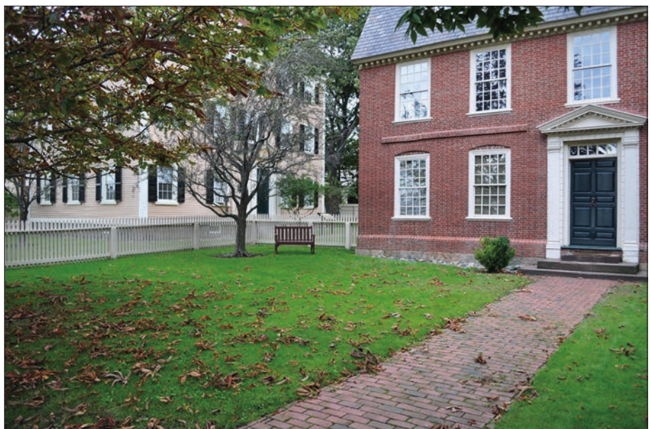
Figure 100. View looking northwest of the Derby House, showing the English hawthorn at the corner of the front lawn and boxwood at either side of the front door, October 2012 (OCLP).
