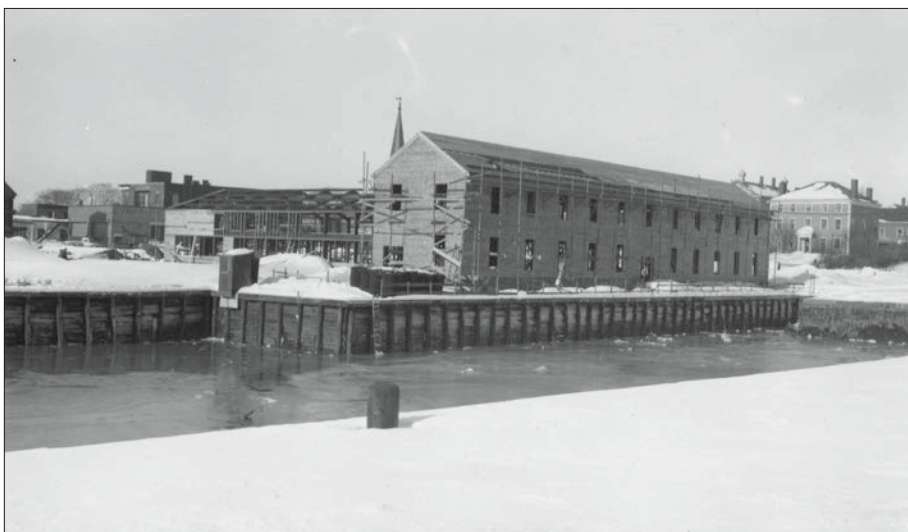
Figure 56. View from Derby Wharf looking northwest at Naval Reserve Training Center on Central Wharf under construction, January 1948 (National Park Service Collections, SAMA 17B-006)
