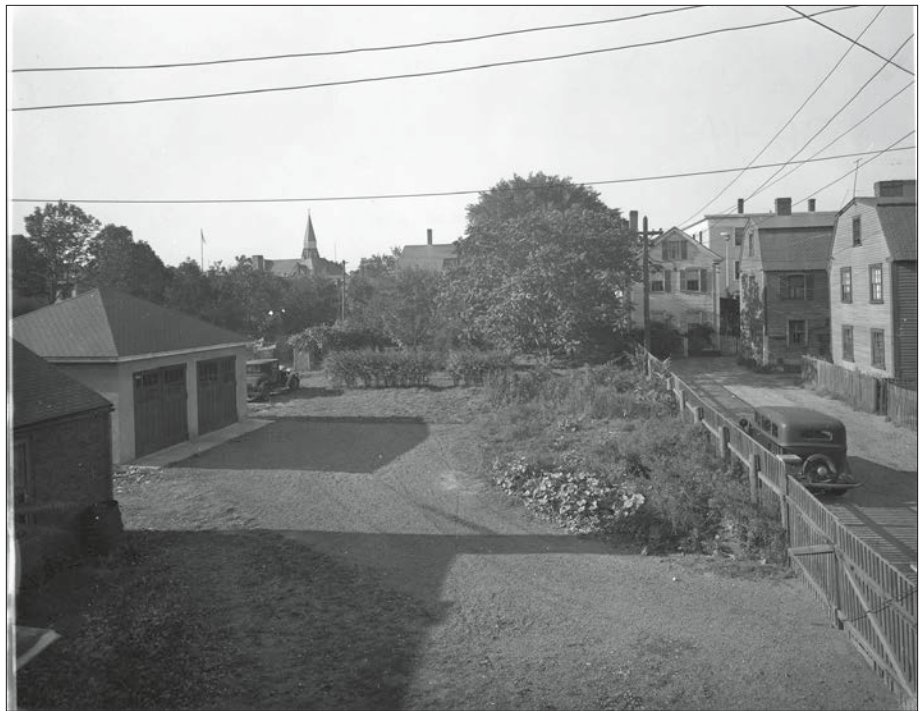
Figure 40. The Derby House back yard with the kitchen ell (far left), two-car garage, and Palfrey Court, September 7, 1937. Vegetation in the yard includes a black walnut, fruit trees, a privet hedge, and garden beds. A wooden fence is visible along the east property line (National Park Service Collections, SAMA 03A-014).
