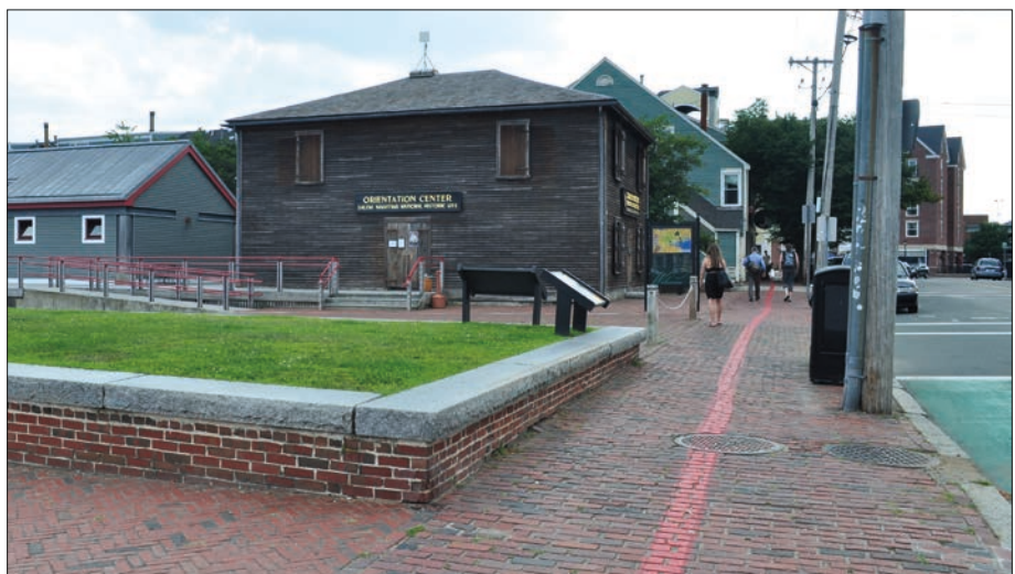
Figure 175. Existing condition of the Forrester's Warehouse foundation, looking east on Derby Street (OCLP).
