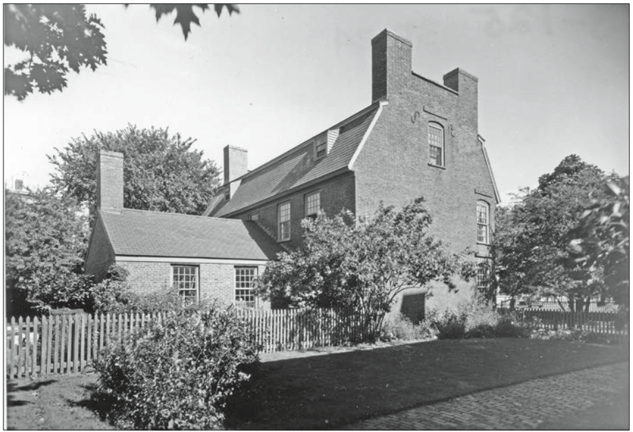
Figure 165. Historic photograph of shrubs near Derby House, August 1958 (Salem Maritime National Historic Site 3B-024).
