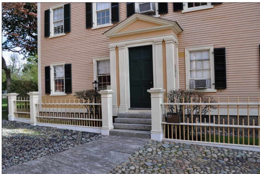
Figure 147. Photosimulation illustrating the rehabilitated Custom House Court, demonstrating the correct rise on the bottom step and granite slab crosswalk (OCLP).
