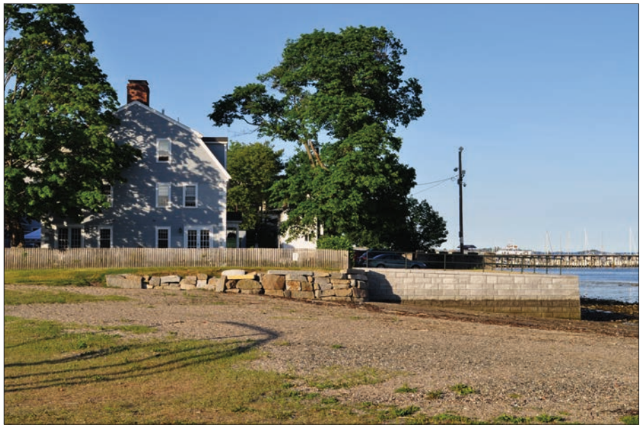
Figure 112. View of a portion of the rehabilitated Tucker's Wharf looking east from Derby Wharf, June 2015 (OCLP).
