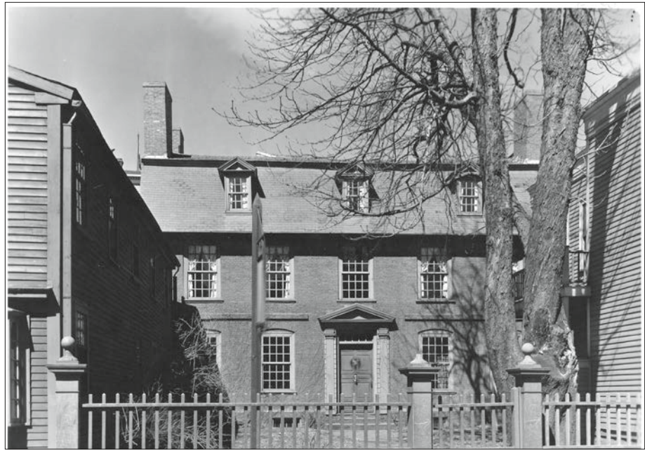
Figure 32. The Derby House and West India Goods Store at left and stores at 166 Derby Street at right just before demolition, 1936. The West India Goods Store was subsequently moved back to its original location on the right. Note the large horse-chestnut tree in front of the Derby House (National Park Service Collections, SAMA 03A-008).
