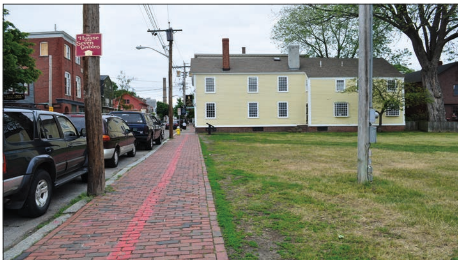
Figure 168. View looking east showing the current conditions along the south side of Derby Street, June 2015 (OCLP).
