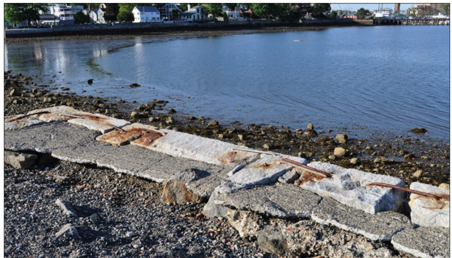
Figure 184. Photograph of steel rods that act as staples to hold together the top course of the granite seawall, also referred to as "hairpins," June 2015 (OCLP).
