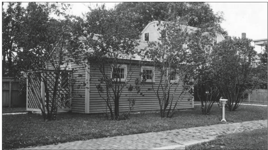
Figure 97. The Comfort Station with screening shrubs and a water fountain in the foreground along the brick walkway, July 1942 (National Park Service Collections, SAMA 08B-005).
