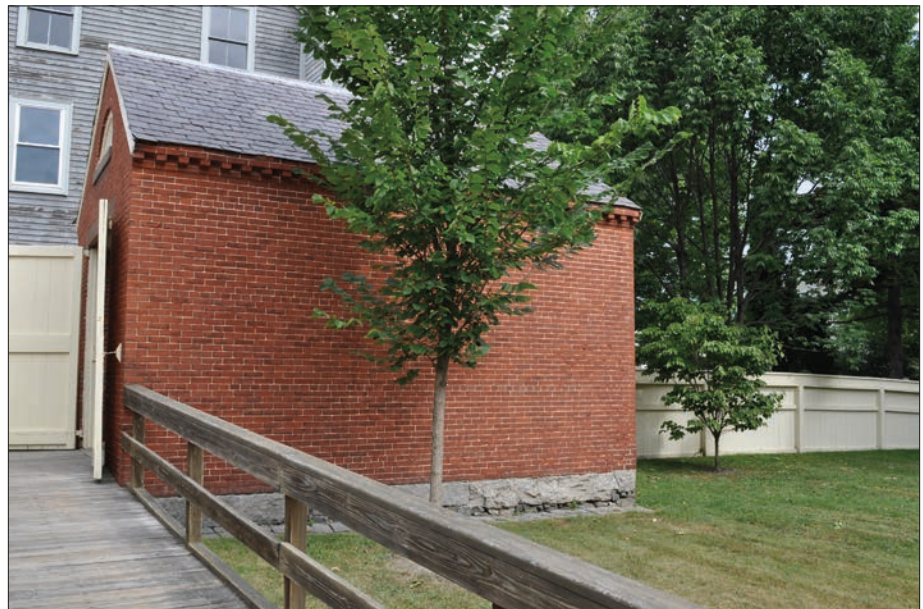
Figure 94. View looking north of the Scale House with a young American elm nearby and a young dogwood to the right, August 2013 (OCLP).
