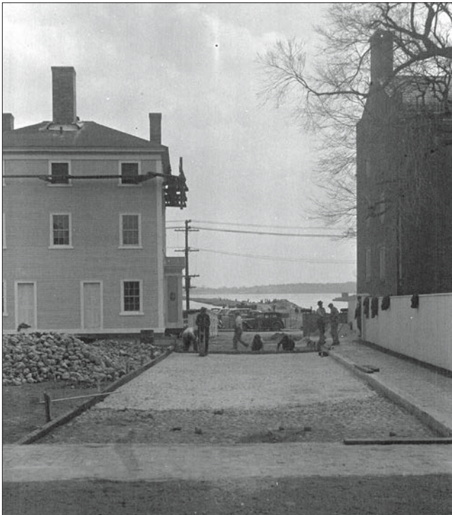
Figure 82. (Right) View south along the length of Custom House Court. The Hawkes House and Public Stores facility are visible as well as a portion of the Custom House-Public Stores brick walk and wooden fence. Pedrick store house and the waterfront are visible in the background, October 2012 (OCLP).
