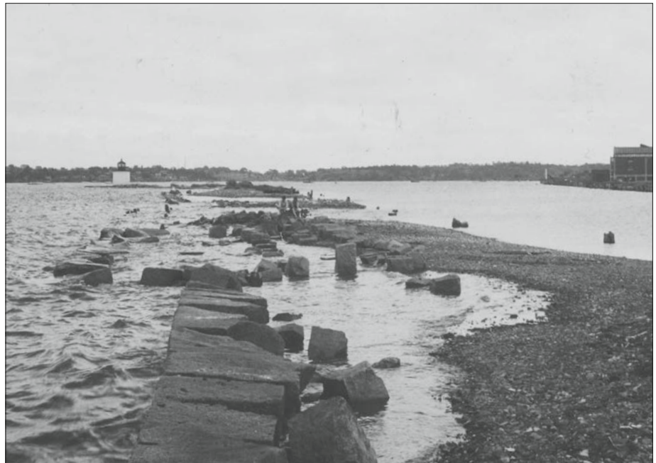
Figure 183. View looking south toward the Derby Wharf Lighthouse showing deterioration of Derby Wharf due to lack of maintenance, April 1937 (Salem Maritime National Historic Site 14B-003, USDOI Allan Rinehart).
