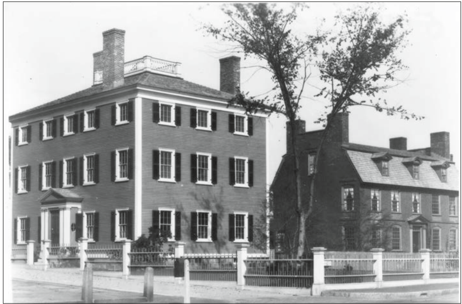
Figure 50. View looking northeast of Hawkes and Derby houses, May 20, 1940. A recently planted elm and a collection of native shrubs grow in the Hawkes House yard. Ornamental fences surround the homes. Bollards that front the Custom House are visible in the foreground. Custom House Court is surfaced with cobbles (National Park Service Collections, SAMA 05B-006. Photograph by Stanley P. Mixon).
