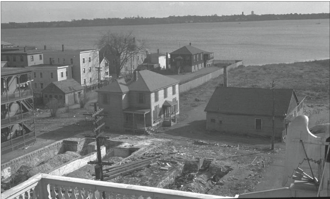
Figure 39. View looking southeast from the Custom House cupola in 1937. Buildings remaining in the foreground include a dwelling and the bakeshop. Buildings beyond the fence in the Derby Beach area include the Polish Socialist Alliance Club, the Polish American Veterans Association building, and a shed. The bakeshop remains in the foreground. Derby Wharf Lighthouse is visible in the distance at right (National Park Service Collections, SAMA 14A-103).
