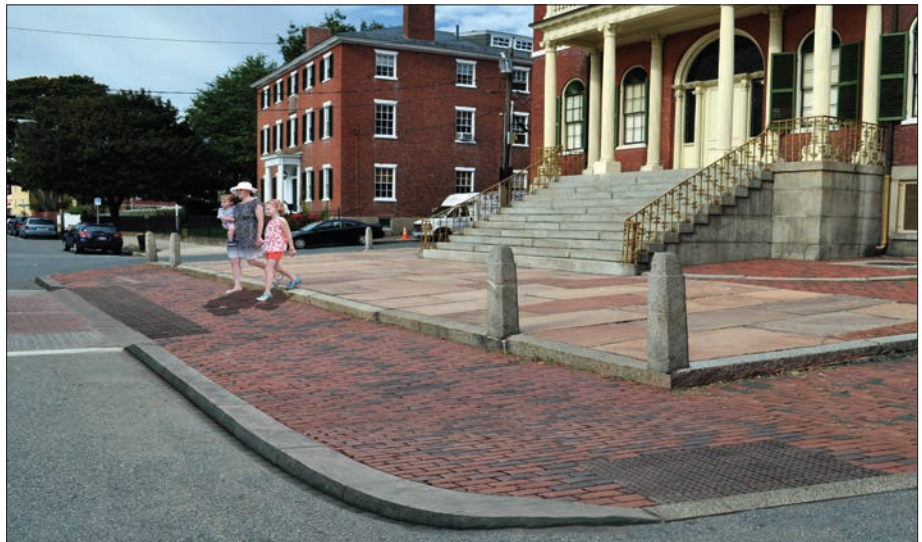
Figure 145. Improve visitor safety by rebuilding the sidewalk with seven inch step from the Custom House terrace to the Derby Street sidewalk as illustrated in the photo simulation (OCLP).
