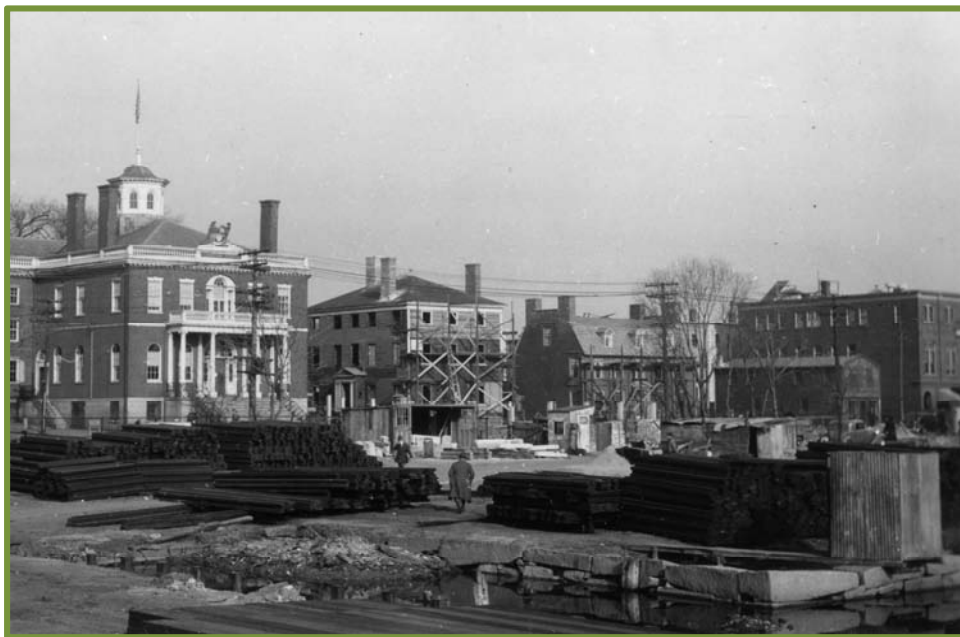
Figure 25. Overview of Derby Counting House location during 1938 wharf rehabilitation
