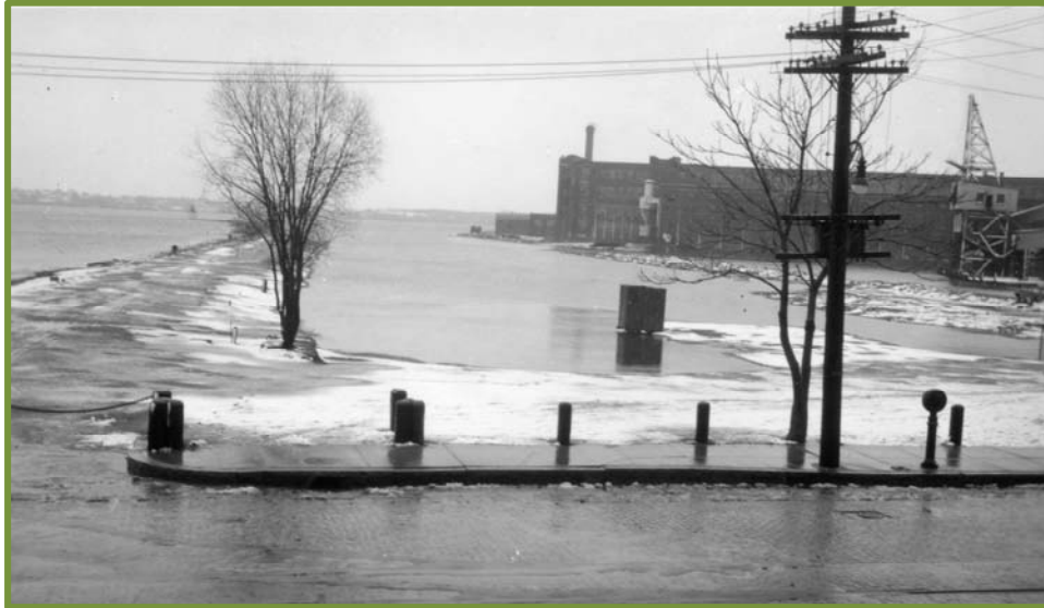
Figure 18. High tide event at Derby Wharf, showing inundation of Derby Counting House location, ca. 1940 Courtesy of SAMA
