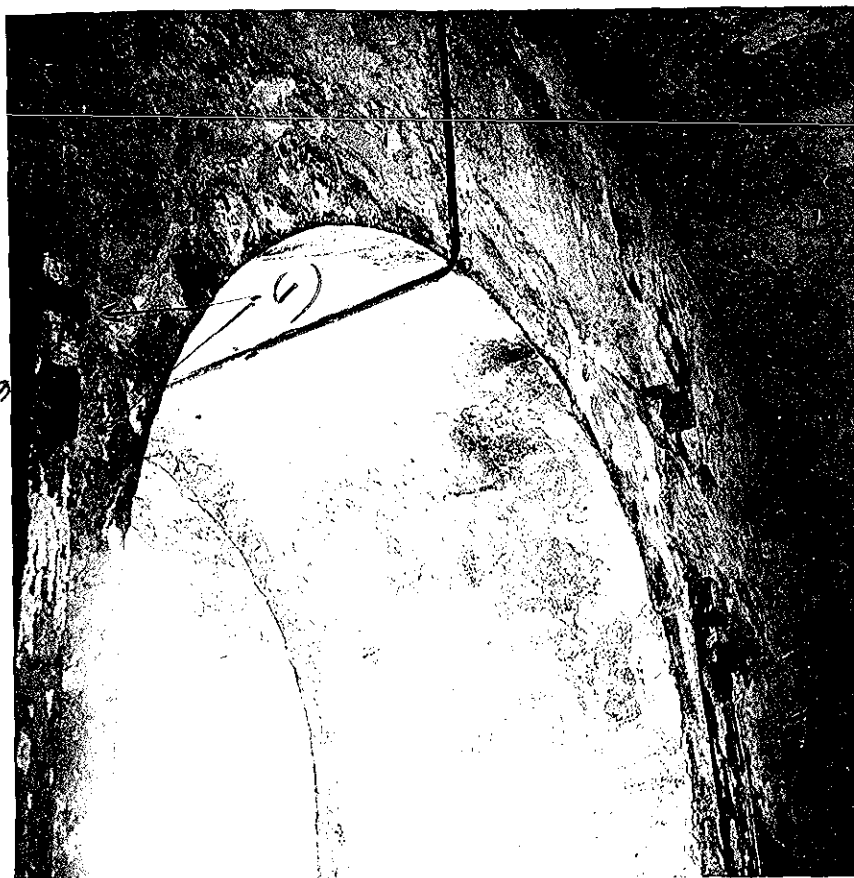
PHOTO 2. Inside of facade looking from vestibule towards fixed bridge. Notice ausubo timbers on both sides of archway. Number (1) in ink shows metal clasps which served as hinges, with screws and nuts on back side of timbers. Each timber has three hinges. The whole thing suggests a folding door.
