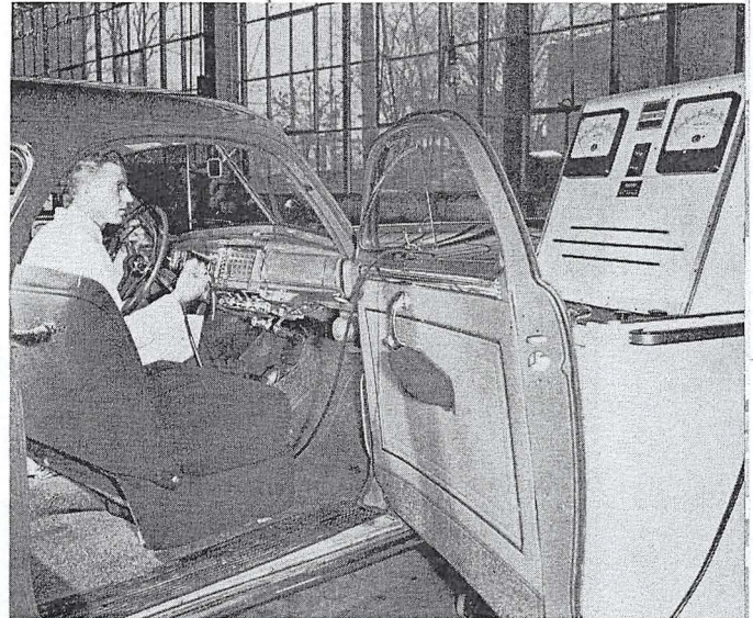
● The portable control consists of two buttons. Pressing on either button will instantly change the pace and load. Steep grades, slow and fast open-road driving and stop-and-go traffic results are all calibrated in rapid order.
