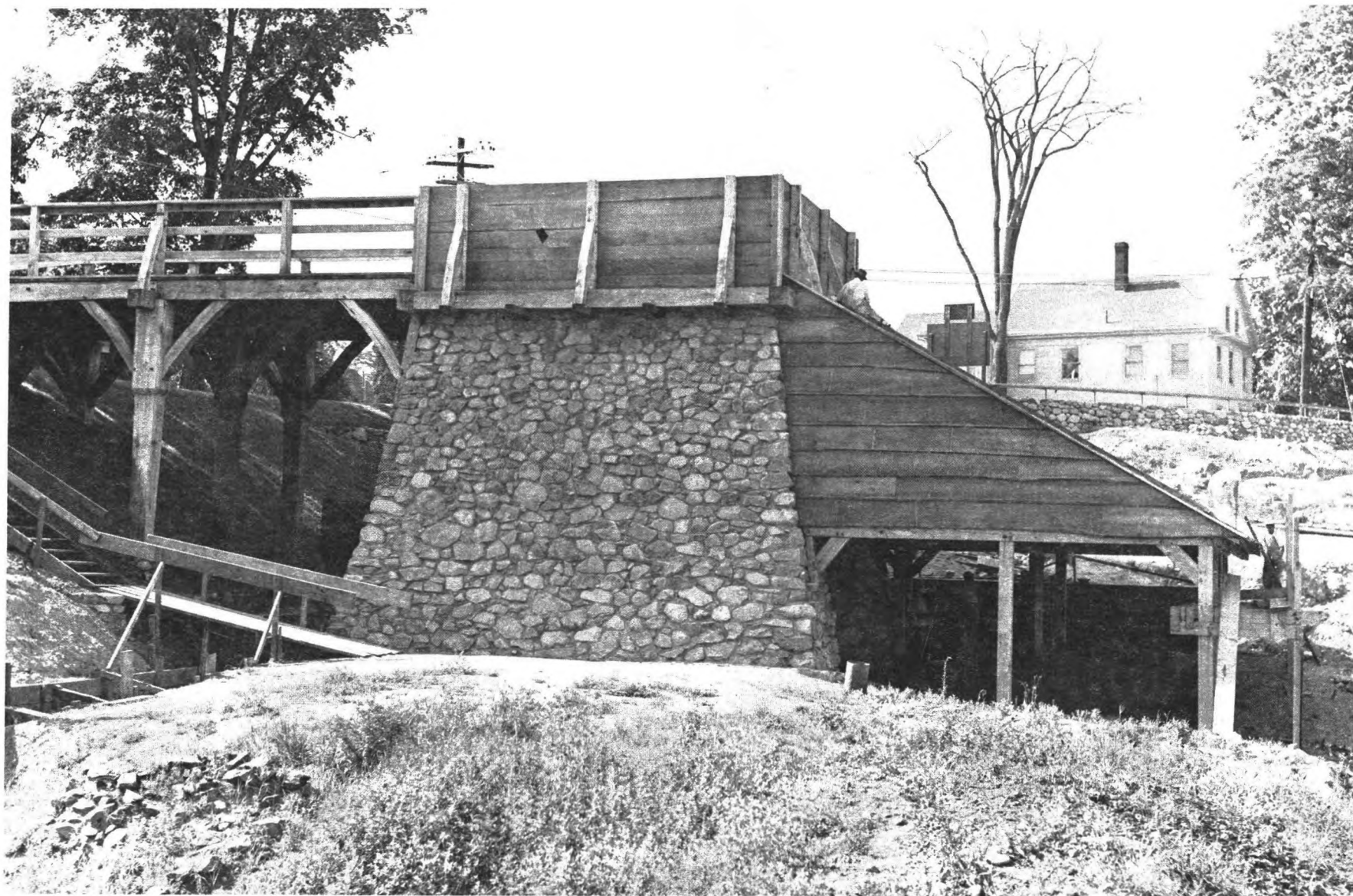
THE FURNACE- THE FIRST TO OPERATE IN MASSACHUSETTS
