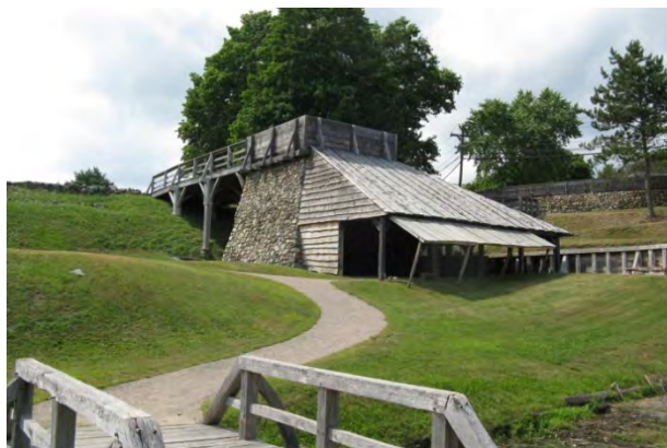
Figure 8. Furnace at Saugus. The ore, flux, and charcoal were dumped into the furnace over the charging bridge from above. The bellows operation is covered by the wooden roof. Note the paved trail in the foreground and the relatively steep slopes surrounding the operation. Photograph by John Phelan, available on Wikimedia Commons via Creative Commons Attribution 3.0 Unported license at http://commons.wikimedia.org/wiki/File:The_Furnace_at_Saugus_Iron_Works_MA.jpg (accessed 21 July 2014).
