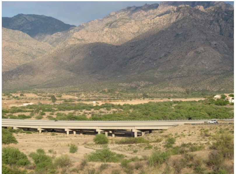
Photo 11. Looking downstream on Big Wash towards the Tangerine Road Bridge, with SR-77 and the Santa Catalina Mountains. Washes provide important corridors for certain species, and in situations like this allow them to pass under roads. Photo from Bier et al. 2006a.
