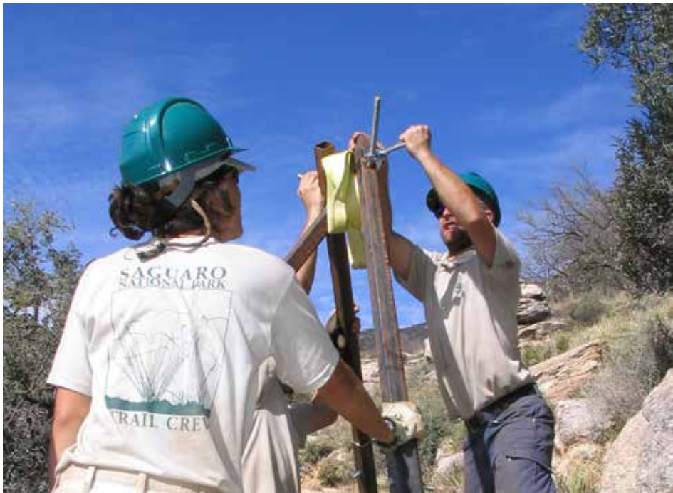
Trails in Saguaro National Park are maintained by our Trail Crew and projects are paid for using fee dollars. Here they are rigging equipment to move large rocks out of the trail.
