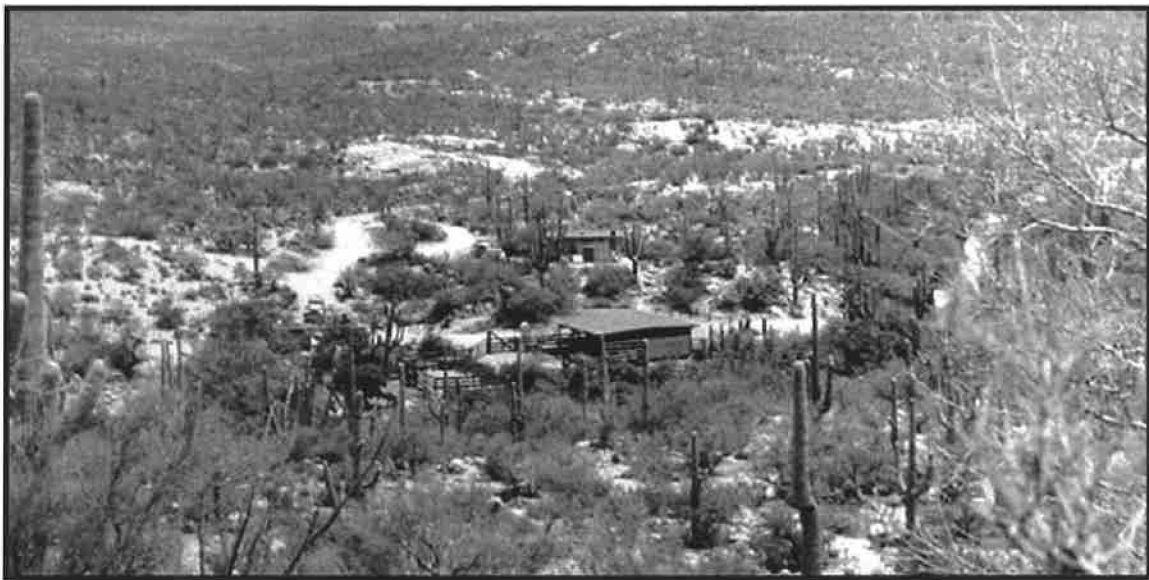
Madrona Pack Base mid to late 1940's. View looking east.
