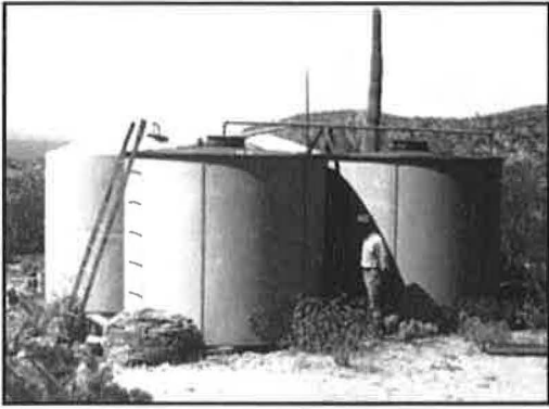
Figure 8. Four water storage tanks in the equipment staging area
