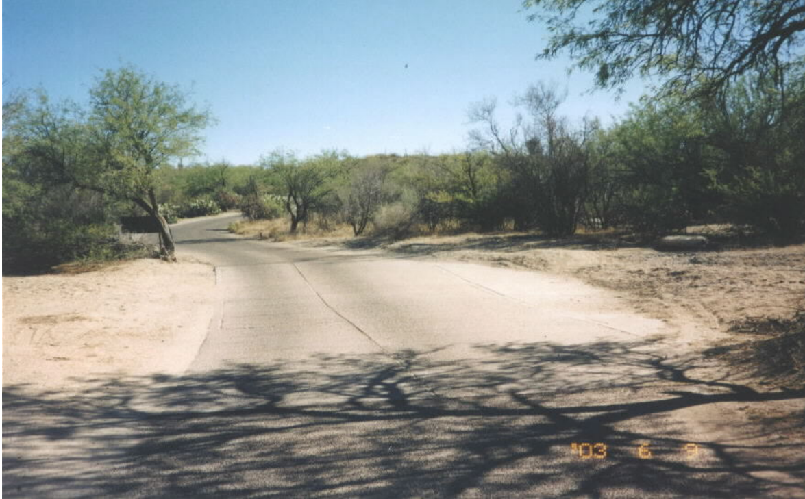
FIGURE 5. ASPHALT LOW-WATER CROSSING
