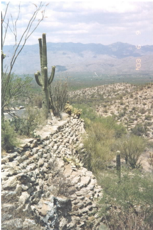
FIGURE 6. CIVILIAN CONSERVATION CORPS CONSTRUCTED WALL
