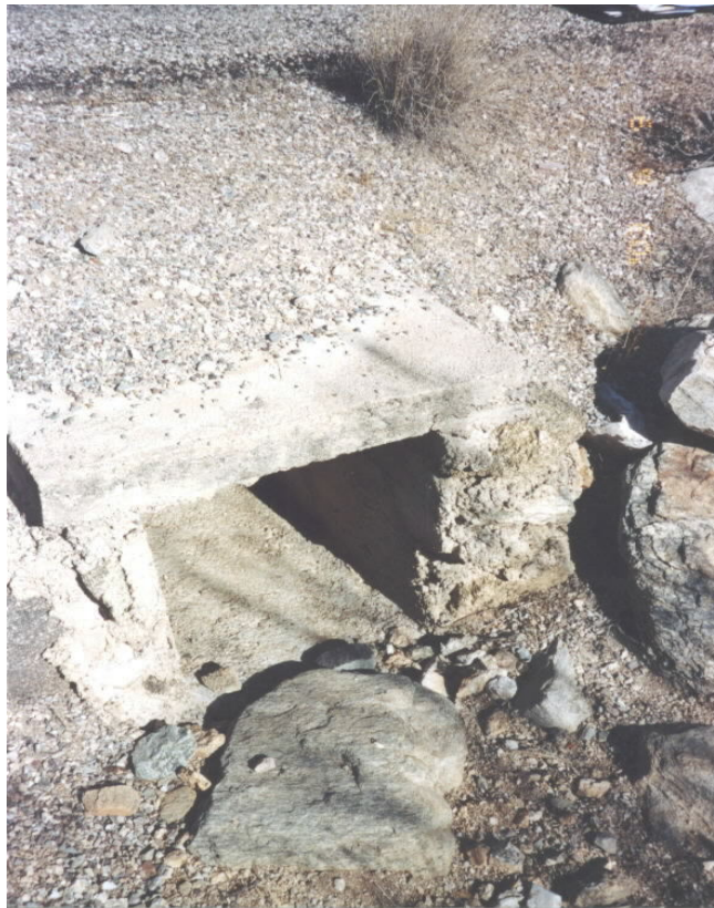
FIGURE 4. REPRESENTATIVE CONCRETE BOX CULVERT
