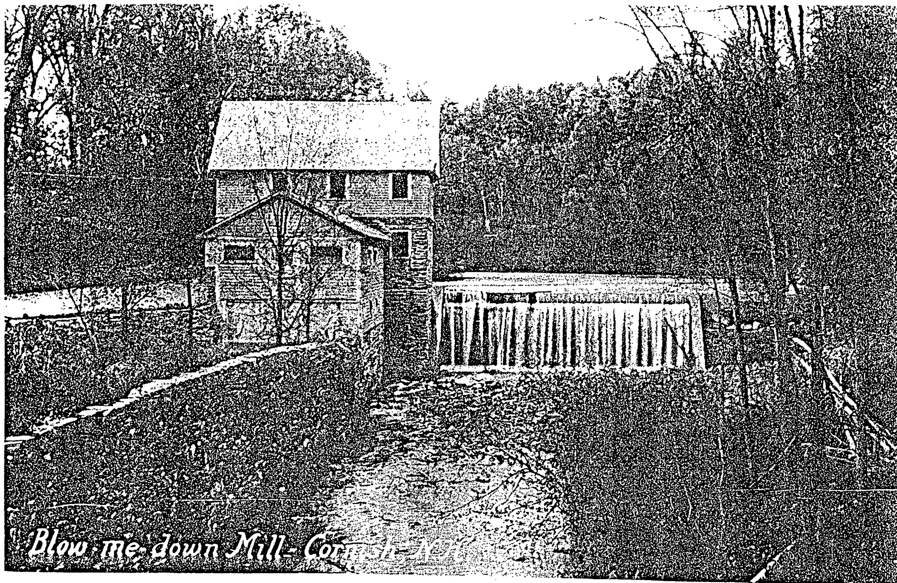
Fig. 8c. Summer low-flow conditions at Blow-Me-Down Dam, around the turn of the century.
