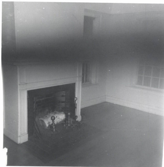
Northwest Room - Second Floor
