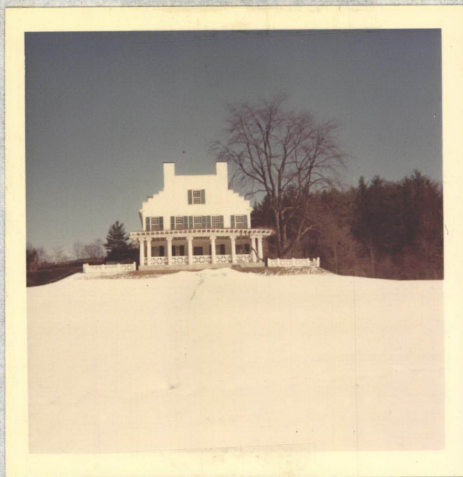
Aspet - View Eastward
