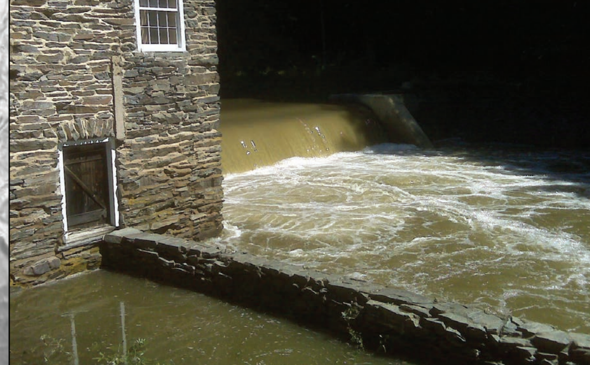
Flooded mill at Blow-Me-Down Brook in 2011. The mill complex is located on the Blow-Me-Down Brook floodplain. NPS photograph.
