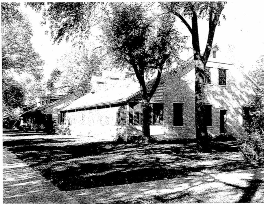
Photo by Mattison, October 1957 Old Officers Row at Fort Lyons No. 2, (Colorado (1867-1889) These buildings, date of construction unknown, are the only surviving buildings of the original fort. Southeast view.
