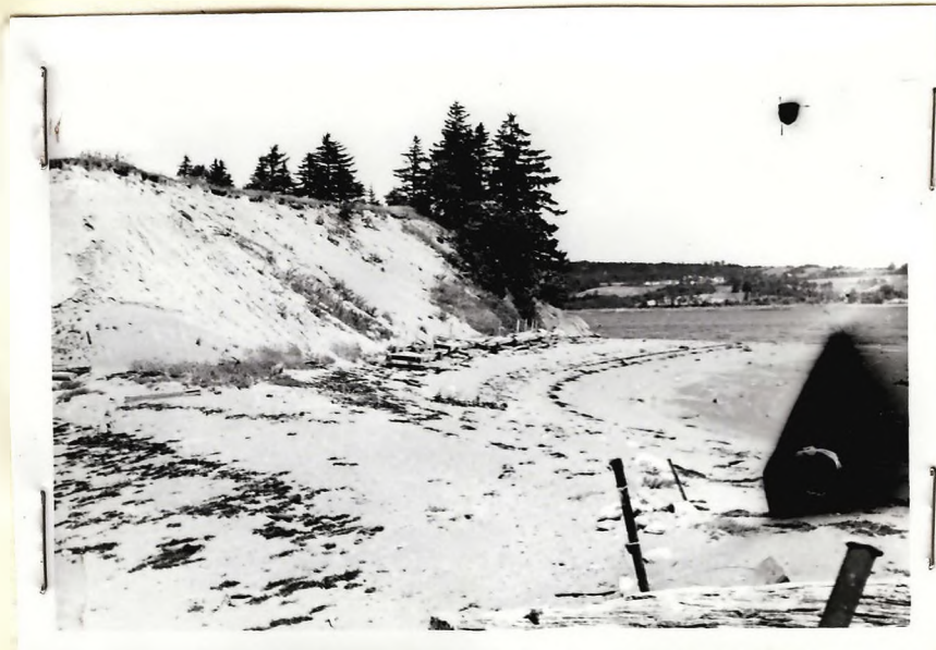
17. Looking across erosional cut at southern tip of island toward Canadian shore; almost low tide.
