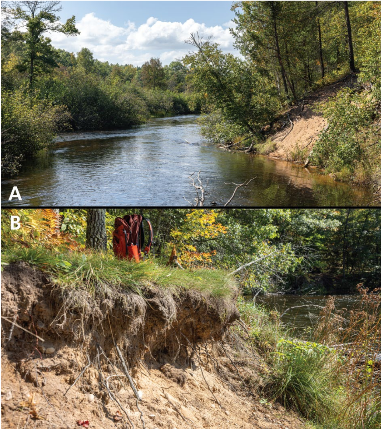
Figure 20. Erosion along the St. Croix and Namekagon rivers often leads to bank undercutting and collapse. A) A tree tilts toward the Namekagon River due to its foundation having slumped into the water. B) Undercutting along a bank of the Namekagon River. The roots of the grasses and plants above will hold together the upper layer as the layer under it eventually collapses into the river. Backpack for scale. Photographs by Matthew Harrington (Colorado State University).
