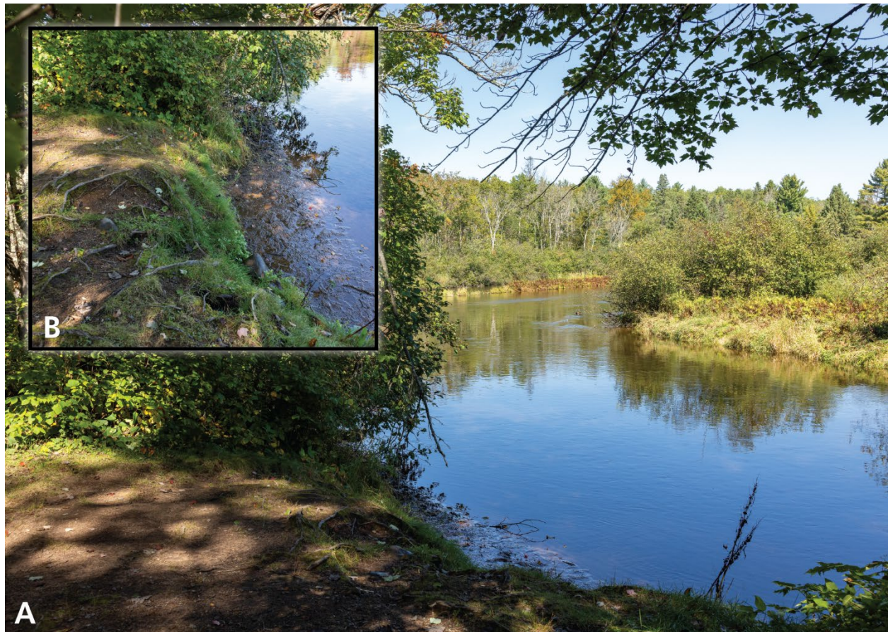
Figure 21. Erosion along river landings has the potential to create challenges for boaters, floaters, and other recreational users. A) Phipps Landing along the Namekagon River has eroded along its access point. The access point is steep and could present issues to floaters attempting to leave the river. B) A close-up of the access point, where roots are holding together what hasn't been eroded away. Photographs by Matthew Harrington (Colorado State University).
