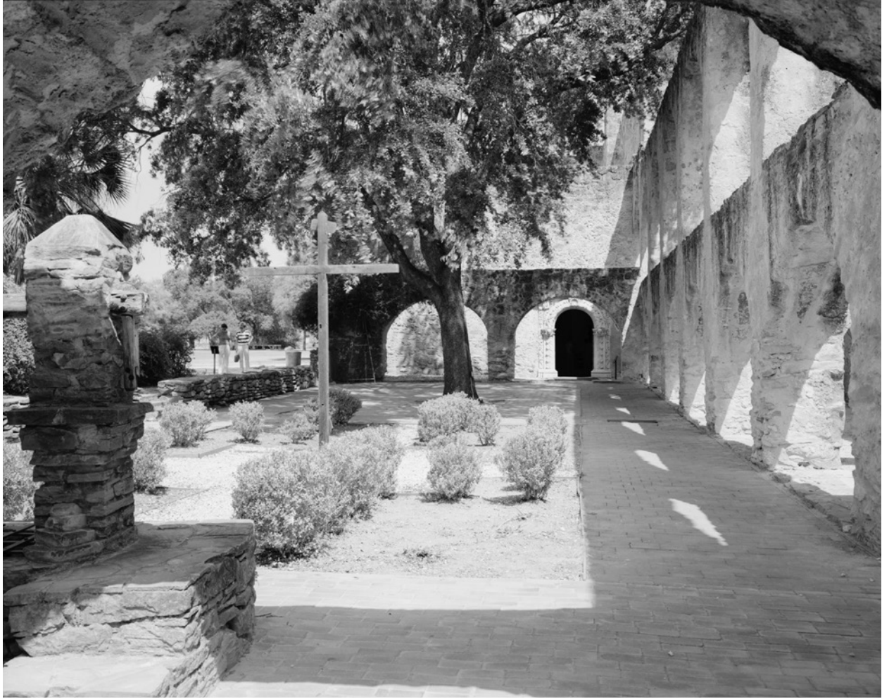
Figure 4.2: This ca. 1983 photograph by John Lowe illustrates the 1948 reconstruction of the portería's lower level (Historic American Buildings Survey [HABS], Library of Congress).
