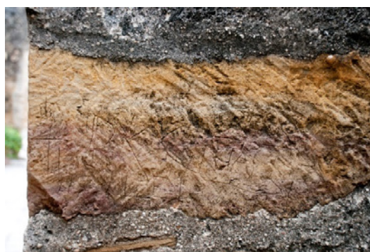
Figure 6.B.98: Room HS 203 B—South wall. Detail of a sandstone in the jamb of door D06, which exhibits marks from a chisel and graffiti.
