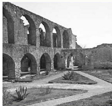
Figure 4.64: West view of the courtyard. The level of the courtyard has been lowered. Unattributed photograph, 1935 (ITC UTSA).
