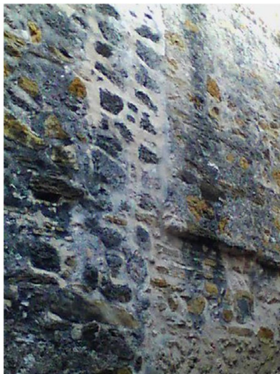
Figures 6.B.31 and 6.B.32: Room HS 203 F—West wall. Same portion of wall is shown in both photos. Left photo shows temperature differences in the wall, indicating different materials exhibit different temperatures. Areas with sandstones tend to be warmer, and 20 th -century additions with cement-based mortars tend to be cooler.
