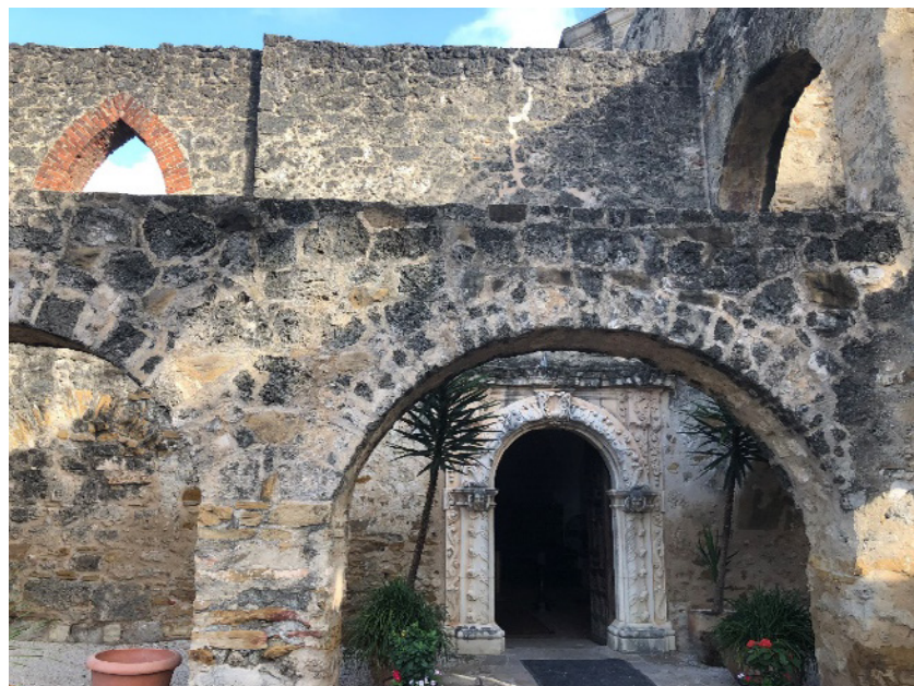
Figure 6.B.234: Exterior walls—Cloister west wall. Detail of the right arch. Masonry changes between the bottom of the pillar and the arch due to the collapse in 1940s and its later reconstruction.
