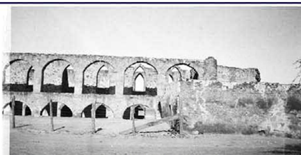
Figure 4.54: Southwest view, clearly demonstrating that the window in the south wall of the east part is closed. E.S. Quillin photograph, 1917 (ITC UTSA).
