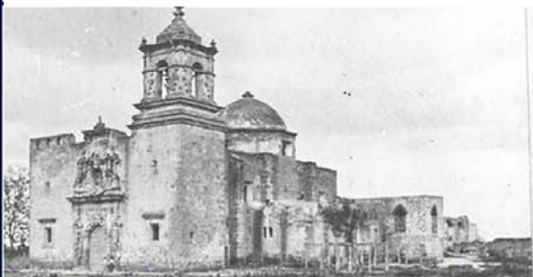
Figure 4.37: West view, showing the upper level of the porteria. In this ca. 1868 photograph, the flying buttress in the south end of the south arcade has become part of a wall (SACS, Raba Collection).
