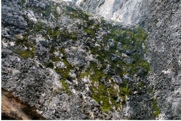
Figure 6.B.101: Room HS 203 B—Transverse arch. Detail featuring moss in its southern end.
