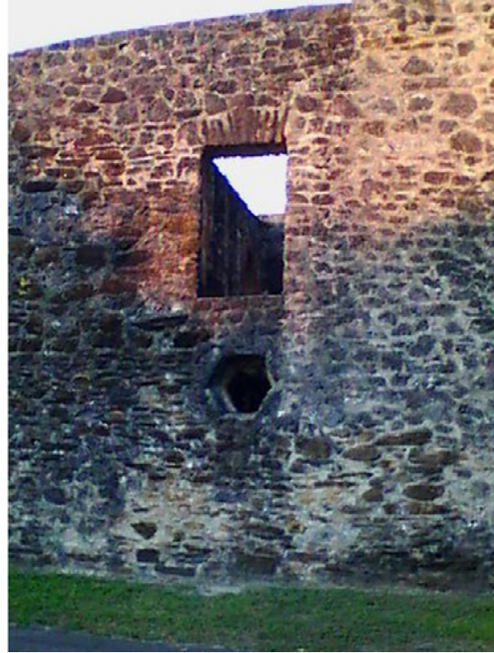
Figures 6.B.192 and 6.B.193: Exterior walls—North wall. Same view of the western end of the wall. The differences in temperature are caused by the different construction materials corresponding to different construction and reconstruction campaigns. The pink circle shape in the bottom left part of the photo features an infill.
