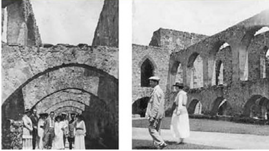
Figure 4.55: View from the south arcade facing west (left image). South view of the courtyard (right image). Unattributed photographs, 1920 (NPS Archive).
