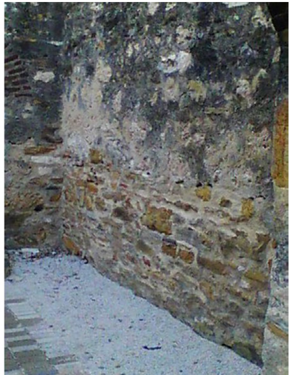
Figures 6.B.94 and 6.B.95: Room HS 203 B—East wall. Both images show the bottom area of the wall. Left photo shows temperature differences in the wall. The colder area of the wall corresponds to the area with a higher level of vegetation growth. The photo on the right also features several delaminated sandstones in the bottom part of the wall and numerous holes.
