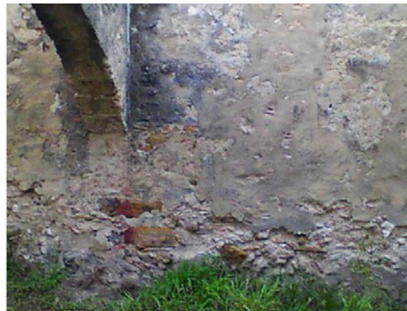
Figures 6.B.55 and 6.B.56: Room HS 203 D—North wall. Same portion of wall—a detail of the right area—is shown in both photos. Left photo shows temperature differences in the wall. The light blue part corresponds to the eroded area of the wall due to rising damp and to the area near the transverse arch where there is an accumulation of vegetation growth. The darker blue area surrounded by light blue could be caused by the detachment of the arriccio (plaster scratch coat) at that point.
