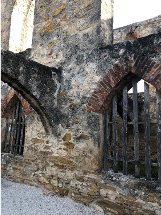
Figure 6.B.112: Room HS 203 E—North wall. Note biological growth and filled crack on the transverse arch. Erosion of the lower wall section.
