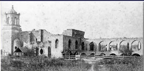
Figure 4.44: South view, E.K. Sturdevant photograph, ca. 1885 (SMU Library).
