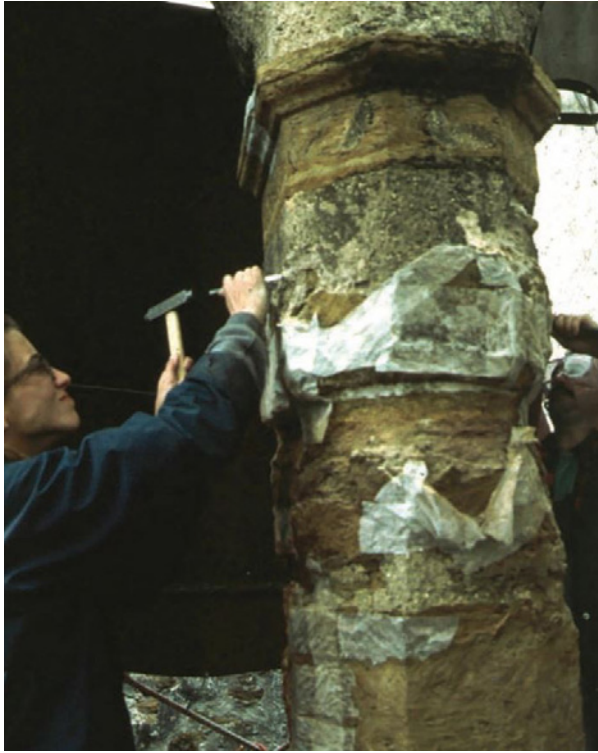
Figure 6.A.7: Application of facings to protect fragile areas during removal of lime and gypsum patches.
