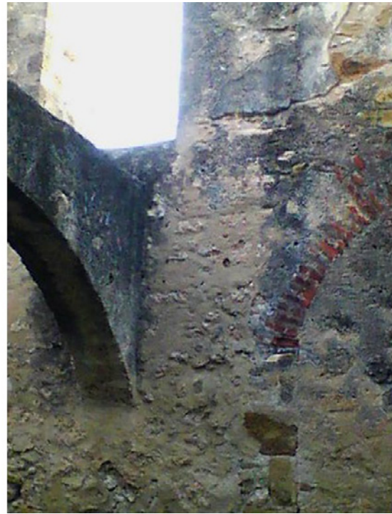
Figure 6.B.72 and 6.B.73: Room HS 203 C—North wall. Both images show the same view of the north wall area to the right of the transverse arch. Left photo shows temperature differences in the wall. Temperature changes in the bottom part appear to be due to rising damp, and those in the right part due to the presence of the former door opening D02, now closed in with masonry infill.
