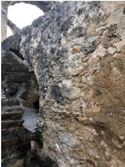
Figures 6.B.225 and 6.B.226: Exterior walls—West wall. Area corresponding to room 203 H. Exhibits vegetation growth in the arch and a high level of erosion.
