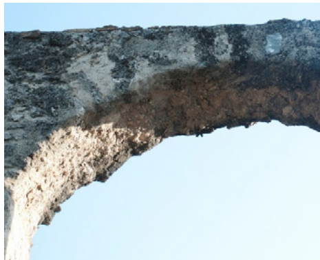
Figures 6.B.146 and 6.B.147: Room HS 203 H—North wall upper-level arch, which features fragmentation and delamination of stones in its right side.
