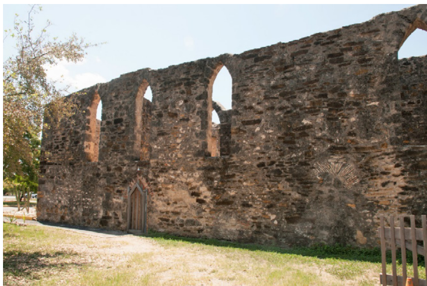
Figure 6.B.191: Exterior walls—North wall. General view of the left (east) part of the wall.
