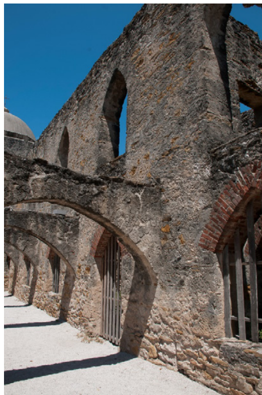
Figure 6.B.109: Room HS 203 E—North wall. General view.
