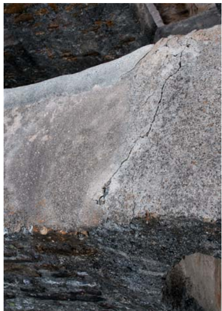
Figures 6.B.251–6.B.253: Wall between 203 D and 203 C—Views of the wall connection, exhibiting a diagonal fracture.
