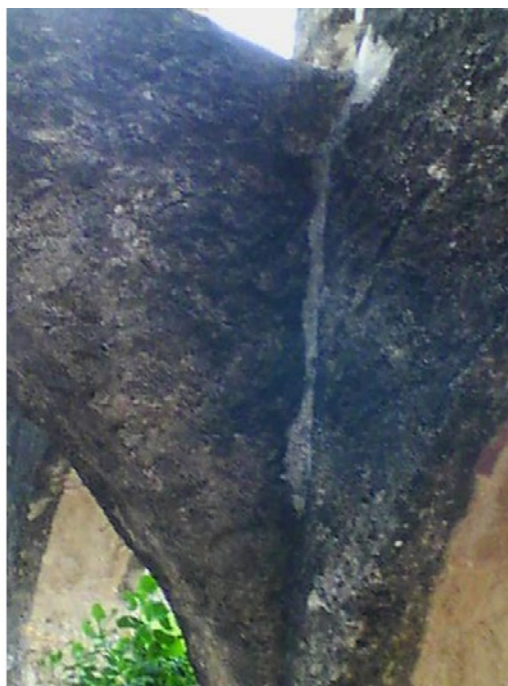
Figures 6.B.127 and 6.B.128: Room HS 203 E—South wall, transverse arch detail. Both images show the same view of the bottom area of the wall. Left photo shows temperature differences in the wall. The cement-based mortar used for filling the crack in the connection of the transverse with the south wall appears hotter than the materials used elsewhere in the wall.
