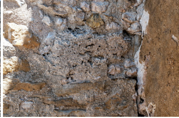
Figure 6.B.165: Room HS 203 K—North wall. Detail of the lower right corner of the wall. Features a crack in the connection of north and east walls and numerous holes.
