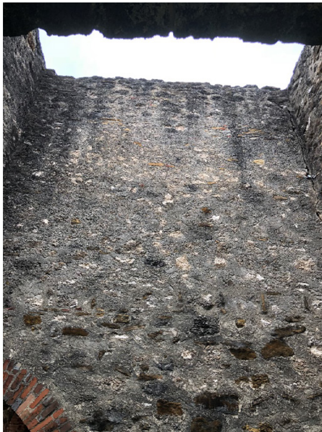
Figure 6.B.64: Room HS 203 D—South wall. Detail of the right bottom lancet arch features vegetation growth, efflorescence, and fragmentation of the brick in the intrados of the arch.
