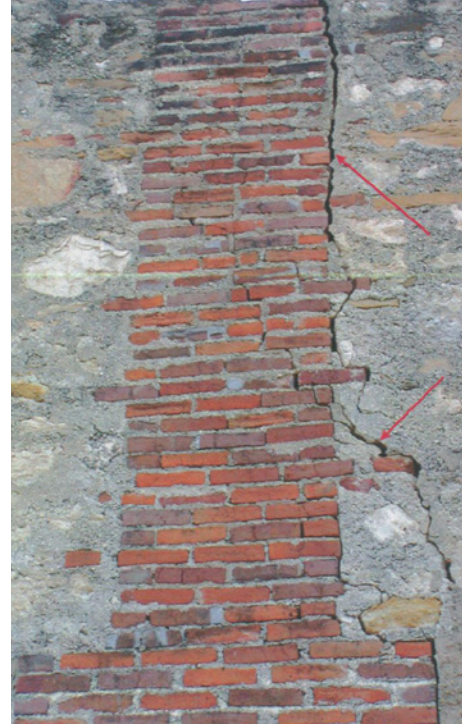
Figure 6.A.15: Kitchen—Eastern Wall in 2002. Crack in the upper section of the opening toward the refectory. Reprinted from Mission San José y San Miguel de Aguayo—Inventory & Condition Assessment Survey and Documentation Report of Spanish Colonial Plasters and Mortars , by Restoration Associates Limited, LLC, 2002, p. 102.
