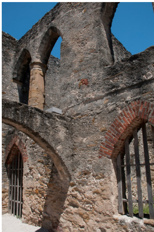
Figure 6.B.108: Room HS 203 E—North wall. Left part general view.
