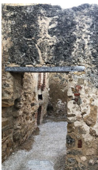
Figures 6.B.149, 6.B.150, and 6.B.151: Room HS 203 H—East wall. General view. Features vegetation growth in the upper part of the wall and erosion in the lower part.
