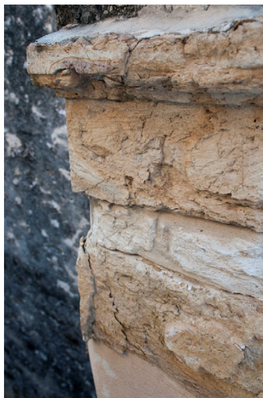
Figure 6.B.111: Room HS 203 E—North wall. Octagonal column, which features fragmentation of the sandstones.
