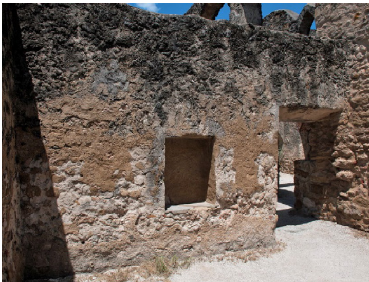
Figure 6.B.171: Room HS 203 K—West wall. General view.
