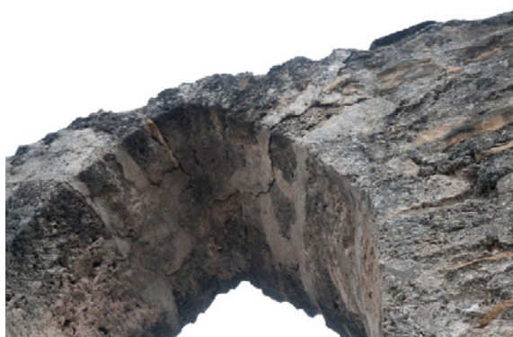
Figure 6.B.88: Room HS 203 B—North wall. Left upper window W11 showing a fracture near the keystone of the lancet arch.
