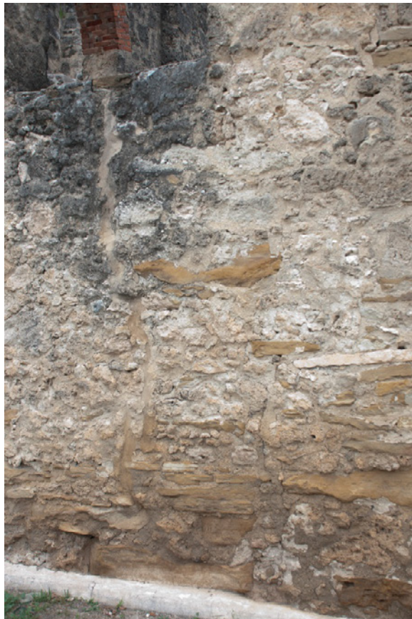
Figure 6.B.239: Exterior walls—South wall. Detail of the area below the window. Feature several cracks that have been filled and erosion of the masonry wall
