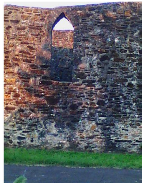
Figures 6.B. 194 and 6.B.195: Exterior walls—North wall. Area corresponding to the 203 D room. The differences in temperature are caused by the different construction materials and moisture content of the wall. It seems that in the bottom part of the wall below the window, there is an area that has been filled.
