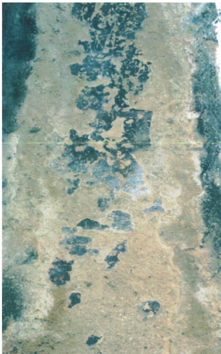
Figures 6.A.29, 6.A.30: Arch 1 D level 1 Detail of Spanish Colonial Plaster fragments.
