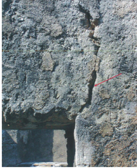
Figure 6.A.15: Kitchen—Eastern Wall in 2002. Crack in the upper section of the opening toward the refectory. Reprinted from Mission San José y San Miguel de Aguayo—Inventory & Condition Assessment Survey and Documentation Report of Spanish Colonial Plasters and Mortars , by Restoration Associates Limited, LLC, 2002, p. 102.
