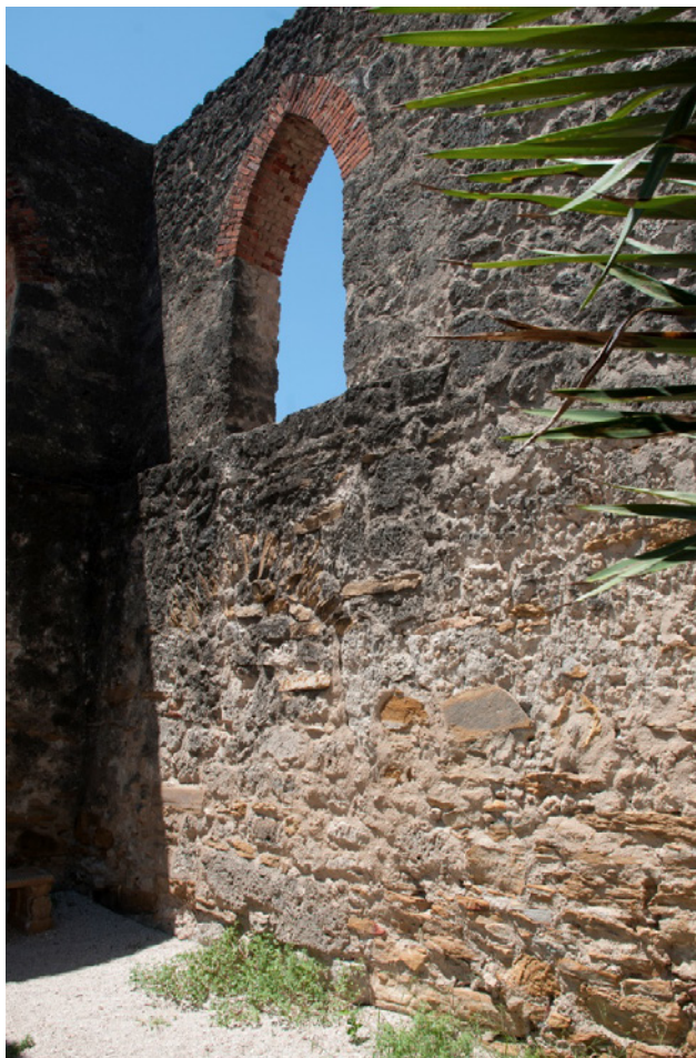
Figure 6.B.11: Room HS 203 S—West wall, south corner general view.
