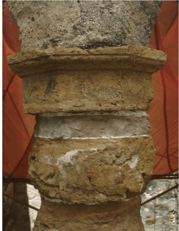
Figure 6.A.8: The column after the removal of patches.
