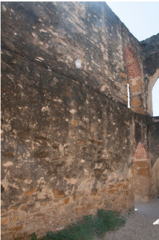
Figure 6.B.23: Room HS 203 F—East wall. General view of the wall.
