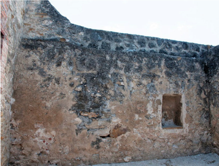
Figure 6.B.165: Room HS 203 K—North wall. Detail of the lower right corner of the wall. Features a crack in the connection of north and east walls and numerous holes.
