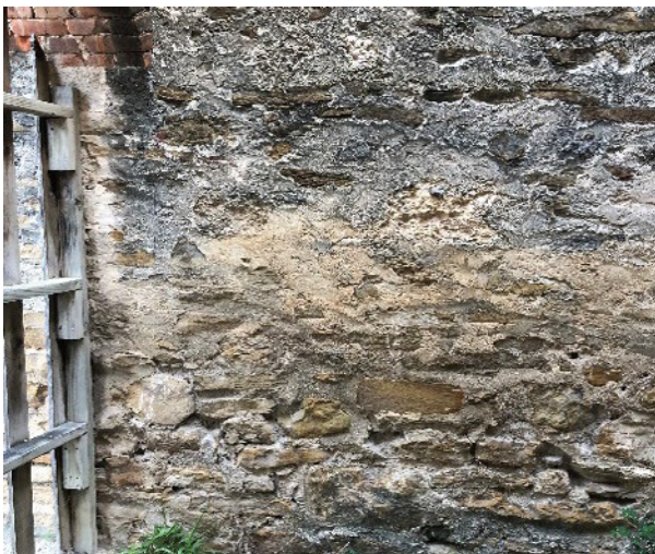
Figures 6.B.46 and 6.B.47: Room HS 203 A—West wall. Patching mortar at the base of the wall has been eroded.
