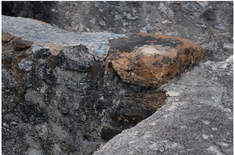
Figure 6.B.250: Wall between 203 A and 203 D—Under the large flagstone, which has evidence of lichens and fragments of waterproofing, there is a sub vertical crack.
