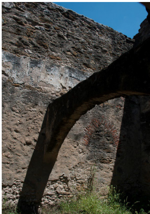
Figure 6.B.49: Room HS 203 D—North wall, right area. General view.
