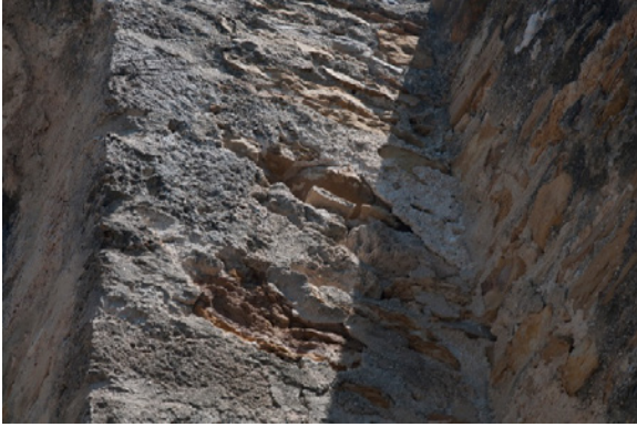
Figure 6.B.92: Room HS 203 B—North wall. Upper right corner features numerous holes and fragmentation of the stones.
