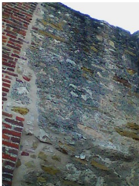
Figures 6.B.162 and 6.B.163: Room HS 203 H—North wall. Same view of the right part of the wall. The differences in temperature are caused by the different construction materials, the presence of humidity and the presence of the flue inside the chimney.
