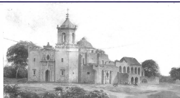
Figure 4.32: 1854 Hermann Lungkwitz drawing shows both the flying buttress and the gable roof in the same position as they were in the 1850 ITC drawing (SACS, Raba Collection).
