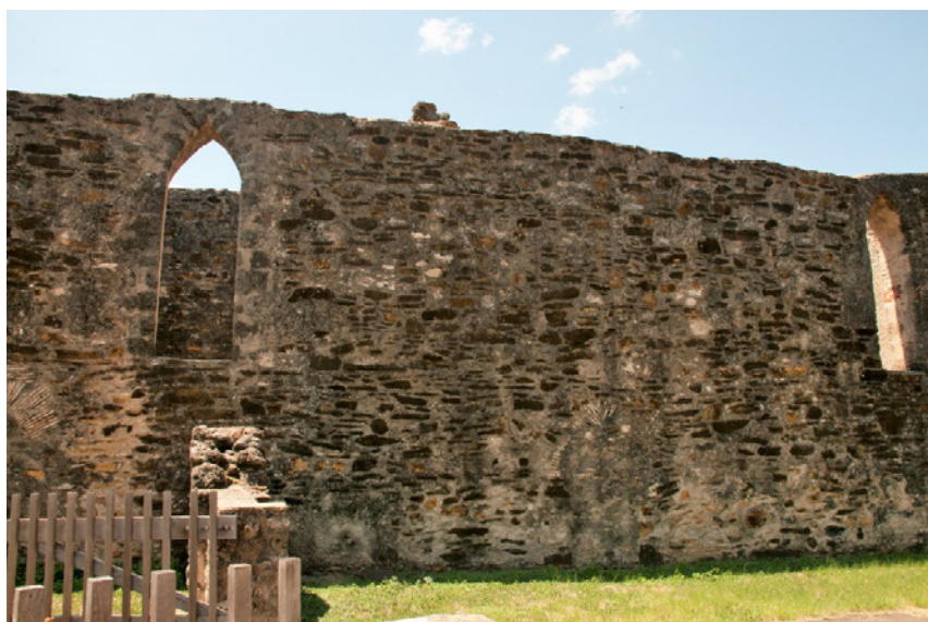
Figure 6.B.190: Exterior walls—North wall. General view of the middle part of the wall.
