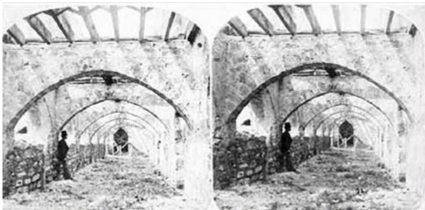
Figure 4.37: West view, showing the upper level of the porteria. In this ca. 1868 photograph, the flying buttress in the south end of the south arcade has become part of a wall (SACS, Raba Collection).
