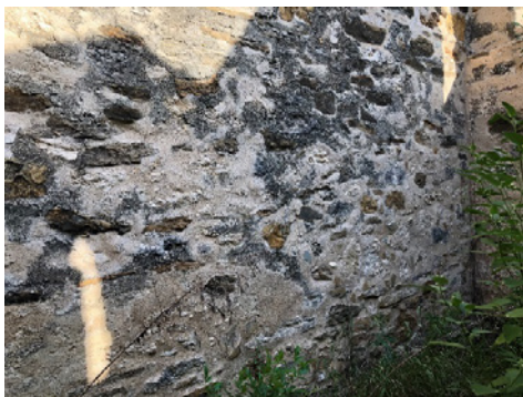
Figure 6.B.140: Room HS 203 P—West wall.
