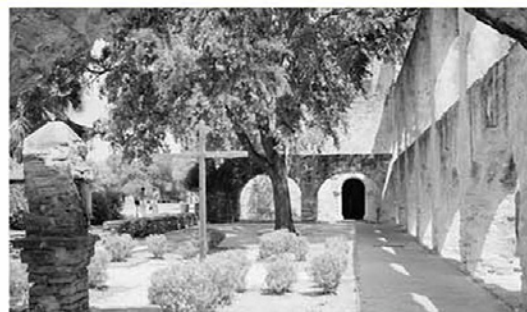
Figure 4.70: Southeast view of the courtyard. The porteria has already been restored to its current state. John Lowe photograph, 1983 (HABS, Library of Congress).
