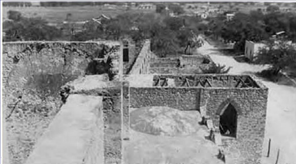
Figure 4.59: View of the convento from the northeast, from the bell tower of the church. The upper part of the porteria hasn't collapsed yet, and the timber structure of its roof can be partially seen. Albert Schaal photograph, 1927-31 (ITC UTSA).
