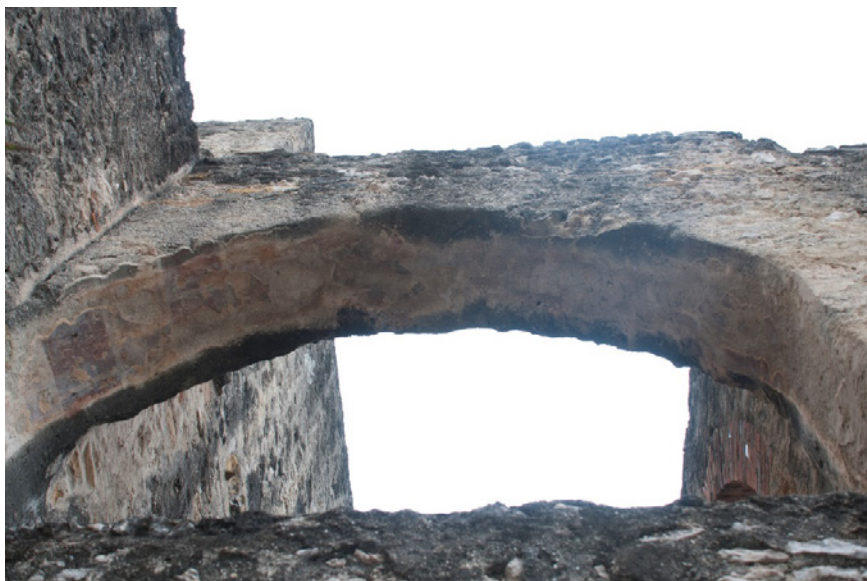
Figure 6.B.2: Room HS 203 S—North wall, upper-level arch showing the remnants of historic painted plaster in its intrados.
