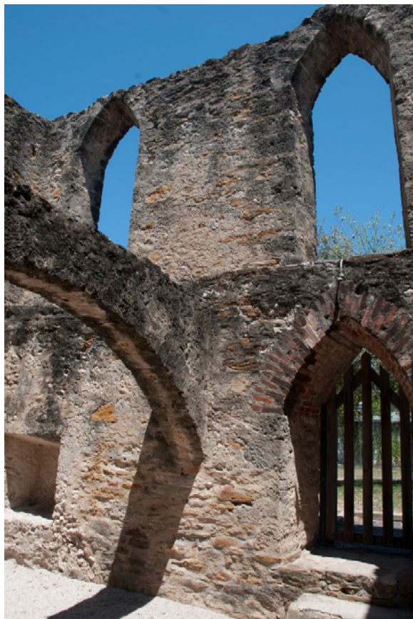
Figure 6.B.87: Room HS 203 B—North wall. General view.
