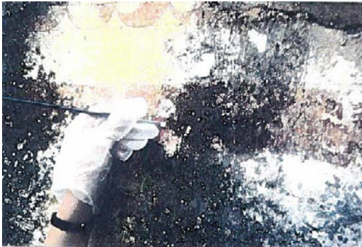
Figure 6.A.33: HS 203C — Dry brush cleaning of painted plaster.
