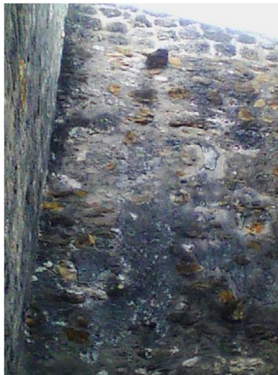
Figures 6.B.35 and 6.B.36: Room HS 203 A—North wall. Same portion of wall is shown in both photos. Left photo shows temperature differences in the wall, indicating different materials exhibit different temperatures. Considering that the wall has areas of old plaster and mortar patching, the difference of temperature can also be due to the detachment of these surfaces.
