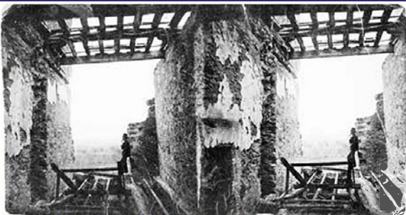
Figure 4.46: View from the upper level of the west part facing north. The timber structure of the roof and floor, as well as the fallen part of the north wall, are visible. Unattributed photograph, ca. 1885 (Personal collection of Lewis Fisher).
