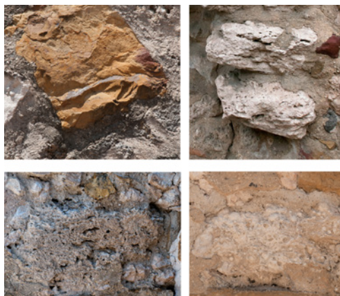
Figures 6.B.1a, 6.B.1b, 6.B.1c, 6.B.1d: These photos illustrate the types of stone found in the walls of Mission San José convento. They are (clockwise from top left ) Wilcox sandstone, white limestone, pisolithic limestone, and the so-called "tufa," which is a macro-porous limestone.
