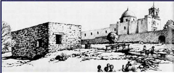
Figure 4.25: View of the North wall of the convento. Rectangular windows are seen in the upper level of the convento, 1790s (Fisher, 1998, p.12; Ernst Schuchard, DRT _ Drawing).
