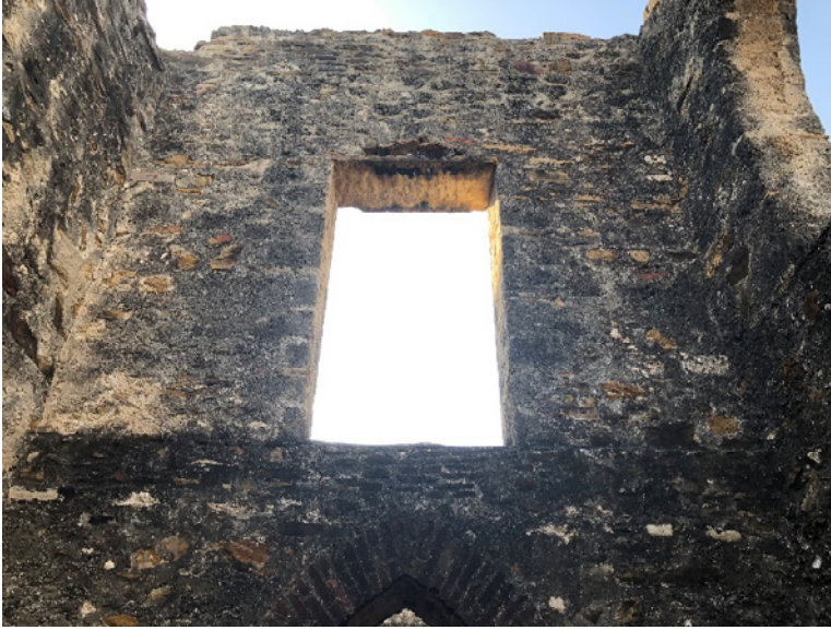
Figure 6.B.60: Room HS 203 D—East wall, upper part features a thick layer of biological growth that is less intense in the upper left area.
