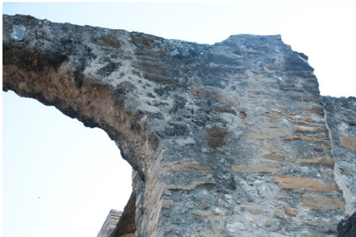
Figures 6.B.146 and 6.B.147: Room HS 203 H—North wall upper-level arch, which features fragmentation and delamination of stones in its right side.
