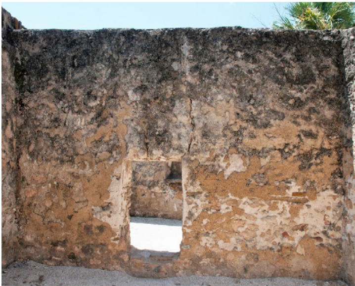
Figure 6.B.169: Room HS 203 K—South wall. General view. Feature biogrowth in the upper part, erosion in the bottom area and visually disturbing mortar patchings.
