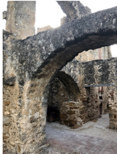
Figures 6.B.225 and 6.B.226: Exterior walls—West wall. Area corresponding to room 203 H. Exhibits vegetation growth in the arch and a high level of erosion.
