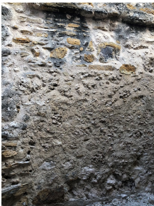
Figure 6.B.34: Room HS 203 F—West wall, which features vegetation growth in the upper part, erosion in the bottom part, and brown mortar patching.
