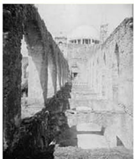
Figure 4.69: View from the upper level of the south arcade toward the west. Arthur W. Stewart photograph, 1936 (HABS, Library of Congress).
