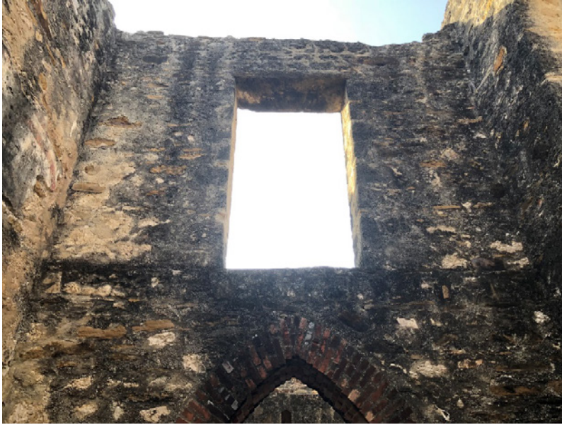
Figure 6.B.80: Room HS 203 C—East wall. General view of the upper level.
