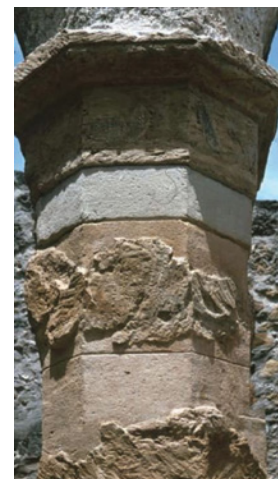
Figure 6.A.9: The Column after treatment.
