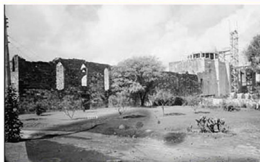
Figure 4.68: Northeast view, restoration work by Harvey P. Smith is visible in the north wall. Arthur W. Stewart photograph, 1936 (HABS, Library of Congress).
