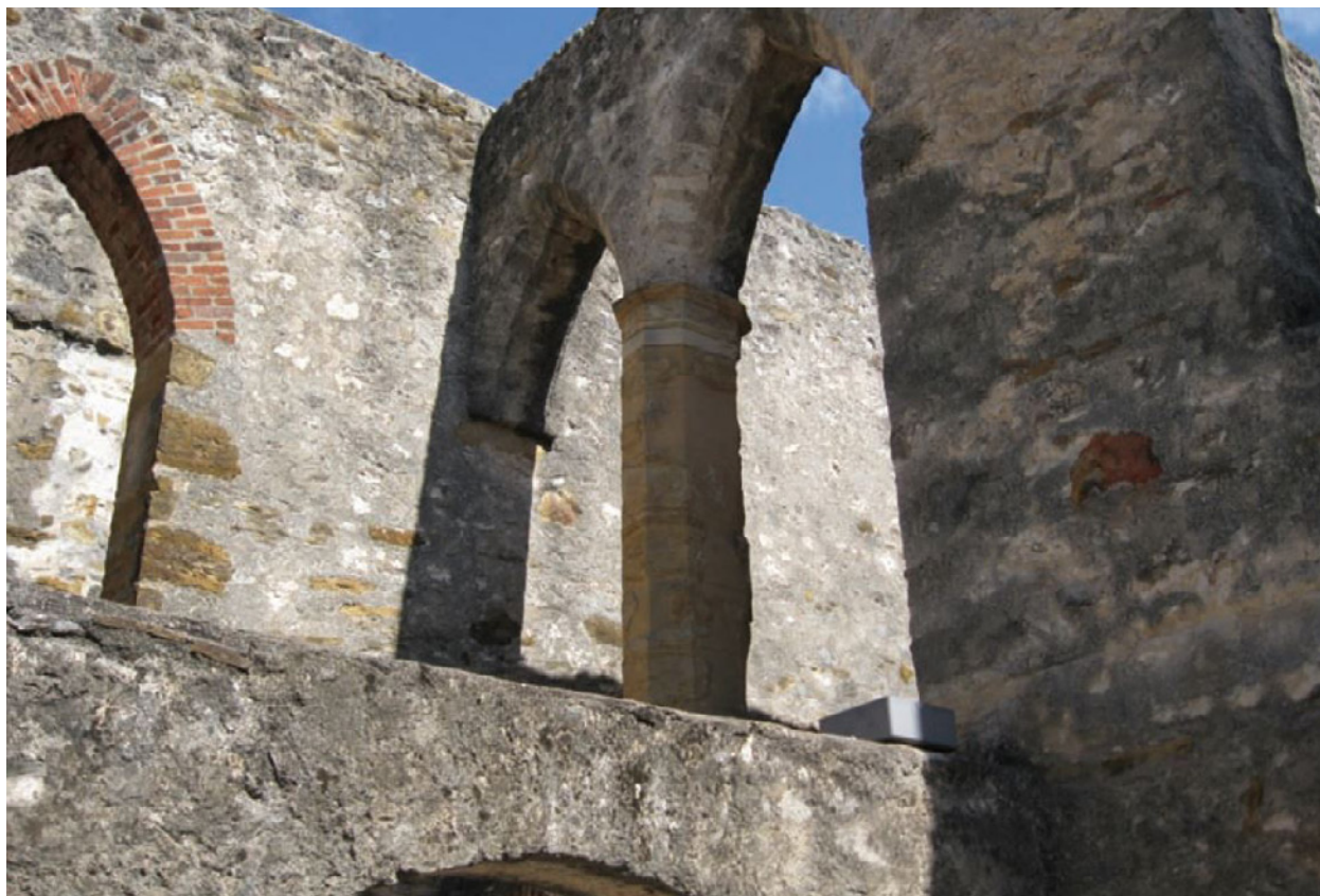
Figure 6.A.1: The octagonal column is constructed out of nine locally impure fine-grained limestone drums and laid with a gypsum-lime bedding mortar. Intended to be an interior element, the column has been exposed to the outdoor conditions since its construction by the Benedictines. The 2012 study by McNabb identifies causes of deterioration of the convento column.
