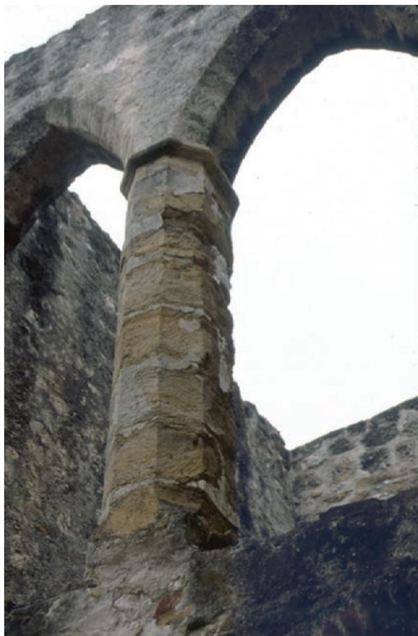
Figure 6.A.5: The southeast elevation of the column prior to the 1993 treatment.
