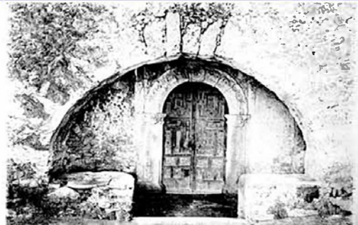
Figure 4.62: View of the right arch of the porteria, prior to 1930s (Noonan Guerra, The Missions of San Antonio, p. 11, DRT Library).
