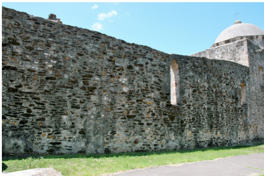
Figure 6.B.189: Exterior walls—North wall. General view of the right (west) part of the wall.
