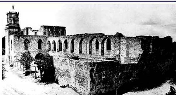
Figure 4.52: Southeast view, demonstrating that the window in the south wall of the east part has been closed. Moreover, a crack in the east wall of the refectory is visible. Unattributed photograph, ca. 1900s, (Nelson, 1998, p. 75).
