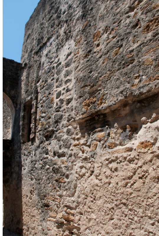
Figure 6.B.26: Room HS 203 F—West wall. General view.
