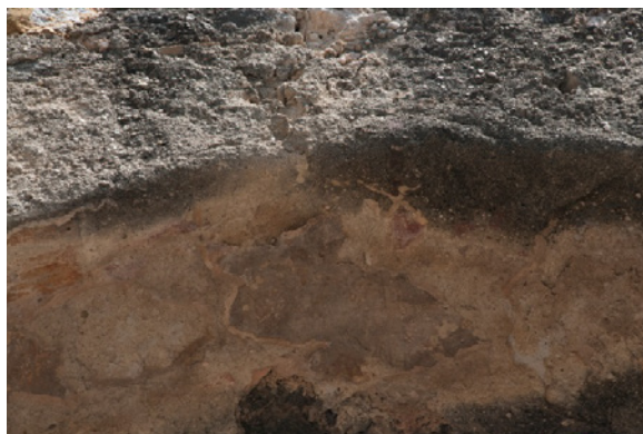
Figure 6.B.3: Room HS 203 S—North wall, upper-level arch. Detail of the painted plaster showing detachment of edges.
