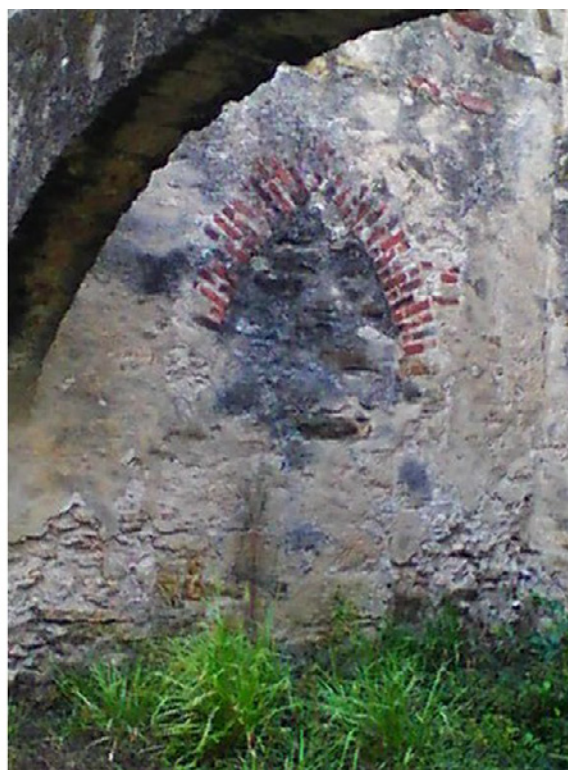
Figures 6.B.58 and 6.B.59: Room HS 203 D—North wall. Same portion of wall—a detail of the right area—is shown in both photos. Left photo shows temperature differences in the wall. The difference in the temperature seems to be caused both by the difference of materials used in construction (brick, limestone, sandstone, mortar) and the level of humidity—the bottom part, which shows erosion due to rising damp, is the colder area.
