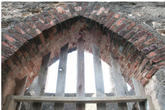
Figure 6.B.64: Room HS 203 D—South wall. Detail of the right bottom lancet arch features vegetation growth, efflorescence, and fragmentation of the brick in the intrados of the arch.
