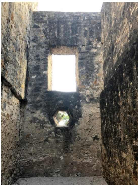
Figure 6.B.14: Room HS 203 F—North wall.
