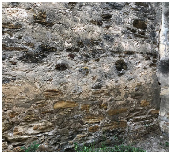
Figures 6.B.46 and 6.B.47: Room HS 203 A—West wall. Patching mortar at the base of the wall has been eroded.
