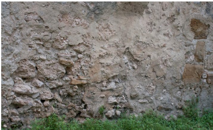
Figure 6.B.72 and 6.B.73: Room HS 203 C—North wall. Both images show the same view of the north wall area to the right of the transverse arch. Left photo shows temperature differences in the wall. Temperature changes in the bottom part appear to be due to rising damp, and those in the right part due to the presence of the former door opening D02, now closed in with masonry infill.
