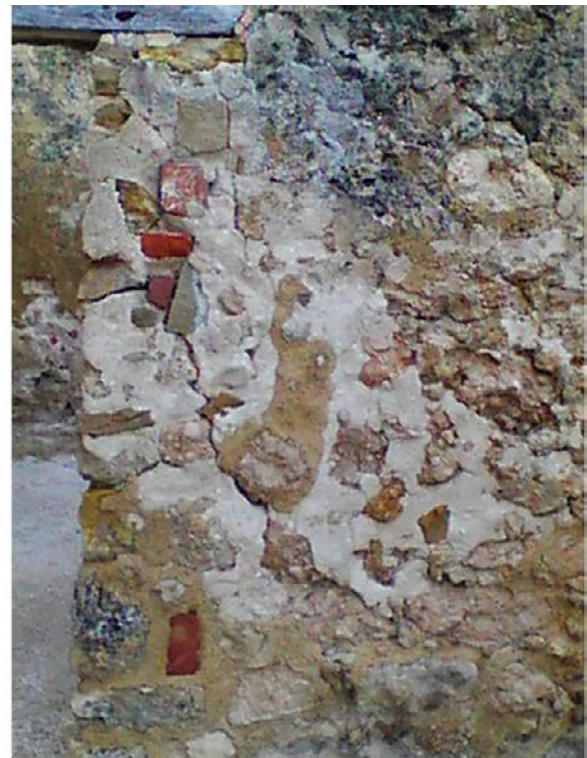
Figure 6.B.155: Room HS 203 H—East wall. Same view of the a detail of the right jamb of door D05 and nearby wall. The differences in temperature are caused by the different construction materials and the presence of humidity. Features a fracture that starts in the upper right corner of the door and develops diagonally downward.
