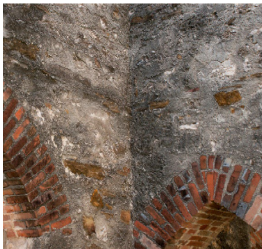
Figure 6.B.66: Room HS 203 D—Southwest corner detail.
