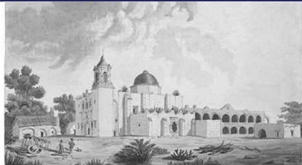
Figure 4.28: Southwest view, showing the canales and flying buttress in the upper level at the end of the south arcade. In addition, a window can be seen in the south wall of the east part. Drawing by Edward Everett, ca. 1847 (Amon Carter Museum).
