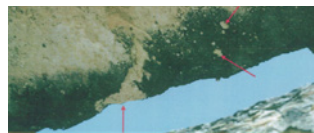
Figure 6.A.24 (above): Arch 1 E—Detail illustrating recent loss of material.
