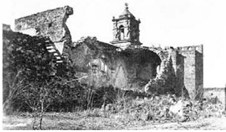
Figure 4.40: Northeast view, showing the collapse of part of the north wall of the church and the convento. The shadows of the timber beams of the roof of the convento can be seen in this ca. 1877 photograph (ITC UTSA).
