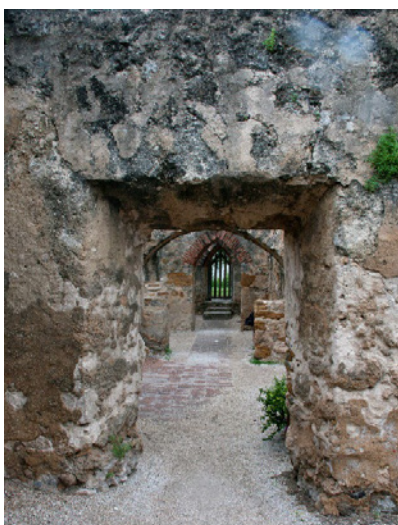
Figure 6.B.175: Room HS 203 R—North wall. Detail of the left door D13. Features a crack in the middle of the architrave.
