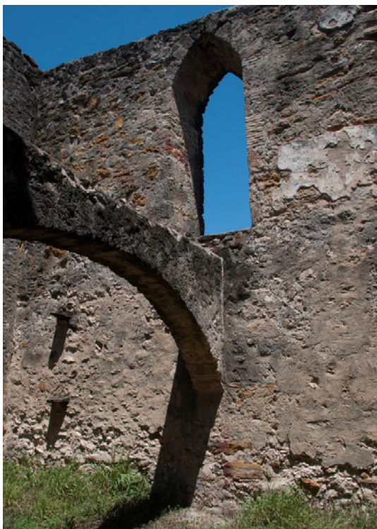
Figure 6.B.48: Room HS 203 D—North wall, left area. General view.
