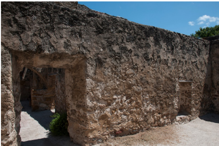
Figure 6.B.175: Room HS 203 R—North wall. Detail of the left door D13. Features a crack in the middle of the architrave.
