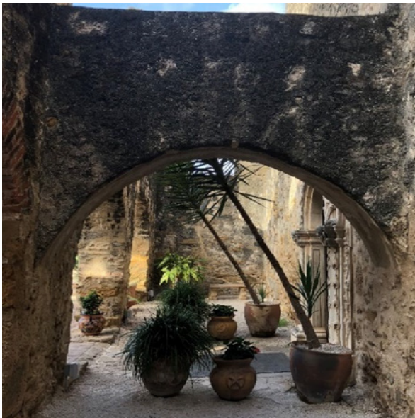
Figures 6.B.28, 6.B.29, and 6.B.30: Room HS 203 F—South wall. Figure 6.B.29 is a detailed photo of the intrados of the upper-level arch, showing the remnants of painted plaster (red color).
