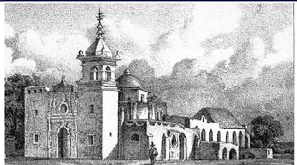
Figure 4.30: View from the west, showing the same features of the previous drawings with the addition of a gable roof in the southern end of the upper level, ca. 1850 (ITC, Rau & Son lithographers, from a drawing by Hermann Lungkwitz).
