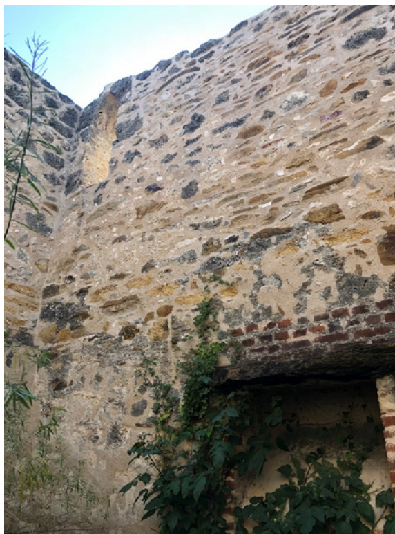
Figure 6.B.138: Room HS 203 P—East wall. The wall has been repointed recently and features several fragmented sandstones.
