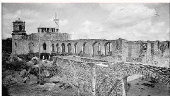
Figure 4.67: Southeast view. A new wall has been added in the southeast corner of the convento. Arthur W. Stewart photograph, 1936 (HABS, Library of Congress).
