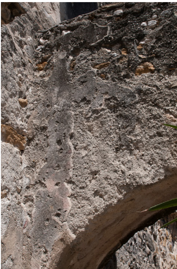
Figure 6.B.5: Room HS 203 S—North wall, lower-level arch. Detail of the left corner of the arch which features remnants of historic plaster.
