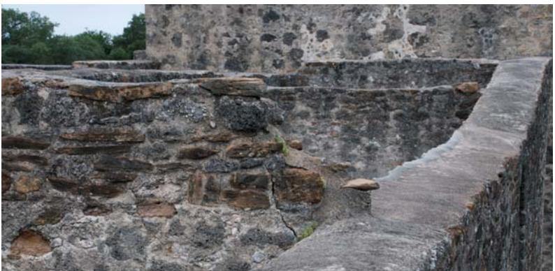
Figures 6.B.251–6.B.253: Wall between 203 D and 203 C—Views of the wall connection, exhibiting a diagonal fracture.
