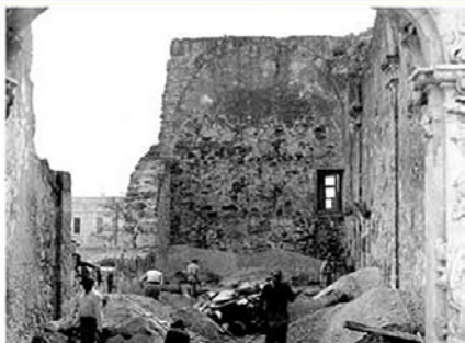
Figure 4.63: View from the door of the church to the east. The north wall has already been partially reconstructed. Unattributed photograph, ca. 1934, (Fisher, p.23).
