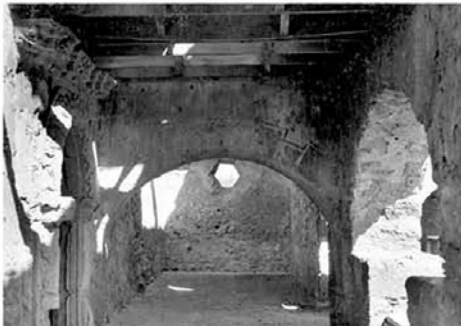
Figure 4.57: View of the ground floor of the porteria toward the northeast, showing the timber roof of this area, as well as the arch's painted decoration. Unattributed photograph, 1927 (ITC UTSA).
