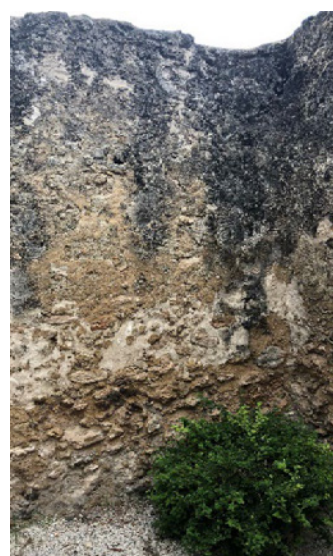
Figures 6.B.149, 6.B.150, and 6.B.151: Room HS 203 H—East wall. General view. Features vegetation growth in the upper part of the wall and erosion in the lower part.
