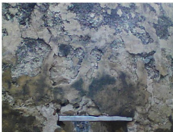
Figures 6.B.177 and 6.B.178: Room HS 203 R—North wall. Same view of the area above the right door. The differences in temperature are caused by the different construction materials, the presence of humidity and the detachment of the patching.
