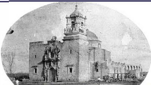
Figure 4.33: In this 1854 photograph, the flying buttress can be seen at the south end of the south arcade (Fisher, 1998, p. 59).
