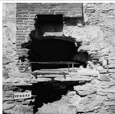
Figure 4.66: View of the northeast wall of the kitchen. In the picture is revealed an arch embedded in the wall. Arthur W. Stewart photograph, 1936 (HABS, Library of Congress).
