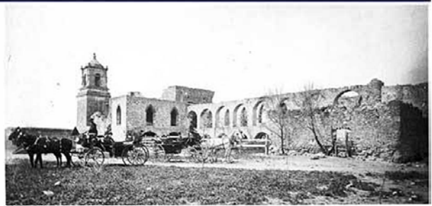
Figure 4.45: South view, from which a window in the south wall of the east part is clearly visible. Unattributed photograph, ca. 1885 (Personal collection of Lewis Fisher).
