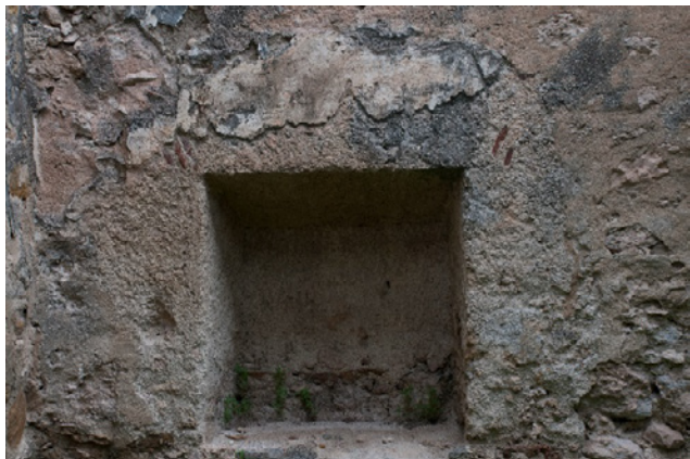
Figure 6.B.71: Room HS 203 C—North wall, lower level. Niche N01 with a fragment of Spanish Colonial plaster finish.
