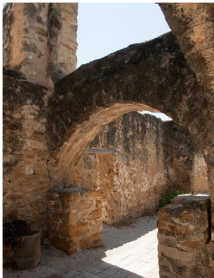
Figure 6.B.123: Room HS 203 E—South wall. View of the lower east end.
