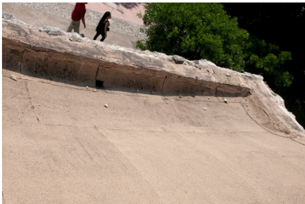
Figure 6.B.239: Roof of the convento. Photo facing southeast, showing the southeast corner of the roof of the library.
