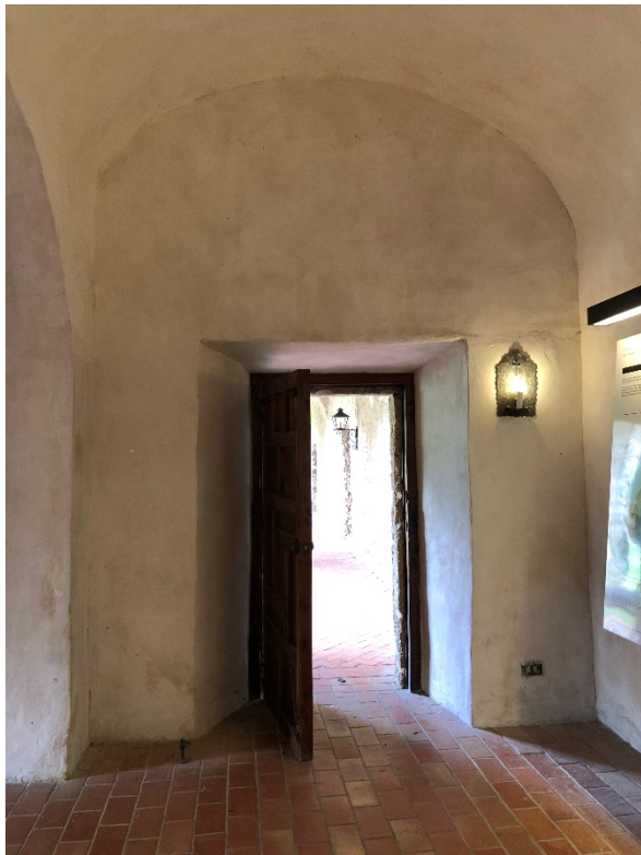
Figure 6.B.104: 104 F Refectory—North wall. Modern plaster covers the wall surfaces of the refectory.
