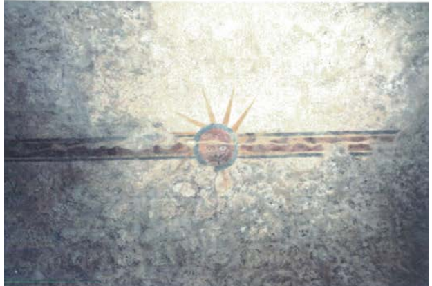
Figure 6.A.53: Post treatment conditions of the vault at the library, July 1988. Reprinted from 1988 Conservation Project Completion Report... , by Anthony Crosby, 1997, p. 61.
