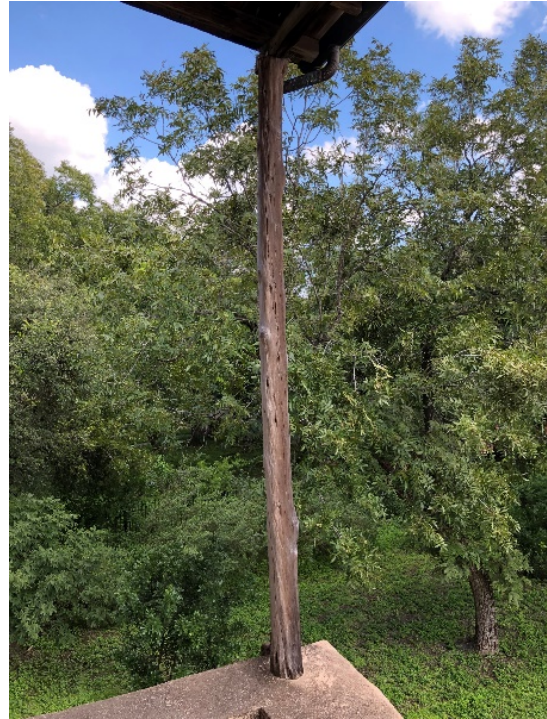
Figure 6.B.144: Wood pillar on the south-eastern corner of the balustrade.
