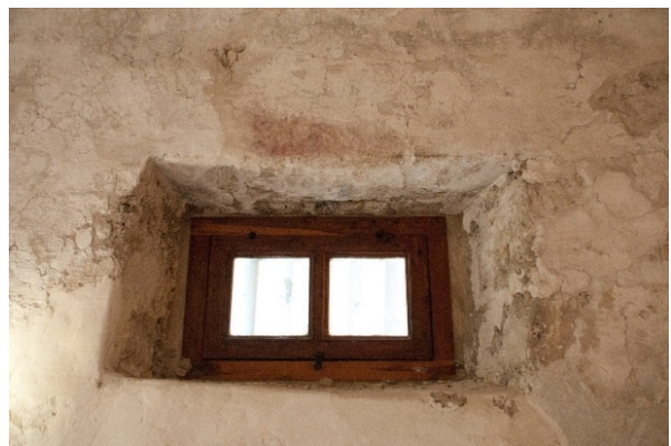
Figure 6.B.48: 104 B—West wall window detail (B4, C4). Detail of the remnants of painted plaster in the upper part of the window.
