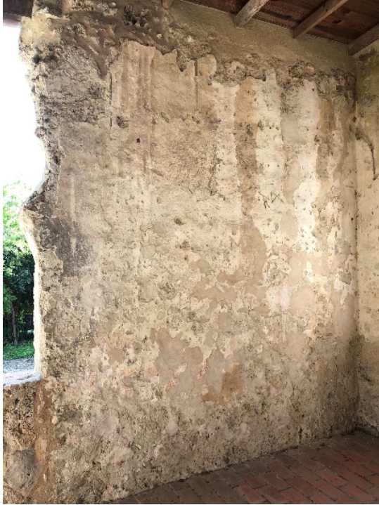
Figure 6.B.143: South wall on the upper floor.
