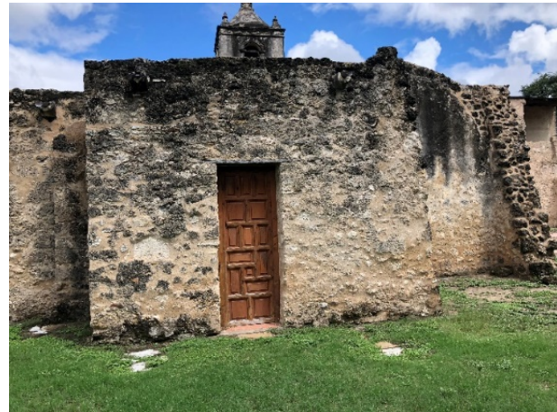
Figure 6.B.204: South wall (segment C), corresponding to the refectory. Also features biological growth, with a darker patina on the parapet.
