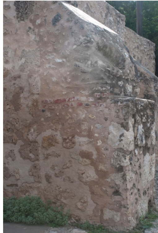
Figure 6.B.225: Exterior southwest buttress, reshaped after 1890s. Note the different types of repointing material
