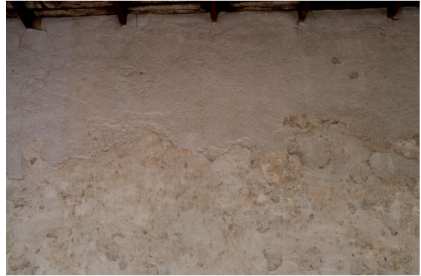
Figure 6.B.127: North wall (D4, D5). Shows the meeting point of the historic plaster and the latex paint from 1980s.
