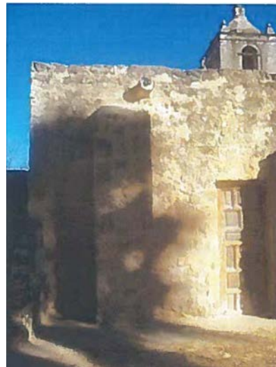
Figure 6.A.85, 6.A.86: e) and f) Rainwater runs through the canal creating splash on the hard surface, causing damp areas on newly repointed surfaces and damage to the painted surface of the interior. Reprinted from Documentation of South & East Exterior Walls... , by Restoration Associates Limited, 2009, p. 7.
