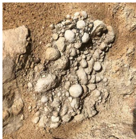
Fig. 6.B.4: Masonry may include some sedimentary limestones, ‘pisolithic stones,’ featuring large aggregates of river origin.
