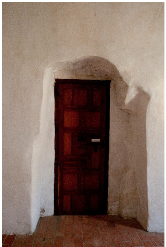
Figure 6.B.111: Room 104 F Kitchen—South wall.
