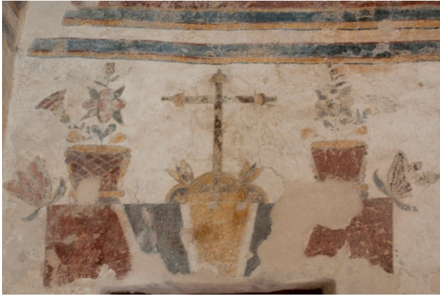
Figure 6.B.78: 104 E Library—North wall (B3, B4, C3, C4). Photo showing the painted decorations around the door that leads to the portería. Some non-intrusive patching has been added to give continuity to the plaster.
