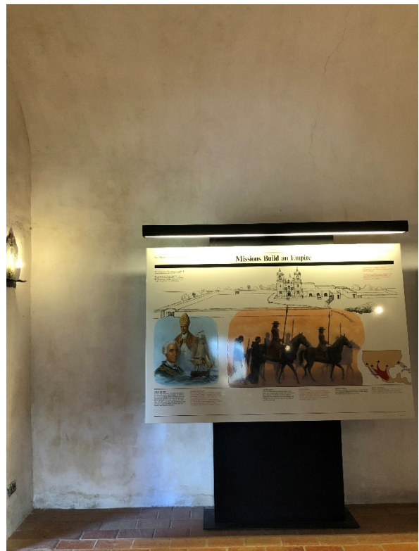
Figure 6.B.105: 104 F Refectory—East wall. On the northeast corner, stains due to moist areas are visible, due to the low porosity of the new plaster materials.
