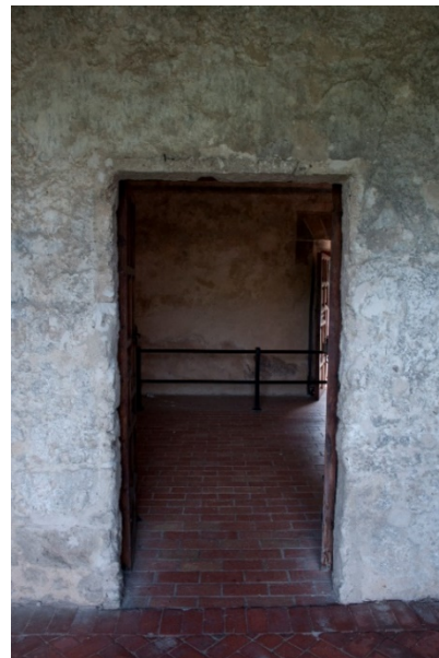
Figure 6.B.15: 104 A—East wall (A16, A17, B16, B17, C16, C17), door leading to the library. At the sides of the door there are areas where limewash has been directly applied to the tufa rubble stone. In the architrave of the door there are remnants of historic plaster.
