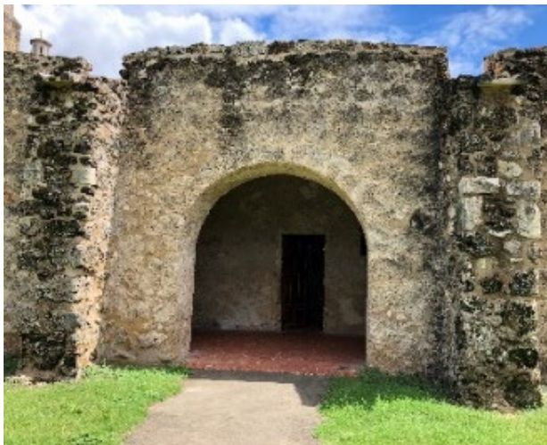
Figures 6.B.184, 6.B.185: West wall features five large buttresses between four arched openings into the corridor.
