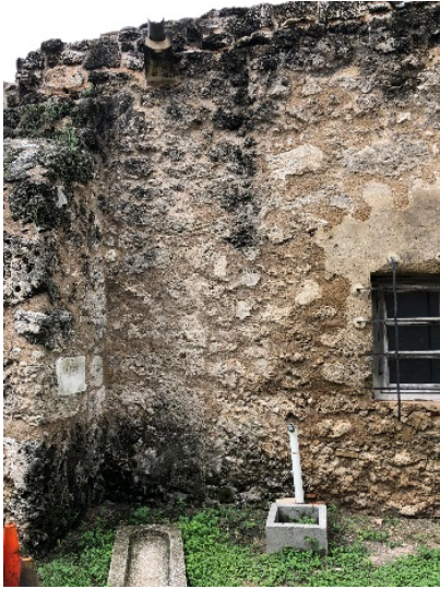
Figures 6.B.212–6.B.214: East wall (segment A), corresponding to the guest room. This wall affected by biological growth, moist areas, stone fragmentation, delamination, and erosion.
