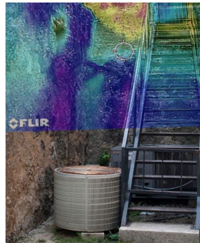
Figures 6.B.215–6.B.216: North wall of the guest room. The condition of this wall is critical, with thick layers of biological growth and wall erosion. High moisture contents are enhanced by incorrect water drainage both at the roof and ground levels.
