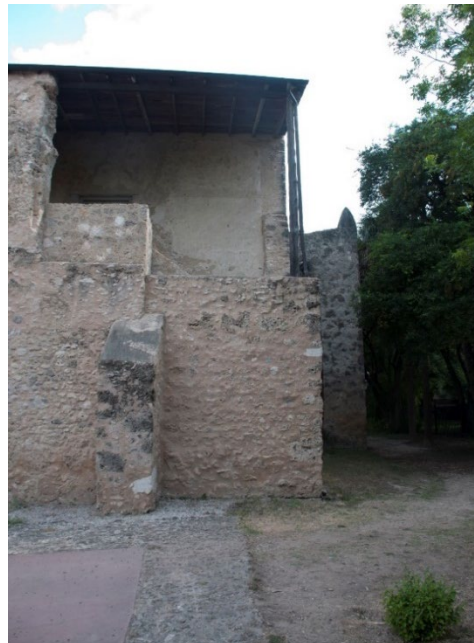
Figure 6.B.223: Exterior south wall.
