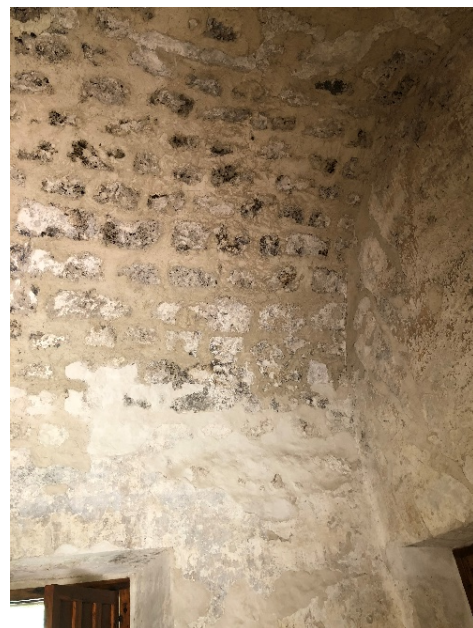
Figures 6.B.72, 6.B.73: 104 D Portería—Portions of the barrel-vaulted ceiling feature a surface made of roughly cut blocks with modern repointing of the joints. Stone blocks are characterized by a darker color, probably due to biological growth. Traces of whitewash are also presents on various blocks.
