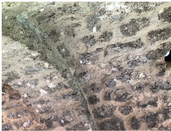
Figure 6.B.19: 104 A—Ceiling detail (B11, B12).
