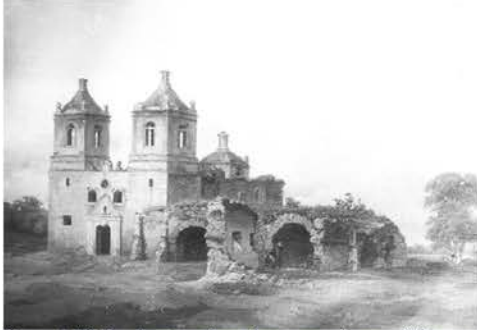
Figure 4.20: The drawing shows how several areas of the convento have collapsed. Photograph of a Hermann Lungkwitz drawing, 1850 (Institute of Texan Cultures)
