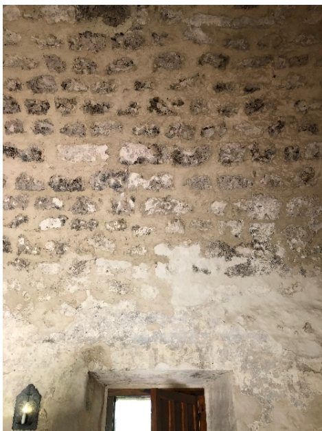
Figures 6.B.72, 6.B.73: 104 D Portería—Portions of the barrel-vaulted ceiling feature a surface made of roughly cut blocks with modern repointing of the joints. Stone blocks are characterized by a darker color, probably due to biological growth. Traces of whitewash are also presents on various blocks.
