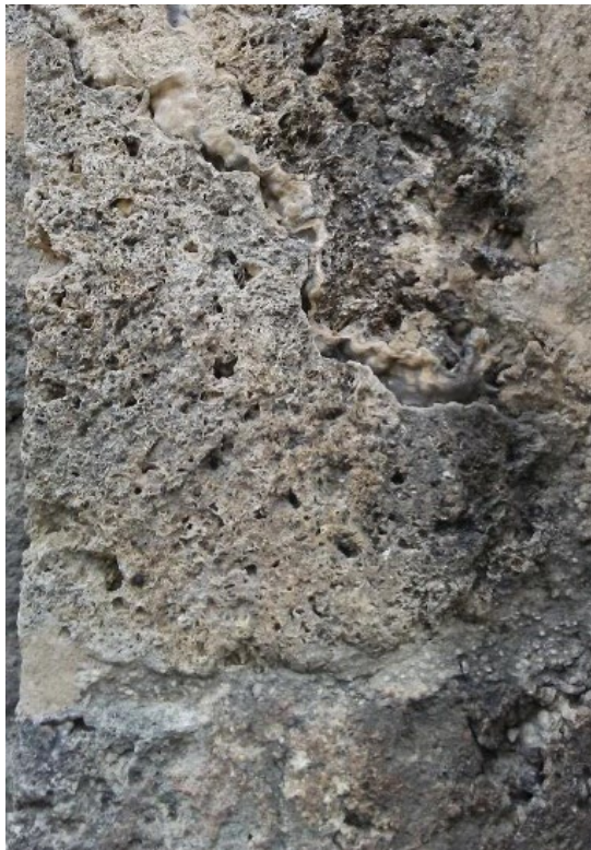
Figure 6.B.209: Brown mortar patching applied on the small tufa rubble.
