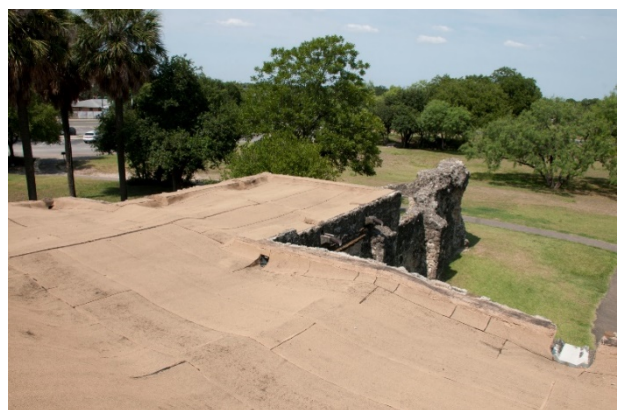
Figure 6.B.236: Roof of the convento. Photo facing the southwest, showing the roof of the west arcade, the refectory and the kitchen.
