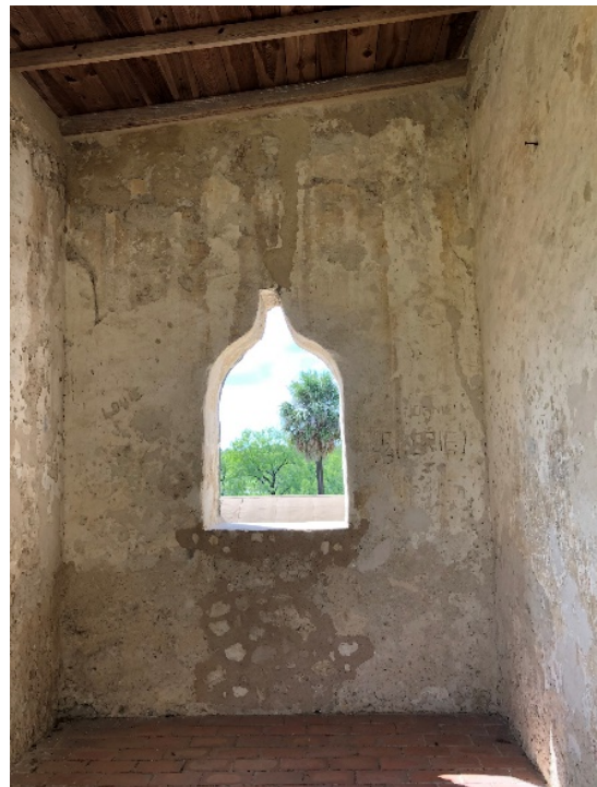
Figure 6.B.146: Moorish-styled window on the west wall.
