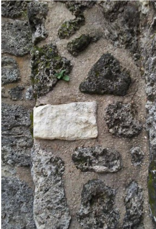
Figure 6.B.198: Infill Austin limestone block. Note the recent mortar repointing.
