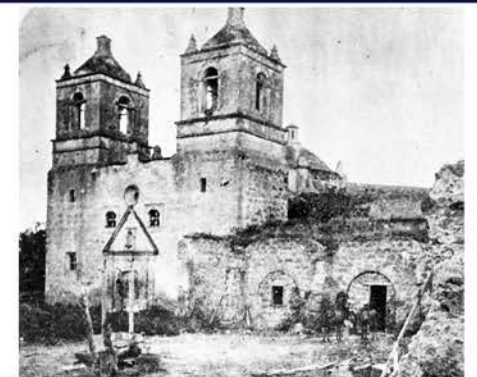
Figure 4.24: The picture shows that two of the arches of the west corridor have been closed. Ca. 1880s photograph (National Park Service Archive)
