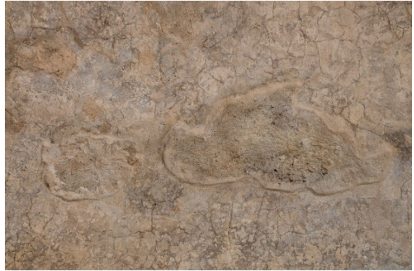
Figure 6.B.100: 104 E Library—West wall (D5). Craquelé of the historic plaster stabilized in one of the previous conservation campaigns. Intrusive brownish mortar patching.
