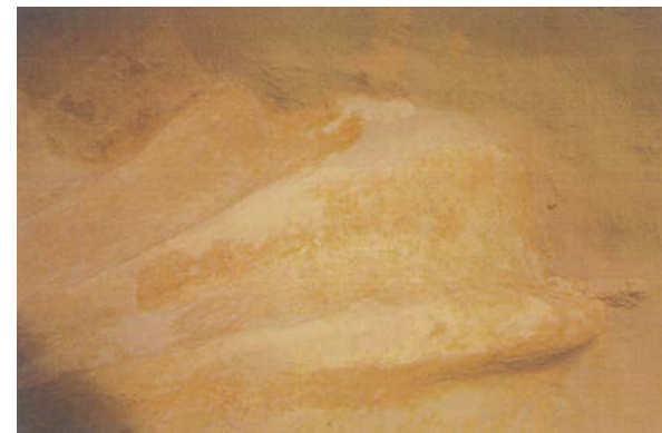
Figure 6.A.75: East wall. Historic tinted ochre lime wash. Reprinted from Exposing Historic Wall Plasters... , by Restoration Associates Limited, 2008, p. 13.
