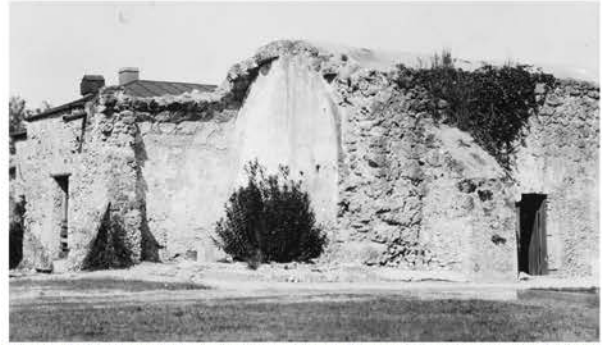
Figure 4.52: View of the southeast corner. Photo indicates the east buttress of the external wall of the refectory (B11) has been reshaped. Unknown date photograph (Institute of Texan Cultures)
