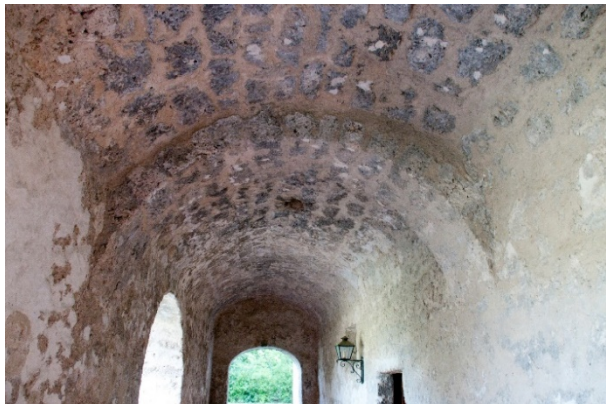
Figure 6.B.17: 104 A—Vault looking north.
