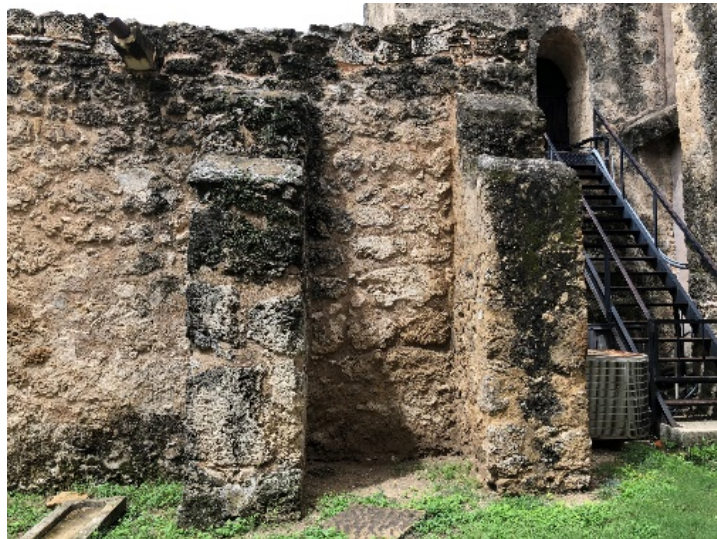
Figures 6.B.212–6.B.214: East wall (segment A), corresponding to the guest room. This wall affected by biological growth, moist areas, stone fragmentation, delamination, and erosion.
