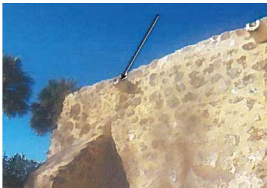
Figure 6.A.85, 6.A.86: e) and f) Rainwater runs through the canal creating splash on the hard surface, causing damp areas on newly repointed surfaces and damage to the painted surface of the interior. Reprinted from Documentation of South & East Exterior Walls... , by Restoration Associates Limited, 2009, p. 7.
