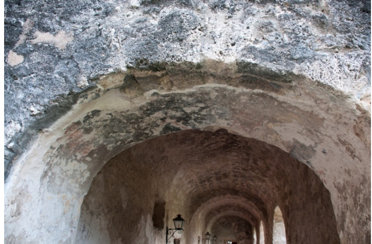
Figure 6.B.179: Exterior north elevation. Arch in the north wall of the corridor. Remnants of painted plaster (red and yellow).
