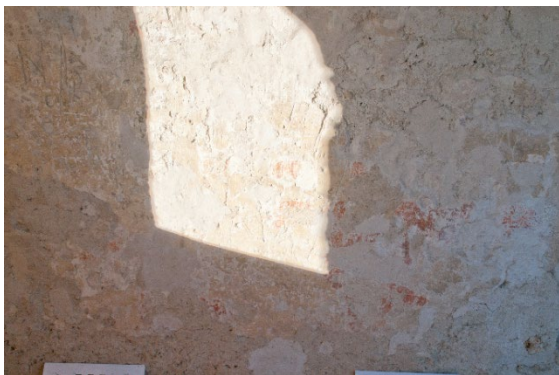
Figure 6.B.156: North wall. Area left of the door. Exhibits remnants of historic painted plaster (red/orange color) and different types of patching and historic graffiti.
