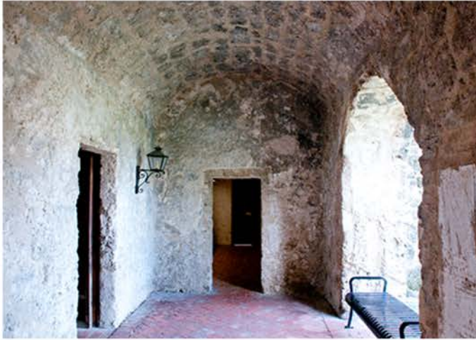
Figure 4.1: West corridor looking south (UTSA CCS)
