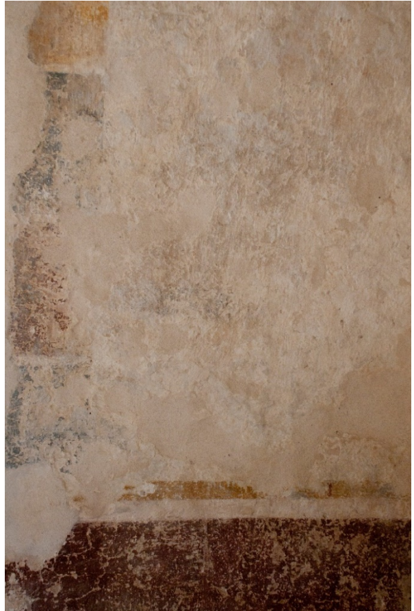
Figure 6.B.103: 104 E Library—West wall (A1, A2). Area on the right of the door. Decorative painted plaster with faux ashlar at the right jamb of the door. Two types of patching are featured—one visually harmonious that allows the visual continuity of the wall surface and another, with a more grayish tone, that is not visually blended.
