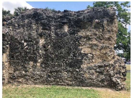
Figures 6.B.193, 6.B.194, 6.B.195: Northern wall covered in thick layer of algae, plants, and moss. The wall surface also features high level of stone erosion, fragmentation, and delamination.
