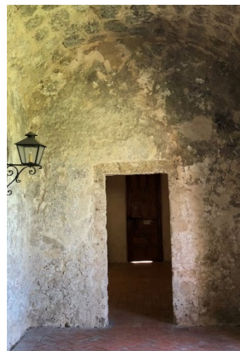
Figure 6.B.32: 104 A—Southern entry into the corridor. The area around the door previously covered by a door frame is clearly readable.
