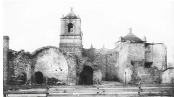
Figure 4.31: View from the south. Photo indicates the buttresses of the south wall of the staircase and the east wall of the convento haven't been built yet. 1898 photograph (USC Library)
