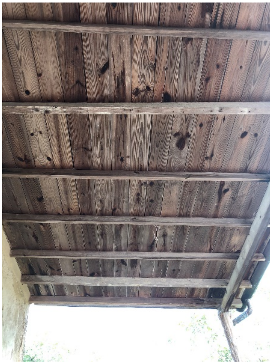
Figure 6.B.145: Ceiling, picture looking east.
