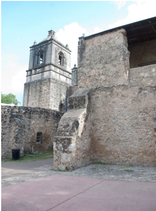
Figure 6.B.222: Exterior south wall. This façade is in good condition, recent repointing work can be seen between the two buttresses.
