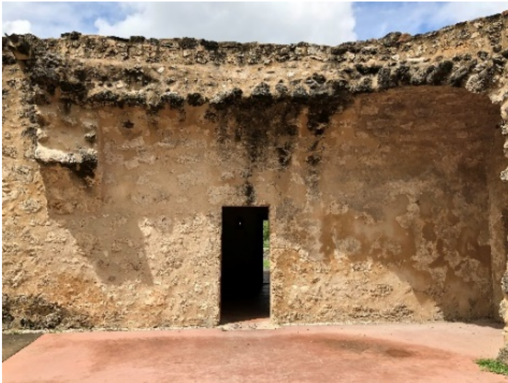
Figure 6.B.208: East wall (segment B), corresponding to the portería, in generally good condition.
