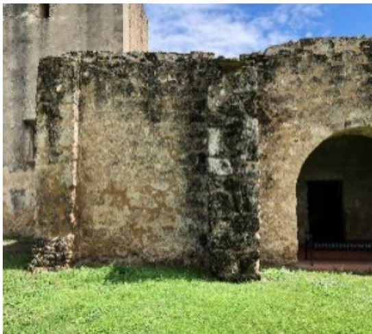
Figures 6.B.180, 6.B.181: West wall features five large buttresses between four arched openings into the corridor.
