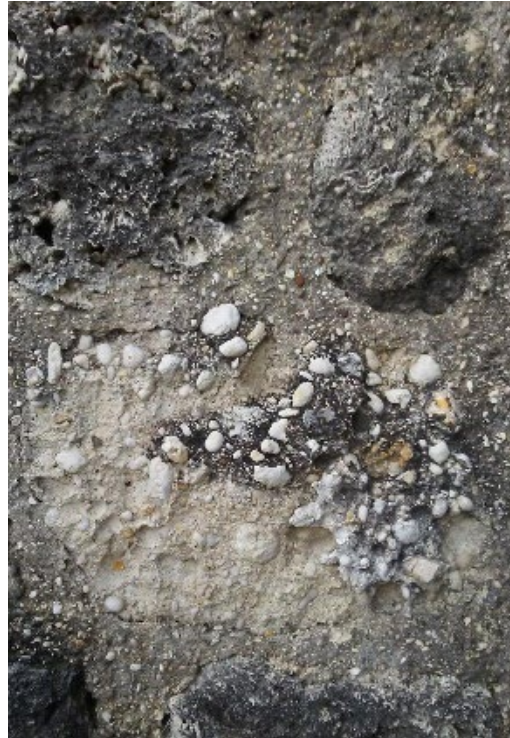
Figure 6.B.199: Differential erosion of a pisolithic rubble.
