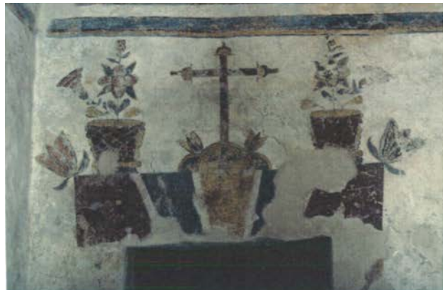
Figure 6.A.51: Post treatment conditions of the north door, August 1988. Reprinted from 1988 Conservation Project Completion Report... , by Anthony Crosby, 1997, p. 61.
