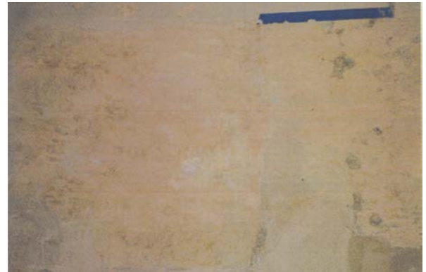
Figure 6.A.78: North wall. Interior door/window. Upper west section. The surface features historic ochre lime wash—with no evidence of incised lines. Reprinted from Exposing Historic Wall Plasters... , by Restoration Associates Limited, 2008, p. 13.
