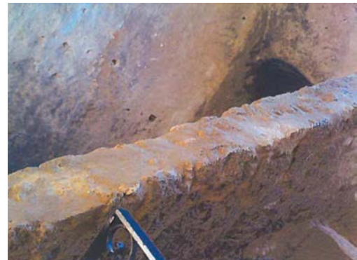
Figure 6.A.87: The top of stair wall was repointed. Reprinted from Documentation of South & East Exterior Walls... , by Restoration Associates Limited, 2009, p. 8.
