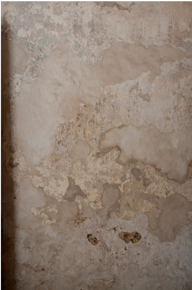
Figure 6.B.76: 104 D Portería—West part ceiling (F4, F5). Roughly executed mortar repointing that partially covers the stones.
