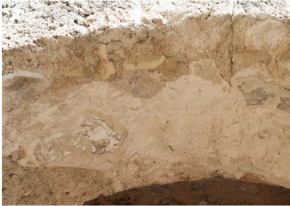
Figures 6.B.186, 6.B.187: Exterior west elevation. Middle arch of the west arcade. Remnants of painted plaster with edge stabilization from the conservation campaign of 1988.
