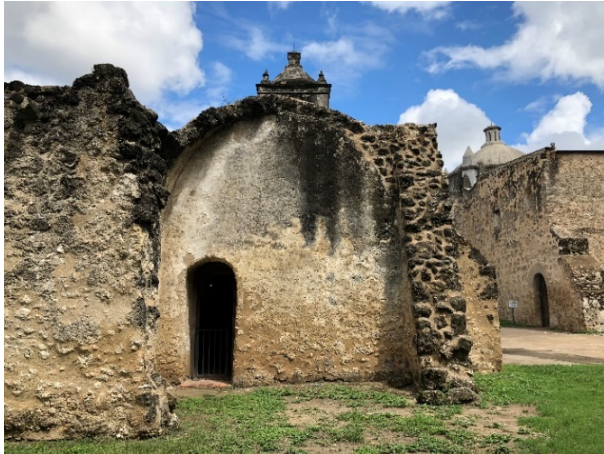
Figure 6.B.201: South wall (segment B), corresponding to the library.
