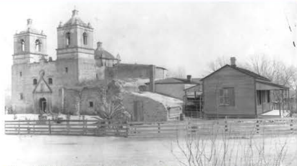
Figure 4.34: The picture shows the room that was built in the western part of the south wing, which included a brick chimney, and that a gable roof has been added to the part of the refectory and the kitchen. 1911 photograph (San Antonio Conservation Society)
