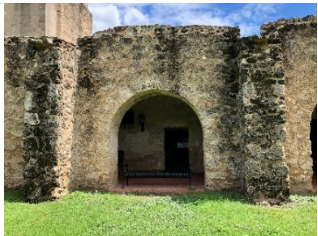
Figures 6.B.180, 6.B.181: West wall features five large buttresses between four arched openings into the corridor.
