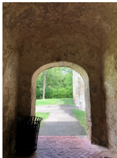
Figure 6.B.33: 104 A—Northern entry into the corridor.
