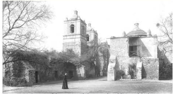
Figure 4.36: Picture of the courtyard showing the addition of the buttresses in the south wall of the staircase and in the east wall of the convento. 1919 photograph (San Antonio Conservation Society)
