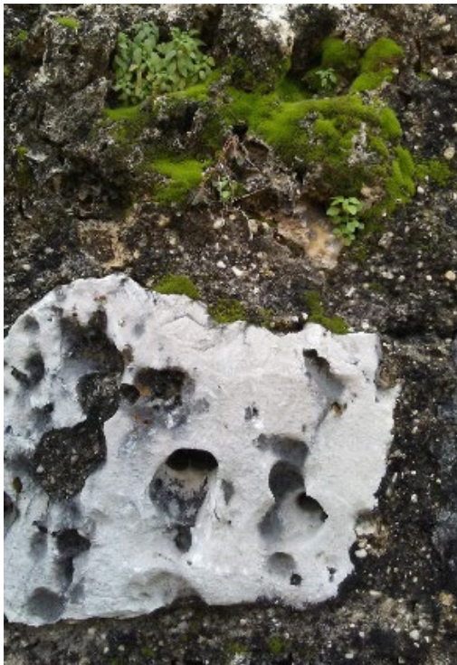
Figure 6.B.200: Detail showing moss (above) and a compact limestone rubble featuring alveolization.
