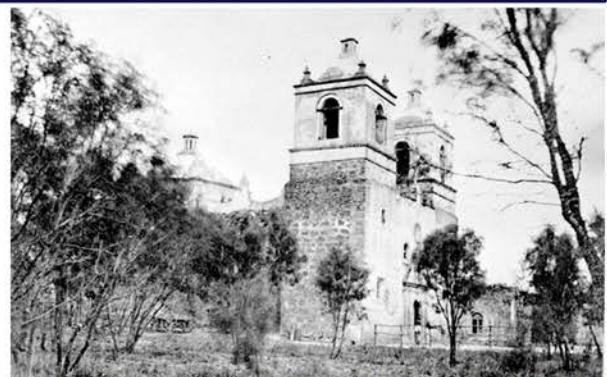
Figure 4.25: The arch of the north wall of the west corridor has also been closed and converted into a window. Date of photograph unknown (Institute of Texan Cultures)
