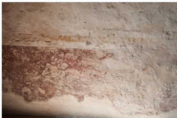
Figure 6.B.97: 104 E Library—West wall (A6). Bottom area of the wall features geometric decorative painted plaster (red and yellow) with well-executed plaster patching and differential erosion of the plaster surface.
