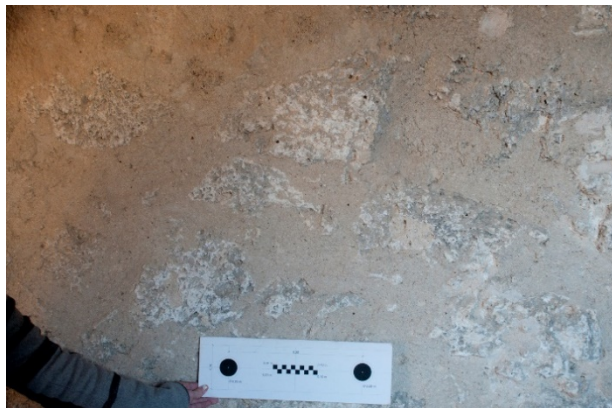
Figure 6.B.22: 104 A—Southern part of the east wall (B14, B15), limewash applied directly on the tufa rubble stone.
