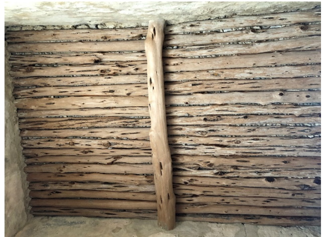
Figure 6.B.175: Modified after the 1850s, the ceiling is made from round wooden rafters, following the traditional Spanish technology of the period.
