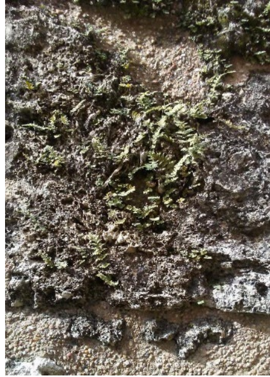
Figure 6.B.218: Detail of dark biological growth on tufa block.
