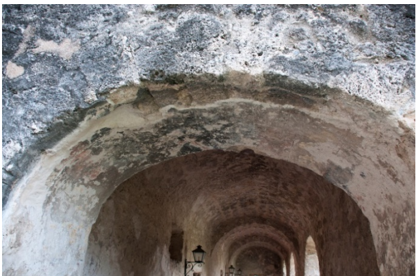
Figure 6.B.20: 104 A—Arch in the north wall of the corridor, remnants of painted plaster (red and yellow).
