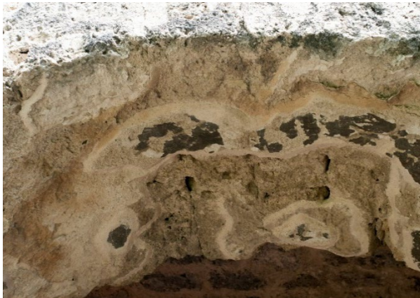
Figures 6.B.188, 6.B.189: Exterior west elevation. South arch of the west arcade. Remnants of painted plaster with painted finish and edge stabilization from the conservation campaign of 1988. Detachment of edges of the plaster layer.
