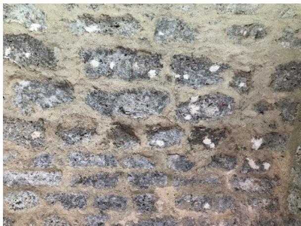
Figure 6.B.18: 104 A—Detail of the vault showing mortar patching.
