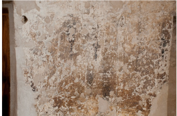
Figure 6.B.58: 104 D—Area between the door and the niche in the north wall (B3) features historic dark ochre colors and vertical black marks with dirt deposit. Small areas of visually intrusive patching.
