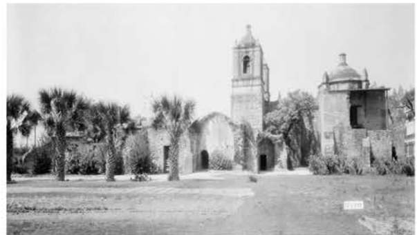
Figure 4.46: View of the convento and church from the south. It can be seen that the roof of Father President's office has been replaced. 1933 photograph (HABS, Library of Congress)
