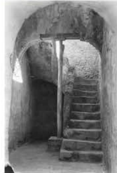
Figures 4.55 and 4.56: View of the staircase looking east. The middle part of the arch has been filled and a timber pillar has been added as structural reinforcement. Date of photographs unknown (Institute of Texan Cultures)
