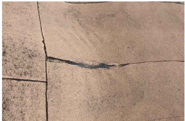
Figure 6.B.240: Roof of the convento. Detail of the roof.
