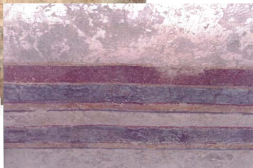
Figure 6.A.41: Cleaning—salts. Wall cornice prior to and after salt removal and cleaning. Reprinted from 1988 Conservation Project Completion Report... , by Anthony Crosby, 1997, pp. 48-49.
