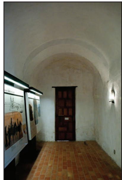
Figures 5.26, 5.27: Walls of the refectory (below) and kitchen (bottom photo) interiors feature a cement-based wash, painted white.
