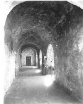
Figure 4.40: View from the inside of the west corridor looking south. 1921 photograph (San Antonio Conservation Society)
