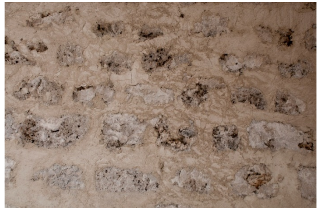
Figure 6.B.76: 104 D Portería—West part ceiling (F4, F5). Roughly executed mortar repointing that partially covers the stones.
