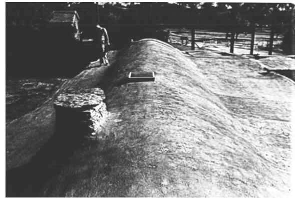
Figure 6.A.7: Roof condition in 1988. A design for roof replacement was carried out in 1988. Reprinted from Summary Project Report for the Paint and Plaster Conservation... , by Anthony Crosby, 1988, p. 10.
