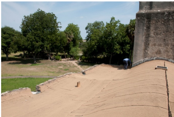
Figure 6.B.233: Roof of the convento. Photo facing north showing the roof of the west arcade and the connection of the convento with the tower of the church.
