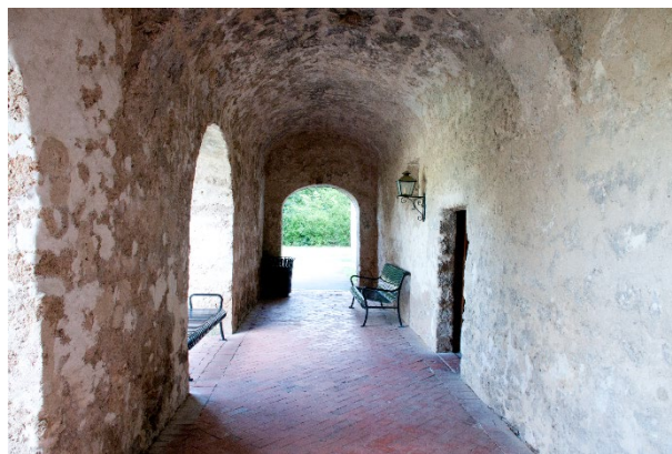
Figure 6.B.7: 104 A—View toward northern entry into the corridor. On the extreme left, the recent NHL (Natural Hydraulic Lime)-based patches are visible.
