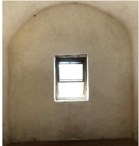
Figure 6.B.109: Room 104 F Kitchen—West wall.
