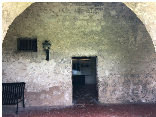
Figure 6.B.8: 104 A—East wall with door toward storeroom. On the left side of the door, a large remnant of historic plaster is visible, featuring erosion of its superficial finishes.
