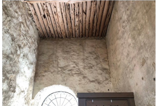
Figure 6.B.174: West wall in good condition.
