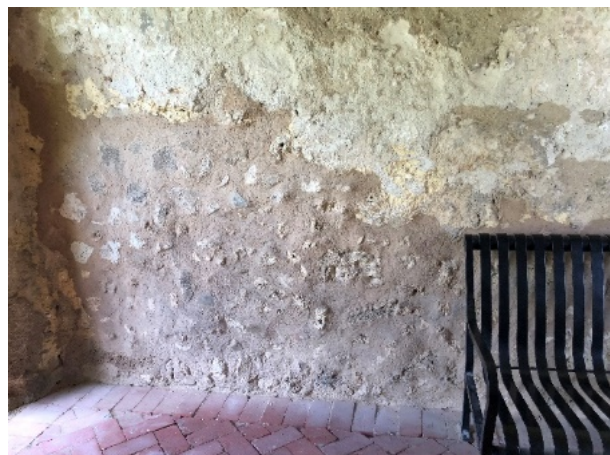
Figure 6.B.10: 104 A—Northern corner of the east wall (A1, A2), featuring brown mortar patching and masonry infill with irregularly laid small rubble limestone.
