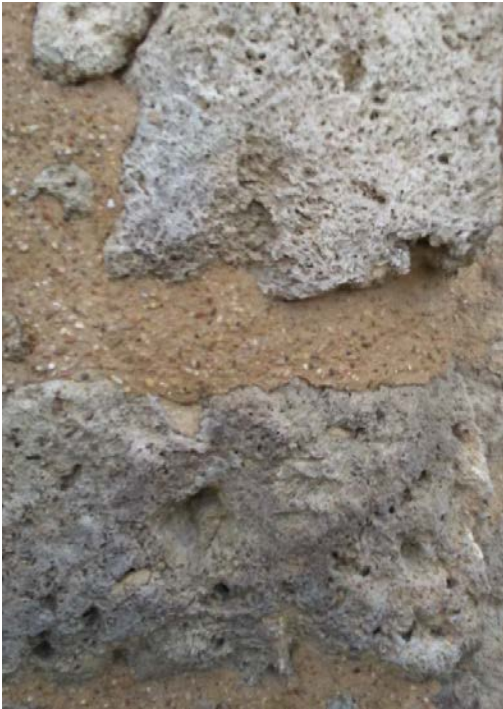
Figure 6.B.190: Detail of a buttress with no evident biological colonization.
