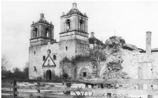
Figure 4.30: Picture indicates the west corridor remains closed and a small room has been built in the west end of the south wing. 1898 photograph (USC Library)
