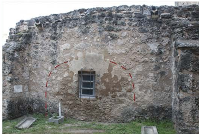
Figure 4.2: East corridor closed arch (UTSA CCS)
