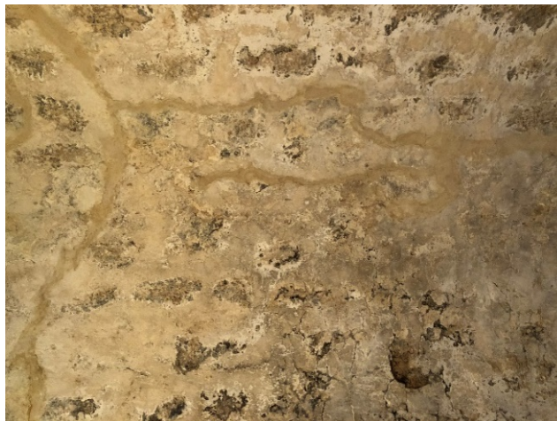
Figure 6.B.52: 104 C—North part of the ceiling (E5, E6, F5, F6). The barrel-vaulted ceiling is characterized by a scratch coat partially covering the rubble stones with numerous filled fractures. Its appearance looks non-historic.
