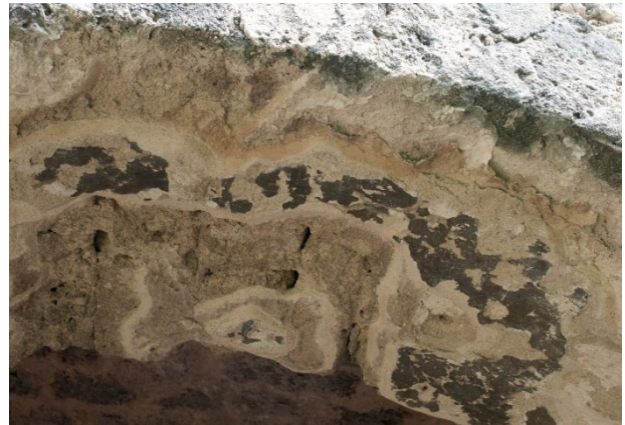
Figures 6.B.188, 6.B.189: Exterior west elevation. South arch of the west arcade. Remnants of painted plaster with painted finish and edge stabilization from the conservation campaign of 1988. Detachment of edges of the plaster layer.
