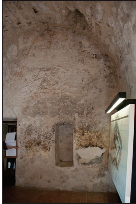
Figures 5.19, 5.20: Portería looking south (photo at far left) and north.
