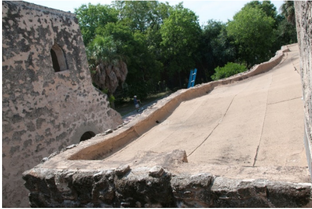
Figure 6.B.231: Roof of the convento. Roof of the guest room, view from the stair leading to the south tower of the church.
