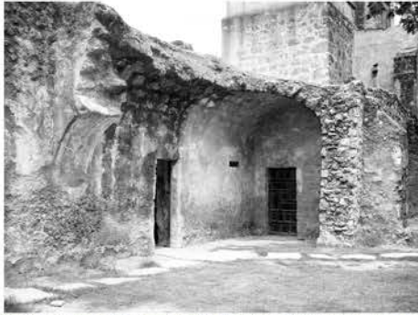
Figure 4.51: View of the east wall. Photo indicates the south buttress of the east wall (B15) has been reshaped. Unknown date photograph (Institute of Texan Cultures)
