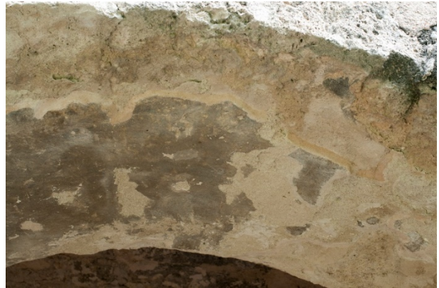
Figures 6.B.182, 6.B.183: Exterior west elevation. North arch of the west arcade. Remnants of painted plaster with edge stabilization from the conservation campaign of 1988. Detachment of edges of the painted finish.
