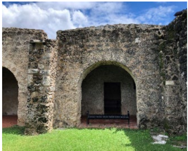
Figures 6.B.184, 6.B.185: West wall features five large buttresses between four arched openings into the corridor.
