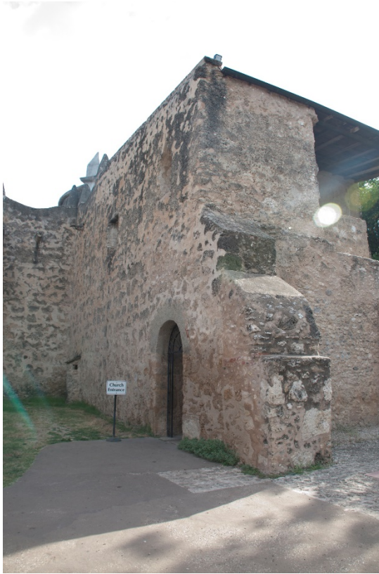
Figure 6.B.224: Exterior southwest corner.
