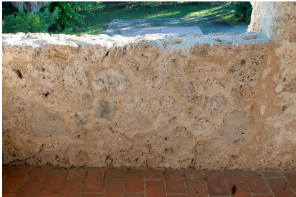
Figure 6.B.166: South wall. Detail of the parapet. A later addition to the historic construction, the parapet has no plaster and only features some missing parts.
