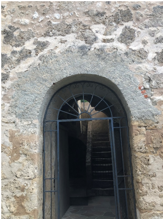
Figure 6.B.226: Exterior west wall. Arched door of entrance to the staircase. Cement mortar finishing was applied over the bricks composing the arch.
