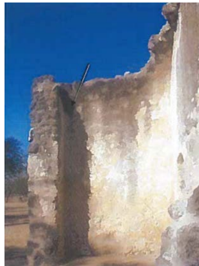
Figure 6.A.81: a) Emergency edge stabilization. Area is indicated by the arrow. Reprinted from Documentation of South & East Exterior Walls... , by Restoration Associates Limited, 2009, p. 4.
