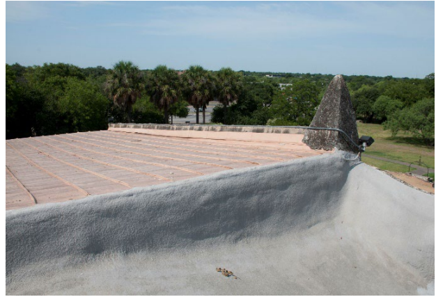
Figure 6.B.229: View of the roof of the Father President's office.
