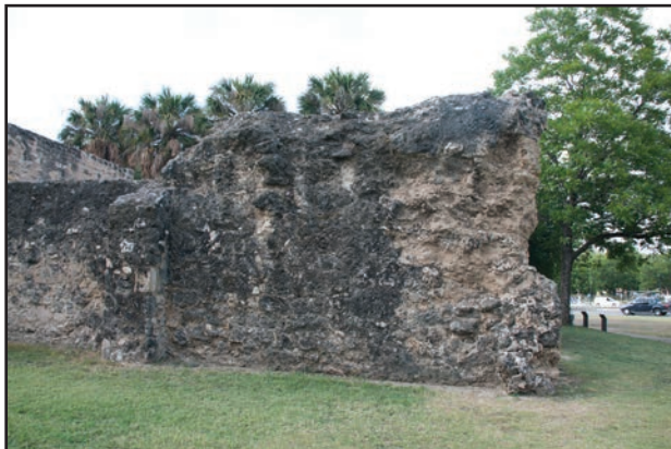
Figure 5.14: North façade wall.
