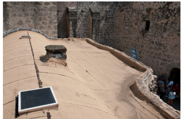
Figure 6.B.234: Roof of the convento. Photo facing north showing the roof of the portería, the storeroom and the guest room.
