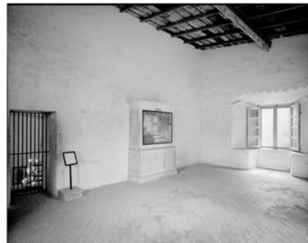
Figure 4.50: View from Father President's office (103 A) looking east. 1933 photograph (HABS, Library of Congress)
