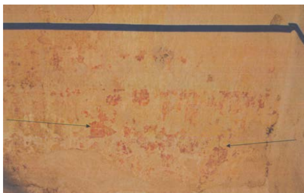
Figure 6.A.74: East wall—36" wainscot with evidence of red pigment, indicated by the arrows. Reprinted from Exposing Historic Wall Plasters... , by Restoration Associates Limited, 2008, p. 12.
