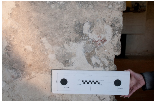
Figure 6.B.23: 104 A—East wall (B6), left jamb of the door that goes to the storeroom, remnants of painted plaster.
