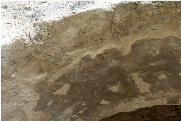
Figures 6.B.182, 6.B.183: Exterior west elevation. North arch of the west arcade. Remnants of painted plaster with edge stabilization from the conservation campaign of 1988. Detachment of edges of the painted finish.
