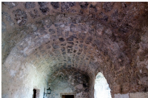
Figure 6.B.16: 104 A—Vault looking south. The vault features regularly laid coursed blocks and modern mortar joints.
