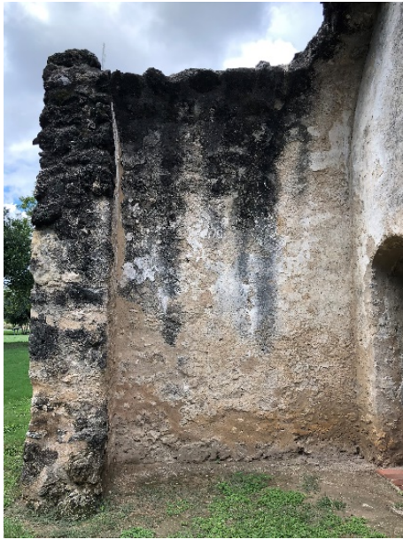
Figure 6.B.206: East wall (segment C), corresponding to the refectory. Features remnant plaster and a thick patina of biological origin.
