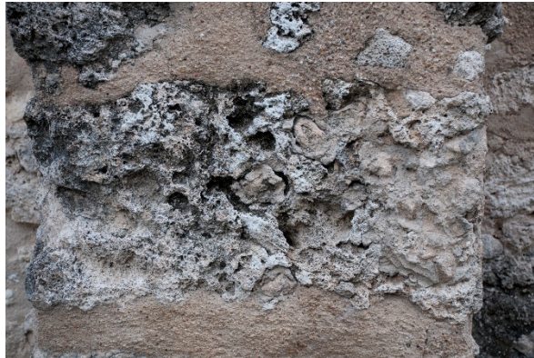
Figure 6.B.1: Detail of a sedimentary 'tufa' block. Tufa stone is characterized by an oversize porosity. The masonry was repointed with a brownish restoration mortar.
