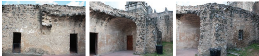
Figures 5.3 5.5: Images of east exterior walls.
