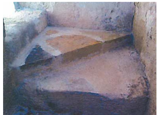
Figure 6.A.90: Removal of a pre-existing wooden ramp and replacement of a stone ramp matching the existing floor. Reprinted from Documentation of South & East Exterior Walls... , by Restoration Associates Limited, 2009, p. 9.
