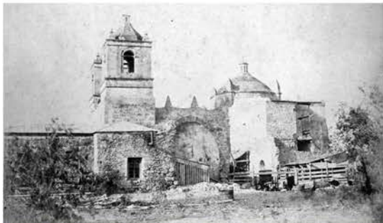
Figure 4.28: Picture shows the south wall of the convento, including the southeast corner of the staircase that collapsed in 1850s. Photograph date unknown (National Park Service Archive)
