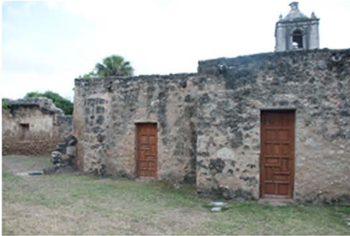
Figure 4.16: Photograph of the south walls of the refectory and kitchen (UTSA CCS)
