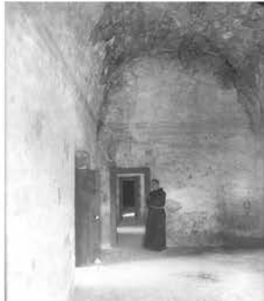
Figure 4.37: Picture inside the Library (104 E) looking north. The tie rod hasn't been added yet. 1919 photograph (San Antonio Conservation Society)
