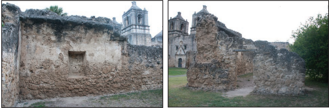
Figures 5.12, 5.13: Former interior north wall (photo at left) and west wall of ruins.
