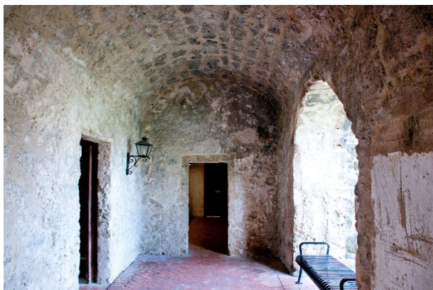
Figure 6.B.6: 104 A—View toward southern entry into the corridor. Note the south wall covered by various layers of historic plaster and finishes.
