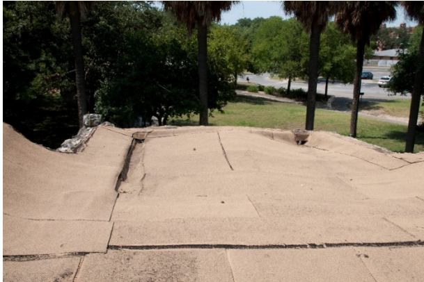
Figure 6.B.237: Roof of the convento. Photo facing south, showing the roof of the refectory.
