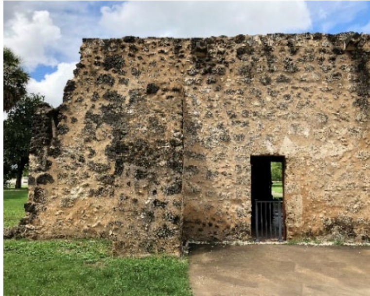
Figure 6.B.207: East wall (segment B), corresponding to the library. This façade is in fairly good condition.
