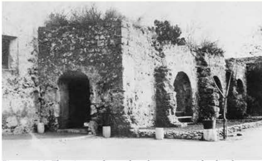
Figure 4.35: The picture shows that the west corridor has been reopened and the decay of the buttresses of the west wall. 1917 photograph (Institute of Texan Cultures)
