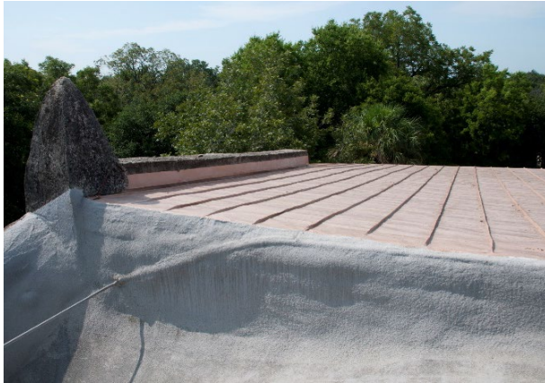
Figure 6.B.228: View of the roof of the Father President's office. The overall condition is good.
