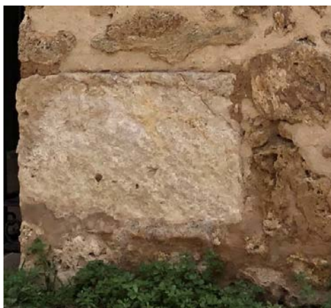
Fig. 6.B.3: Ashlar stone block made of a whitish fine-grained, compact limestone, also called Austin limestone.
