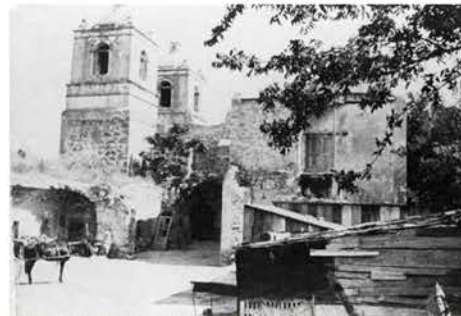
Figure 4.29: Picture shows the south wall of the staircase, indicating the buttresses currently in place haven't been built yet. 1895–1905 photograph (SMU Library)
