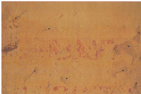
Figure 6.A.72: East wall. Sequence (from top to bottom) of a red pigment 2" band with incised lines, a 2" band with an ochre wall color, followed by a red pigment wainscot. Arrows indicate historic plaster losses. Reprinted from Exposing Historic Wall Plasters... , by Restoration Associates Limited, 2008, p. 11.
