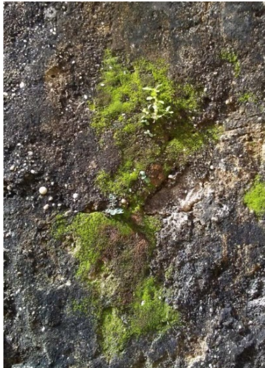
Figure 6.B.219: A dark-colored, thick layer of algae and moss completely covers the top part of the northmost buttress.
