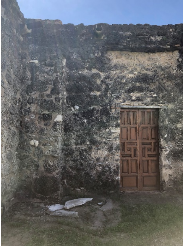
Figures 6.B.193, 6.B.194, 6.B.195: Northern wall covered in thick layer of algae, plants, and moss. The wall surface also features high level of stone erosion, fragmentation, and delamination.
