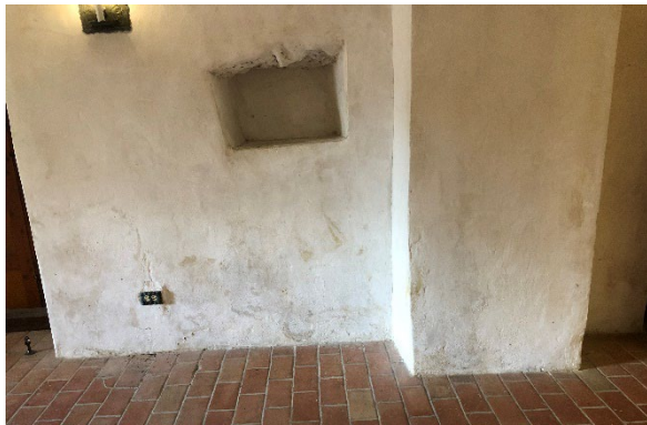
Figure 6.B.110: Room 104 F Kitchen—North wall. Stains due to moisture, likely the result of both rising damp and water ingress from the door during rain season.
