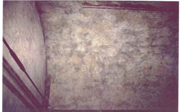
Figure 6.A.49: Library vaulted ceiling—example of aesthetic integration/mitigation. In the final integration treatment, the dark stones were tinted not to stand out from the surface, but to blend with the plaster, August 1988. Reprinted from 1988 Conservation Project Completion Report... , by Anthony Crosby, 1997, p. 60.
