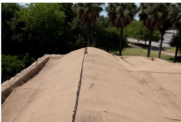
Figure 6.B.235: Roof of the convento. Photo facing south, showing the roof of the library.
