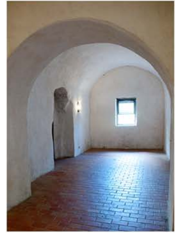
Figure 4.17: Photograph, the arch between the refectory and the kitchen has been opened (UTSA CCS)
