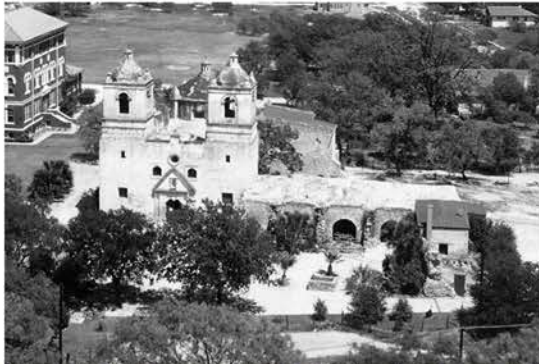
Figure 4.39: Aerial photo looking at the building from the west. 1920 photograph (San Antonio Conservation Society)
