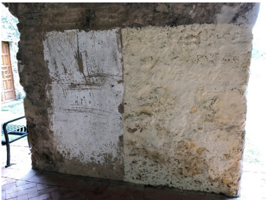
Figure 6.B.30: 104 A—West wall (A5, A6, A7, B5, B6, B7). Modern concrete patch and wash (left) and shelter coats of three layers (right). There are also natural hydraulic lime-based patchings (upper right corner of the image) which are compatible with the masonry but visually intrusive.
