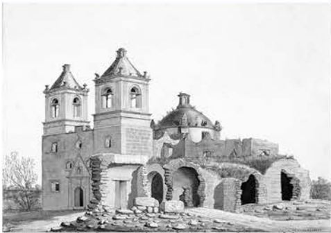
Figure 4.18: The drawing shows how several areas of the convento have collapsed. Drawing by Edward Everett, ca. 1846 (Amon Carter Museum)
