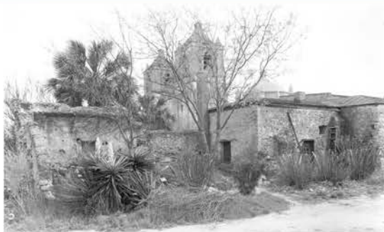
Figure 4.59: View of the southwest part. Photo indicates the western buttress of the kitchen's south wall was lower than the current one. 1945-50 photograph (National Park Service Archive)
