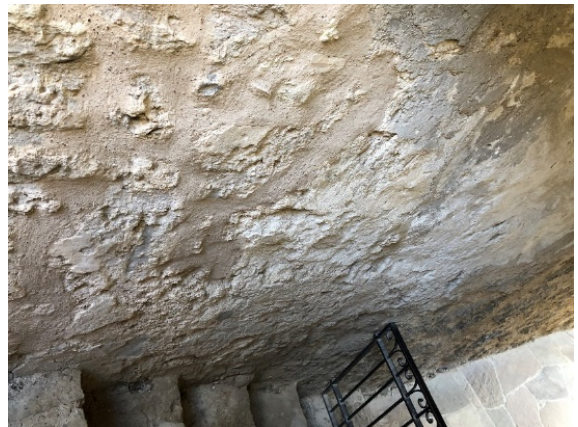
Figure 6.B.170: South wall of the staircase. Brown mortar patching restoration is in generally good condition.
