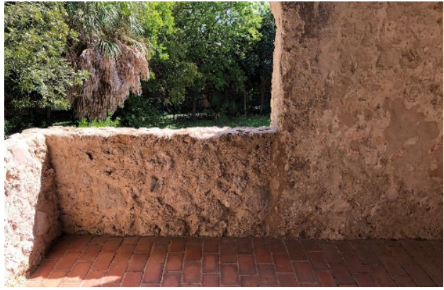
Figure 6.B.165: South wall. Left part. Shows the connection of the historic part of the wall (right), with the later addition of the parapet (left).
