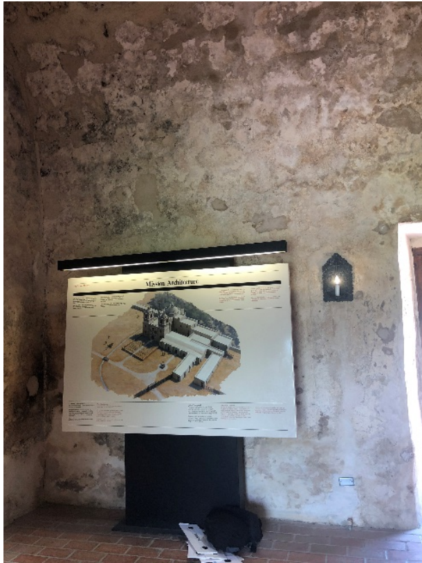
Figure 6.B.61: 104 D Portería—East wall, partially covered by the information banners.
