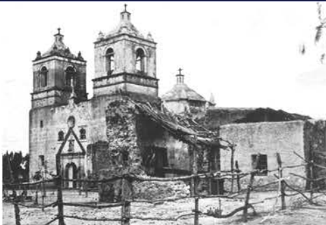
Figure 4.22: Picture indicates the west end of the south wing has been closed. Photograph by Ernst Wilhem Raba, 1868 (Raba Collection, San Antonio Conservation Society)
