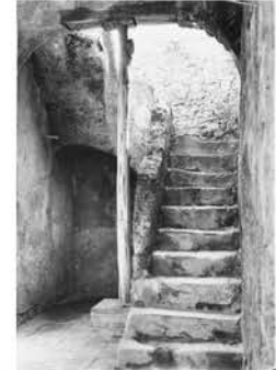
Figures 4.55 and 4.56: View of the staircase looking east. The middle part of the arch has been filled and a timber pillar has been added as structural reinforcement. Date of photographs unknown (Institute of Texan Cultures)
