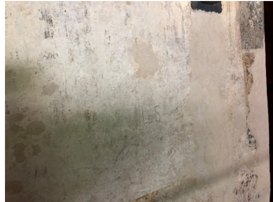
Figure 6.B.98: 104 E Library—West wall (A4, B4). Area on the left of the door. Visually intrusive patching under the modern lamp, historic incisions, and graffiti in the painted finish.
