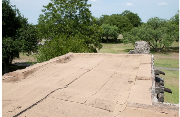
Figure 6.B.238: Roof of the convento. Photo facing west, showing the roof of the kitchen.
