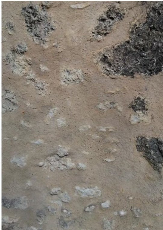
Figure 6.B.209: Brown mortar patching applied on the small tufa rubble.
