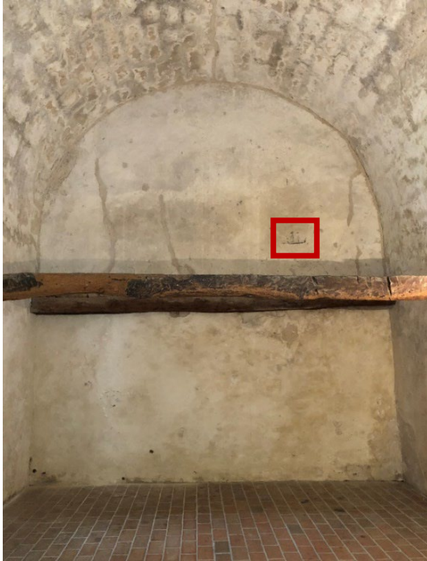
Figure 6.B.34: 104 B—North wall general view. The whole wall was replastered probably in the 1930s. It features a nice graffiti (located in the red box placed on the photo by the HSR team) representing a boat.
