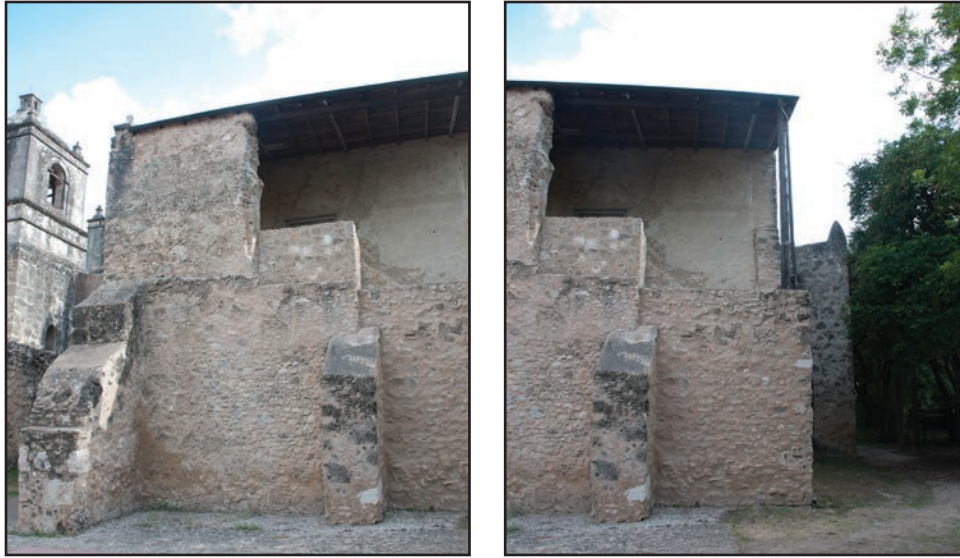
Figures 5.30, 5.31: Exterior south wall of the Father President's office.
