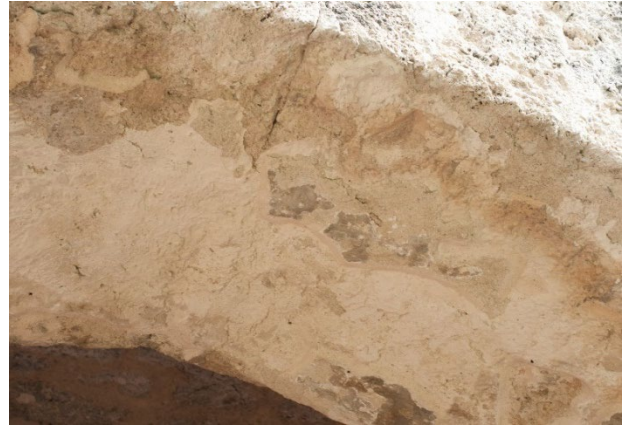
Figures 6.B.186, 6.B.187: Exterior west elevation. Middle arch of the west arcade. Remnants of painted plaster with edge stabilization from the conservation campaign of 1988.
