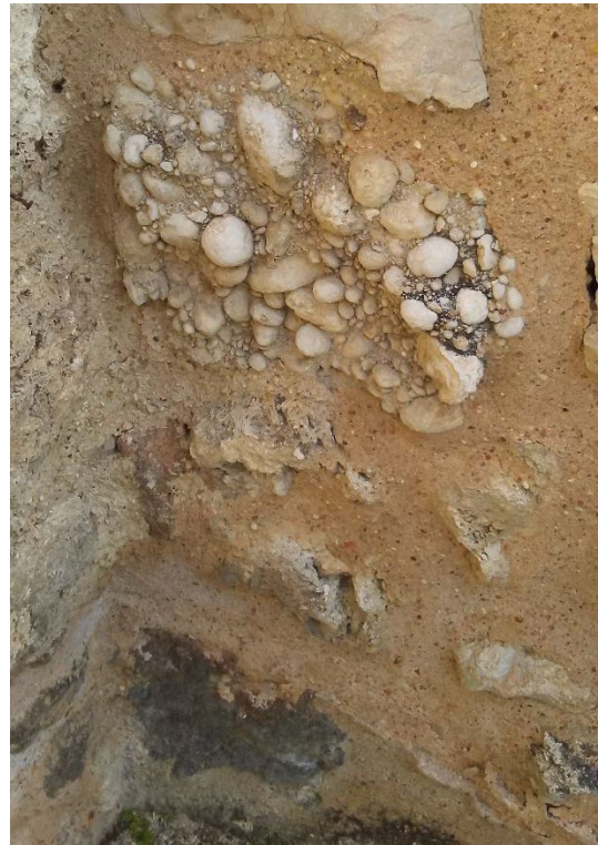
Figure 6.B.210: More pisolithic rubble, with its typical differential erosion.
