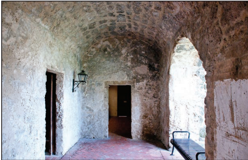
Figures 5.15, 5.16: The corridor looking north (top photo) and south.
