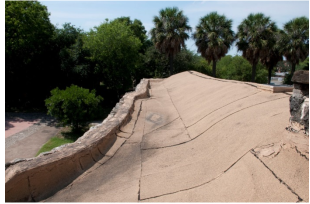
Figure 6.B.232: Roof of the convento. View of the east part of the convento's roof, showing the increased parapet. Photo facing south.
