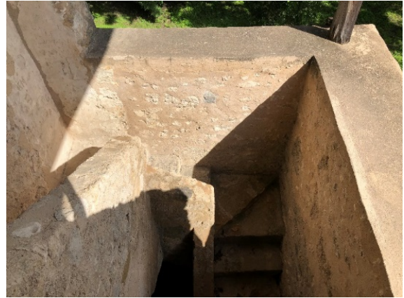
Figure 6.B.169: East wall of the staircase features brown mortar patching, in generally good condition.
