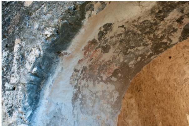
Figure 6.B.21: 104 A—Arch in the north wall of the corridor detail, remnants of painted plaster (red and yellow). The red and yellow faux voussoir colors are partially covered by a gray paint.
