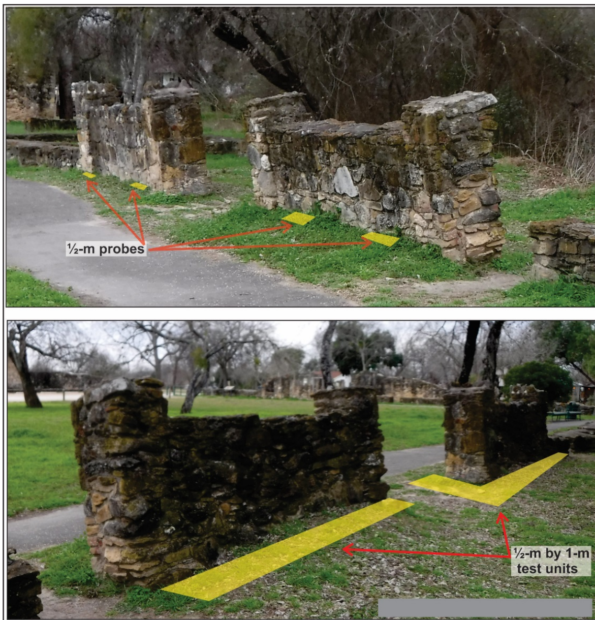
Figures 4.1 and 4.2: North gate showing the approximate location of probes and test units.
