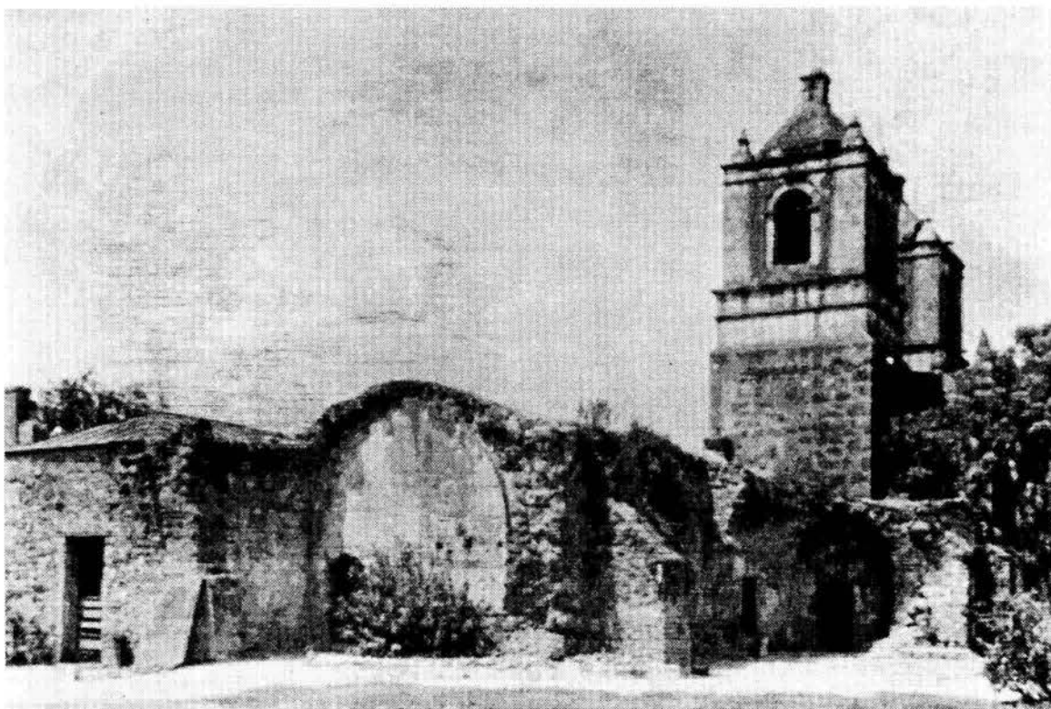
Figure 19. This photograph of Mission Concepción's south elevation, taken circa 1910 by C.O. Lee, indicates the state of the convento ruins and vegetation at the time.
