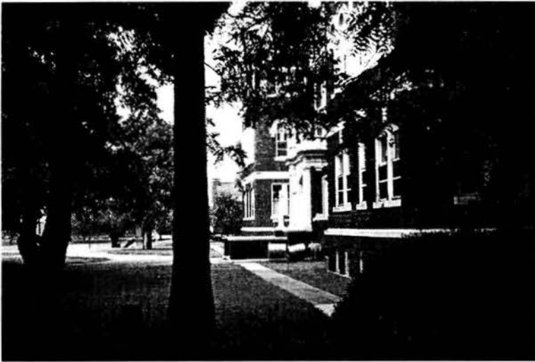
Figure 52. The front (west) facade of the main building at former St. John's Seminary, looking north.
