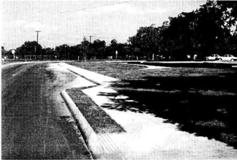
Figure 54. View northwest along Mission Road showing bus parking and accessibility ramp.
