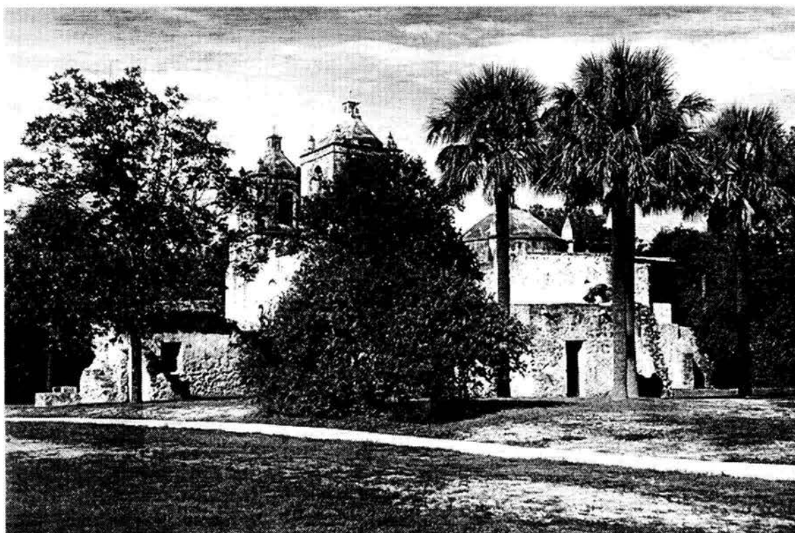
Figure 97d. These four photographs of Mission Concepción all include the church, convento, and sacristy. Some landscape features that were present in the late 1800s, have been removed or replaced over time: the wood fencing has been removed, the hard-packed earth has been replaced with concrete walks, and the newly planted shade trees have been replaced with palms.
