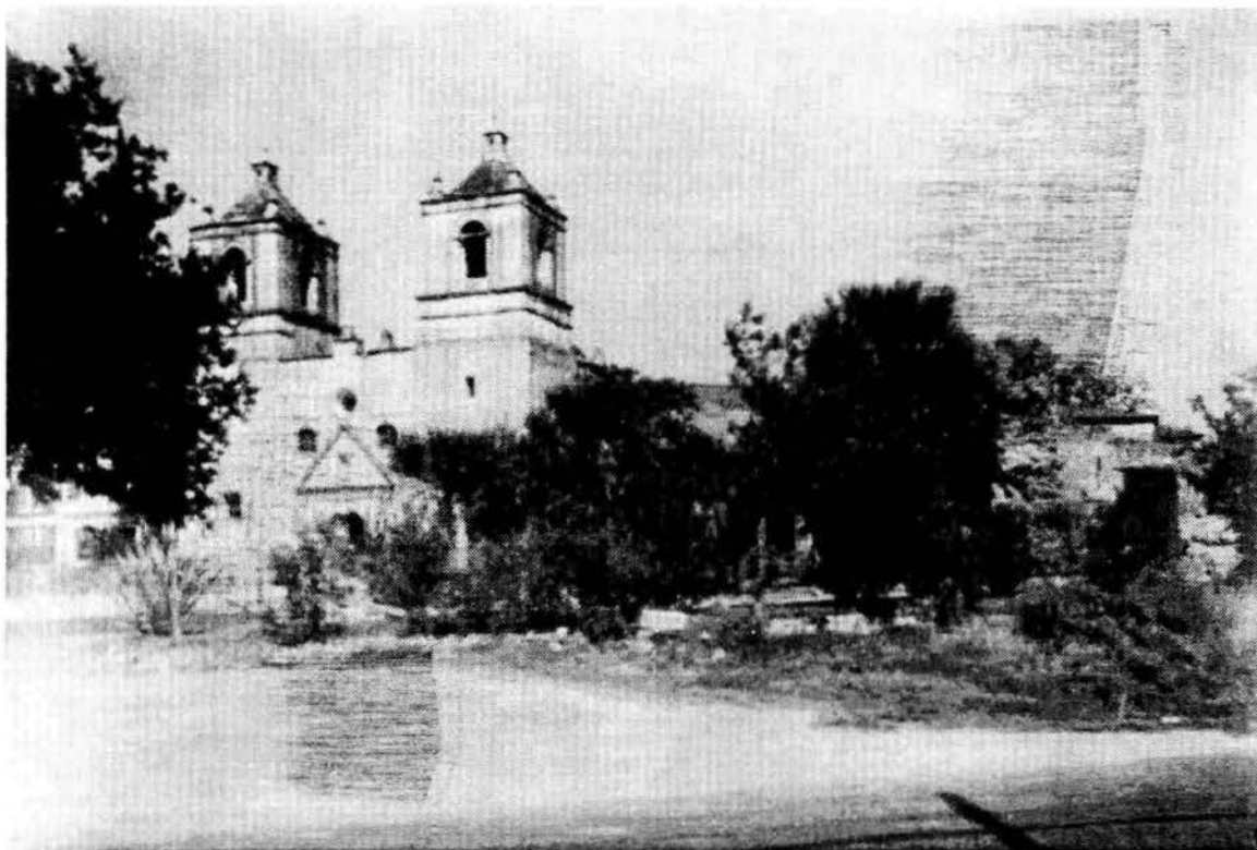
Figure 35. The area southwest of the church appears to be heavily vegetated in this 1936 HABS photograph.
