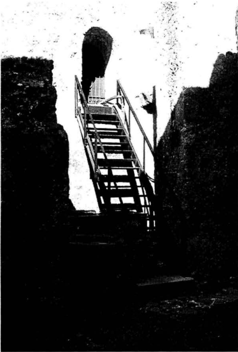
Figure 87. A flight of steel stairs leads from the northwest corner of the courtyard to the second floor of the church's south tower; air-conditioning equipment is clustered at its base.
