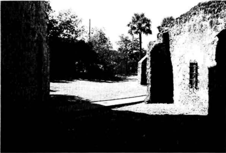
Figure 78. The courtyard is drained by an earthen, grass-lined swale; the plywood walkway that traverses the courtyard is structured to permit through-drainage.
