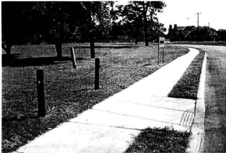
Figure 63. The public sidewalk along Mission Road includes accessibility ramps with rumble strips.
