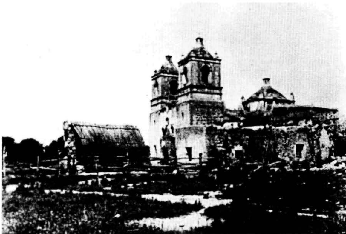
Figure 6. A circa 1870 photograph of the south side of the mission compound illustrates the stabilization efforts of the Brothers of Mary, which concentrated on the Father President's office (note the tin roof) and the other rooms directly next to the church.
