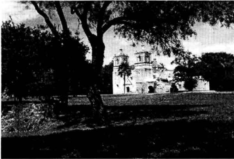
Figure 92. View of mission complex from the quarry looking northeast.
