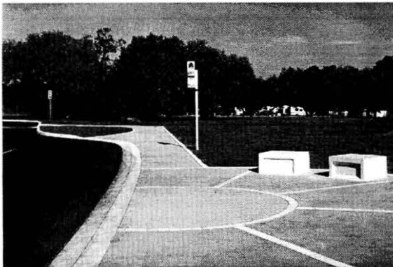
Figure 62. Feature strips of white stone pavers accentuate the concrete paving at the bus stop and visitor arrival area.
