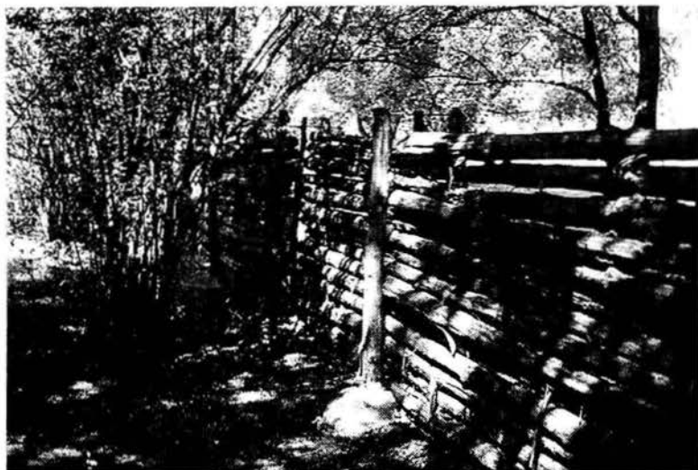
Figure 84. Wood fencing of staggered, peeled-log panels defines the mission boundary north and east of the church.
