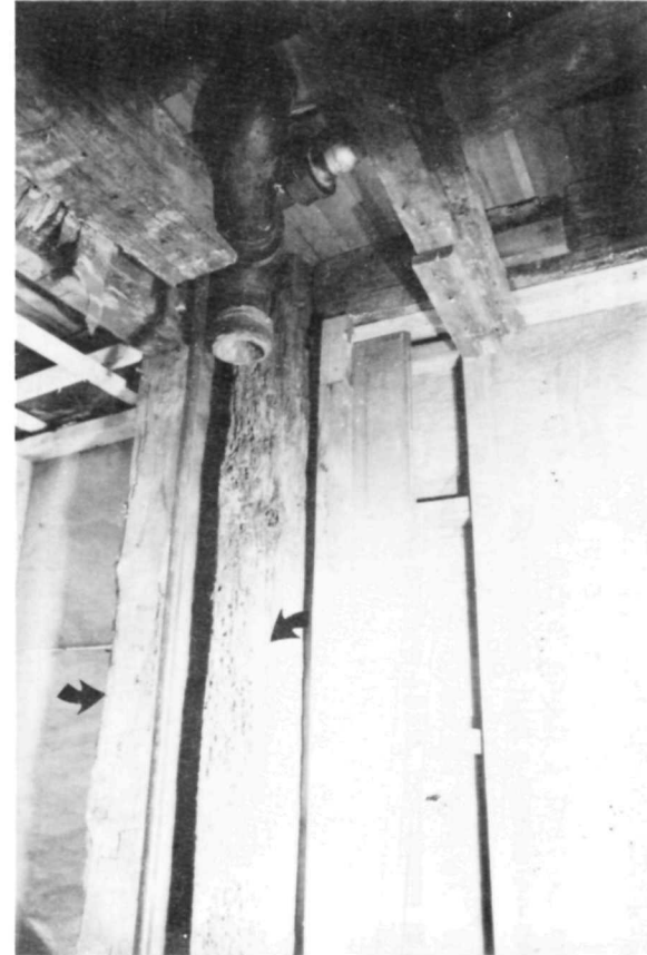
Illustration 35. Antram-Gray House: West-Wall Framing of First Story, Showing Adjacent Circa-1730 and Circa-1798 Corner Posts and End Girts.
