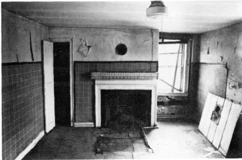
Illustration 63. Antram-Gray House: Room 202, Looking South.
