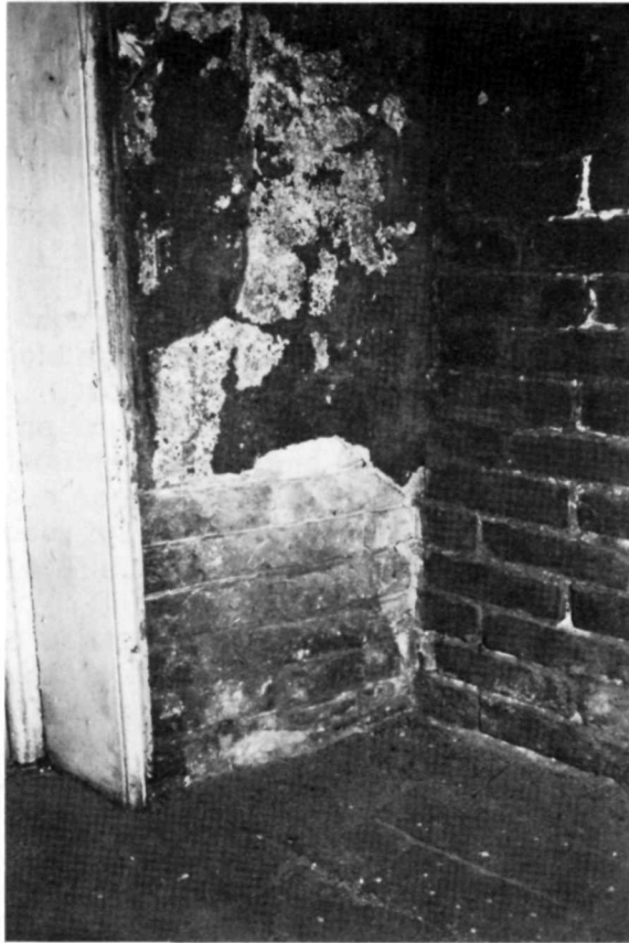
Illustration 44. Antram-Gray House: Fireplace in Room 202, East Side of Firebox, Showing Natural-Cement Pargeting.
