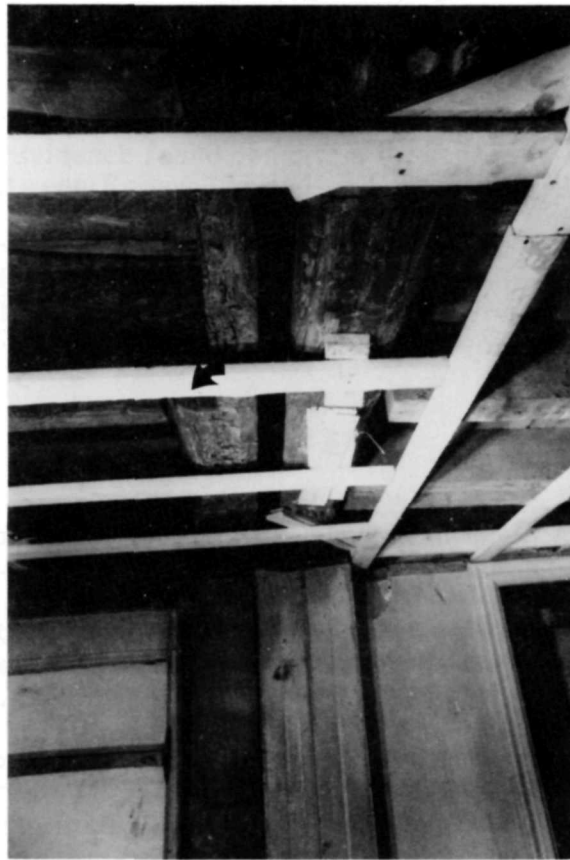
Illustration 48. Antram-Gray House: First-Floor Framing, Showing Circa-1730 South Girt Cut Out for Southeast Stair.
