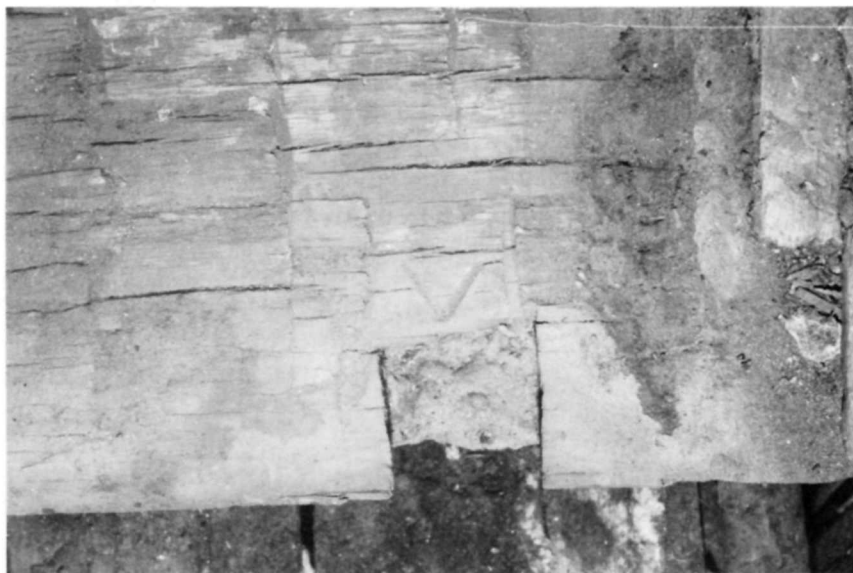
Illustration 49. Antram-Gray House: Framing Evidence of Southward Shift of Northwest Stair.
