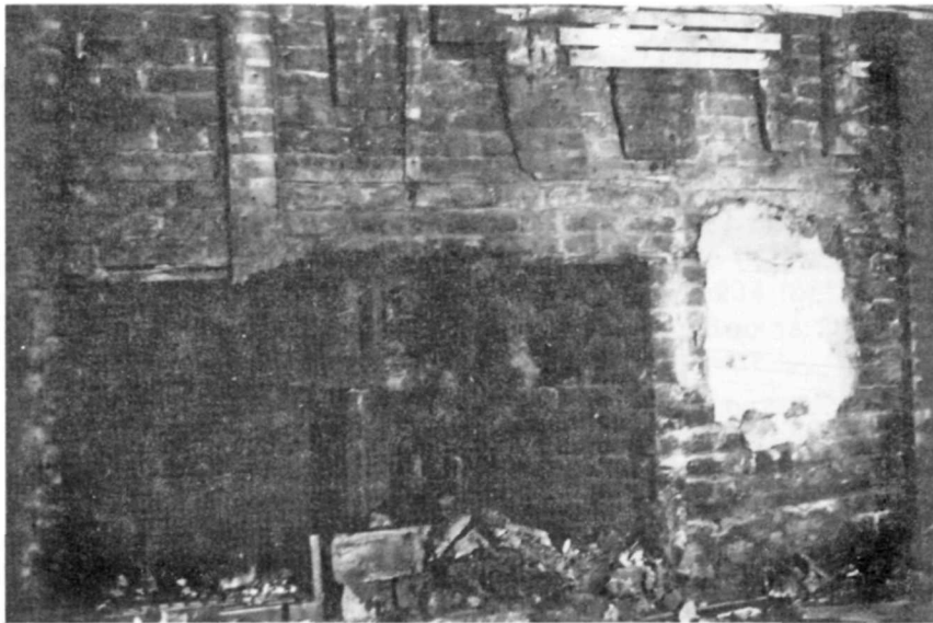
Illustration 52. Antram-Gray House: Uncovered First-Story Fireplace at North End of West Wall (Formerly in Room 204).
