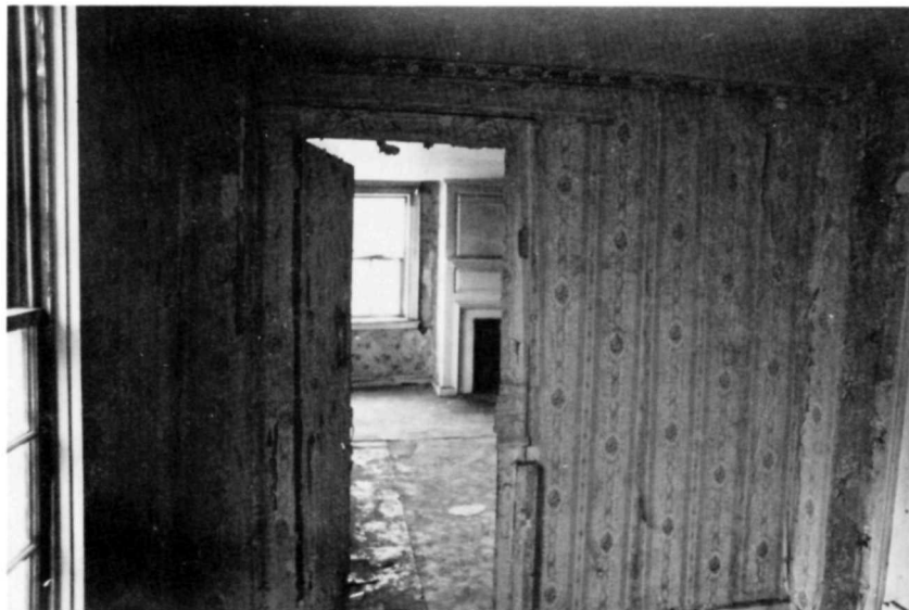
Illustration 66. Antram-Gray House: Room 205, Looking South.
