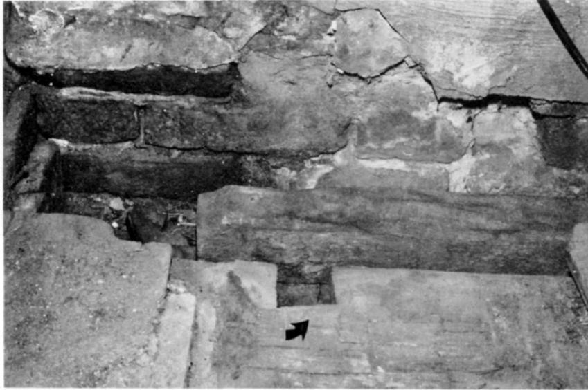
Illustration 24. Antram-Gray House: Raising Numerals on Attic-Floor Framing Members.
