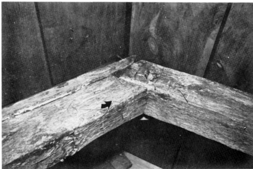
Illustration 25. Antram-Gray House: Raising Numerals on Roof Rafters.
