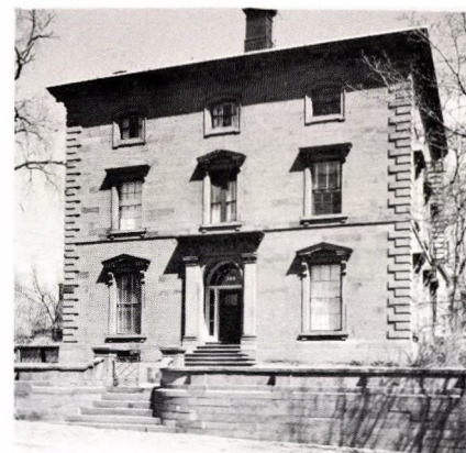
Tully Bowen House. HABS.
