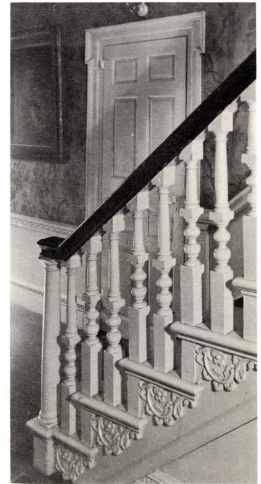
Seril Dodge House, 1787, stairs.
