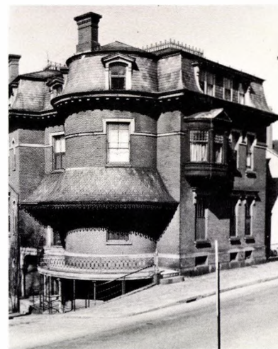
General Ambrose Burnside House HABS
