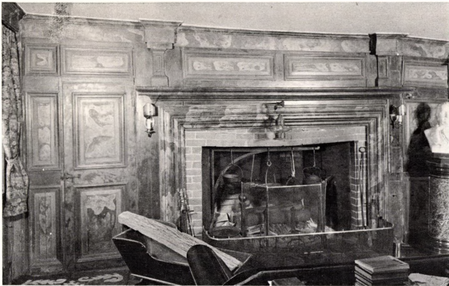
Reynolds House, Bristol, 1700, showing bolection paneling and marbled wall decoration.
