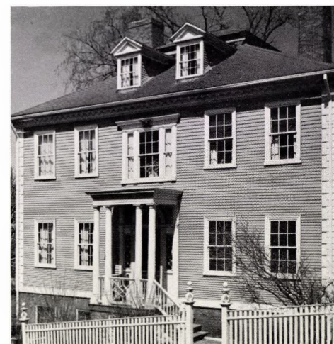
Richmond House, 36 Bowen St., Hip roof. HABS.
