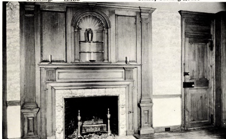
Parlor, Cushing House, showing over mantel shell cupboard. HABS.
