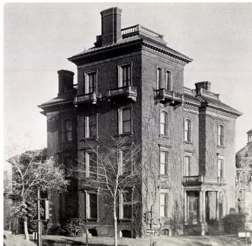
George Corliss House, HABS
