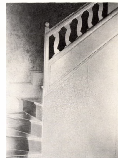
Samuel Gorton house, 1680, stairs.
