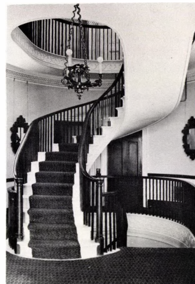
Ives House, spiral staircase.
