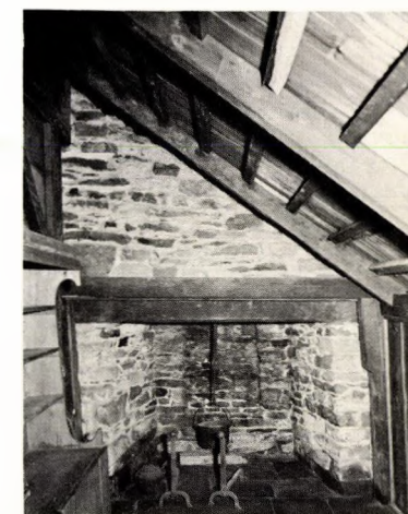
Attic story, Clemence House, showing braced framing, rafters and purlins. HABS.
