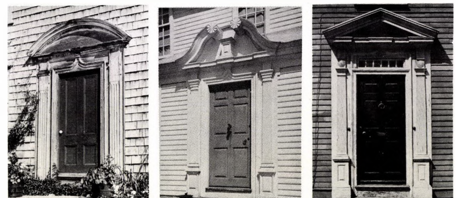
Bowler House, Portsmouth, Segmental pediment. Dr. Babcock House, Westerly - Broken scroll - pediment high base. Cushing House, Providence - triangular pediment.
