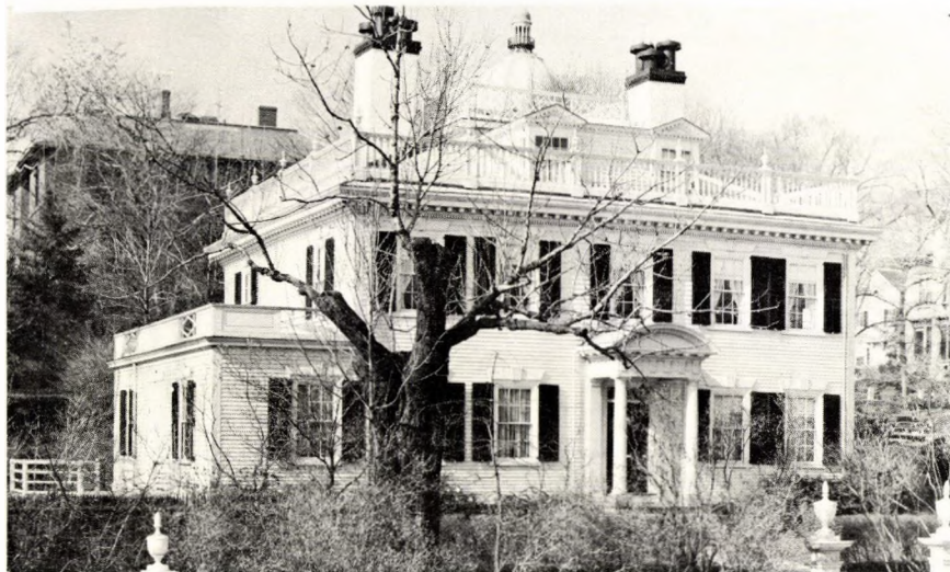
Captain George Benson House, 1796. HABS.
