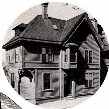
House at 336 Benefit St., HABS.
