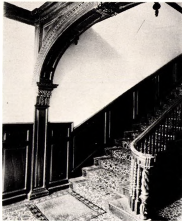
Stairs, Cheeseborough House, c. 1740, Newport, showing twisted balusters and hall arch.
