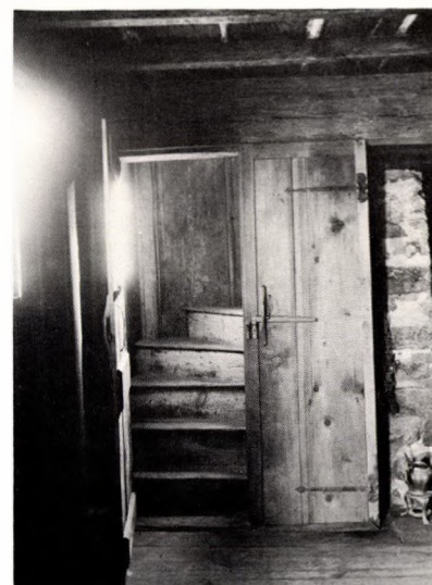
Clemence House, stairs.
