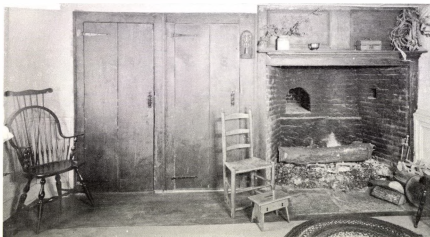
Tripp House, c. 1720, Manton, Interior showing oven on back wall of fireplace.
