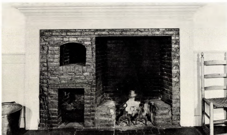
"Shakespear's Head", kitchen fireplace showing oven at side. HABS
