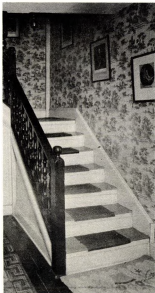
Reynolds House, stairway, showing closed string course.
