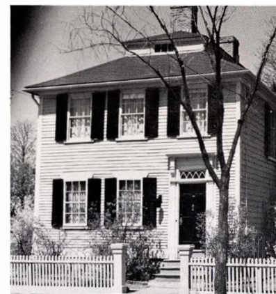
House, 160 Power St., Monitor Roof. HABS.
