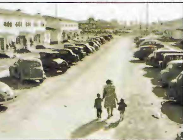
Wartime apartment complex for workers NPS
