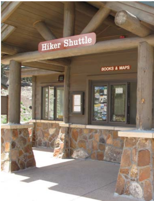
TOP: Subalpine Zone roof uses appropriate Hartford Green color (right); color at left is too light for Subalpine zone.
