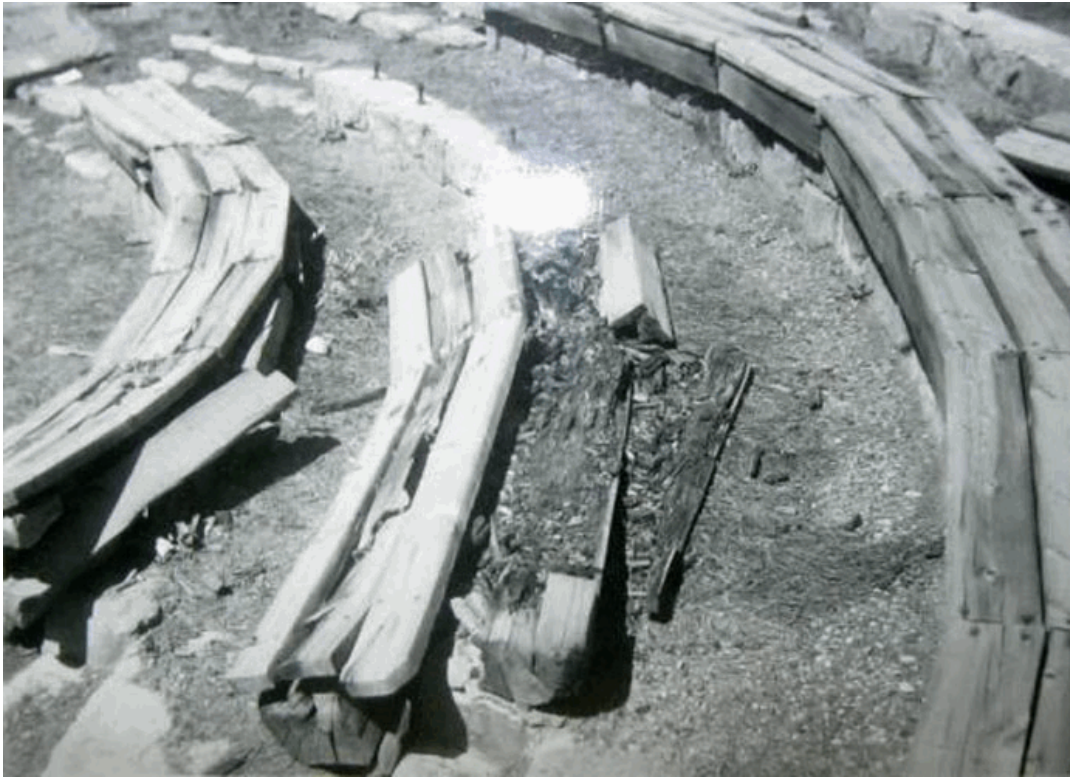
View of the deteriorated wood seats in the amphitheater, 1955. Source: Urgently Needed Construction Projects, ROMO Archives.
