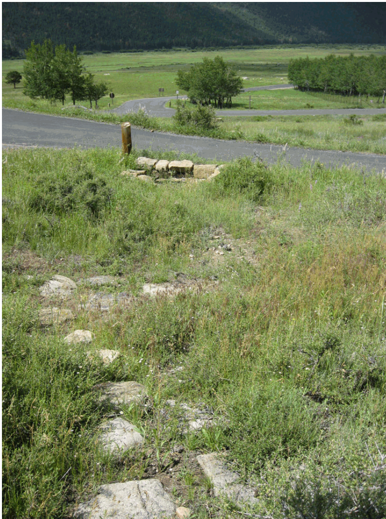
Stone drainage structure along entrance road to Moraine Park Museum and Amphitheater, July 2010. Source: C. Mardorf, NPS.
