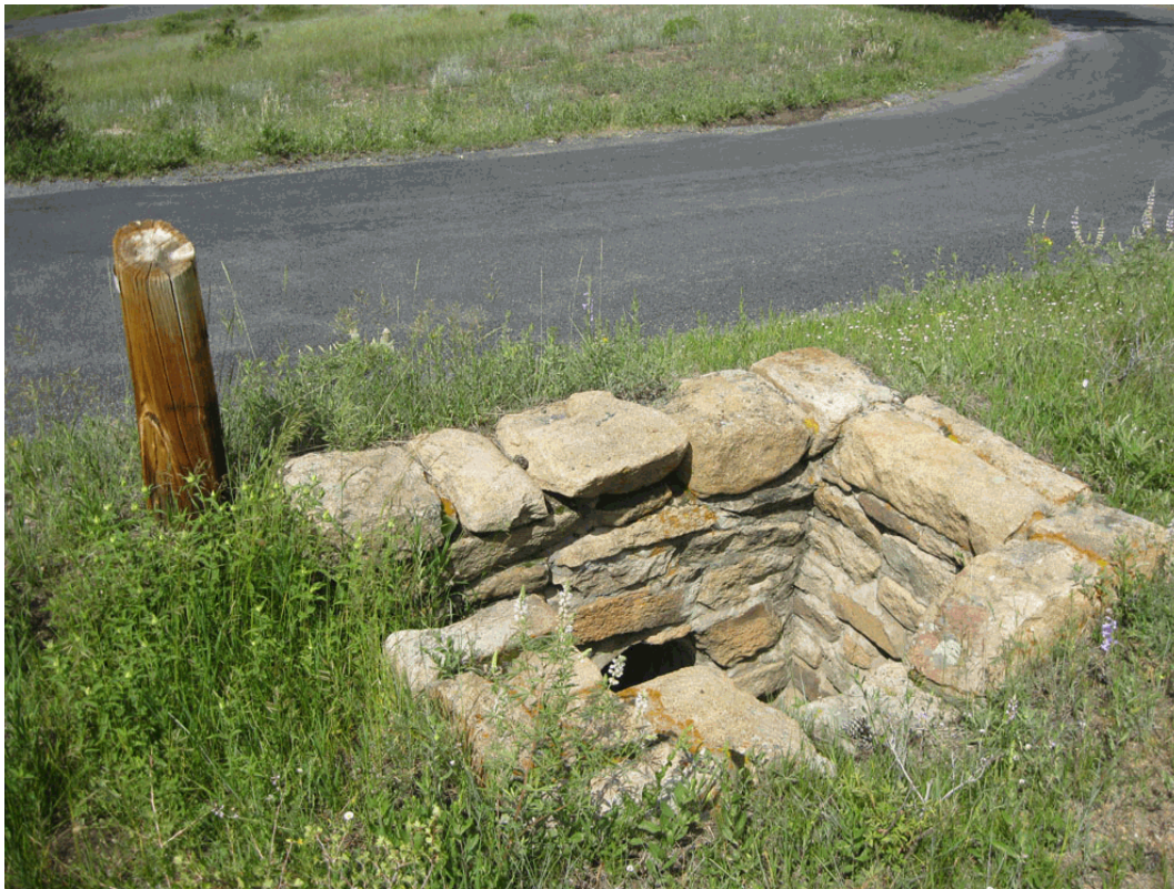
Stone drainage structure along entrance road to Moraine Park Museum and Amphitheater, July 2010. Source: C. Mardorf, NPS.
