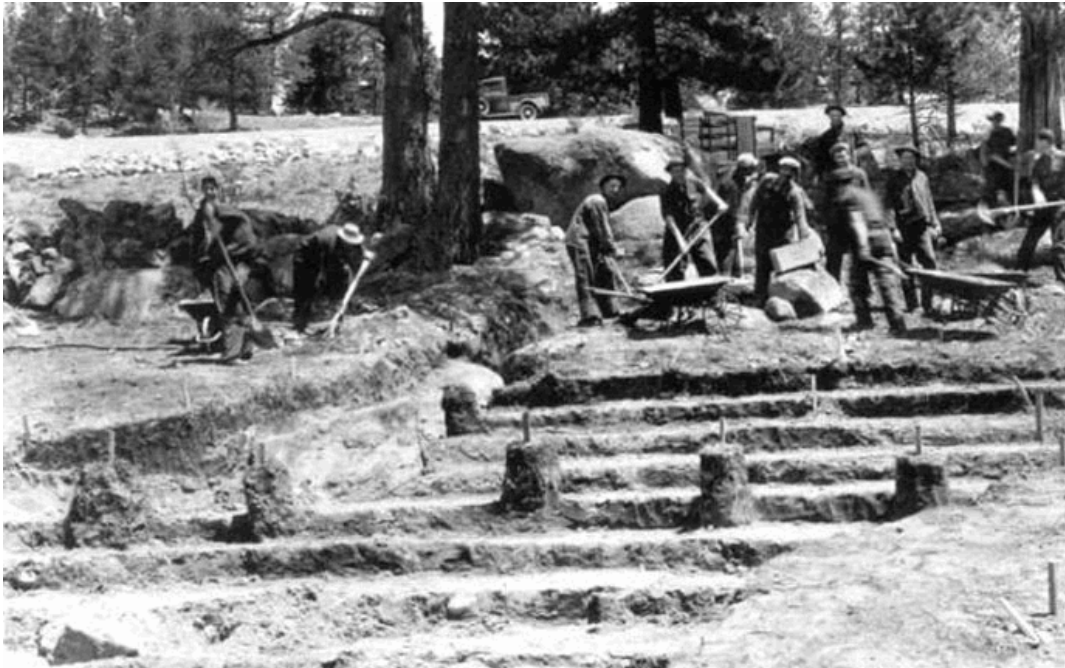
Moraine Park Museum Amphitheater construction, May 29, 1936. Source: NPS-ROMO, 11—5, album 4008, neg 3132; NR nomination.
