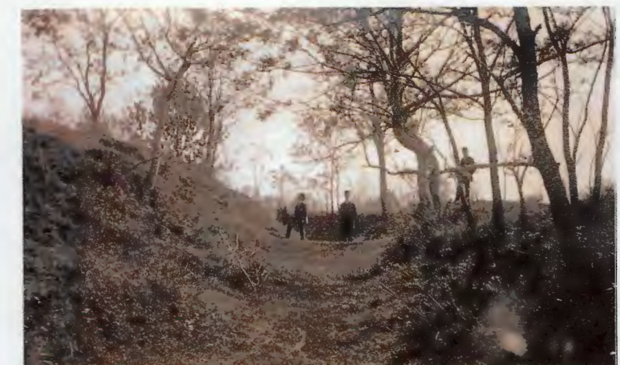
Fort Stevens Parapet, 1900, Courtesy of Ron Harvey, Jr.
