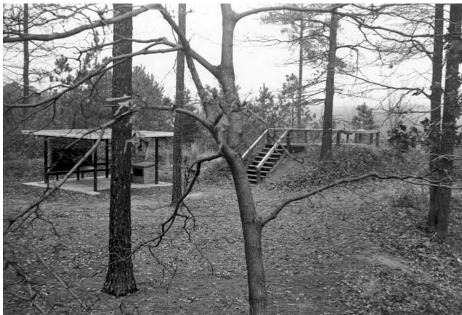
Figure 6. Interpretive shelter and viewing platform in 1976. (HSI 006744, 1976)
