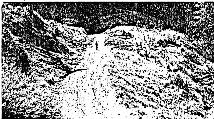
Photos 5 and 6 (August and October, 1978): Before and after views showing outsloping of road and installation of cross road troughs to drain the road cutbanks--note the elimination of the culvert and the inboard ditch in the October photo. C-90 Road, Harry Weir (Emerald) Creek.
