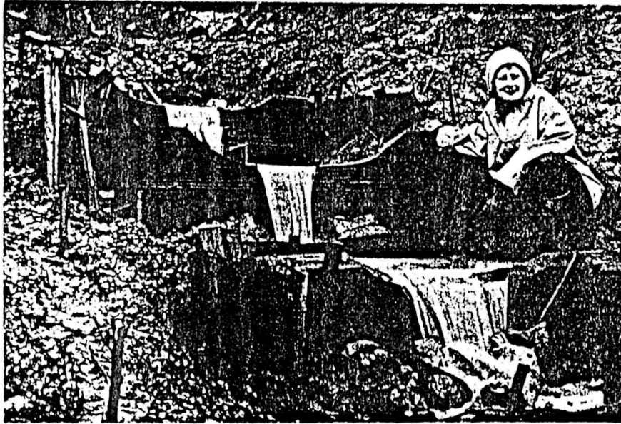
Photo 14 (December, 1978): Recently installed split-board check dams along an intermittent, second-order tributary in Redwood National Park. Each dam is ponding water, and sediment will settle out in the basin up to the height of the spillway. Note the close spacing of check dams, and the rock energy dissipation below the spillways; both measures protect the dams from gully downcutting. Note stem cuttings of willow (poles in gully bank) which are planted to accelerate revegetation. Drainage just below C-10 Road, Miller Creek.
