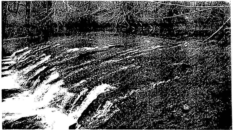
View north, across dam face. Note the north wing wall and deteriorating condition at bottom of dam face.
