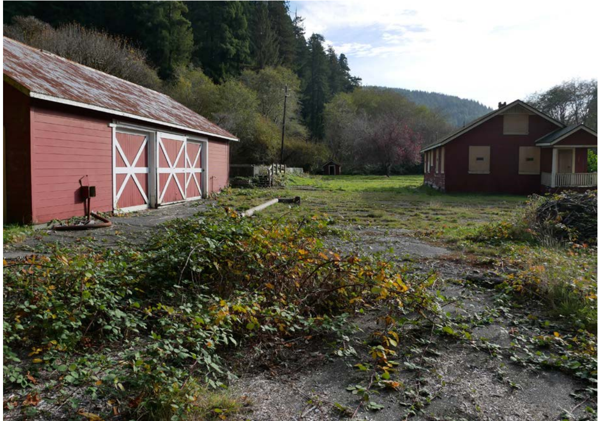
Figure 85 : Asphalt paving, view south, west of Garage-shop, non-contributing (CLRG, 2019)
