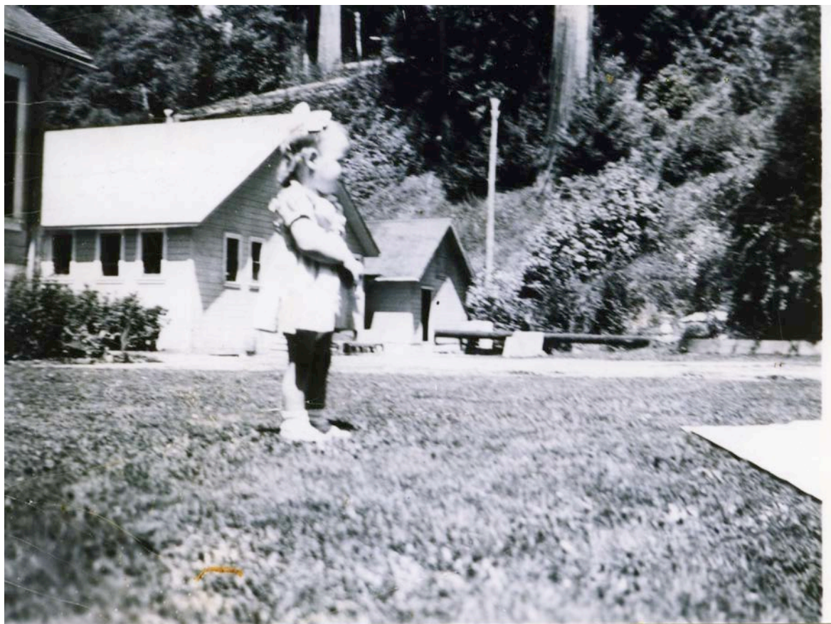
Sliver of Assistant Superintendent House and lawn, with the Hatchery Building and Filter House (Rock Filter) in background (Smedley, 1943).
