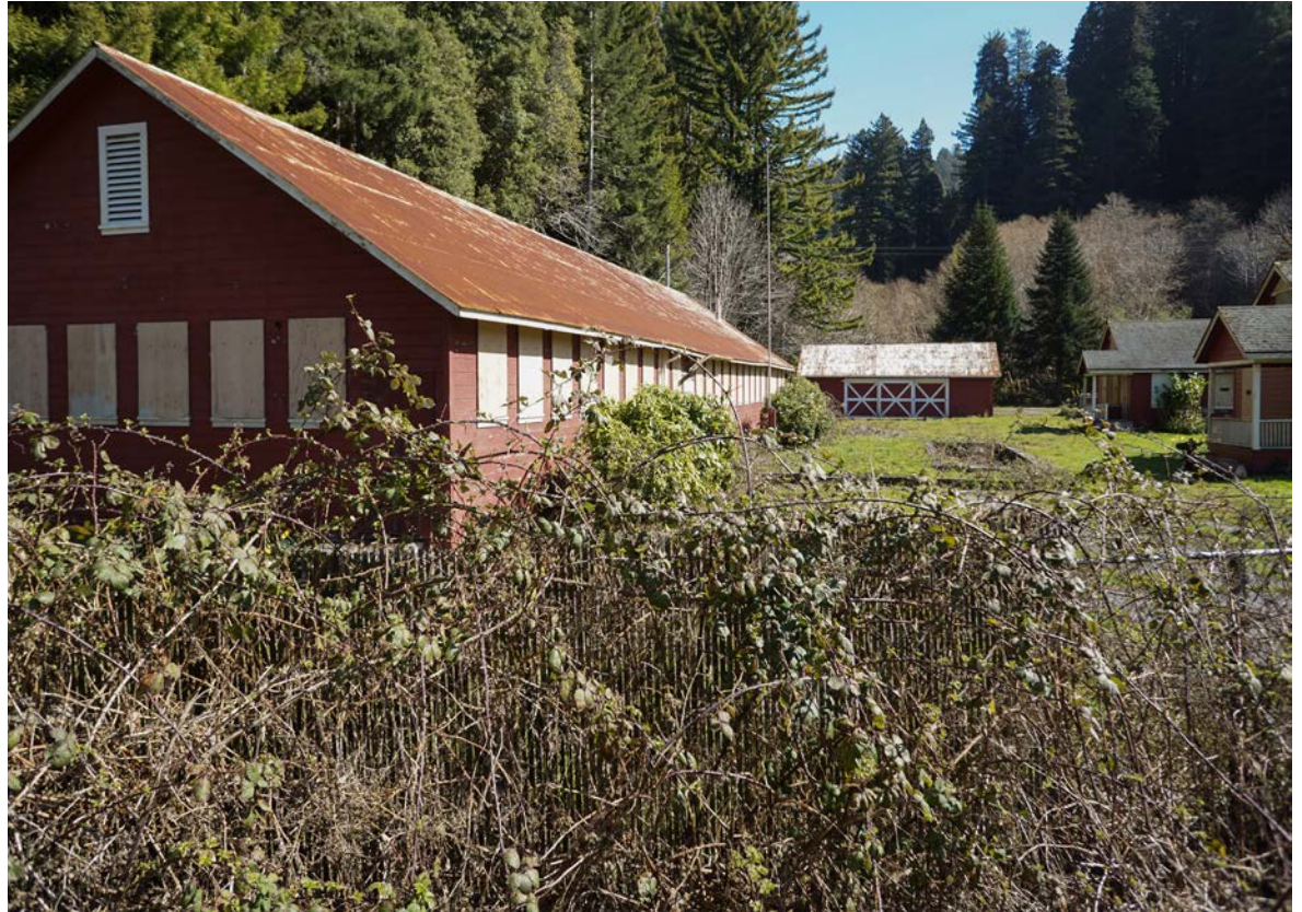
Figure 112 : Northeast view (2020) of existing conditions: Himalayan blackberries grow on chain-link fence in front of original entrance. Central open space, Hatchery Building, Garage, Assistant Superintendent's House and Superintendent's House in background (CLRG, 2020).
