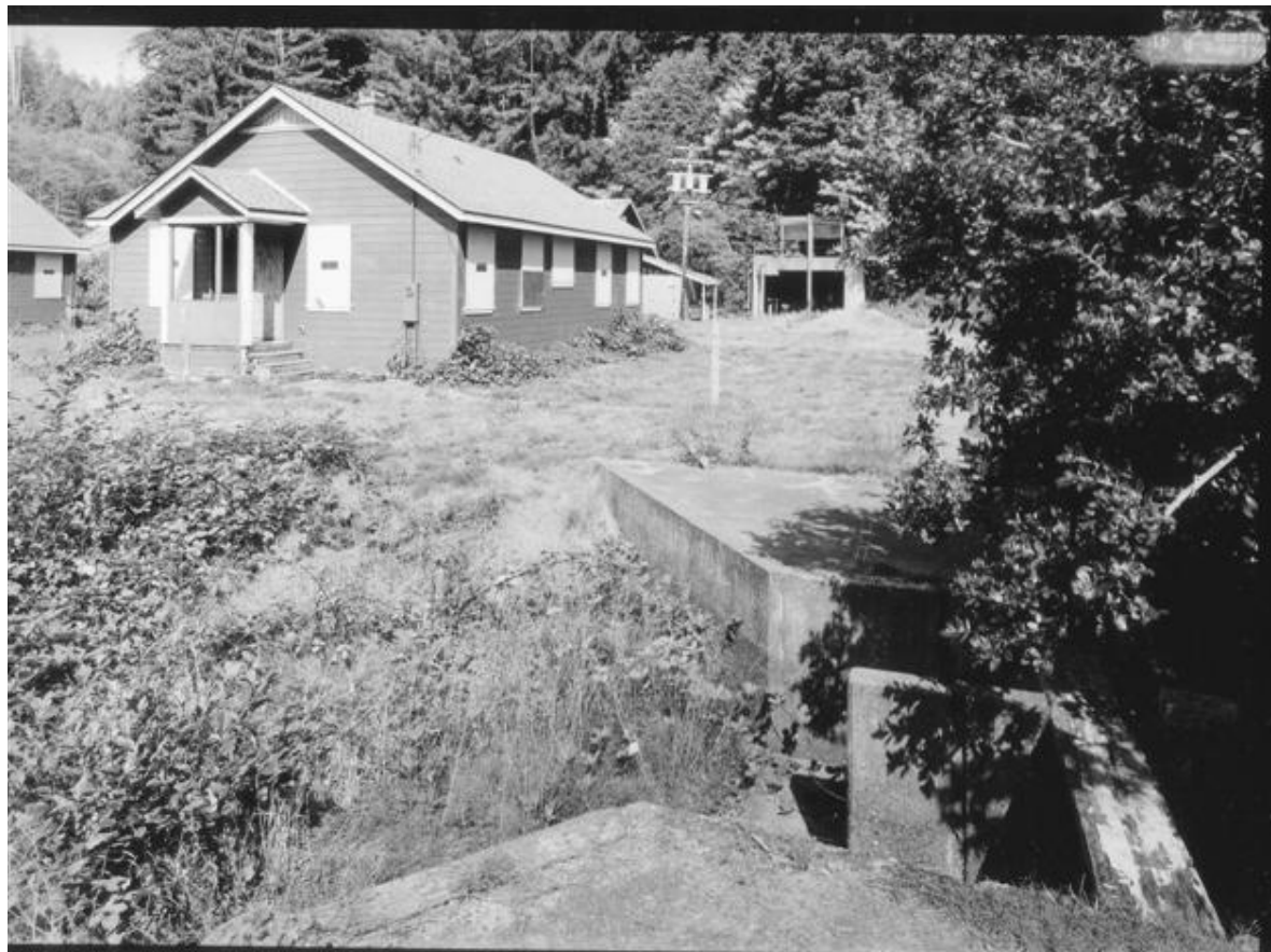
CA-334-19 Superintendent and assistant superintendent's quarters with the tank in the foreground. View to the southeast.
