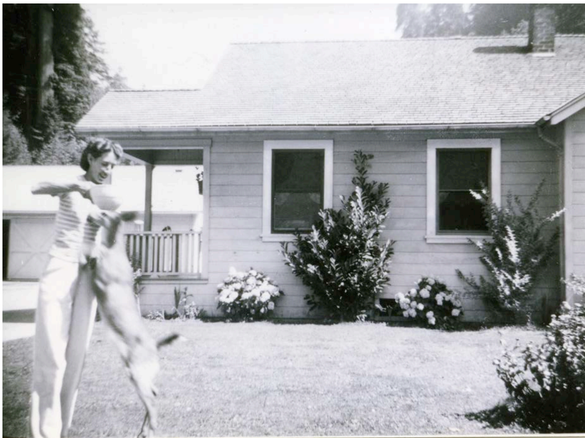
Assistant Superintendent House, with the garage in background (Smedley, 1943).
