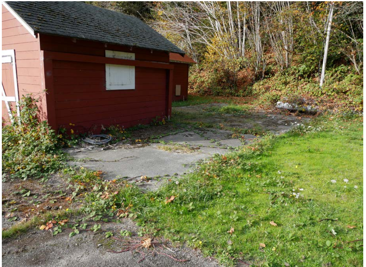
Figure 86 : Concrete paving north of Shed, non-contributing (CLRG, 2019)
