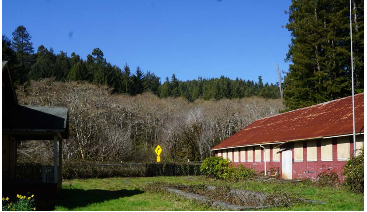
Figure 110 : Northwest view (2020) of existing conditions: Superintendent's House Porch, dedication pond and Hatchery Building (CLRG, 2020).
