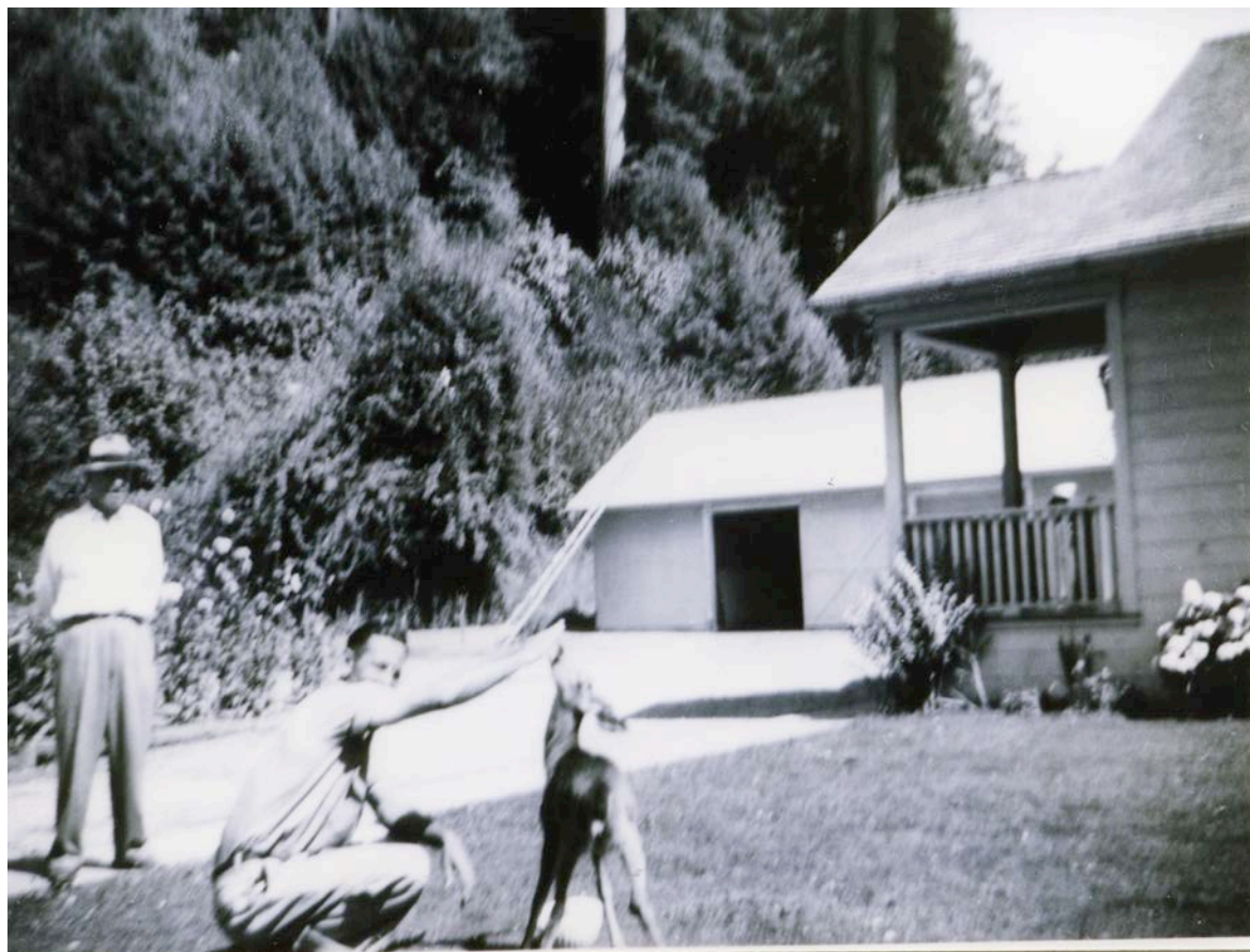
Garage and Assistant Superintendent House Porch (Smedley, 1943)
