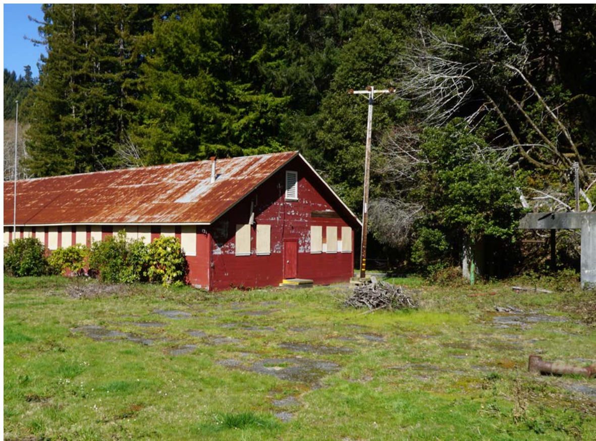
Figure 115 : Northwest view (2020) of existing conditions: Hatchery Building and Aeration Tower (CLRG, 2020).
