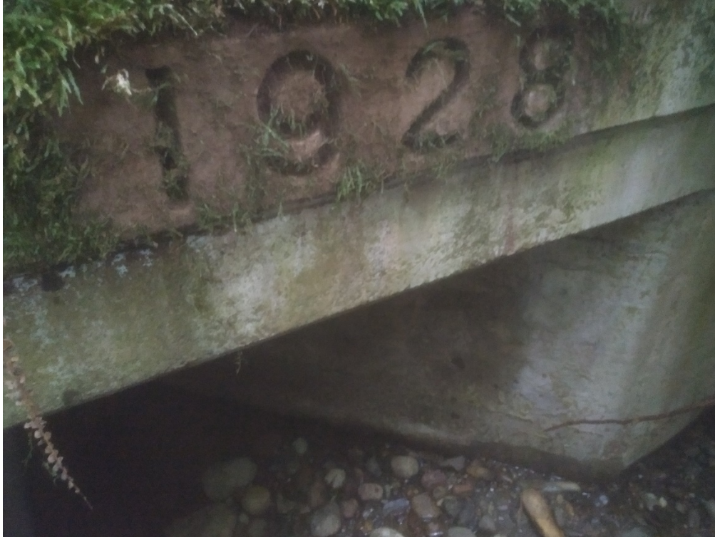
Figure 65. Contributing concrete box culvert below Newton B Drury Parkway with the date of construction embossed on the headwall (NPS 2019).
