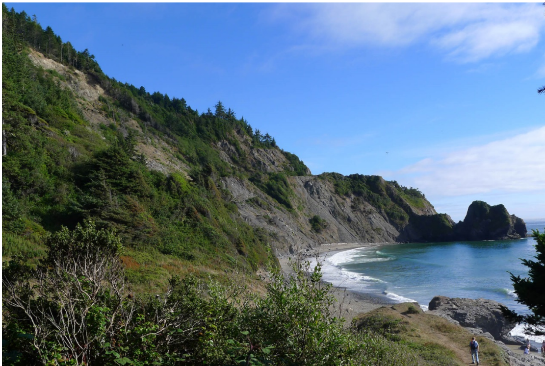
Figure 72. View of Coastal Trail Nickel Creek Section from above Enderts Beach. The abandoned old highway is seen in middle of photo as a terraced area approximately 75 feet above shoreline. One of many rockslides can be seen to the left and covers the abandoned old highway (NPS PWR 2013).
