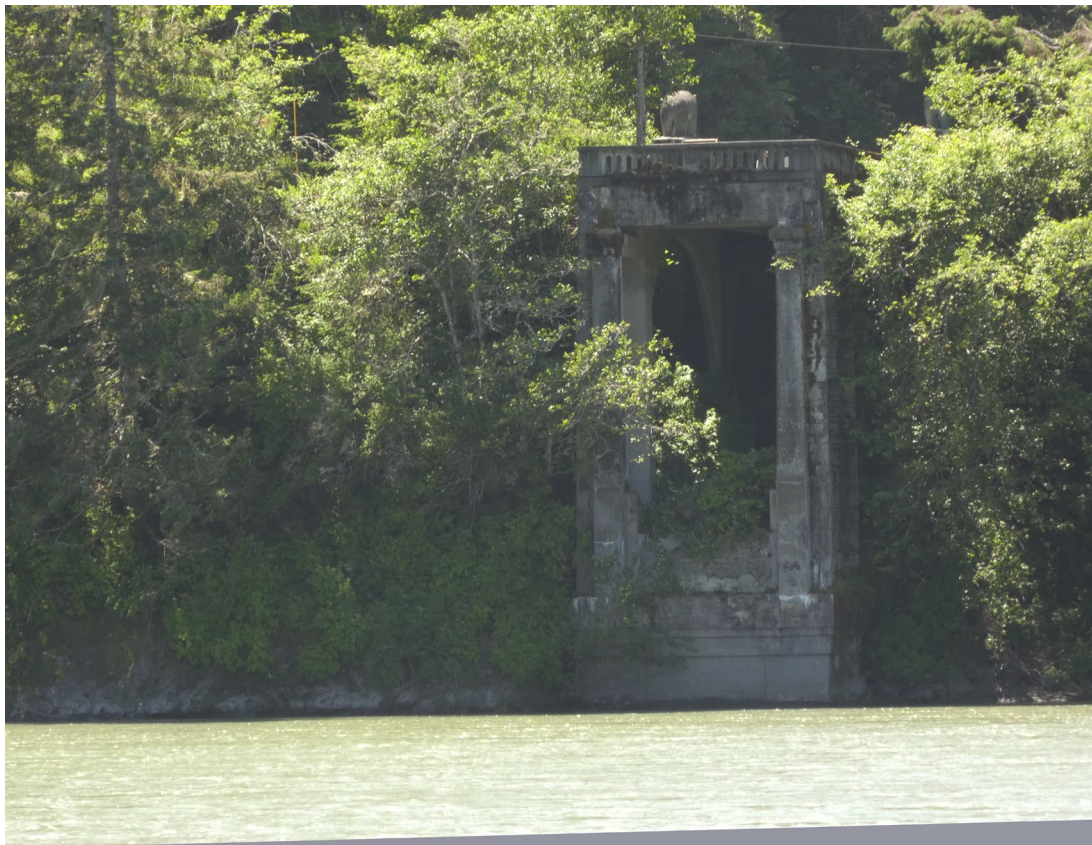
Figure 68. Douglas Memorial Bridge abutment looking south across the Klamath River. (NPS 2018).
