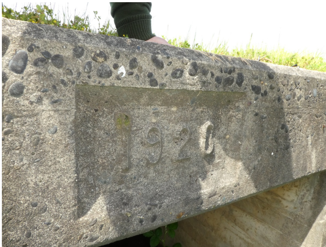
Figure 62. Date stamp on concrete box culvert under Enderts Beach Road (NPS 2017).
