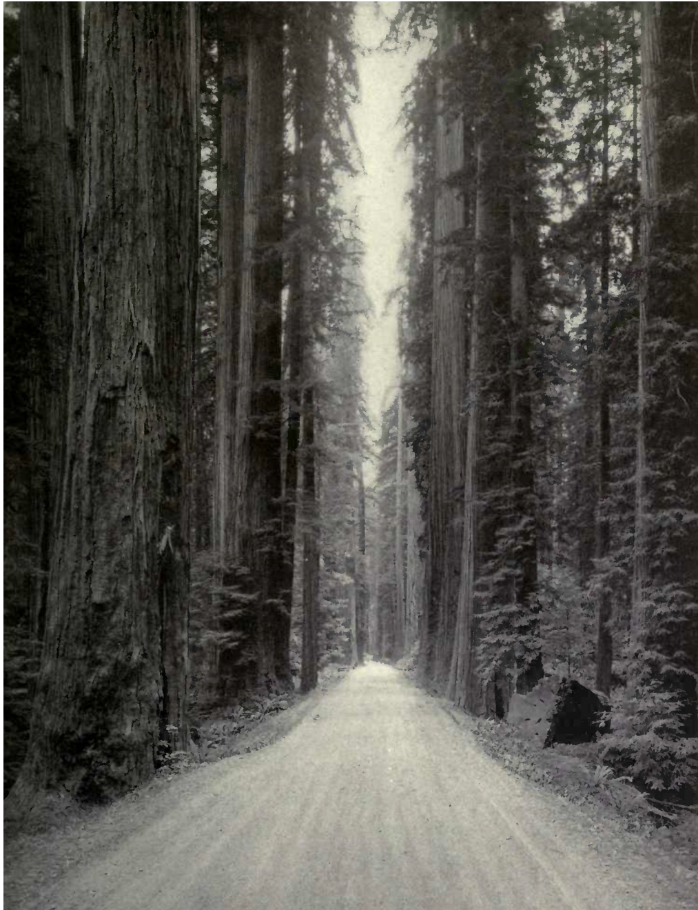
Figure 9. View of the Redwood Highway in 1917 showing quality and character of the road in its earliest phase of development. The road has been graded to approximately 16 to 21 feet wide and has been surfaced with macadam. Note the absence of shoulders, bringing the road margins right up to the surrounding trees allowed highway engineers to avoid falling more trees than was necessary, but it also increased the drama for motorists by emphasizing the great size of the redwoods pressing so close upon the highway. This section of the Redwood Highway is in Humboldt County south of the study area, probably on Bull Flat near the south fork of the Eel River. [Illustration from Madison Grant, "Saving the Redwoods: An Account of the Movement During 1919 to Preserve the Redwoods of California," [New York] Zoological Society Bulletin 22, no. 5 (1919): 117; photograph by the Freeman Art Co., Arcata, Calif.]
