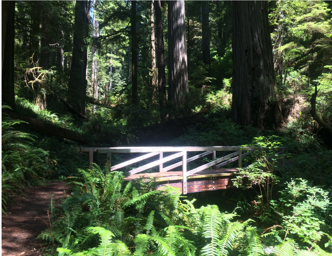
Figure 69. Current footbridge across Damnation Creek in Del Norte Coast Redwoods State Park (NPS 2017).
