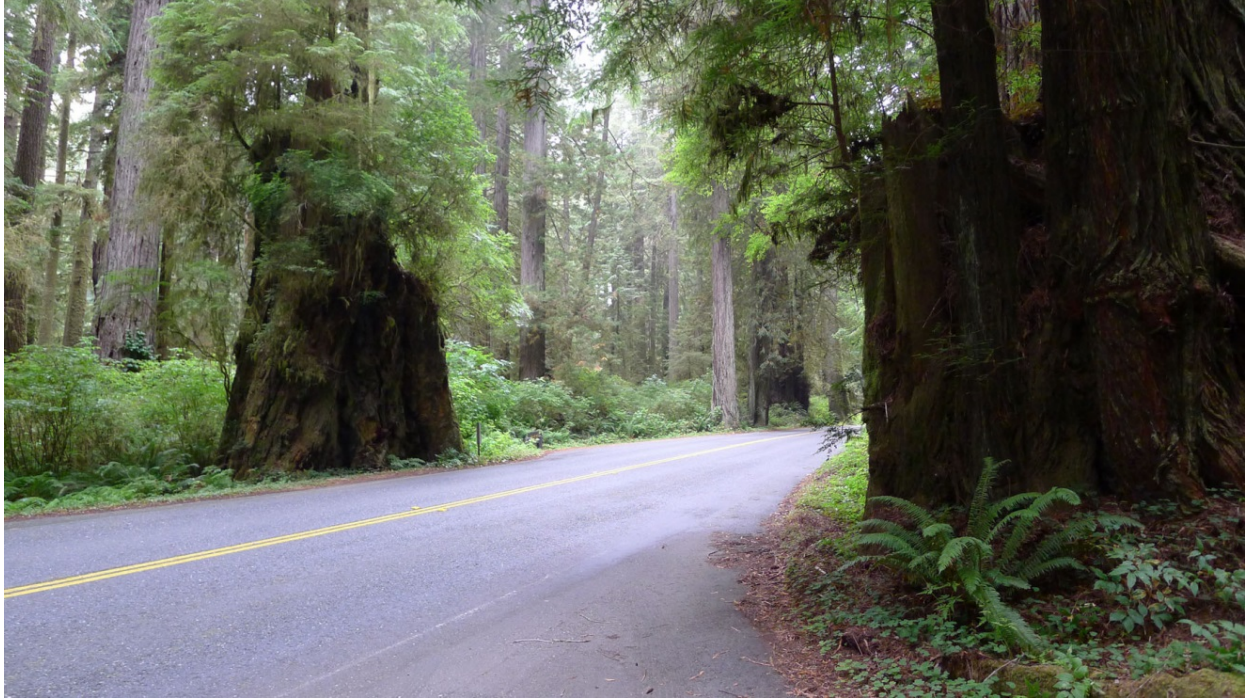
Figure 58. Newton B Drury Parkway, U.S. Highway 101 until 1992 with paved turnout in the foreground (PWR Cultural Resources 2013).
