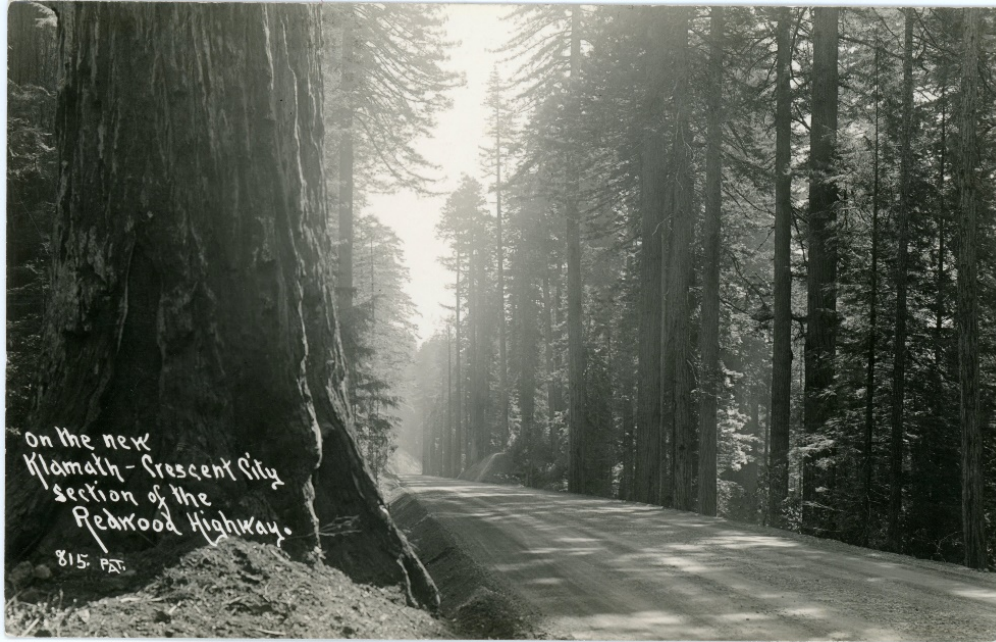
Figure 22. View in Del Norte Coast Redwoods State Park along a portion of the 1934 Redwood Highway realignment. The highway has been constructed to a similar standard as the 1928 improvements in Prairie Creek Redwoods State Park, with a grade width of approximately 30 feet and a macadam surface (See Image #12). [Humboldt State University Library, Special Collections, Tim McKay Coll., 2007.02.2060.]
