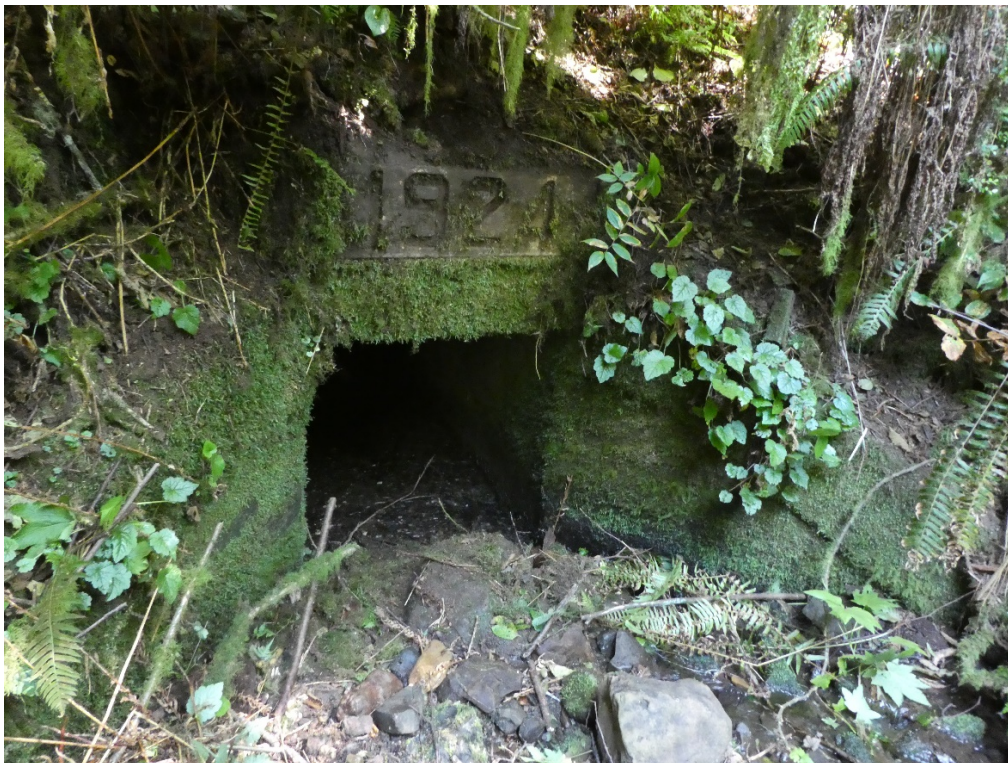
Figure 64. Contributing concrete box type culvert below Alder Camp Road with angled wing walls and the date of construction embossed on the headwall (NPS 2017).
