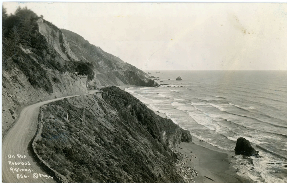
Figure 10. View of coastal section of Old Redwood Highway looking south from a point just south of Cushing Creek. Photograph dates from the mid-to-late 1920s. The road has been graded to approximately 16 feet in width and surfaced with macadam. This section of the road would change very little over the subsequent decades, the most significant modification being the application of an asphalt surface. (Compare Image #13.) [Humboldt State University Library, Special Collections, Tim McKay Coll., 2007.02.2083.]
