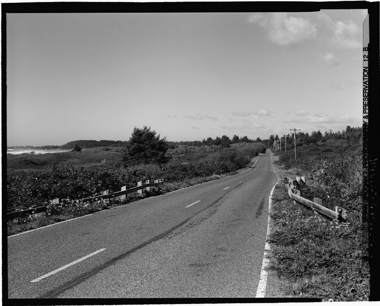
Figure 43. Enderts Beach Road looking north. Although the surrounding grade is somewhat obscured by the invasive Himalayan Blackberry, the causeway is about six feet above the adjoining former farm fields. Crescent Beach and the Pacific Ocean can be seen to the left. The wood guard rails above the culvert are not historic and no longer exist. (Leach and Grogon, HAER 2001).
