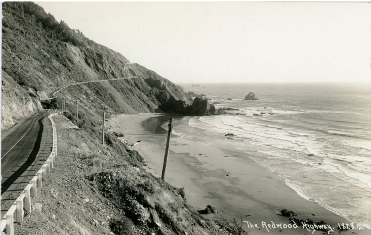
Figure 23. View of coastal section of Old Redwood Highway, possibly south of Crescent Beach Overlook and north of Nickel Creek. The photograph probably dates from the 1930s. The only apparent improvements to the original road are the asphalt surface and the wooden guardrail. Compare Figure 10 from the 1920s. [Humboldt State University Library, Special Collections, Tim McKay Coll., 2007.02.2084.]
