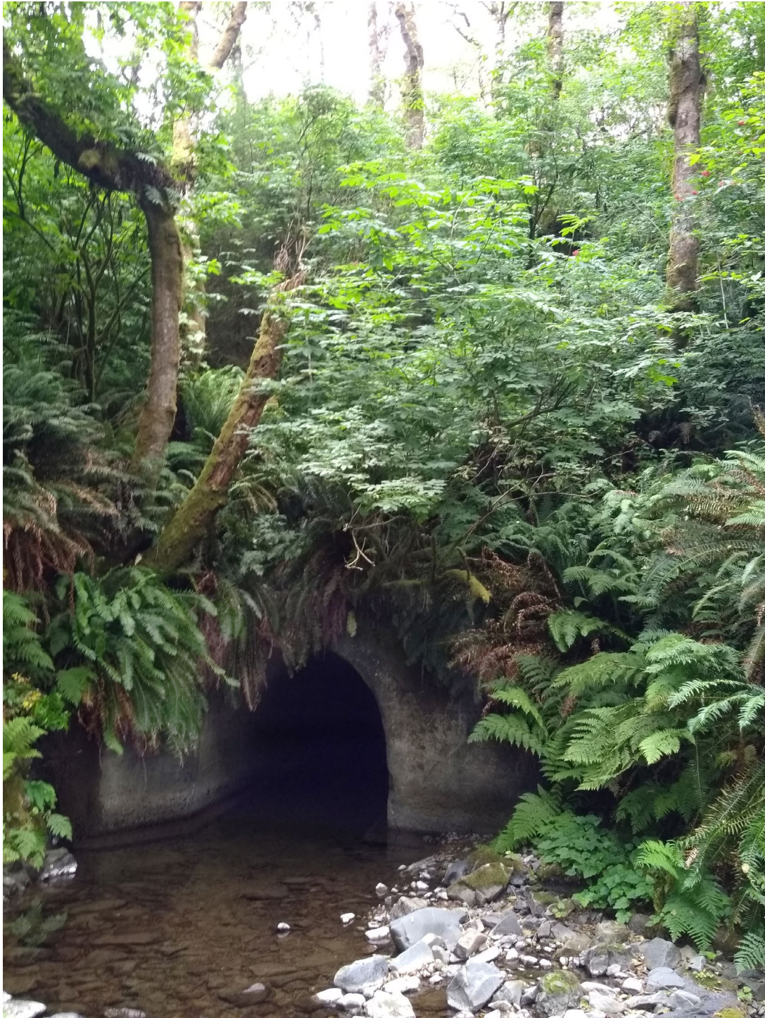
Figure 66. Largest contributing culvert on Old Redwood Highway at Nickel Creek. Although also made of concrete, the size and design make it a distinct type from the concrete box. Current trail level approximately 30 feet above (NPS 2018).
