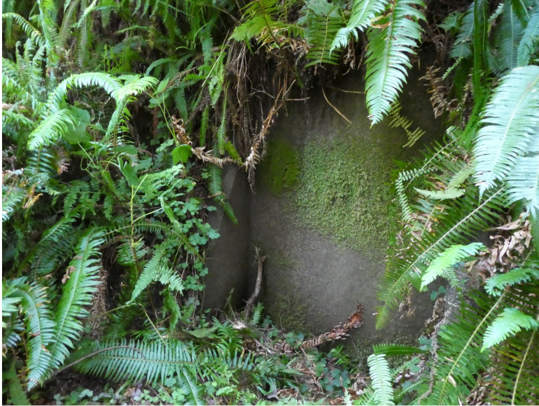
Figure 63. Typical steel pipe with retaining wall type culvert found along the Old Redwood Highway on the Coastal Trail Damnation Creek Section. The uphill side of many culverts have a narrow retaining wall a short distance from the pipe opening (NPS 2017).
