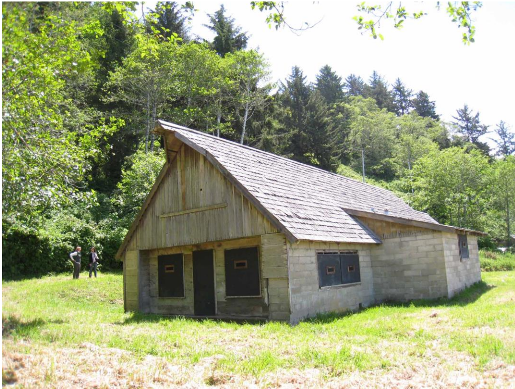
Operations Building, looking southeast (PWR, CL Program, 2012).
