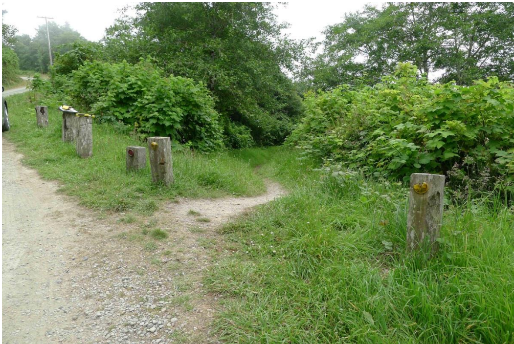
Non-contributing bollards located at entrance to site, looking southwest (PWR CL Program, 2012).
