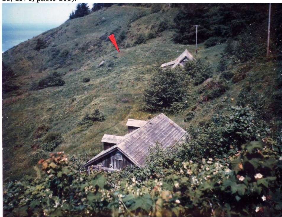
Photo of station, looking north, indicating location of a machine gun pit (REDW Museum Collection, Maintenance Division, Buildings and Utilities, Historic Preservation Files, Catalog No. REDW33659, May 18, 1978, photo 10c).
