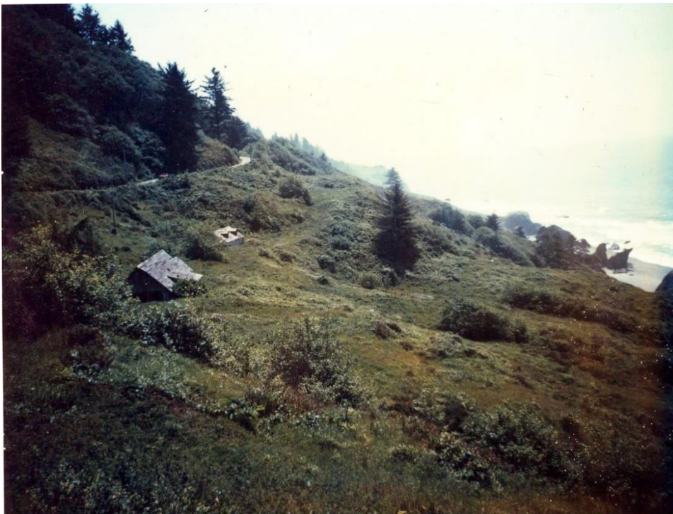
Radar Station, looking south. Note sparse vegetation along entire slope, and mud flow that encroached upon the Power Building, center (REDW Museum Collection, Maintenance Division, Buildings and Utilities, Historic Preservation Files, Catalog No. REDW33659 , May 18, 1978, photo 10a).
