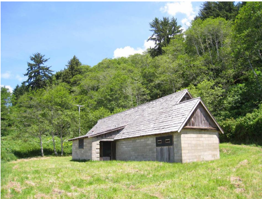
Natural Systems and Features #2: View looking north with the leveled bench used for the antenna field in the foreground, to the left of the Operations Building. The alder forest, located along the upper slopes of the hill, is visible in the background (PWR CL Program 2011).
