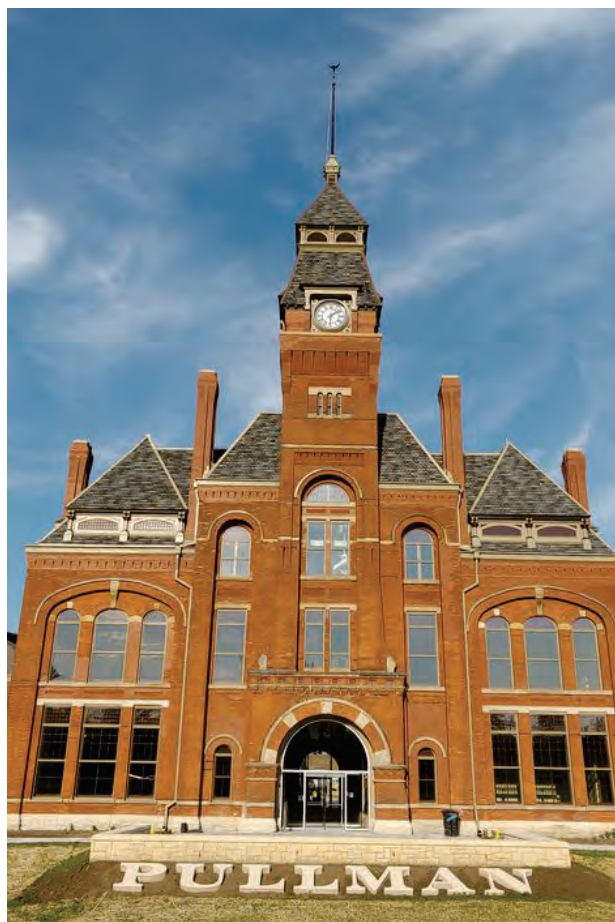
After decades of damage and neglect, the giant clock atop the restored Pullman Administration Clock Tower once again keeps perfect time.
