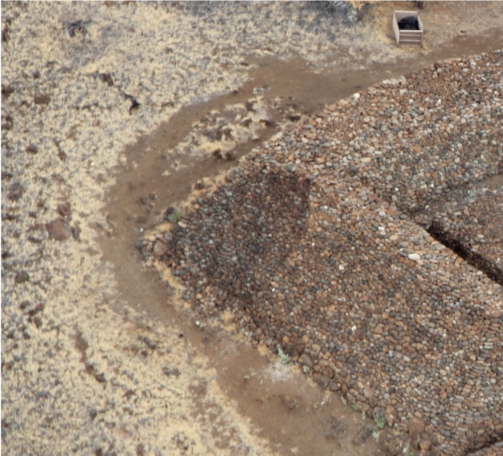
Figure 42. The northeast corner of Pu'ukoholā Heiau. The dark brown stones mark the last original face of the exterior north wall; the lighter sections adjacent to this face have been stabilized (Adam Johnson, personal communication, July 8, 2015).
