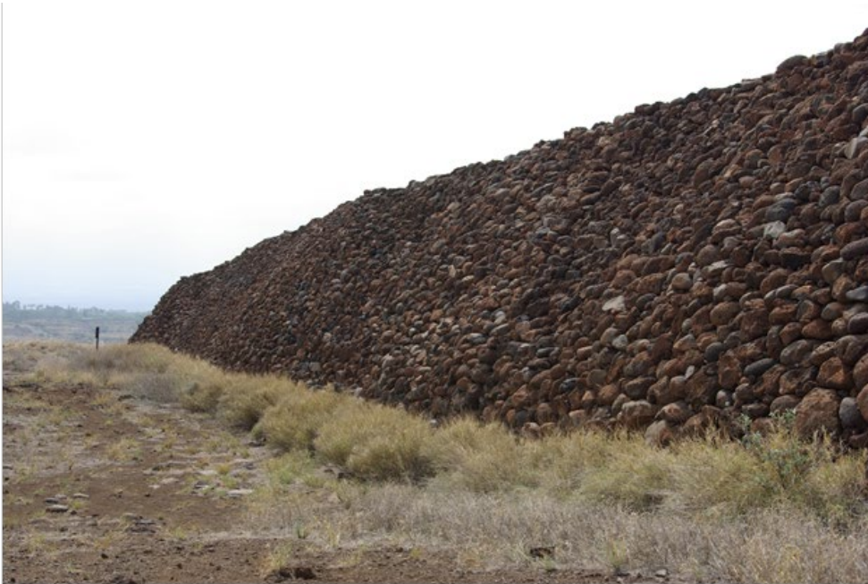
Figure 40. The east wall of Pu'ukoholā Heiau. The vertical bulges in the wall were formed during the 2006 earthquakes. Photograph courtesy of NPS.
