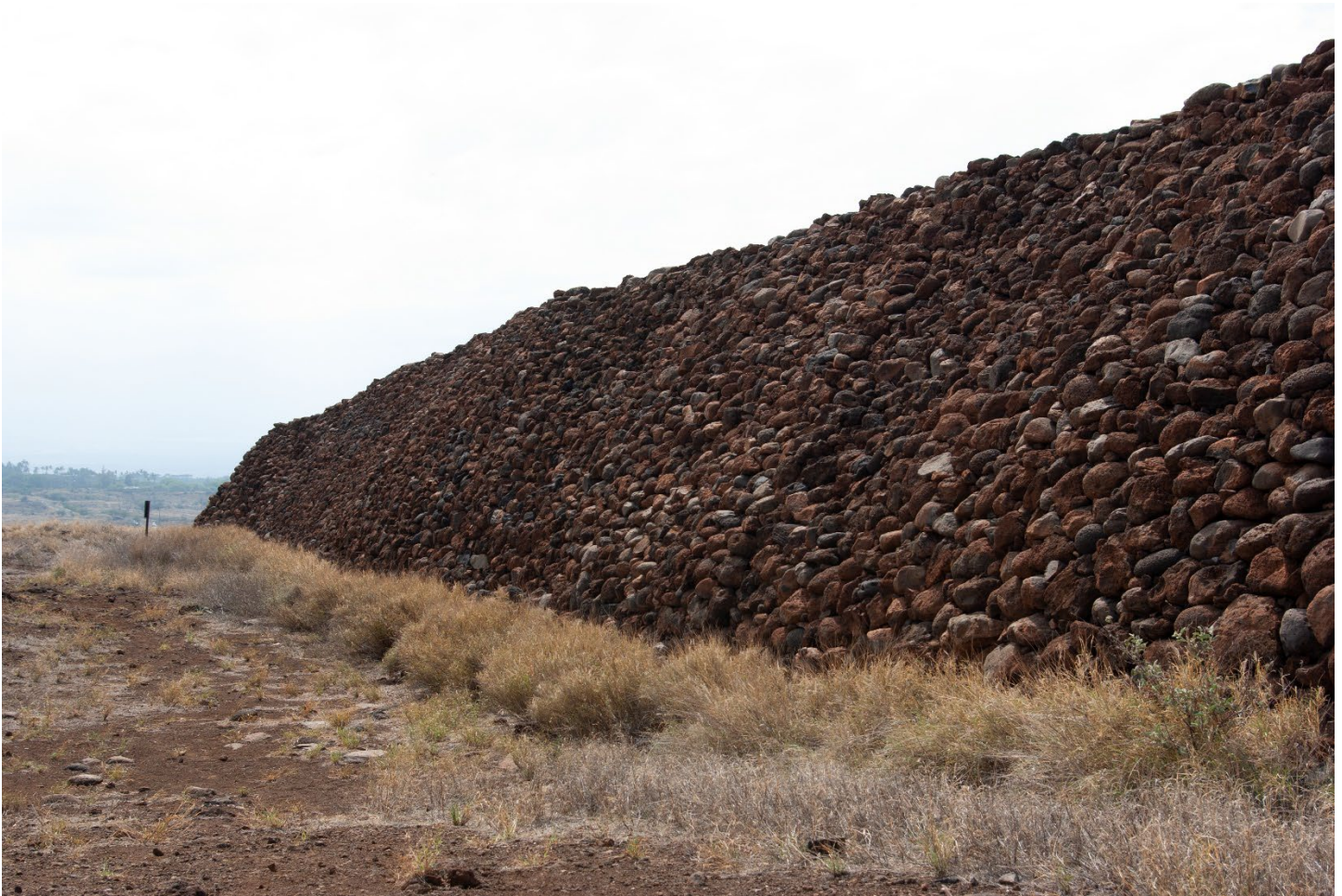
Photo #19 of 81 (HI_Hawaii_Puukohola Heiau NHL_0019)
