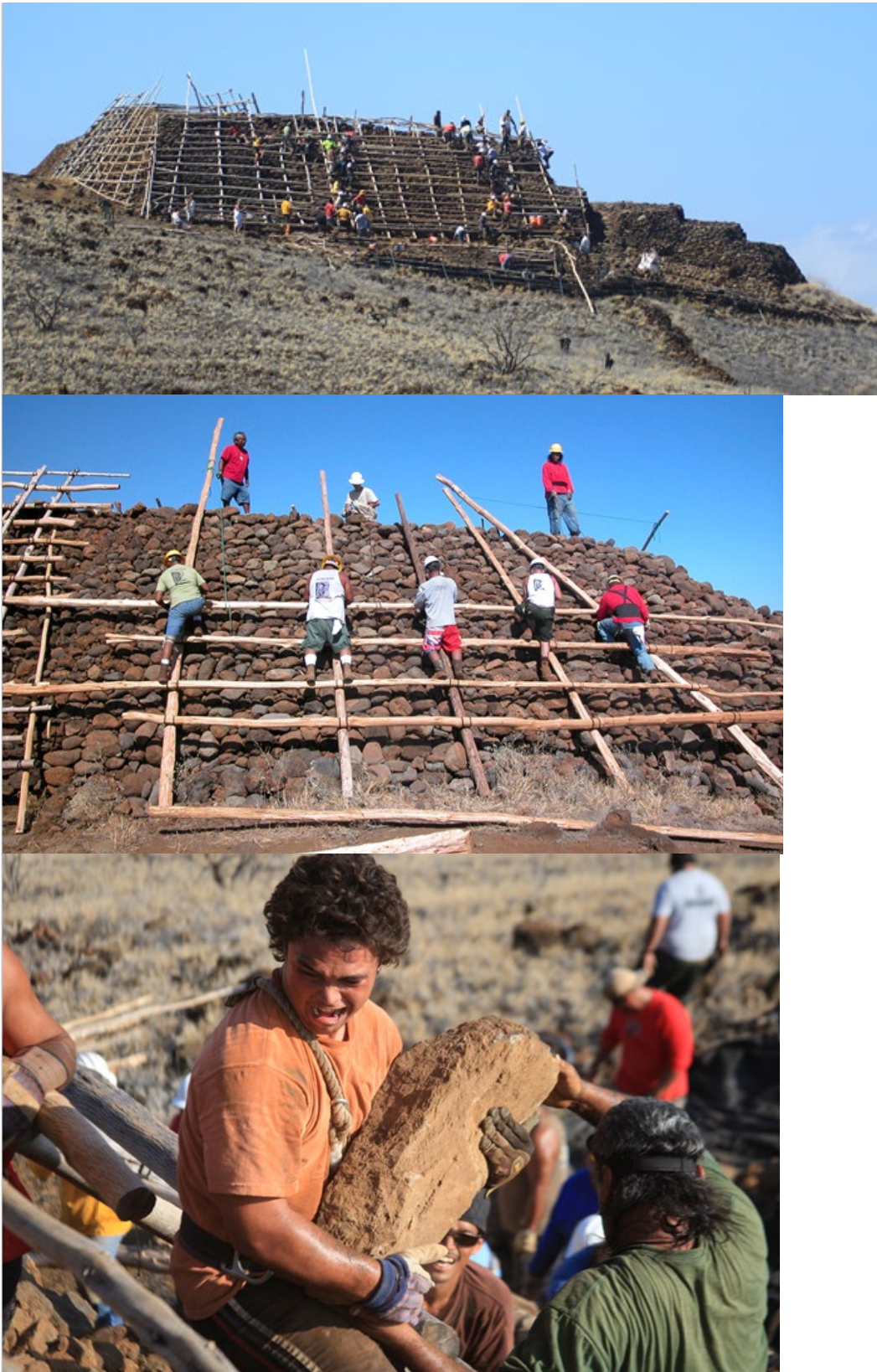
Figure 41. Emergency stabilization efforts at Pu'ukoholā Heiau following the 2006 earthquakes. Photographs courtesy of NPS.
