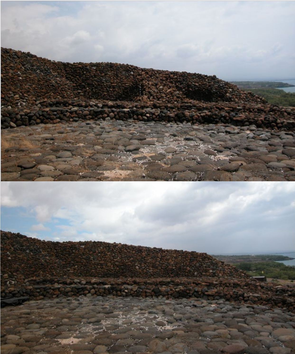
Figure 39. Comparative images of a wall in the southern section of Pu'ukoholā Heiau, showing damage caused by the 2006 earthquakes (top), and repairs completed during emergency stabilization efforts (bottom). Photographs courtesy of NPS.
