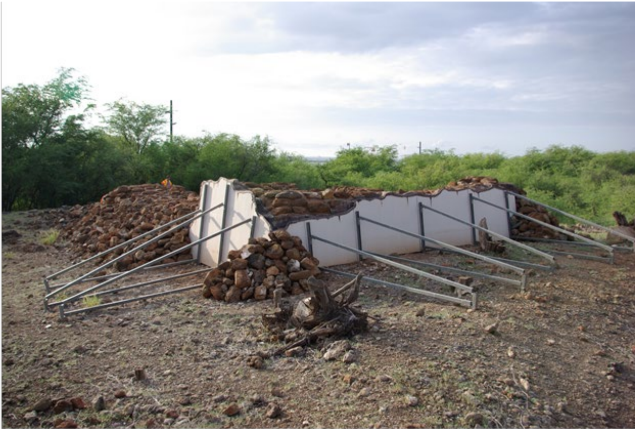
Figure 43. John Young's primary residence at the John Young Homestead. Steel bracers and cement board siding protect original portions of the eastern and southern walls from the weather. View to the northwest.
