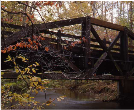
The CCC-built bridge along Scenic Drive is one of the most beautiful spots along the 11 mile road. NPS Photo.
