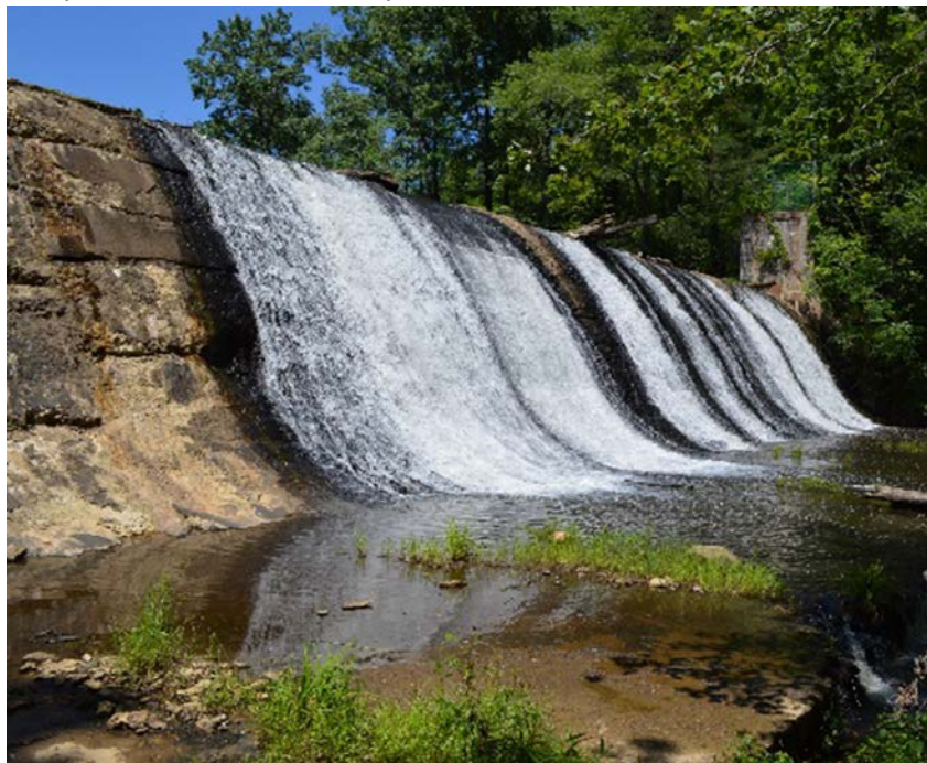
Figure 36: This historic concrete dam (CRIS-HS# 997876), built by the CCC, services the lake for Cabin Camp 2 (it is sited outside the Cabin Camp 2 CLI boundary adjacent to Cabin Camp 5) (UPenn 2023).
