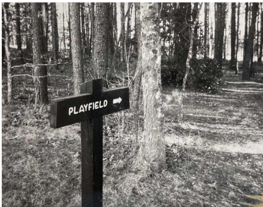
Figure 40: This Mission 66-era sign at an unknown camp employed the historic aesthetics of Rustic-style design, but featured angled edges and was constructed using dimensional lumber (PRWI Collections 2226).
