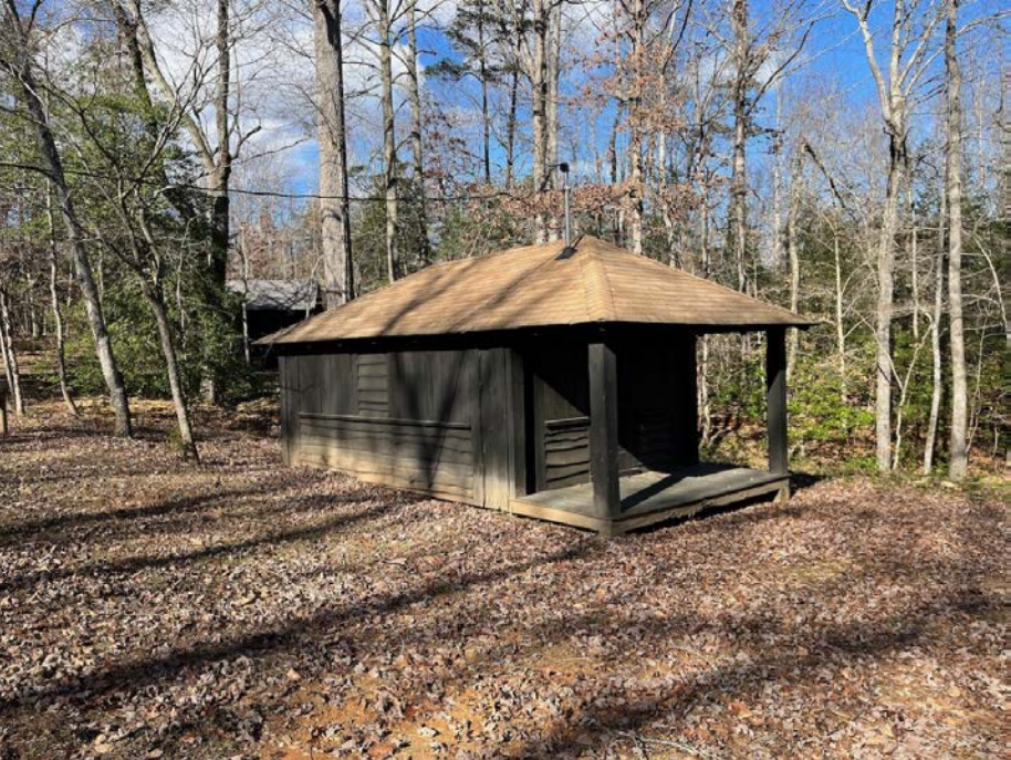
Figure 32: Type B cabins, such as these in Camp 2, are elongated in plan, featuring end-gables or hipped roofs (UPenn 2023).
