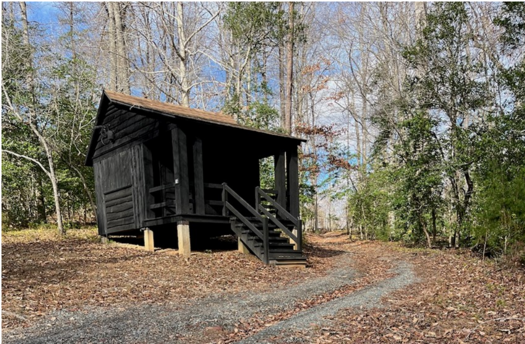
Figure 19: When constructing building and structures, the CCC seldom manipulated the natural topography; rather, buildings and structures were placed on footings that allowed them to respond to the topography. (UPenn 2023)
