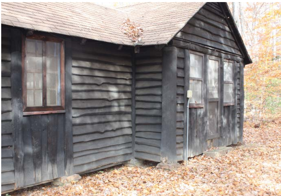
Feature Name: Building 1-50, Administration Building rear Direction: South West
