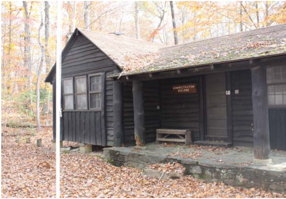
Feature Name: Building 1-50, Administration Building Direction: South East CLI Feature Number: 148773 LCS ID Number: 45270 FMSS: 16413
