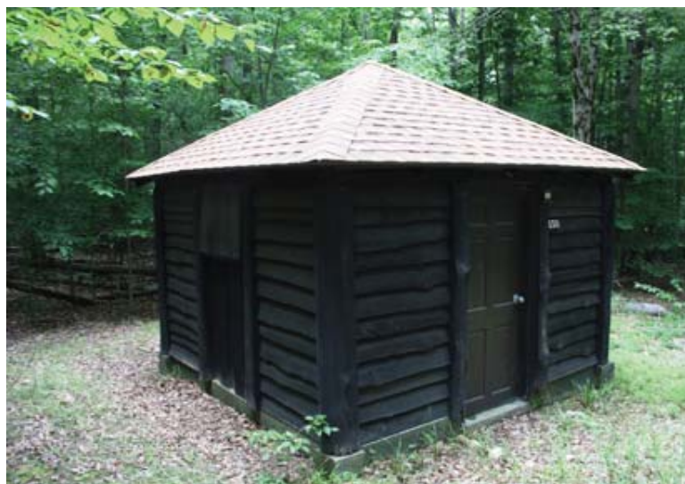
Feature Name: Building 1-330, Pump House,(from 2014 LCS Survey Direction: South CLI Feature Number: 148787 LCS ID Number: 5359 FMSS: 35540
