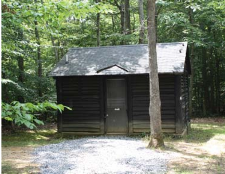
Feature Name: A-10 Latrine ,(from 2014 LCS Survey Direction: South CLI Feature Number: 148759 LCS ID Number: 1003427 FMSS: 16432
