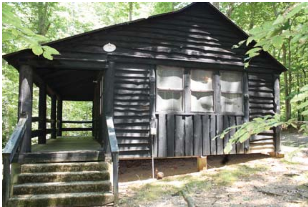
Feature Name: Building 1-65 Staff Quarters,(from 2014 LCS Survey Direction: South CLI Feature Number: 148785 LCS ID Number: 45261 FMSS: 35659
