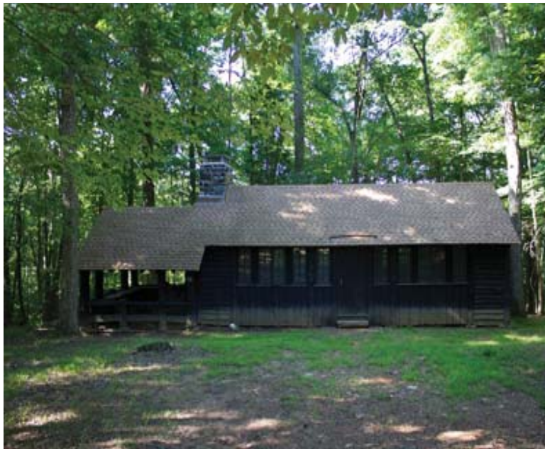
Feature Name: C-12 Lodge ,(from 2014 LCS Survey Direction: South West CLI Feature Number: 178573 LCS ID Number: 1003425 FMSS: 16452
