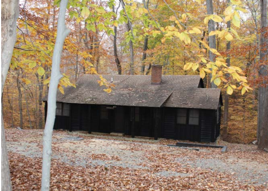
Feature Name: Building 1-70, Infirmary
