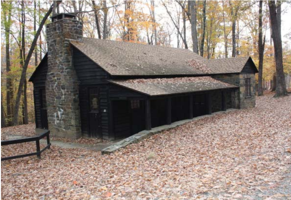
Feature Name: Building 1-55, Craft Lodge Direction: South East CLI Feature Number: 148763 LCS ID Number: 45265 FMSS: 16414
