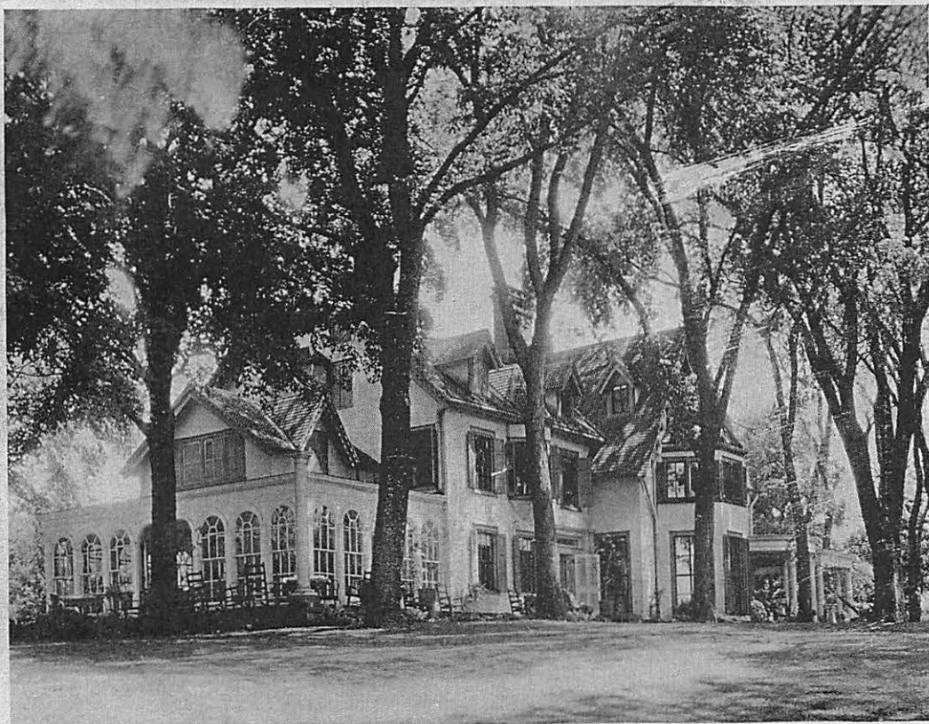
SOUTH VIEW OF THE RINGWOOD HOUSE SHOWING FRONT TERRACE AND TREES PLANTED IN HONOR OF PEACE OF GHENT BY MRS. RYERSON.
